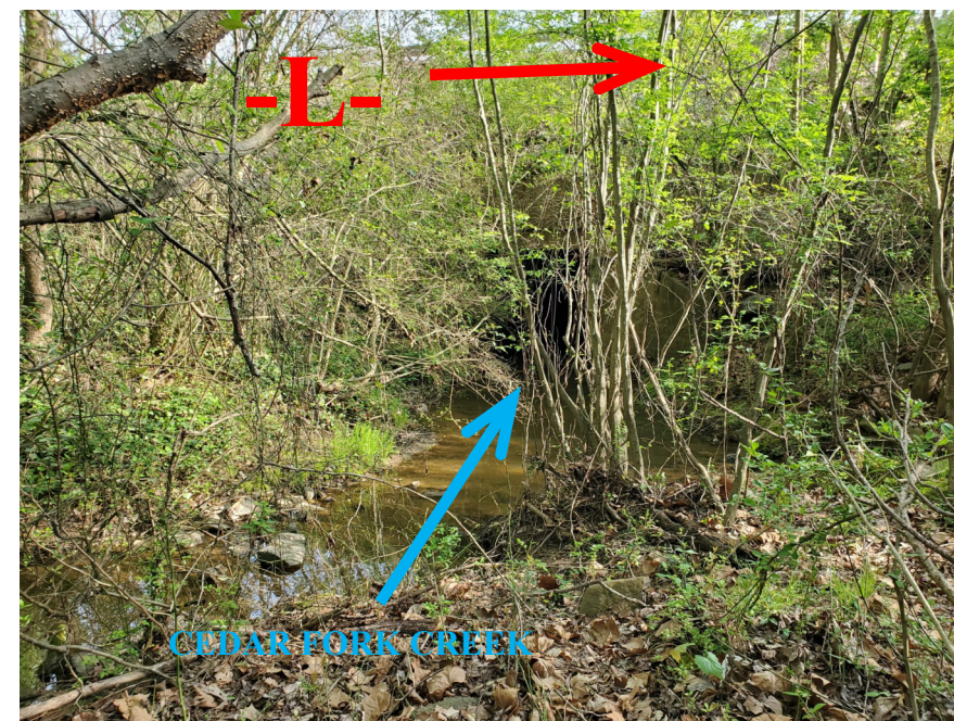
Looking North at the Upstream Inlet of Culvert
