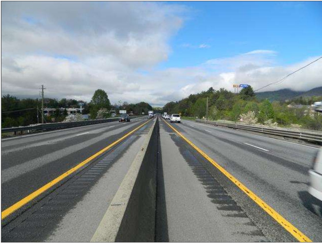
EAST APPROACH LOOKING WEST
