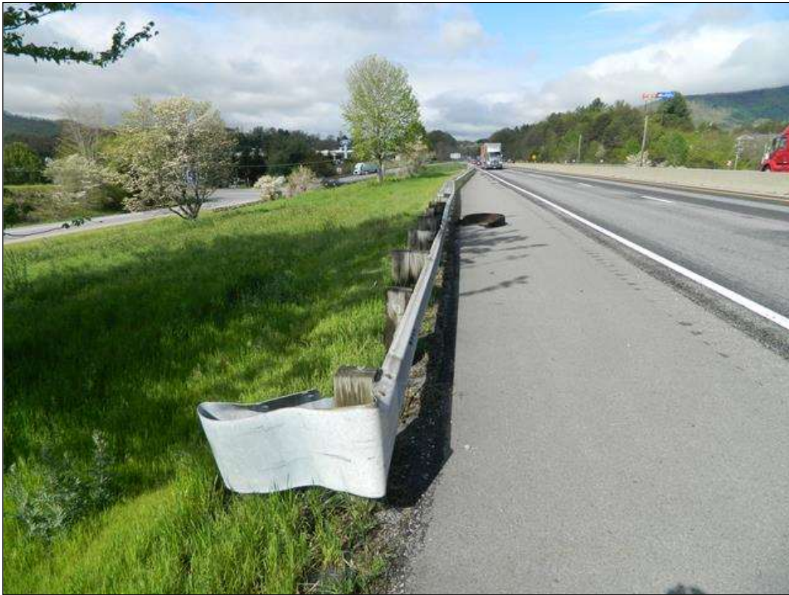
GUARD RAIL END AT THE SOUTH EAST CORNER OF THE BRIDGE.
