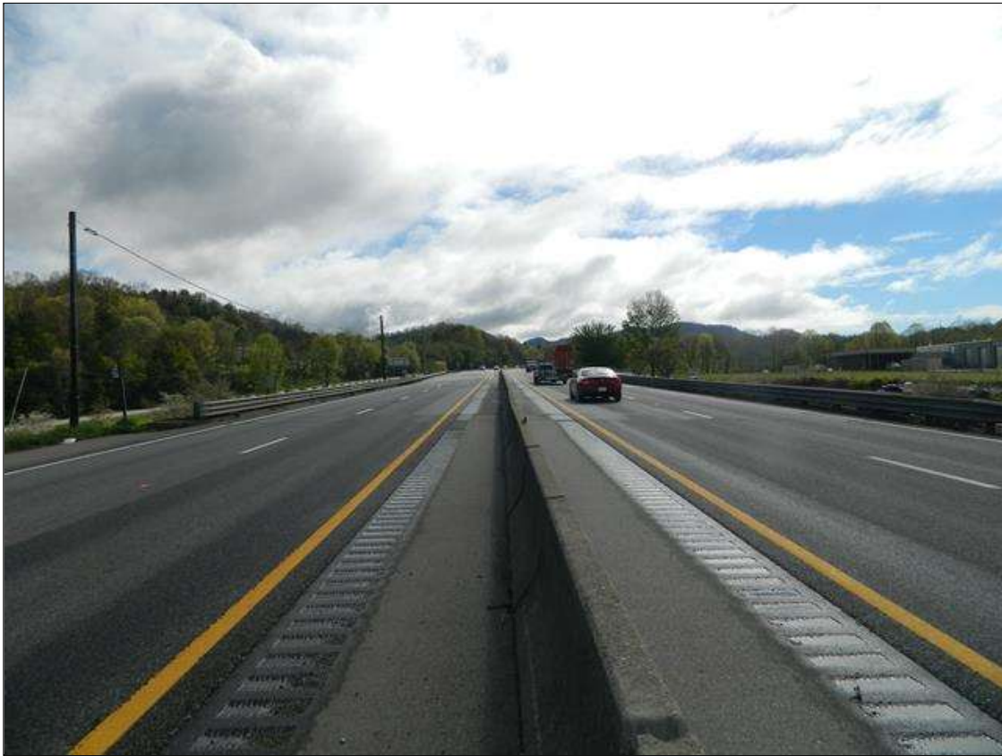
WEST APPROACH LOOKING EAST
