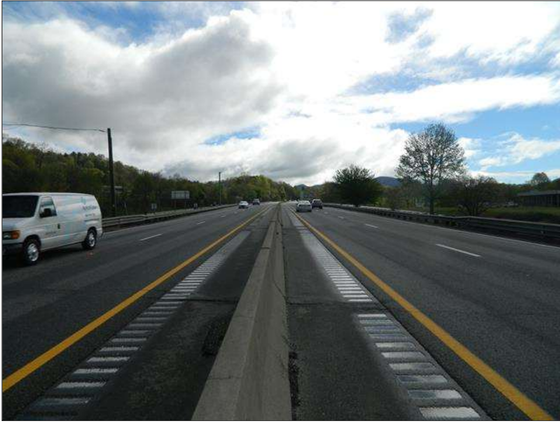
GUARDRAIL LOOKING EAST
