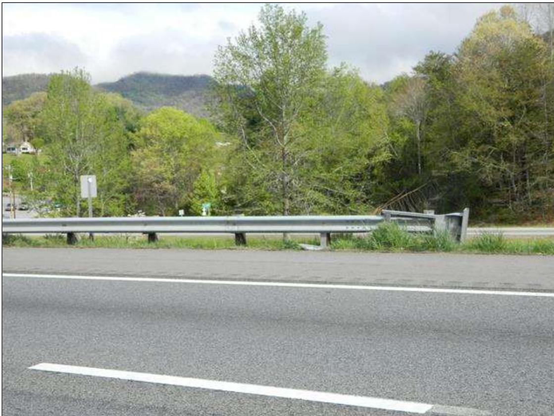
GUARD RAIL END AT THE NORTH EAST AND SOUTH WEST CORNERS OF THE BRIDGE.
