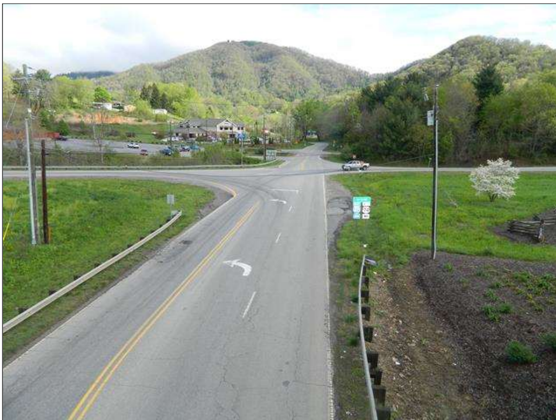
LOOKING NORTH FROM TOP OF STRUCTURE
