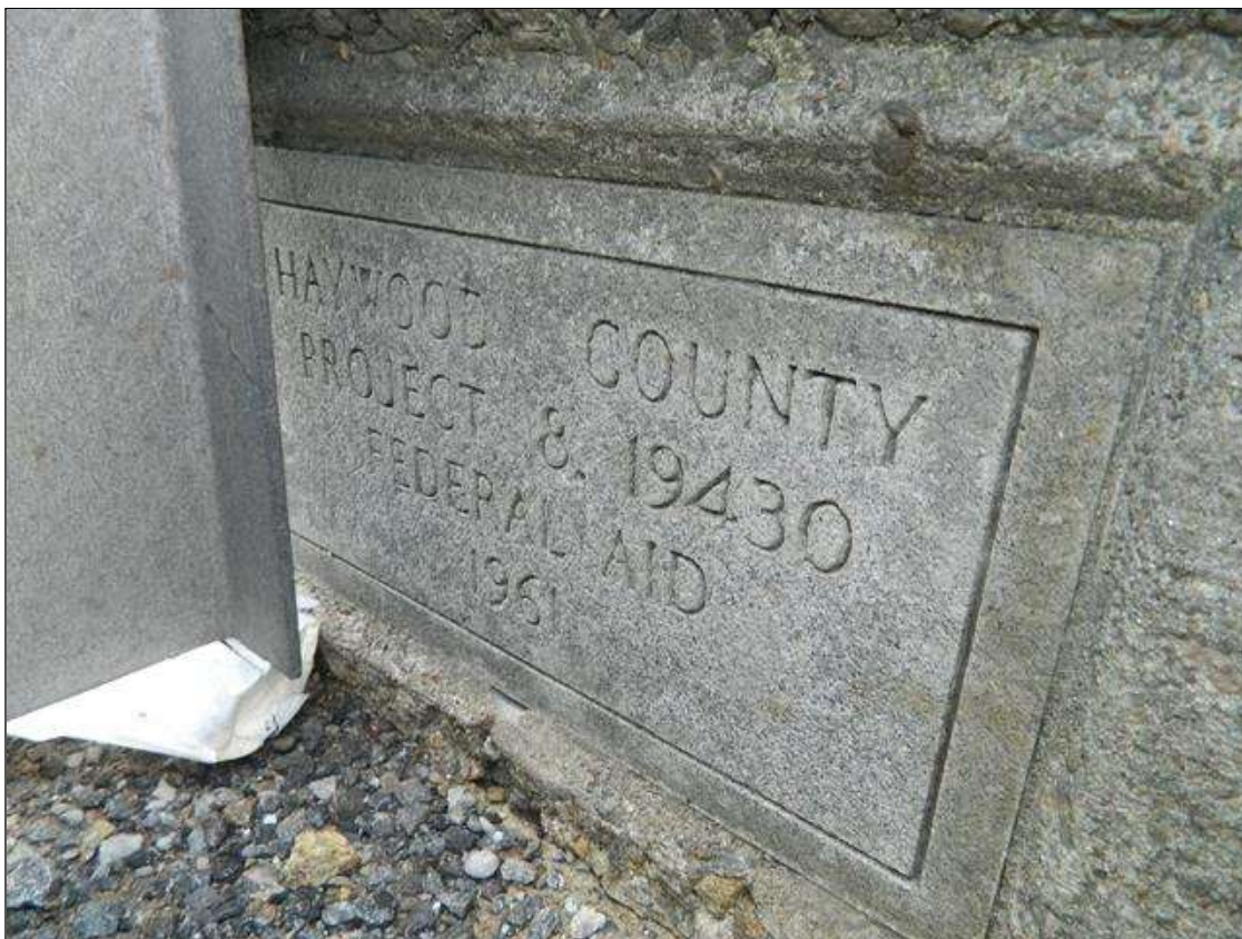
STRUCTURE INFORMATION PLATE AT THE SOUTH WEST AND NORTH EAST CORNERS
