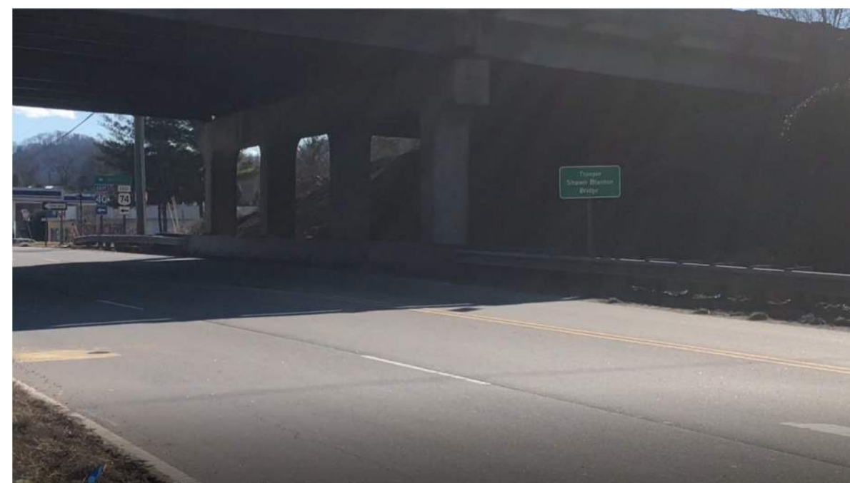
Photo 4: Looking southwest towards End Bent 1 and Bent 1 under Bridge 243
