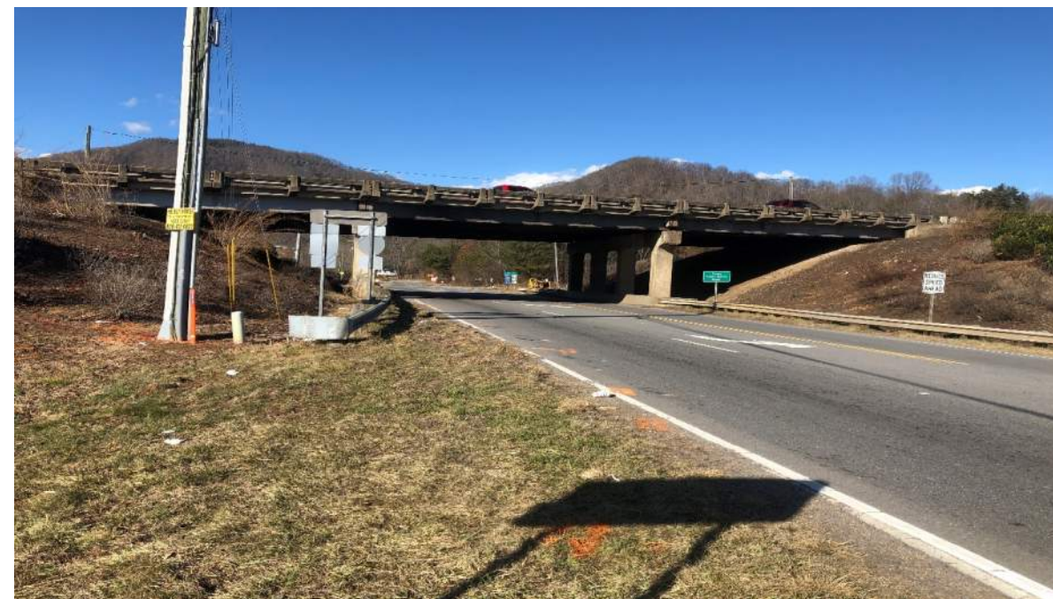
Photo 2: Looking North towards End Bent 2 and Bent 2
