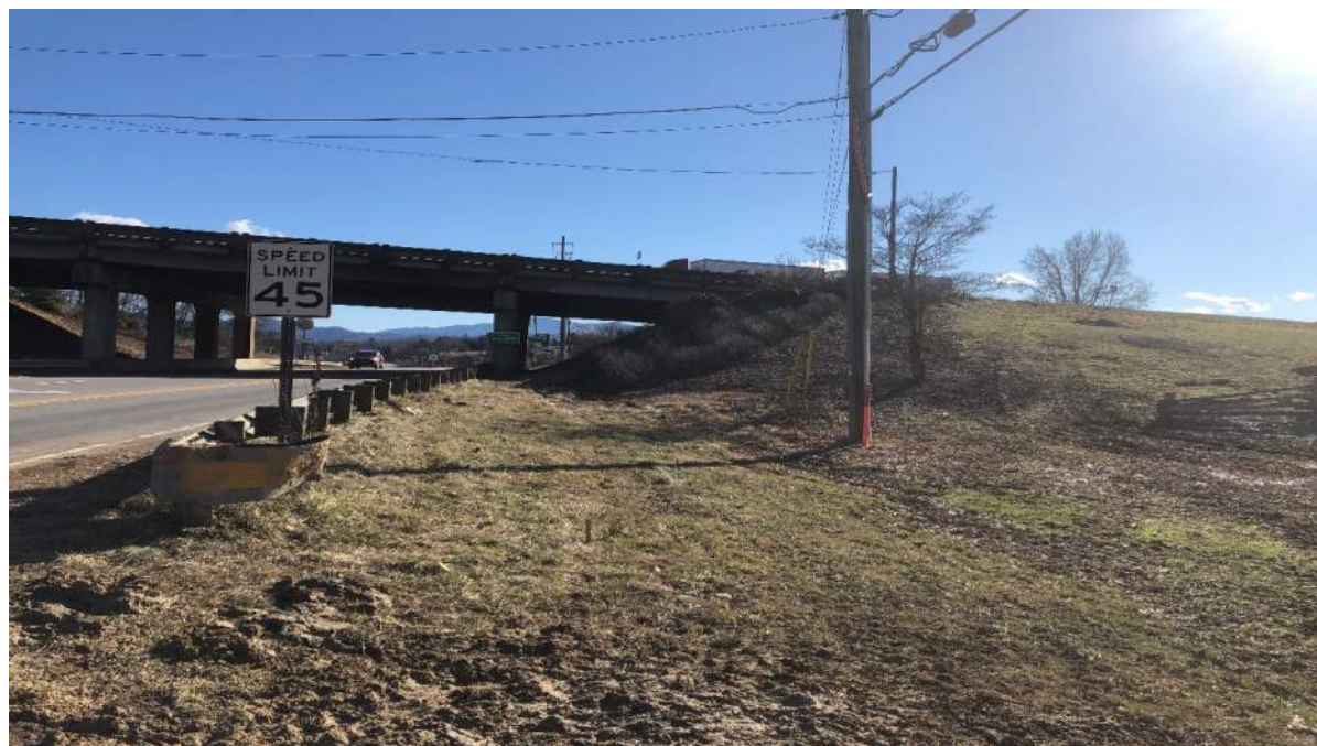
Photo 1: Looking South towards End Bent 1 and Bent 1
