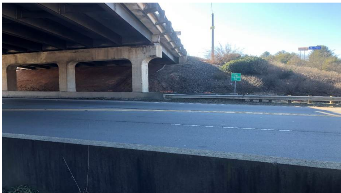
Photo 3: Looking East towards End Bent 2 and Bent 2 under Bridge 243
