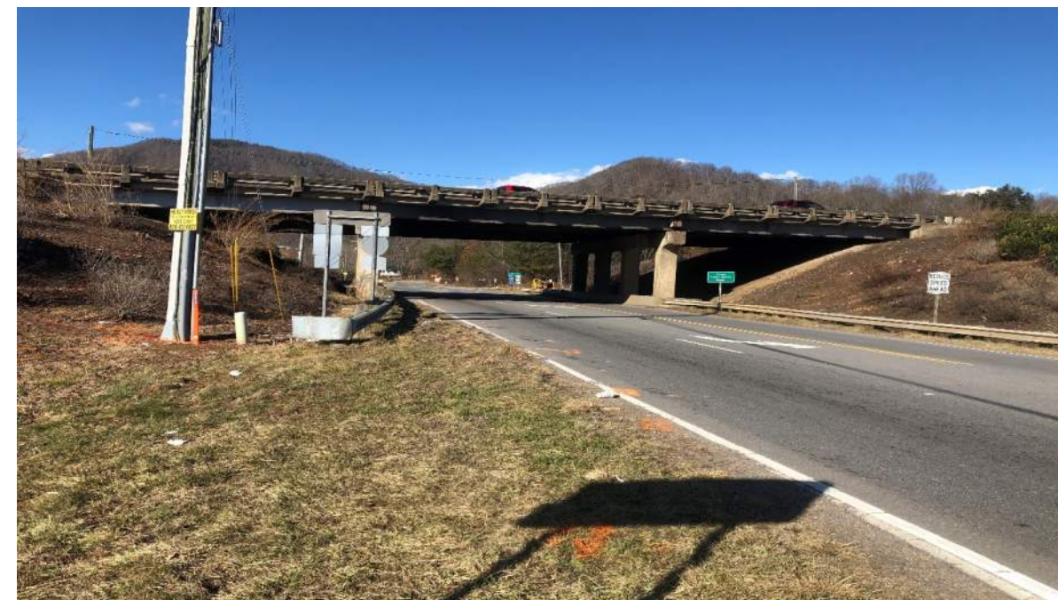
Photo 2: Looking North towards End Bent 2 and Bent 2
