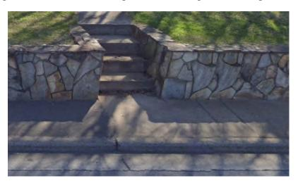
All texture is to be in addition to the nominal thickness of each element within tolerances. Relief of any texture is to have a minimum depth of ½ inch, a maximum depth of 4 inches, and an average of  $2\frac{1}{2}$  inches.
