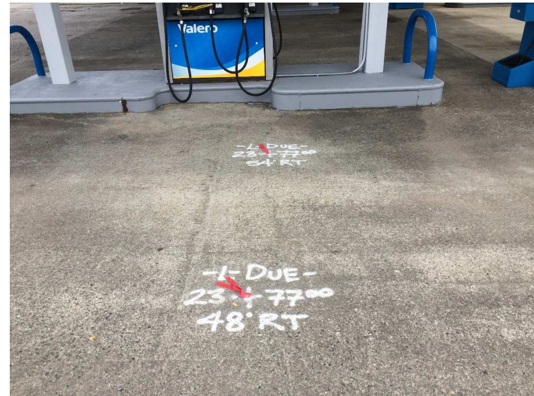
D. Photo of NCDOT easement markings on west side of western pump island.
