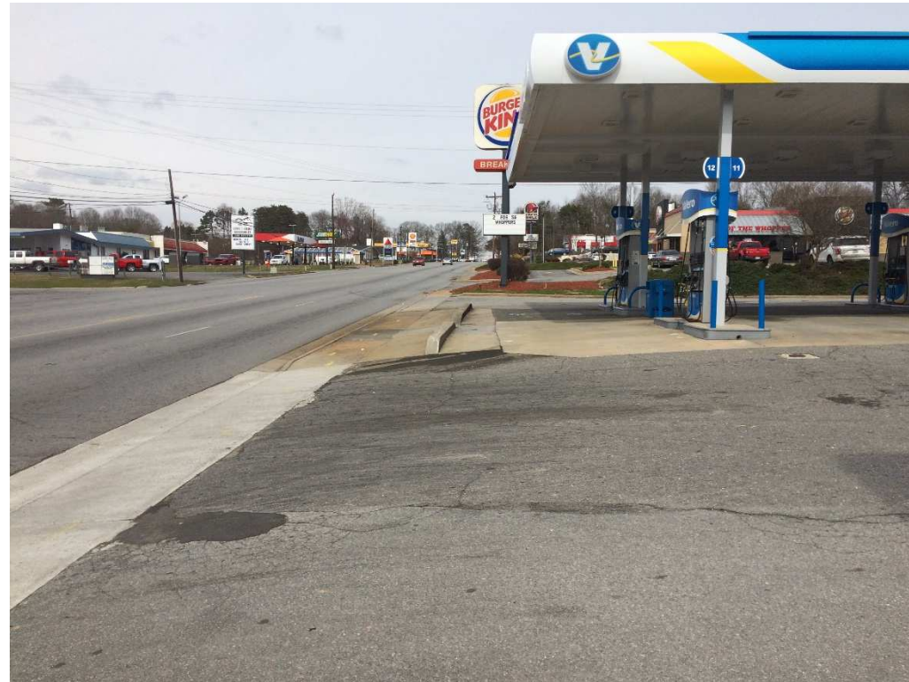
D. Photo of proposed easement area, looking north.
