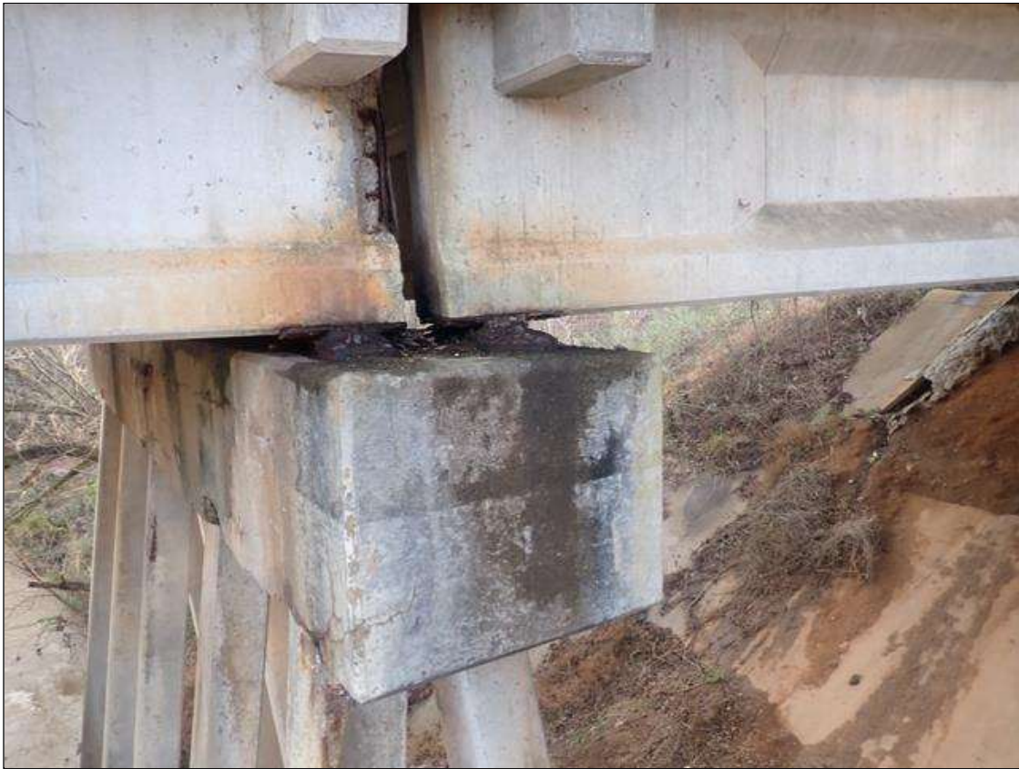
beams over bent 1
