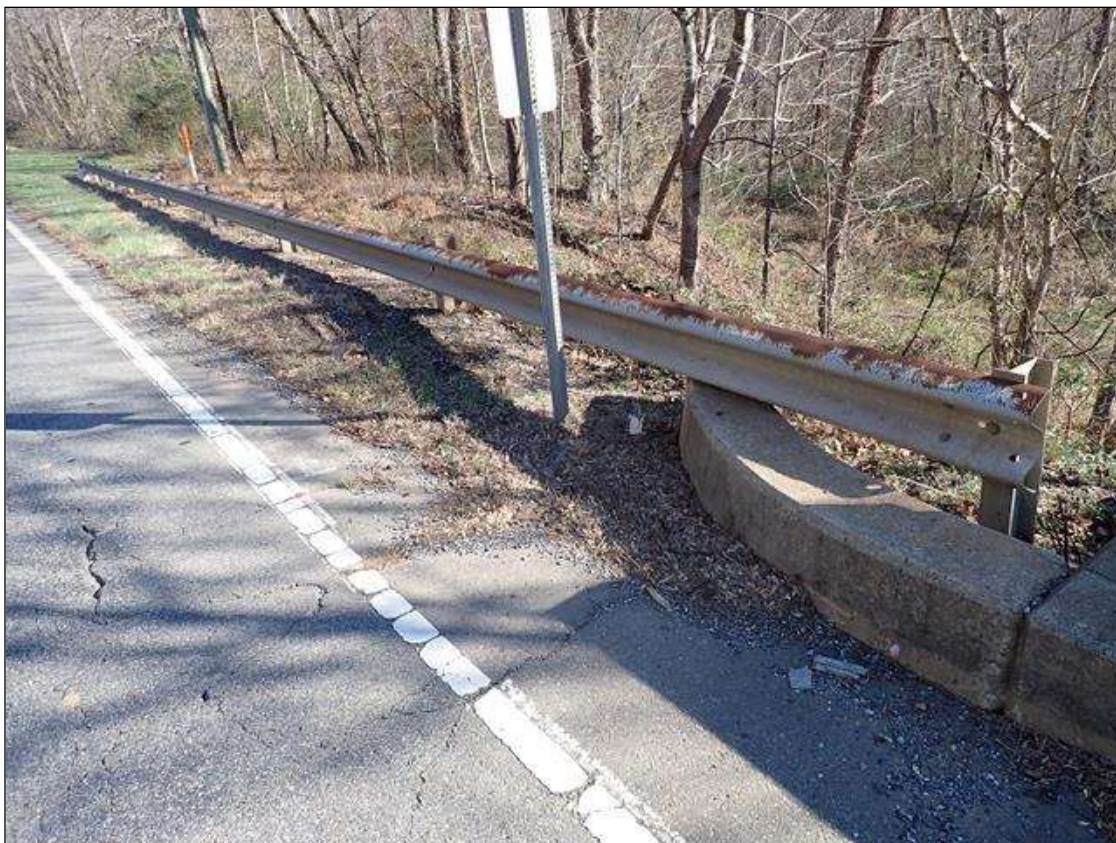
southeast guardrail and post spacing
