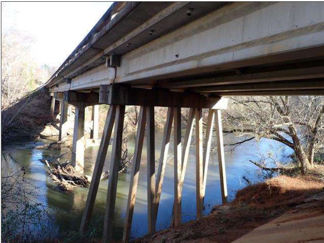
upstream profile looking south
