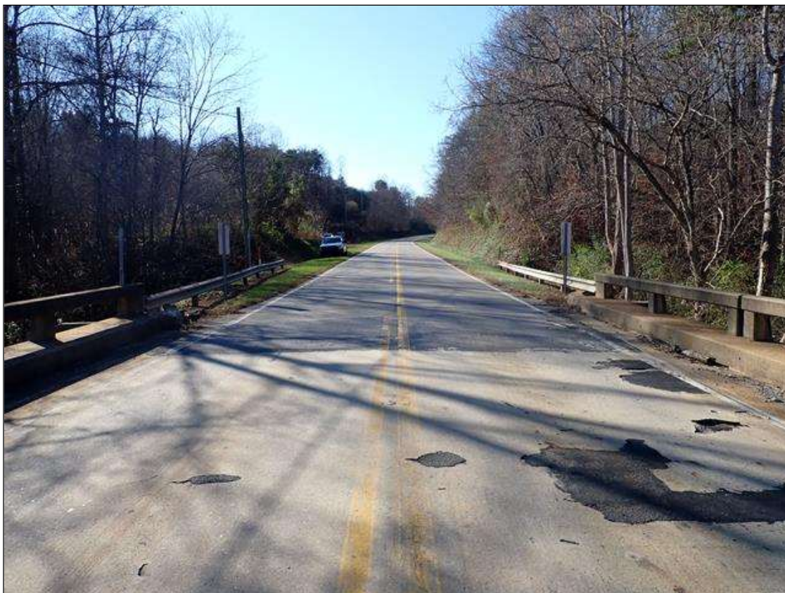
west approach, looking west (backstation)
