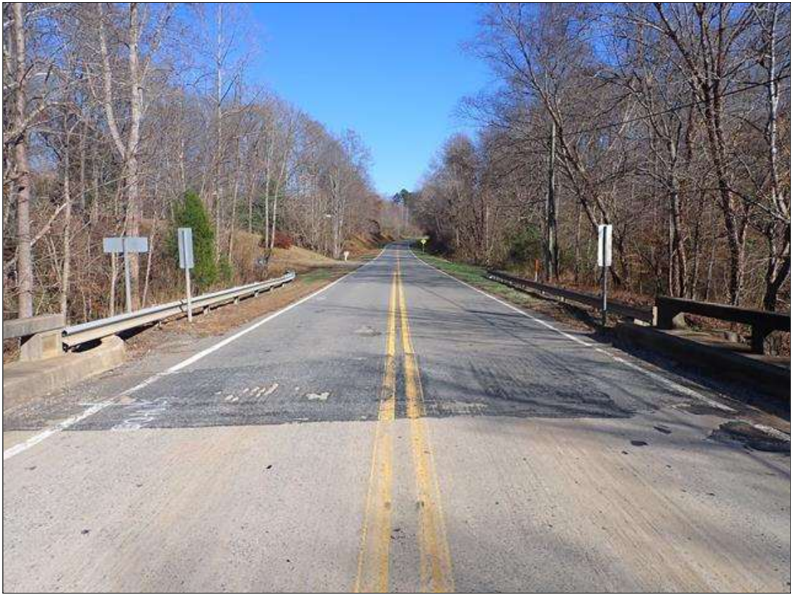
east approach, looking east (upstation)
