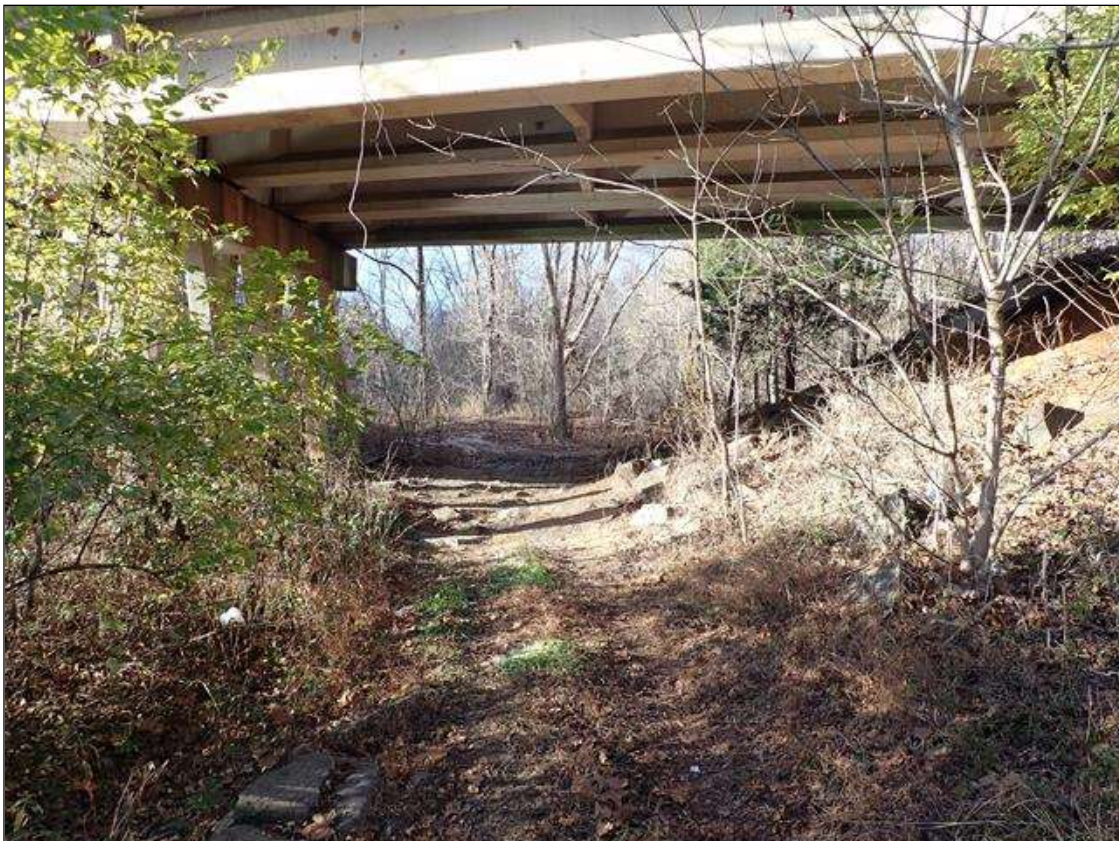
looking north through span 5
