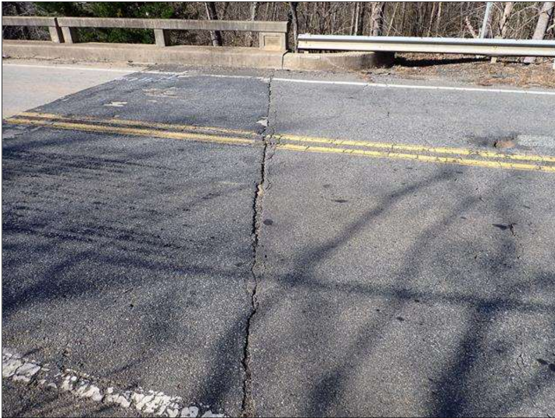
asphalt wearing surface over end bent 2
