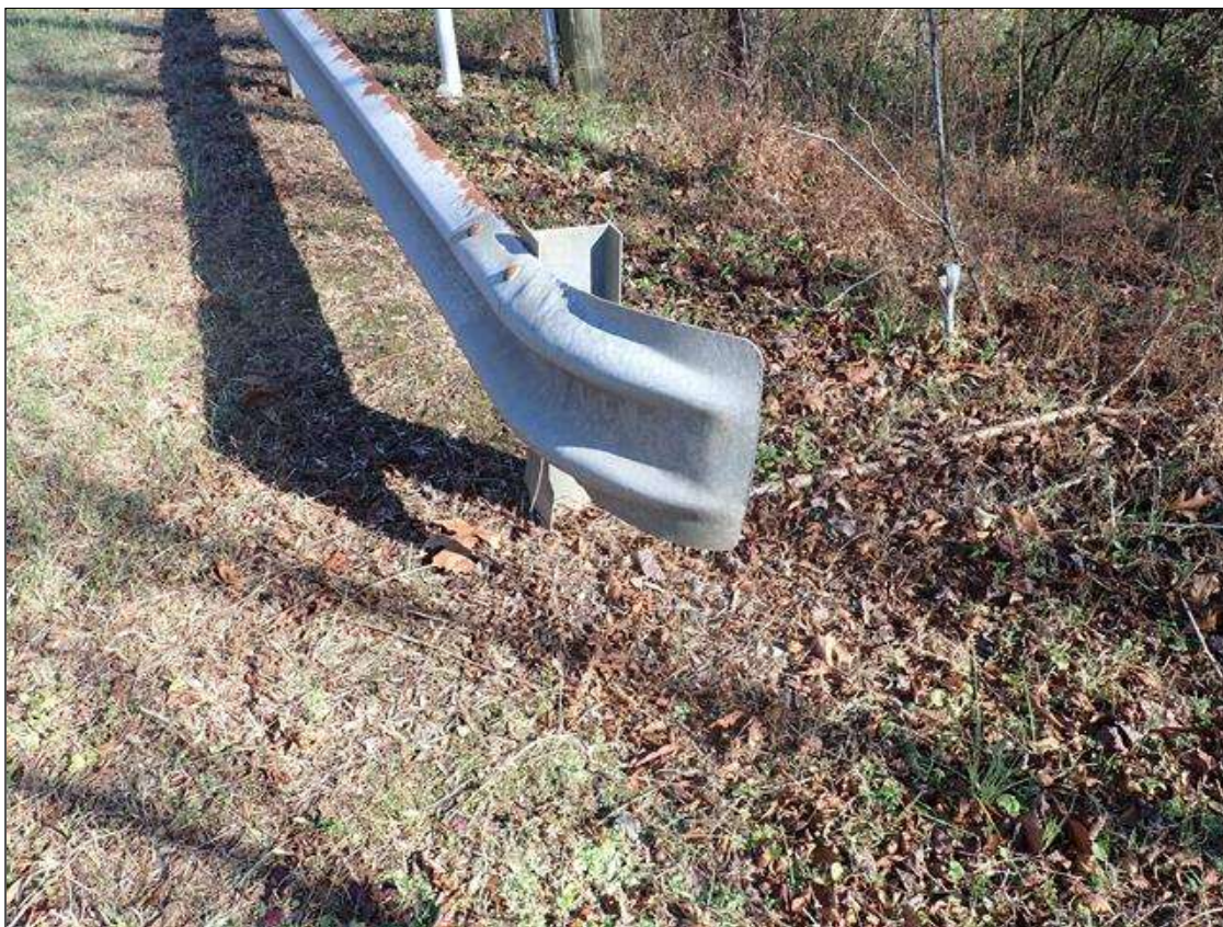
southwest guardrail termination
