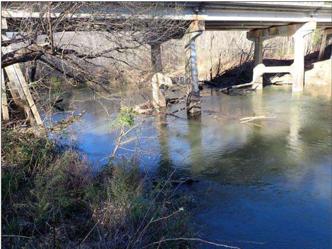
stream underview, looking upstream (north)
