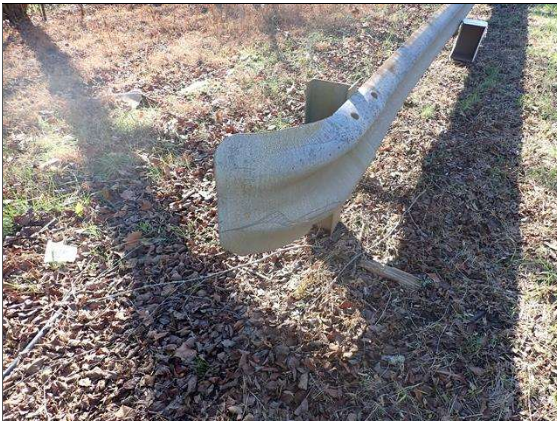
southeast guardrail termination
