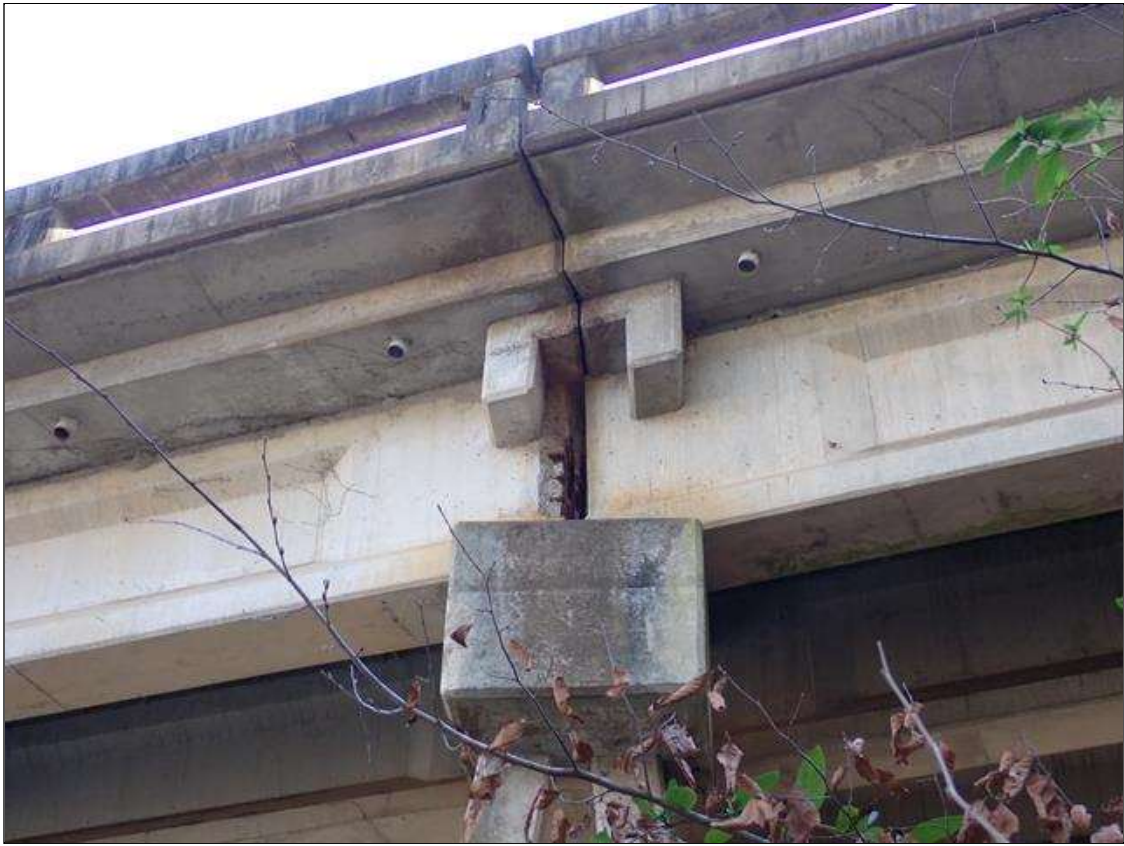
beams over bent 1
