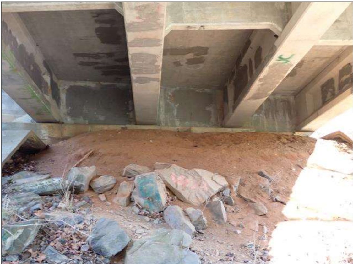
end bent 2 and slope protection
