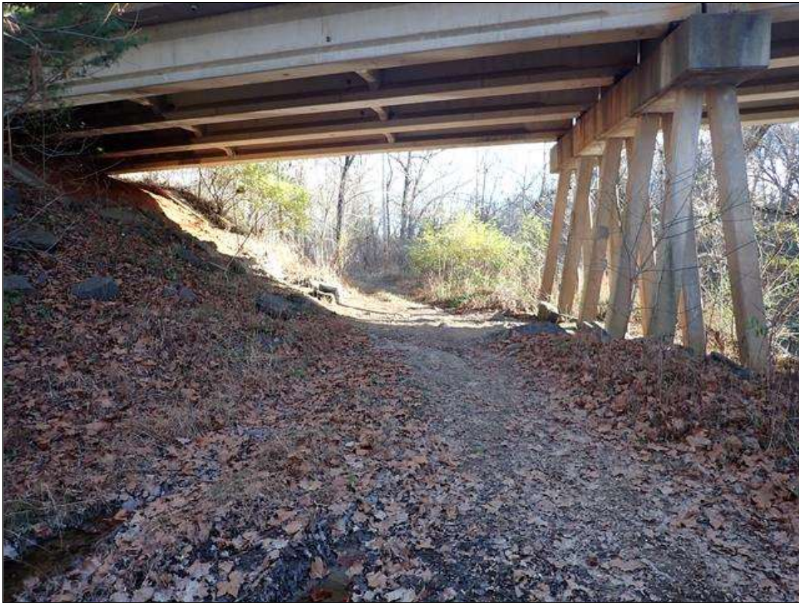
looking south through span 5
