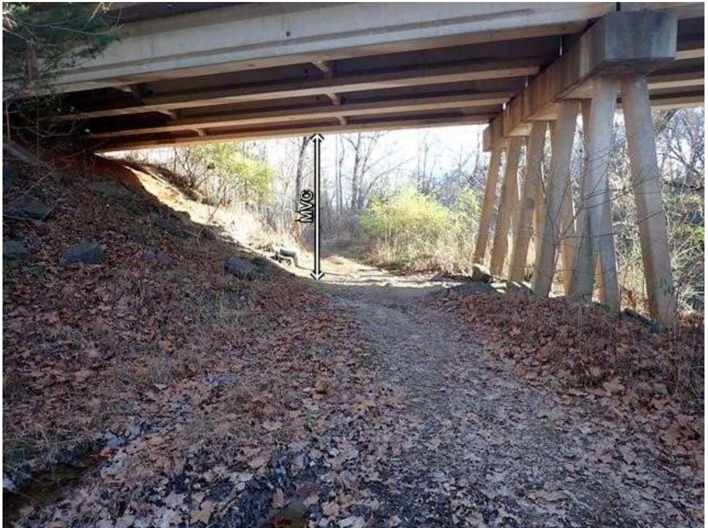
looking south through span 5
