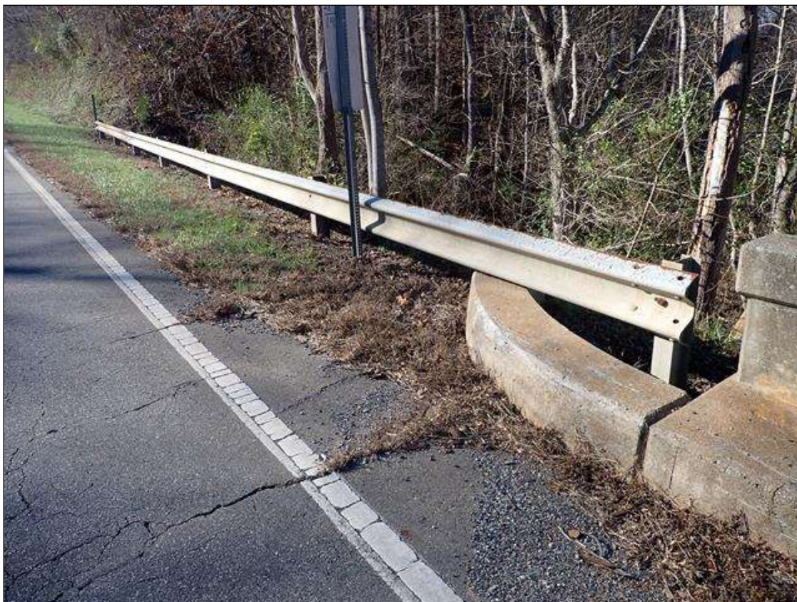
northwest guardrail and post spacing
