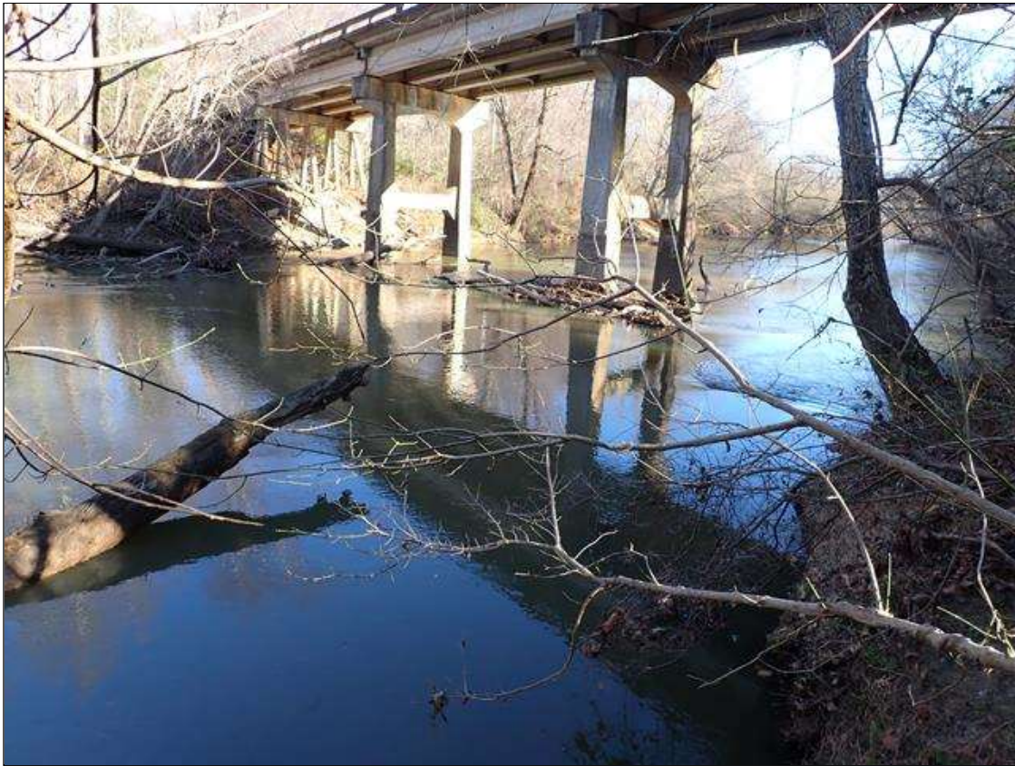
stream under view, looking downstream (south)
