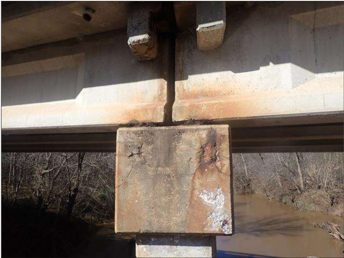
beams over bent 2
