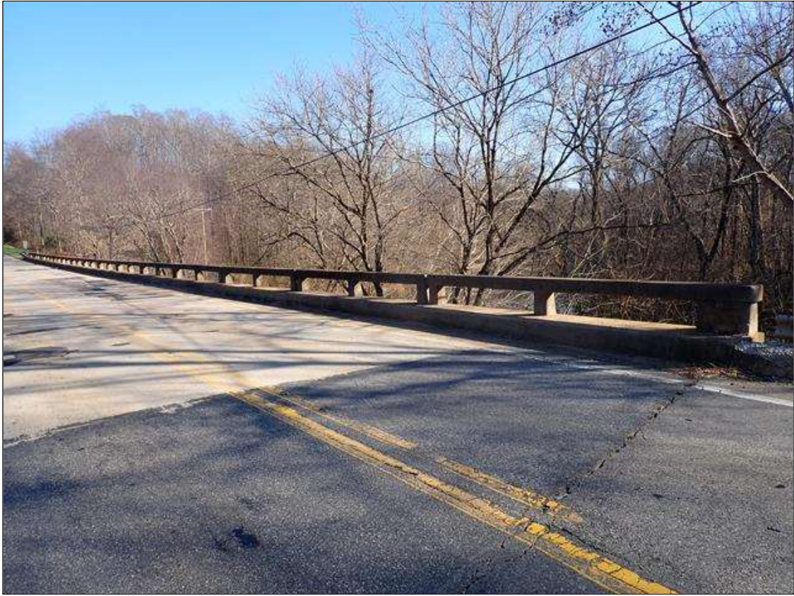
south bridge rail
