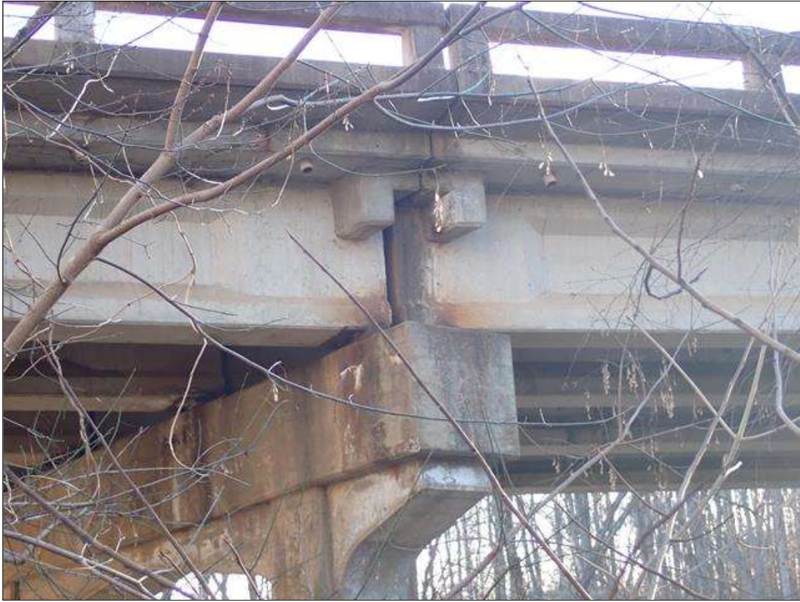
beams over bent 3
