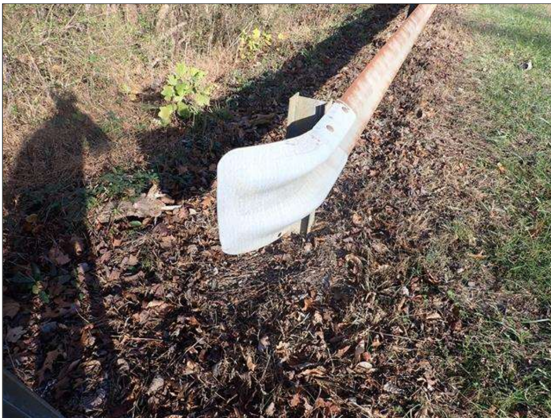
northwest guardrail termination
