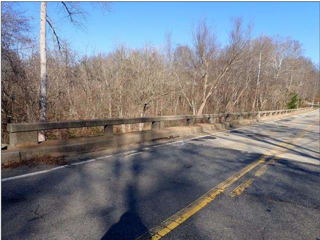
north bridge rail
