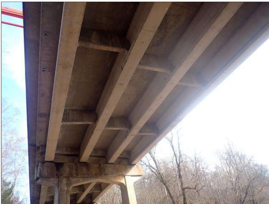
underside of deck
