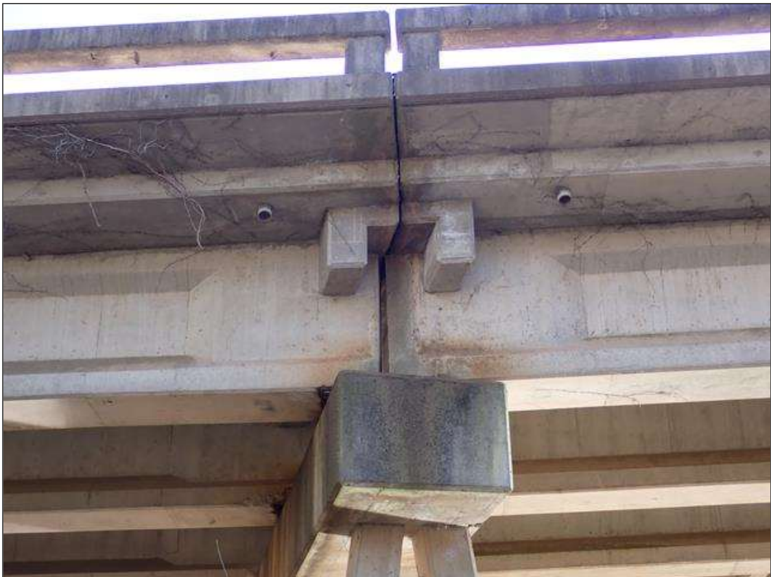
beams over bent 4
