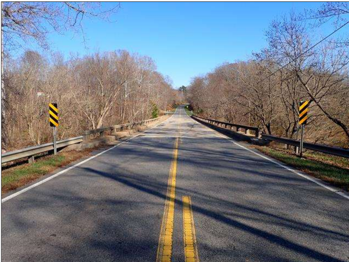
west approach, looking east
