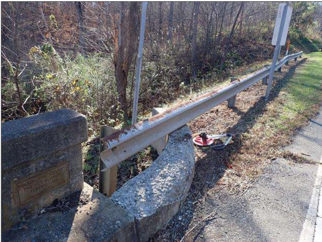
southwest guardrail and post spacing
