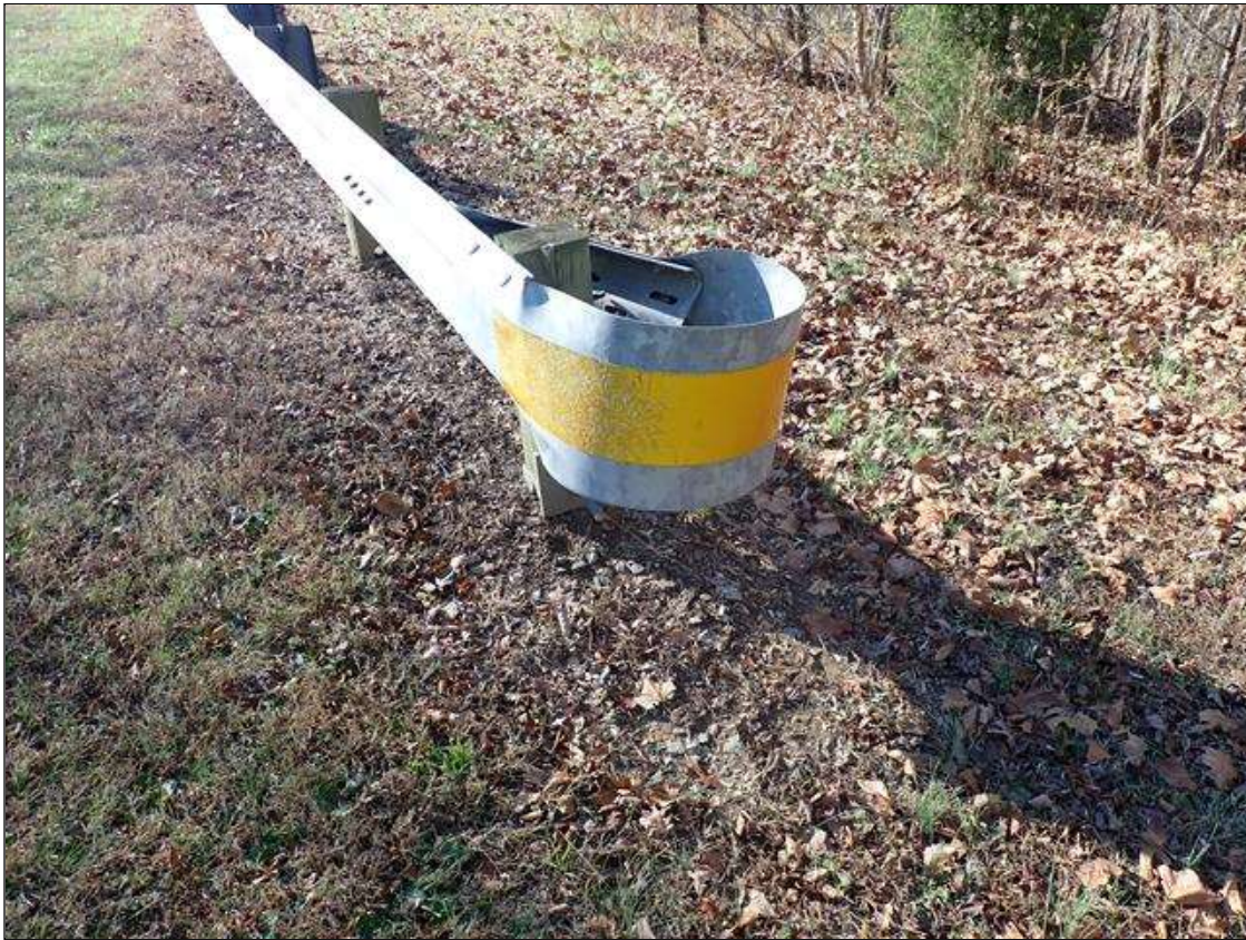
northeast guardrail termination
