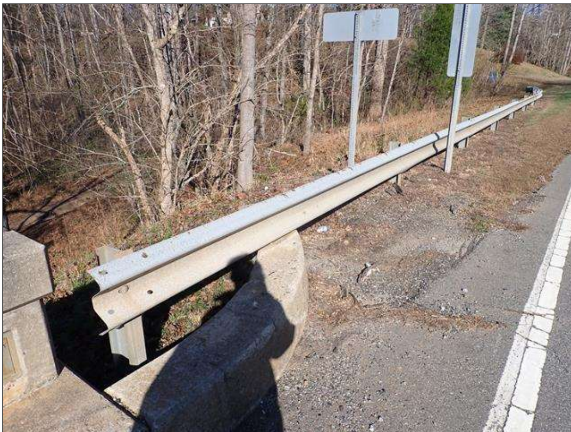
northeast guardrail and post spacing
