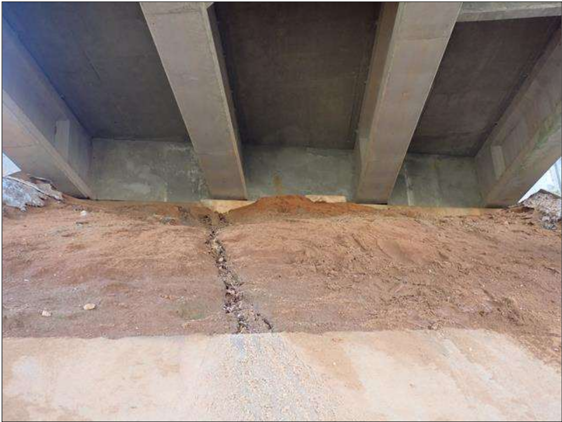
end bent 1 and slope protection
