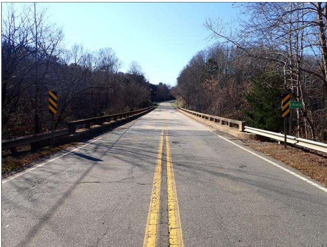
east approach, looking west
