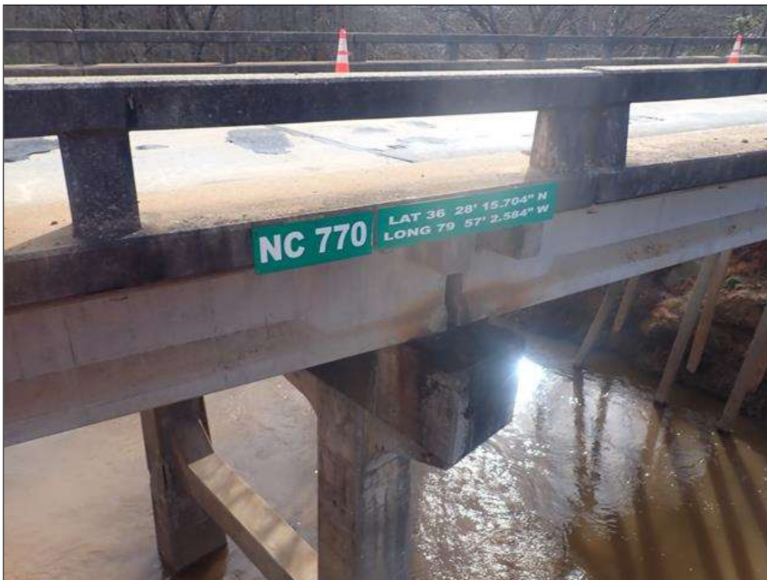
bridge sign at bent 2
