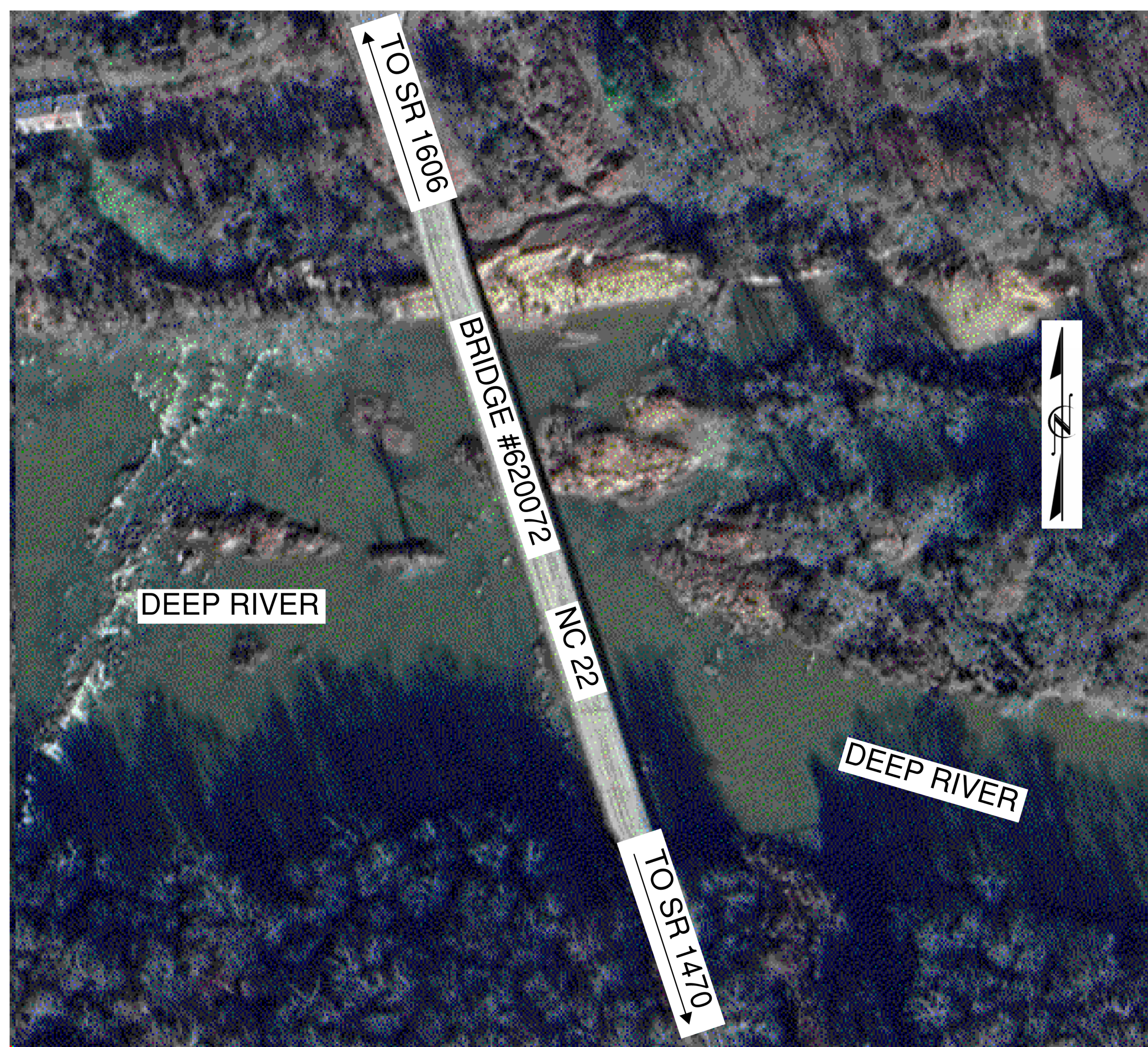
BRIDGE 620072 - LATITUDE: 35°28'41.54"; LONGITUDE: 79°31'11.52"
