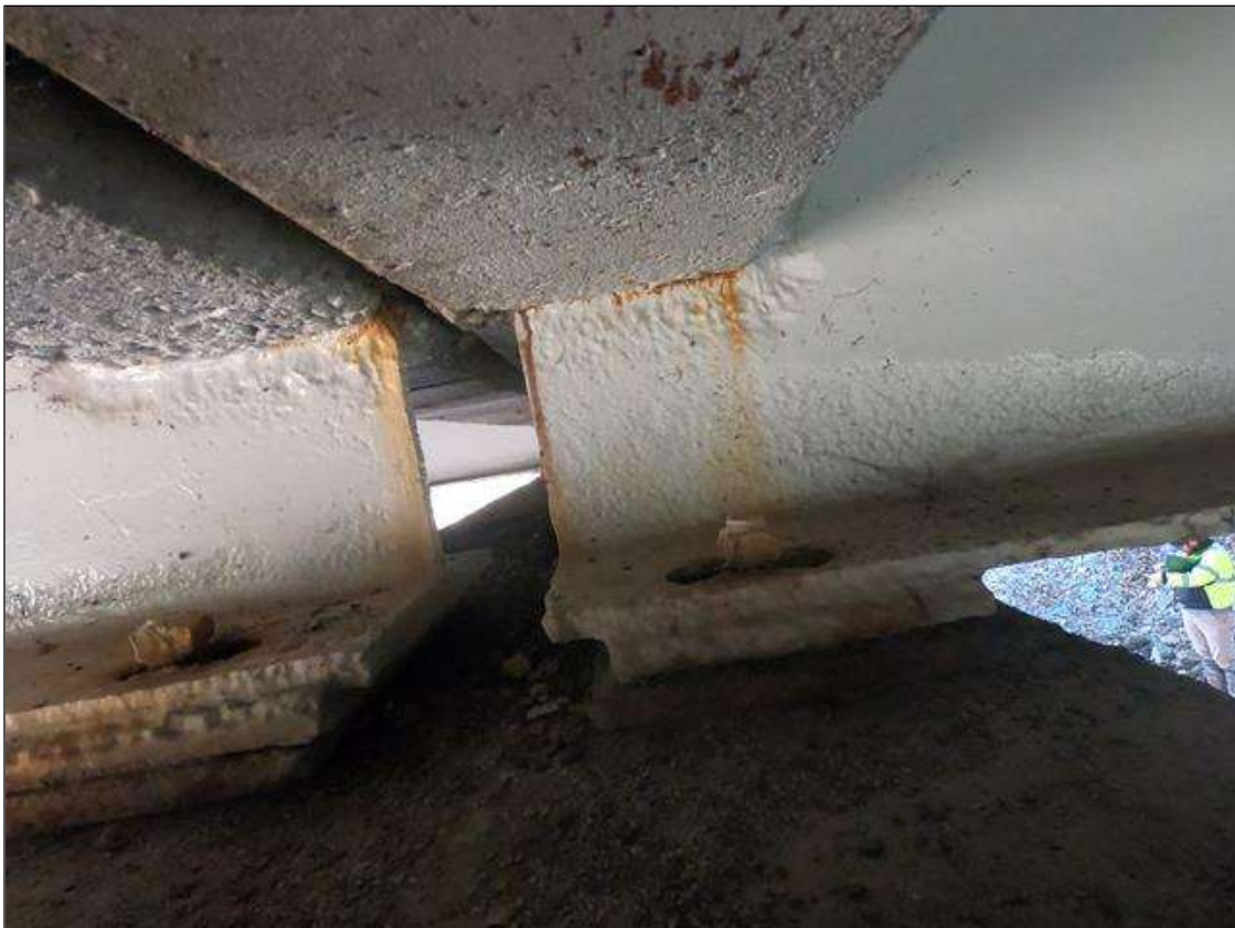
INTERIOR BENT BEARING
