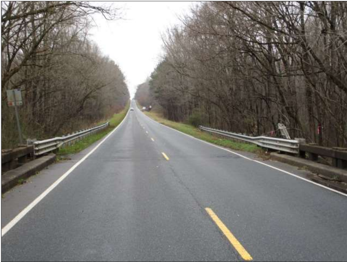
LOOKING NORTH FROM BRIDGE
