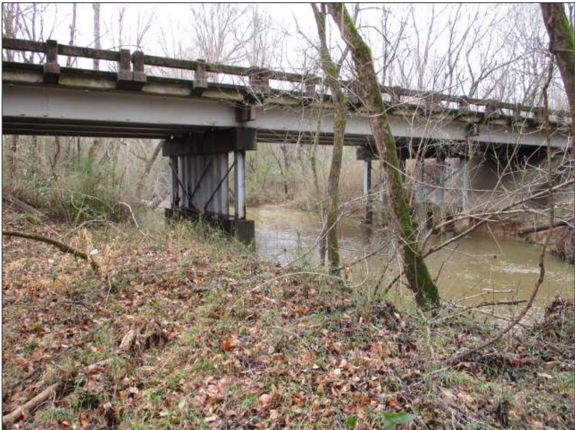
LOOKING WEST UPSTREAM UNDER SPAN 2
