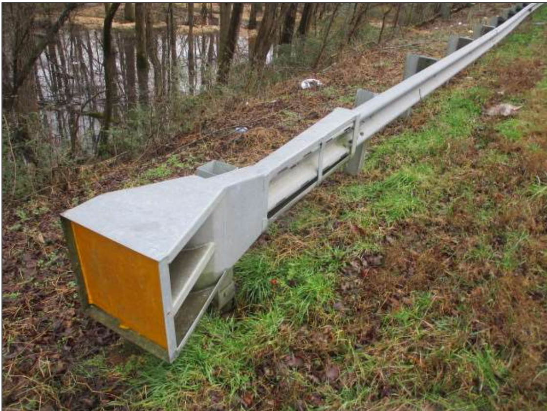
NORTHEAST GUARDRAIL END TREATMENT
