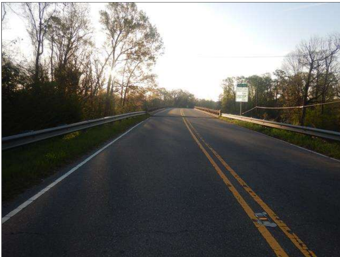
WEST APPROACH LOOKING EAST
