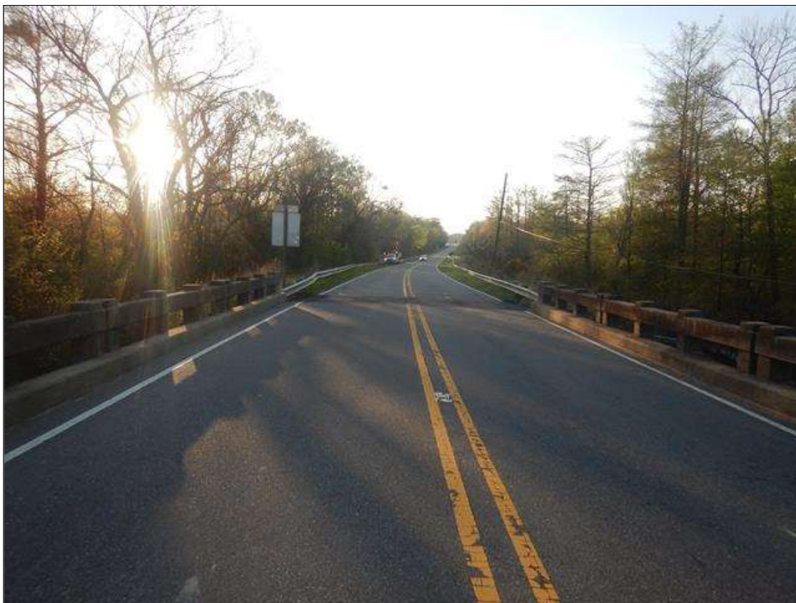
EAST APPROACH LOOKING EAST
