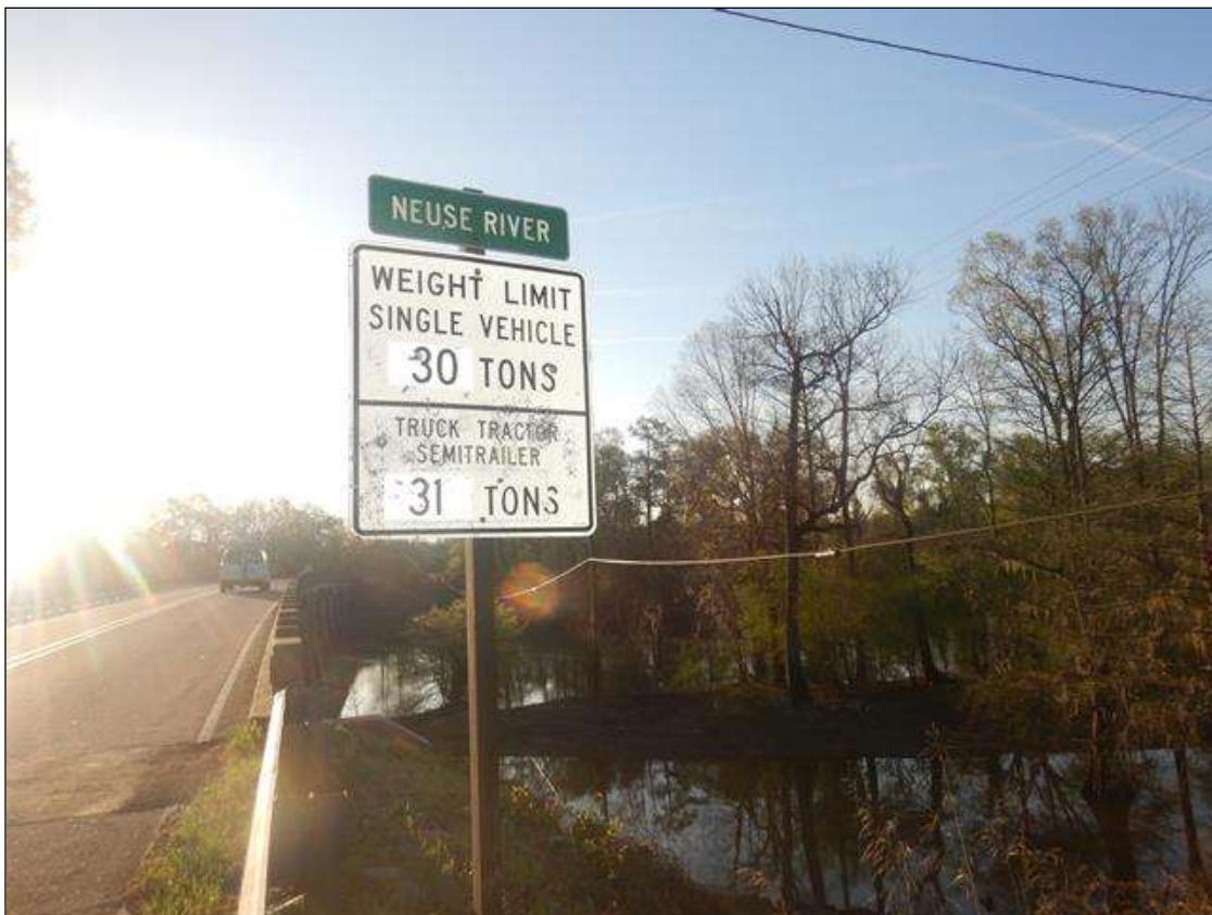
WEIGHT POSTING SIGN, WEST APPROACH SHOWN
