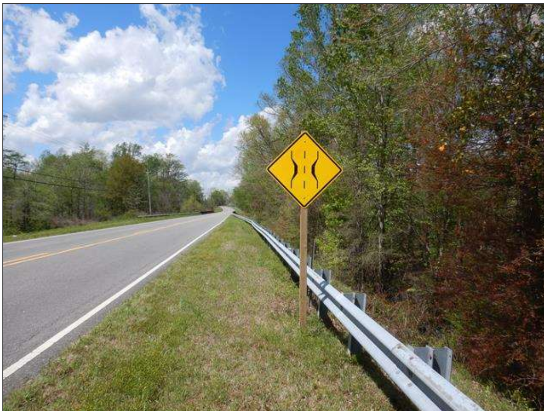
EAST APPROACH NARROW BRIDGE SIGN, 0.02 MILES FROM END BENT 2
