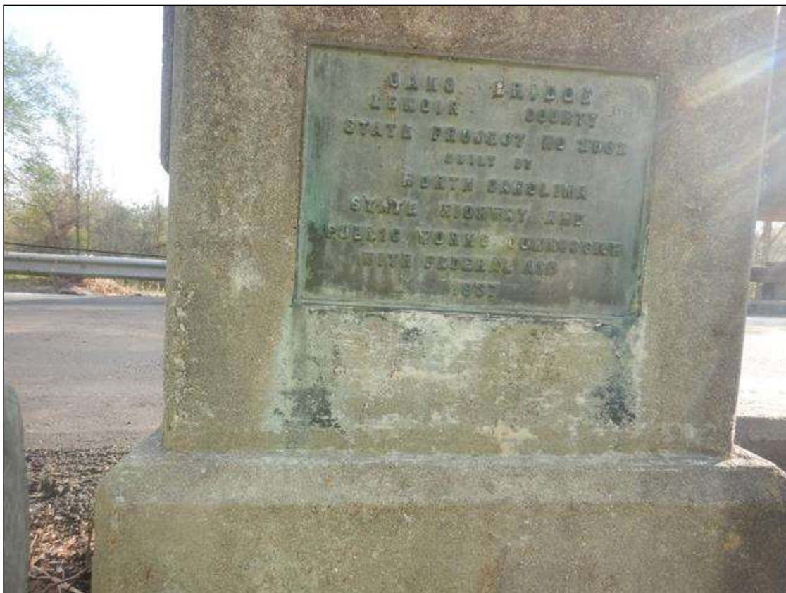
TYPICAL BRIDGE PLAQUE
