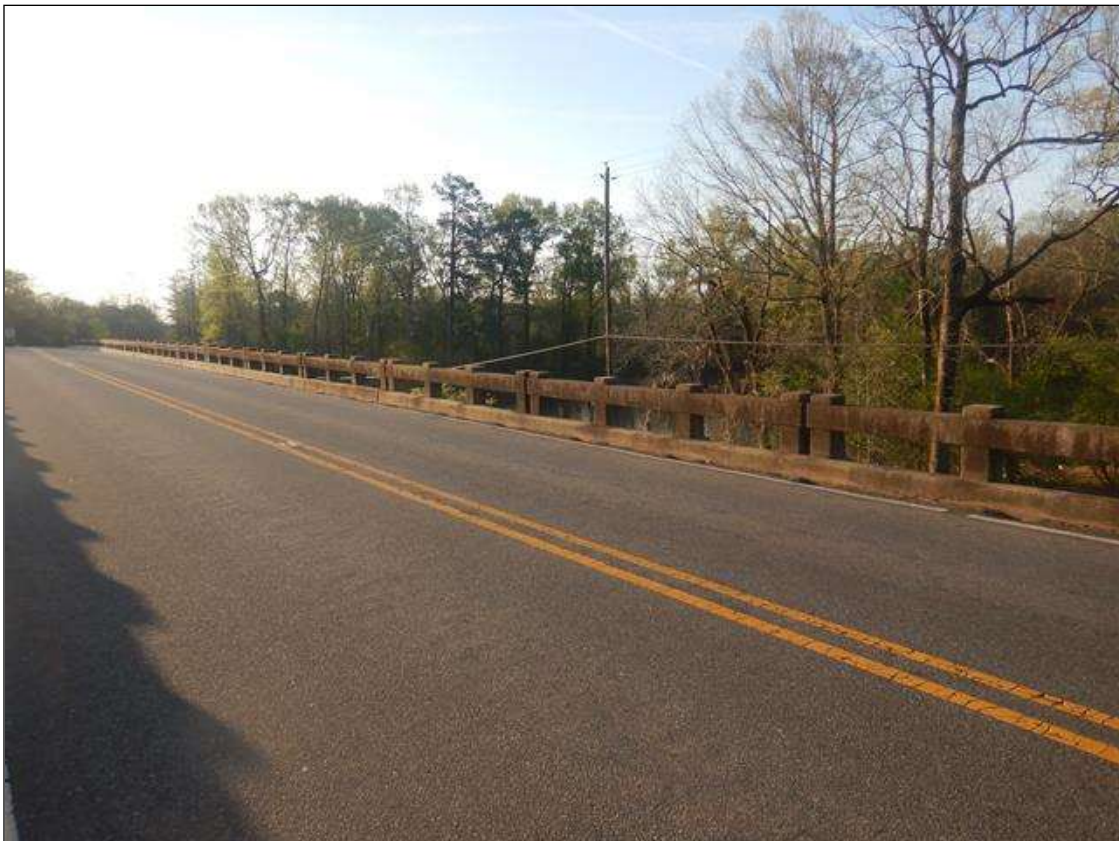
RIGHT BRIDGE RAIL, LEFT BRIDGE RAIL SIMILAR
