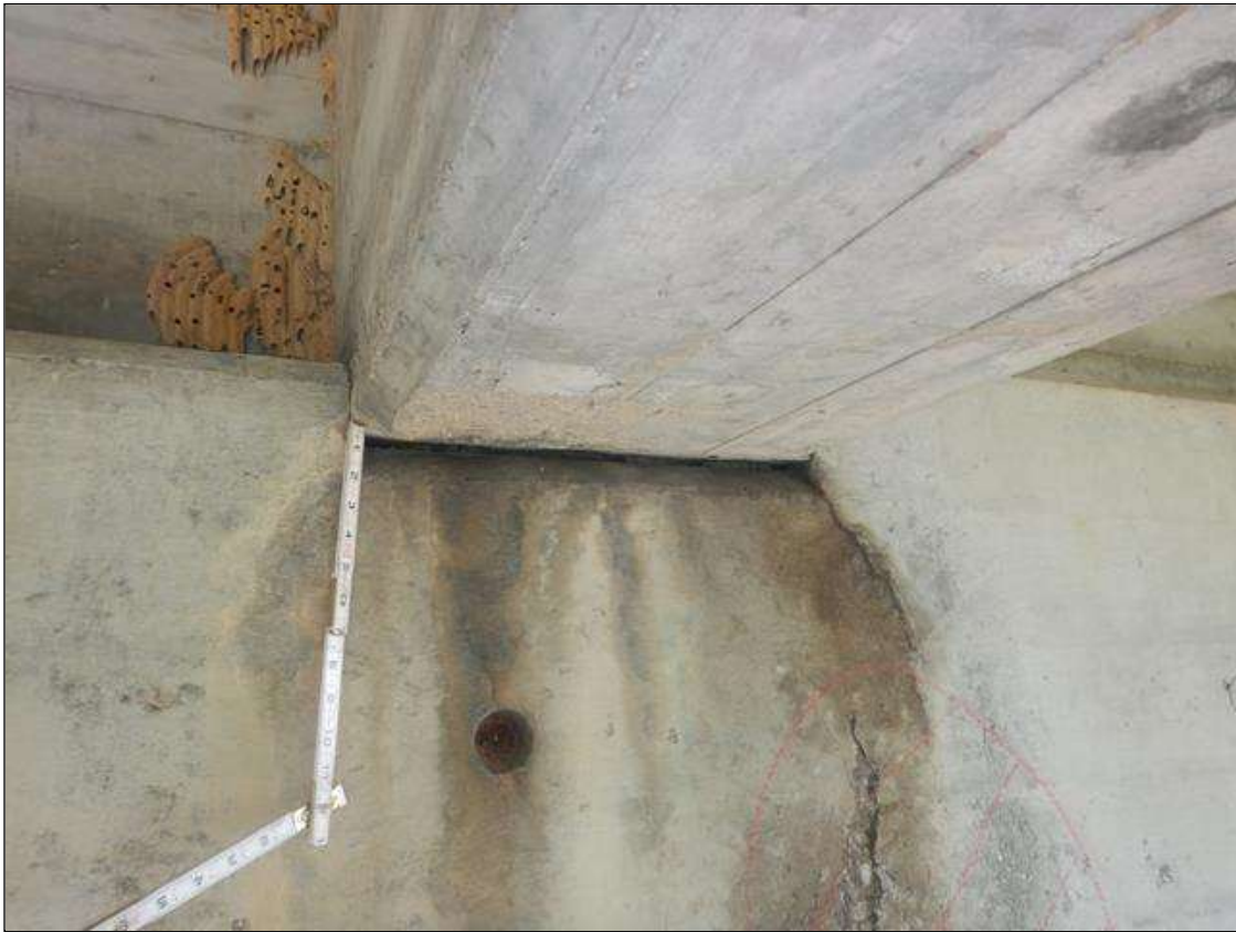
TYPICAL BEARING, SPAN 9 BEAM 2 NEAR BEARING SHOWN
