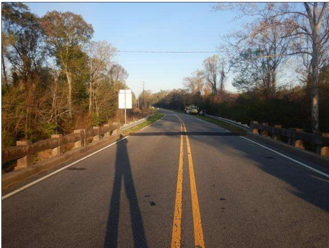
WEST APPROACH LOOKING WEST
