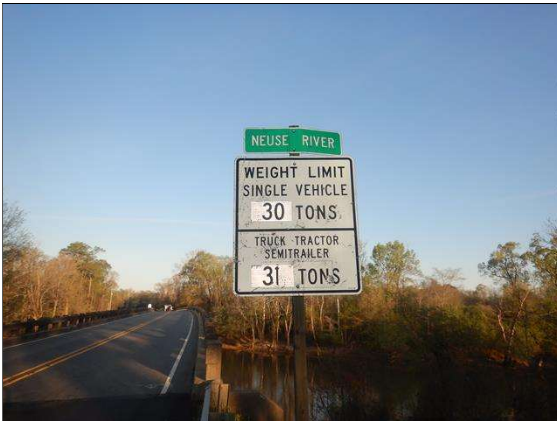
WEIGHT POSTING SIGN, EAST APPROACH SHOWN
