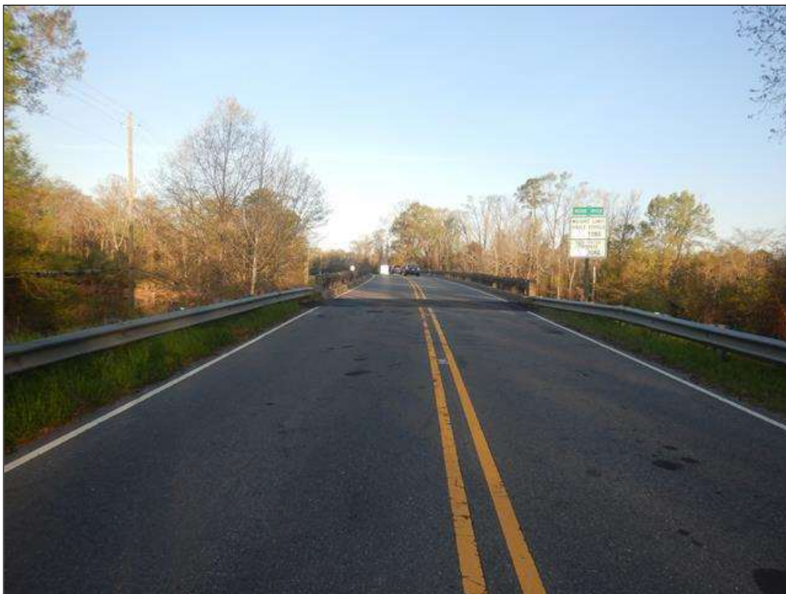
EAST APPROACH LOOKING WEST
