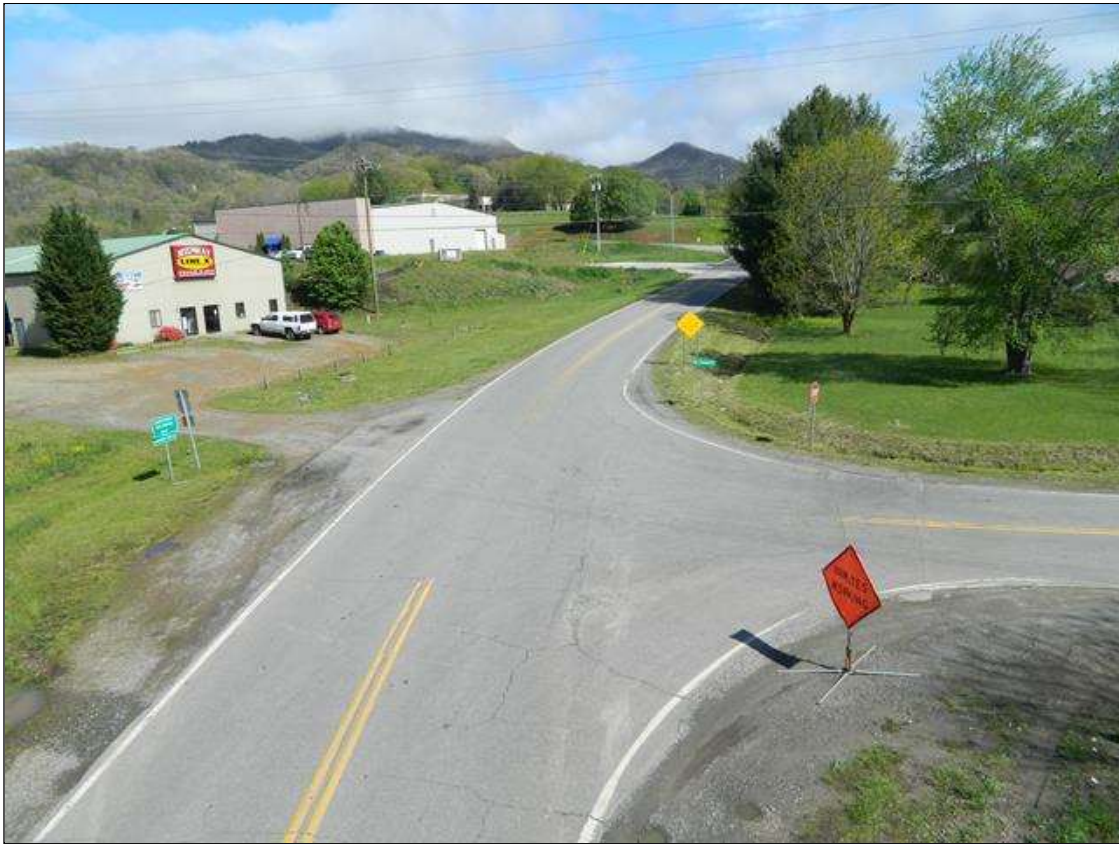
LOOKING NORTH FROM TOP OF STRUCTURE
