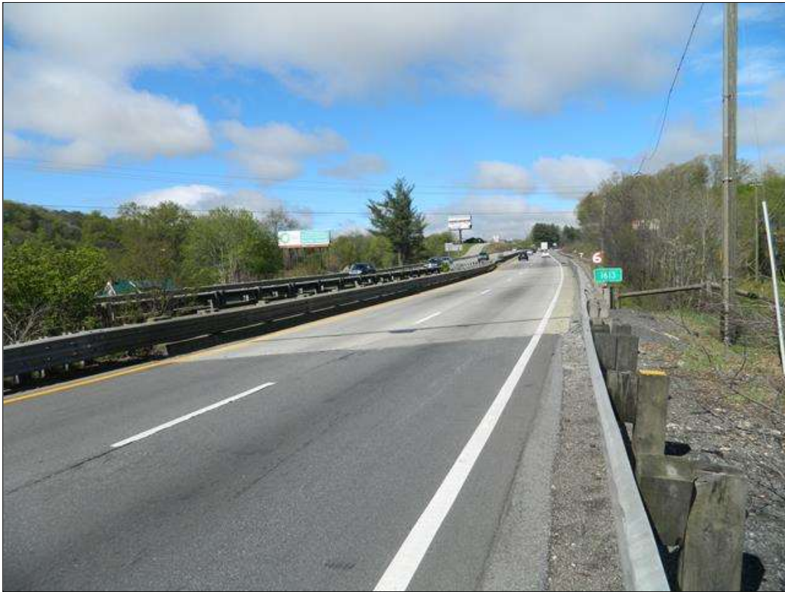
EAST APPROACH LOOKING WEST
