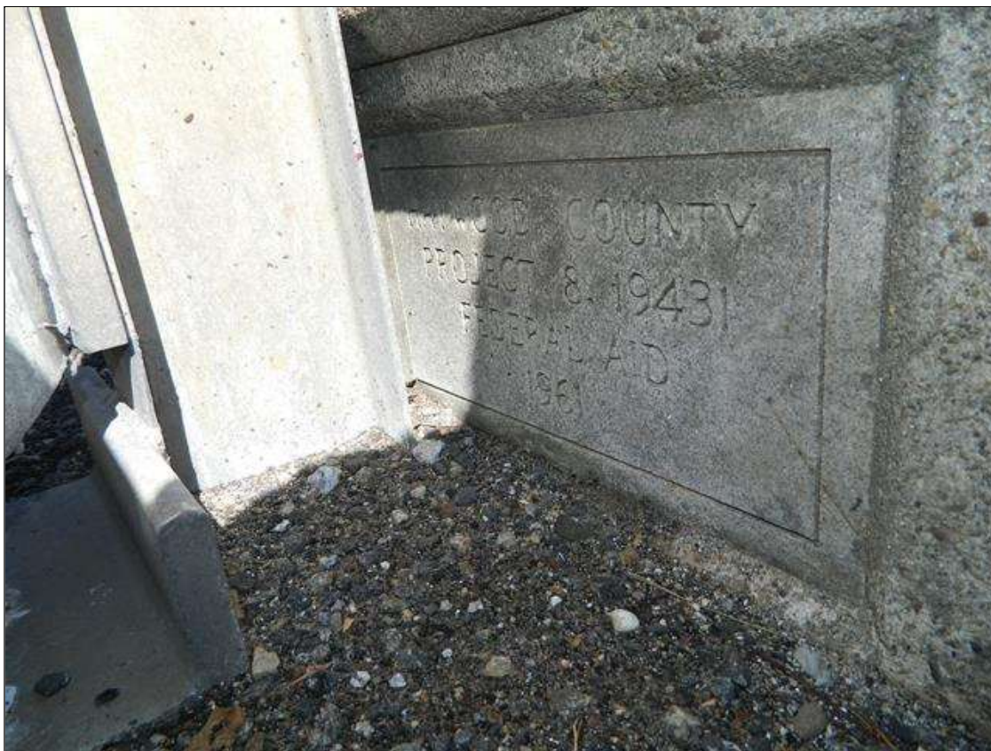
STRUCTURE INFO PLATE AT THE NORTH WEST CORNER.
