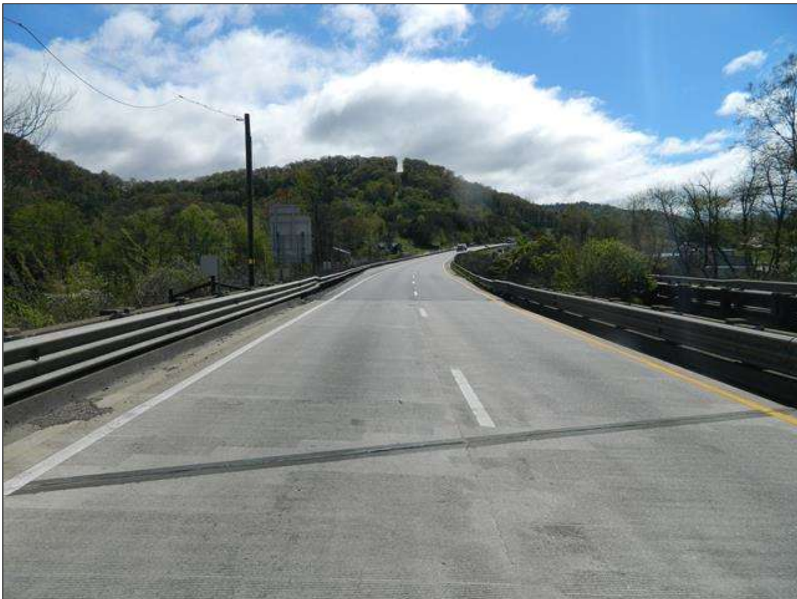
GUARDRAIL LOOKING EAST
