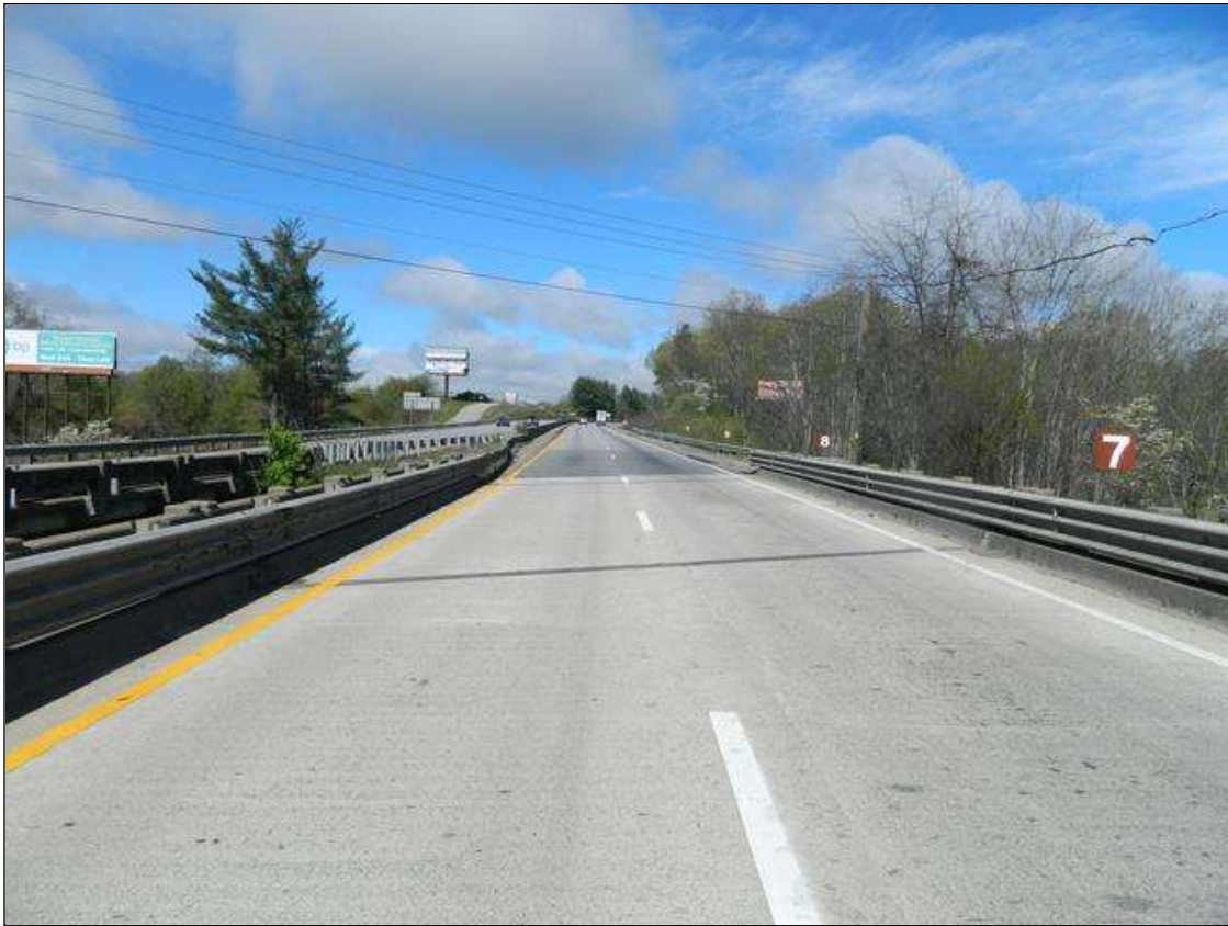
GUARDRAIL LOOKING WEST
