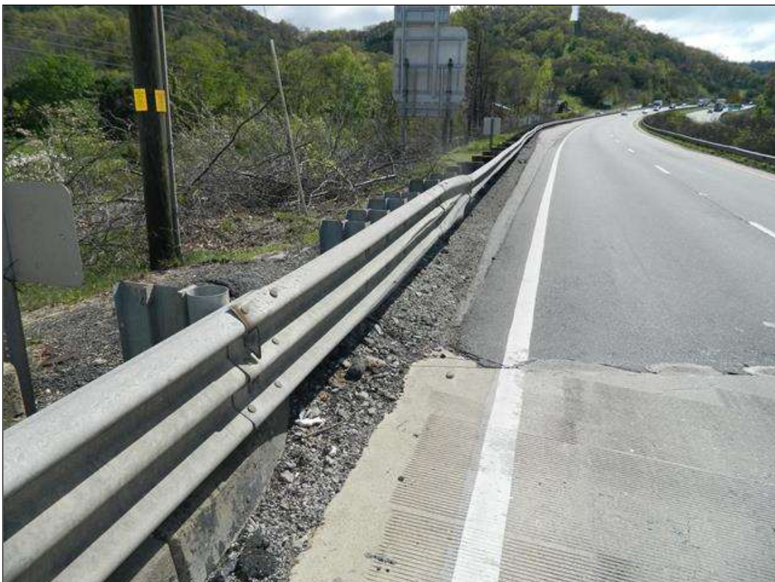
RETROFIT RAIL IS CONTINUOUS WITH APPROACH RAIL.
