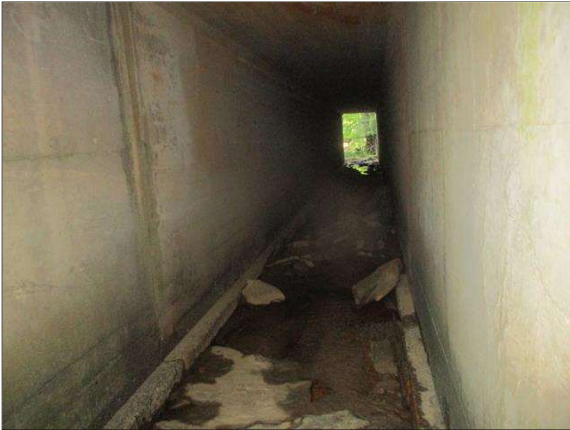
LOOKING DOWNSTREAM BARREL 1
