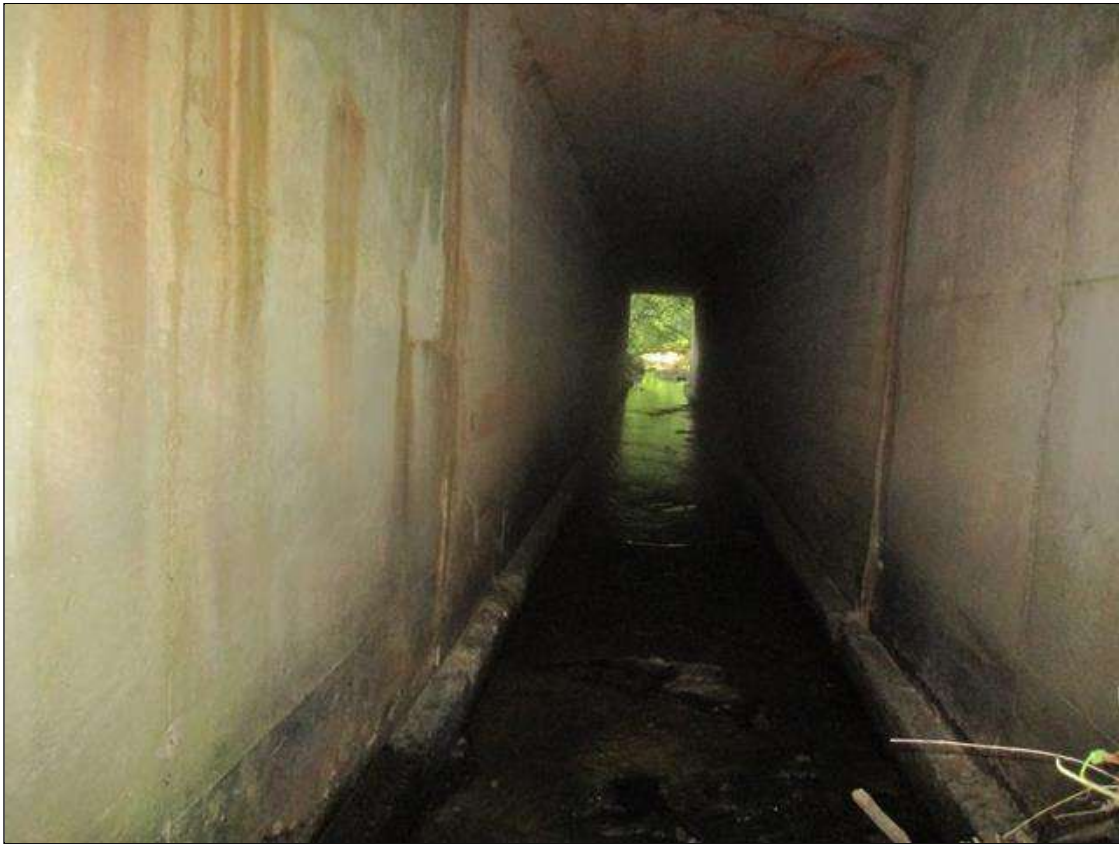
LOOKING DOWNSTREAM BARREL 3
