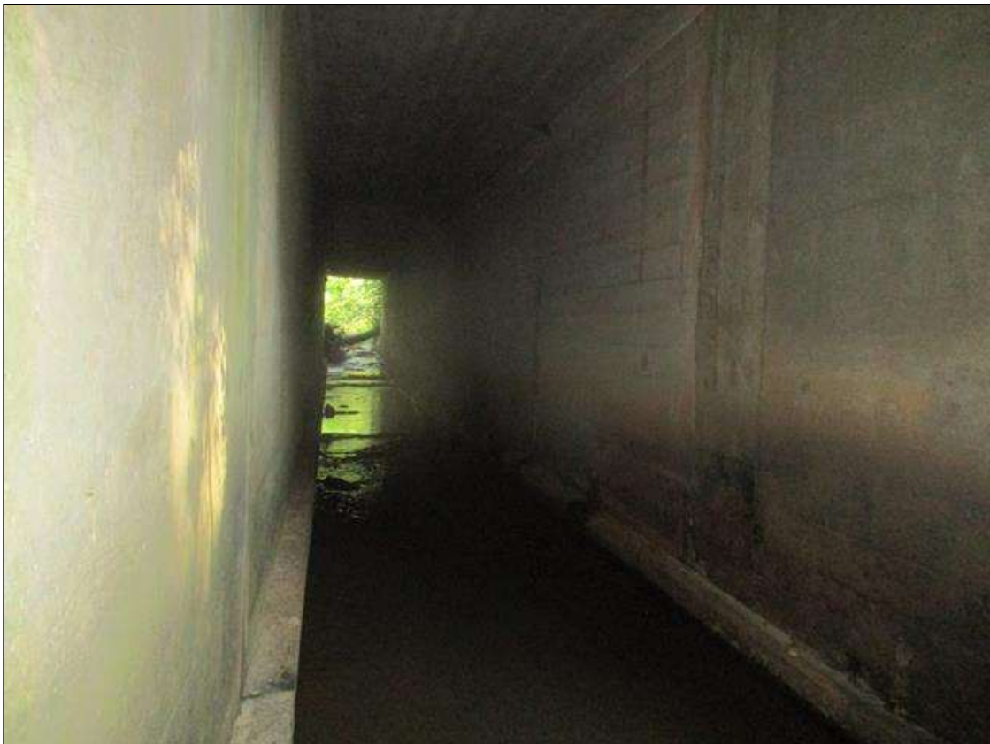
LOOKING UPSTREAM THROUGH BARREL 3
