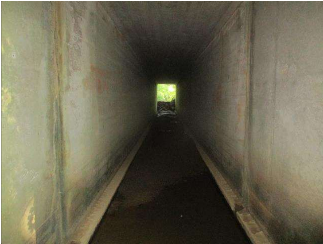
LOOKING UPSTREAM THROUGH BARREL 2
