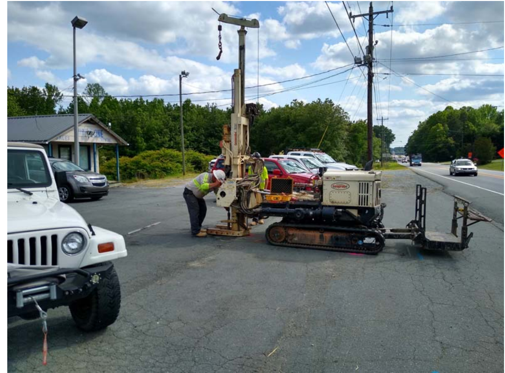
D. Photograph of drilling operations, looking southwest.
