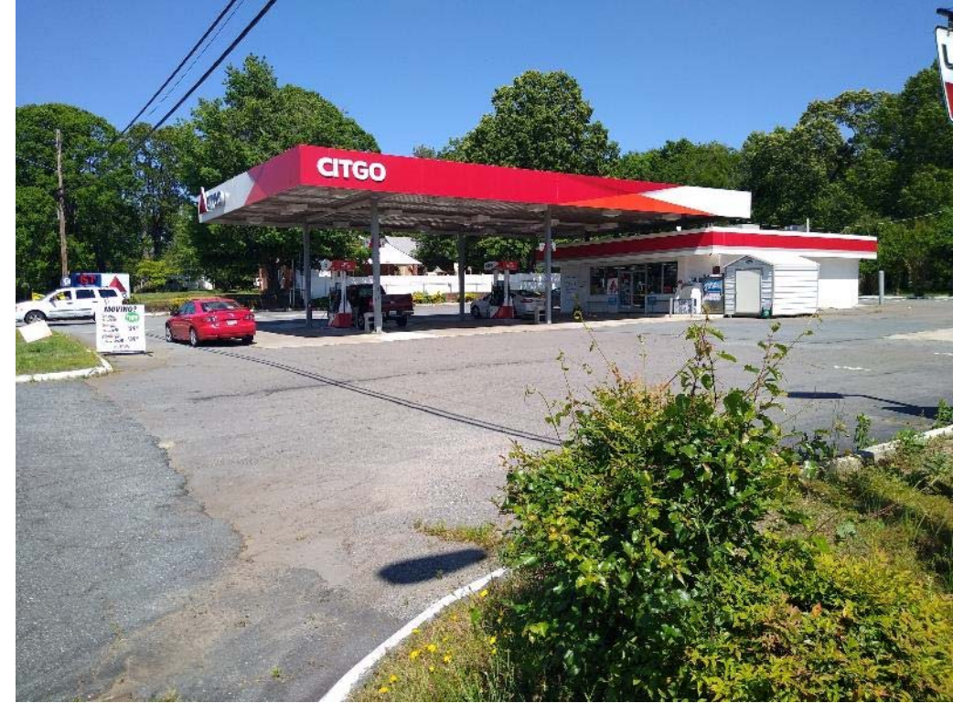
B. Photograph from southwest corner of parcel, looking northeast.
