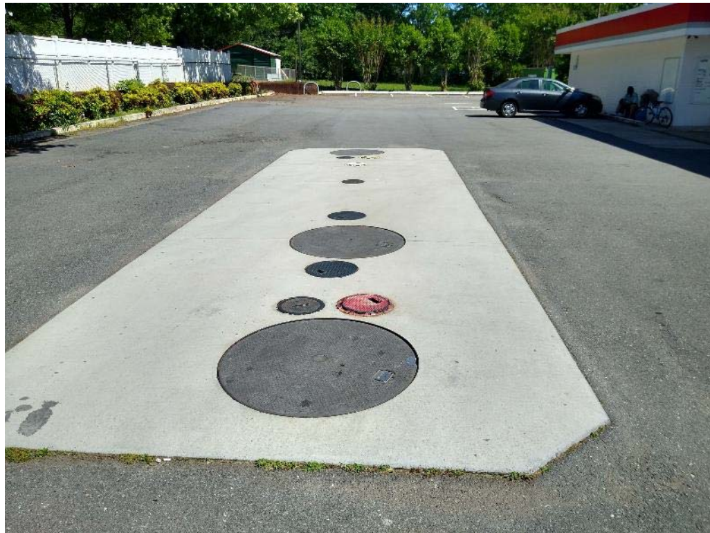
C. Photograph of tank bed, looking southeast.
