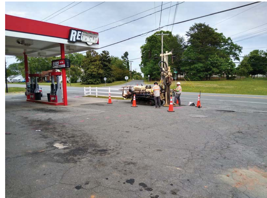
D. Photograph of drilling operations, looking northeast.
