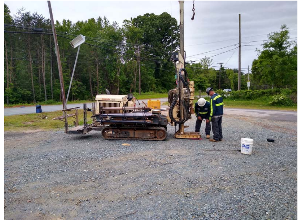
D. Photograph during drilling operations.
