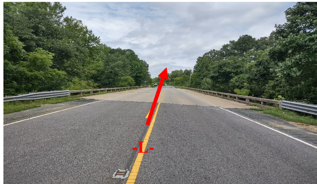
View of Along Bridge 0001 Looking Downstation
