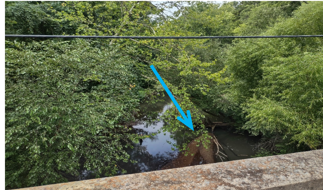
View Looking Upstream from Bridge 0001
