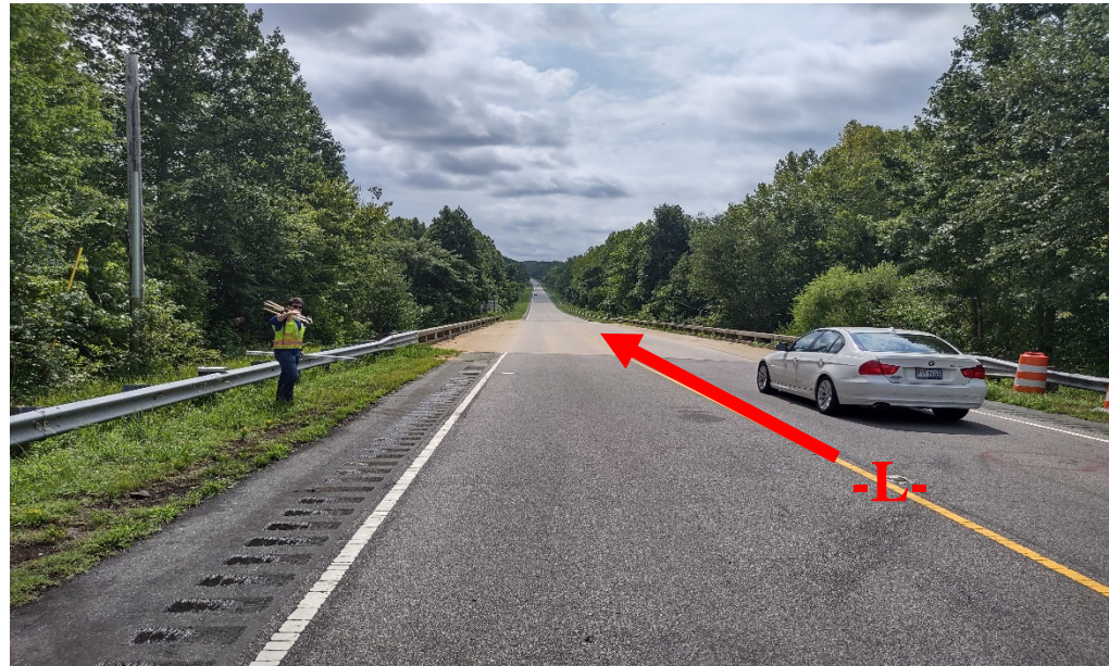
View Along Bridge 0001 Looking Upstation
