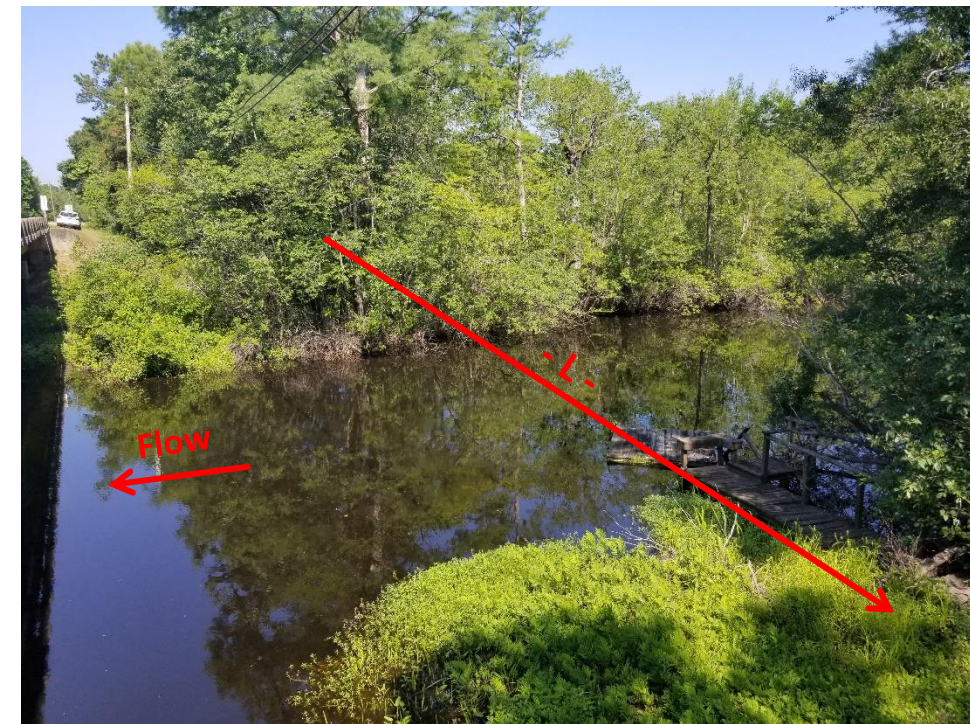
Photograph No. 4: View from existing End Bent 2 slope looking west toward proposed End Bent 1
