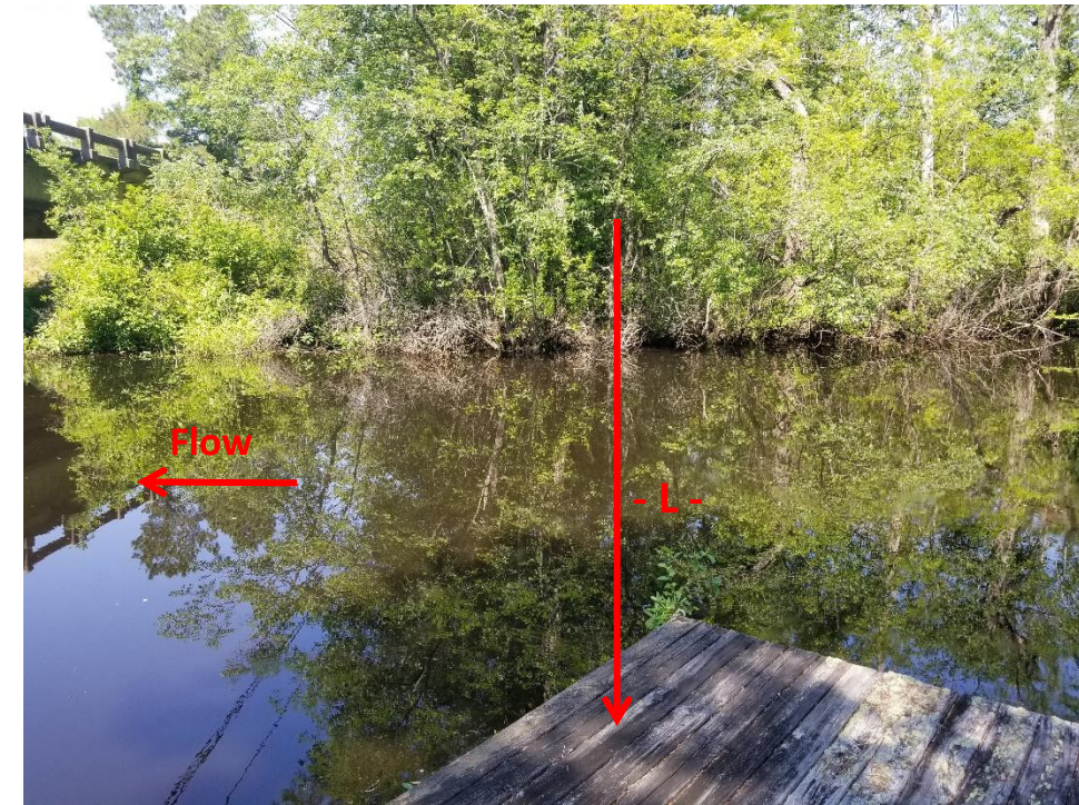
Photograph No. 3: View looking west toward proposed End Bent 1
