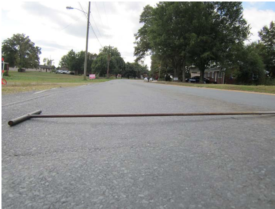
Exhibit A-17: Photograph of Moderate Rutting along Potter Road south of the Intersection
