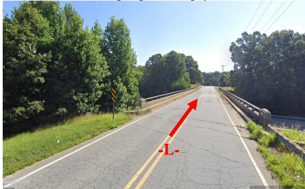
View Along Bridge 170 Looking Upstation
