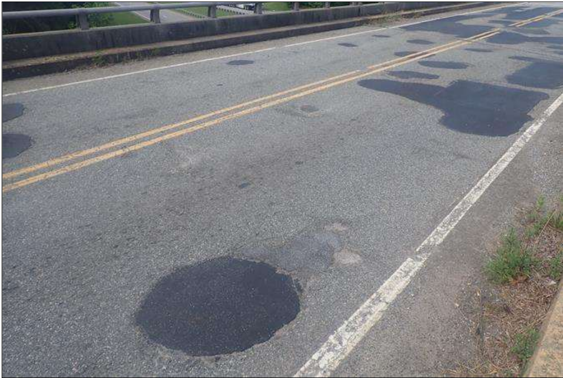
Span 1 Wearing Surface: Several sound asphalt patches in travel lanes
