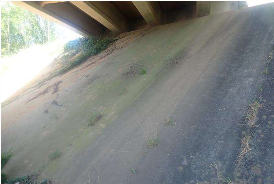
end bent 2 slope protection
