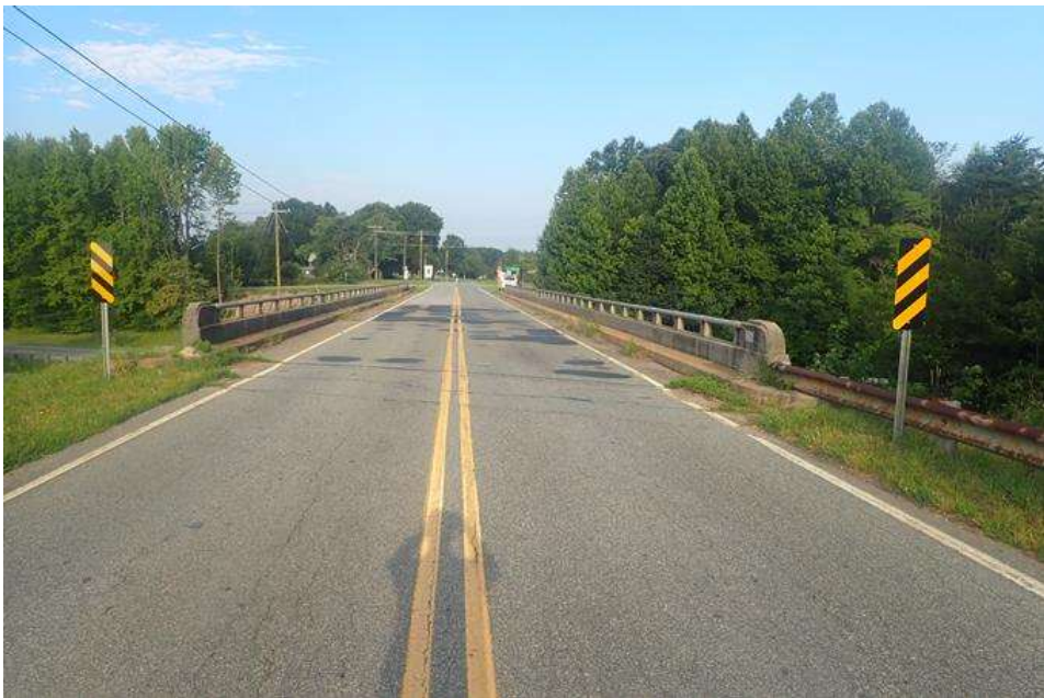
south approach looking north
