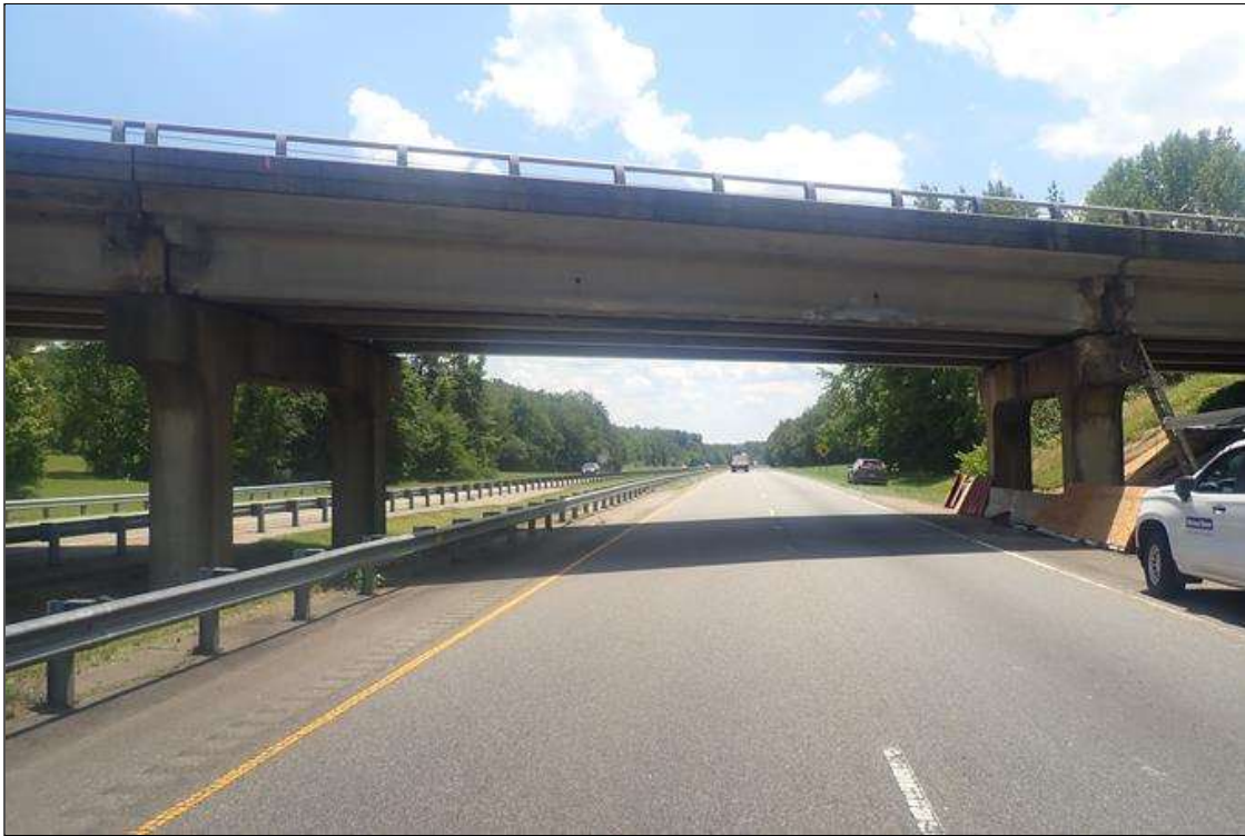
roadway under span 3, looking west (US-220 southbound)
