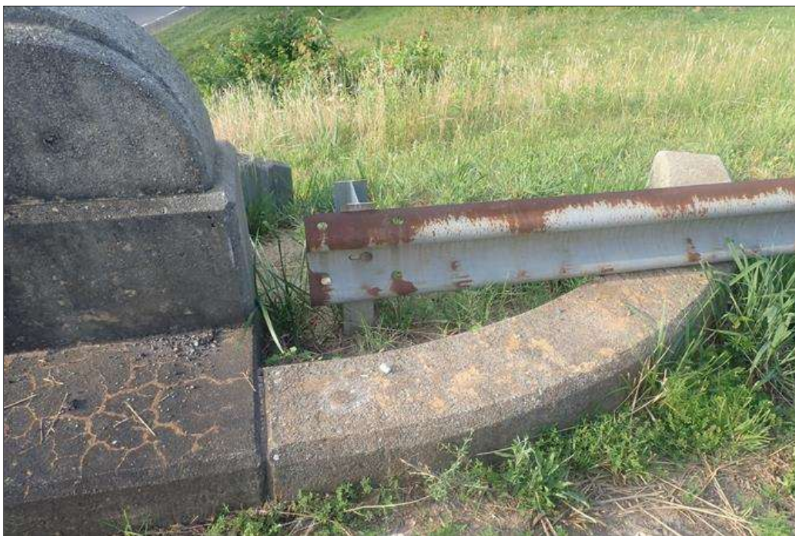
northwest guardrail at bridge
