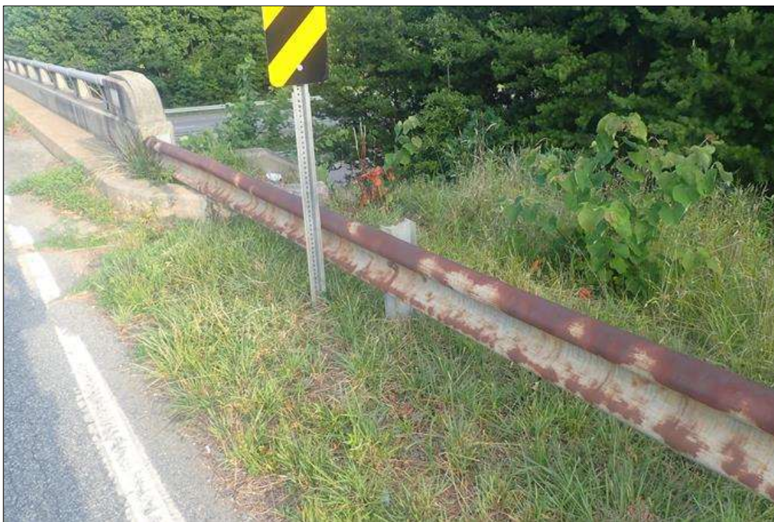
southeast guardrail, no transition
