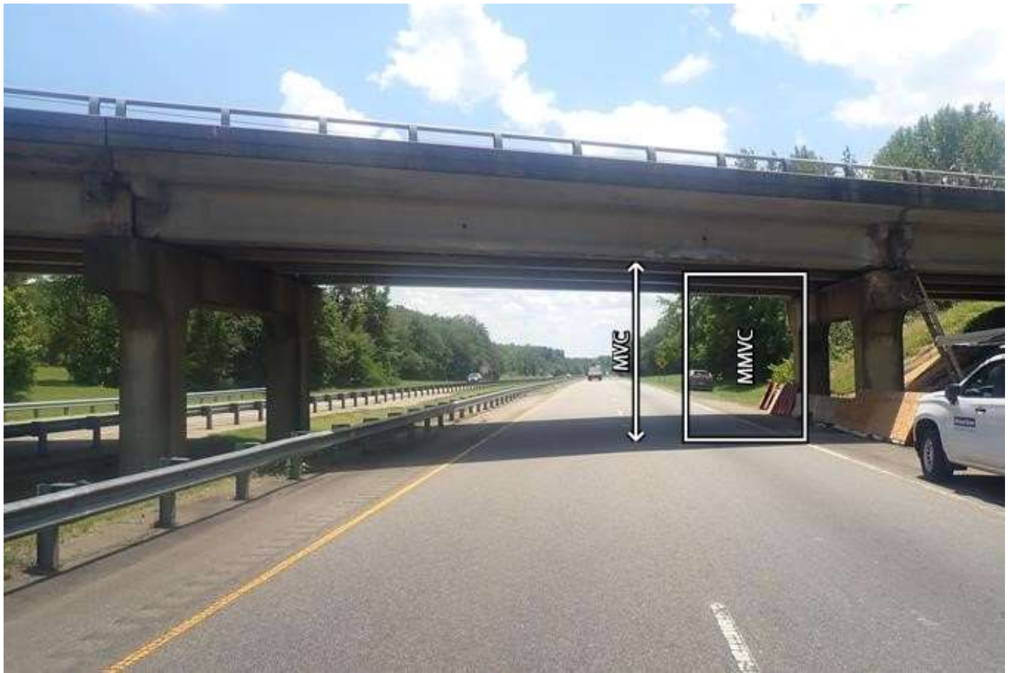
roadway under span 3, looking west (US-220 southbound)
