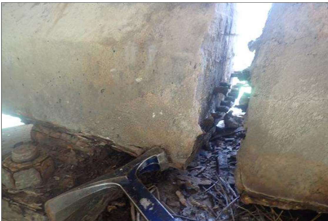
Span 1 Beam 1: 6 INCH X 5 INCH PATCHED AREA THAT IS SOUND ON RIGHT SIDE OF BOTTOM FLANGE OVER PIER 1.
