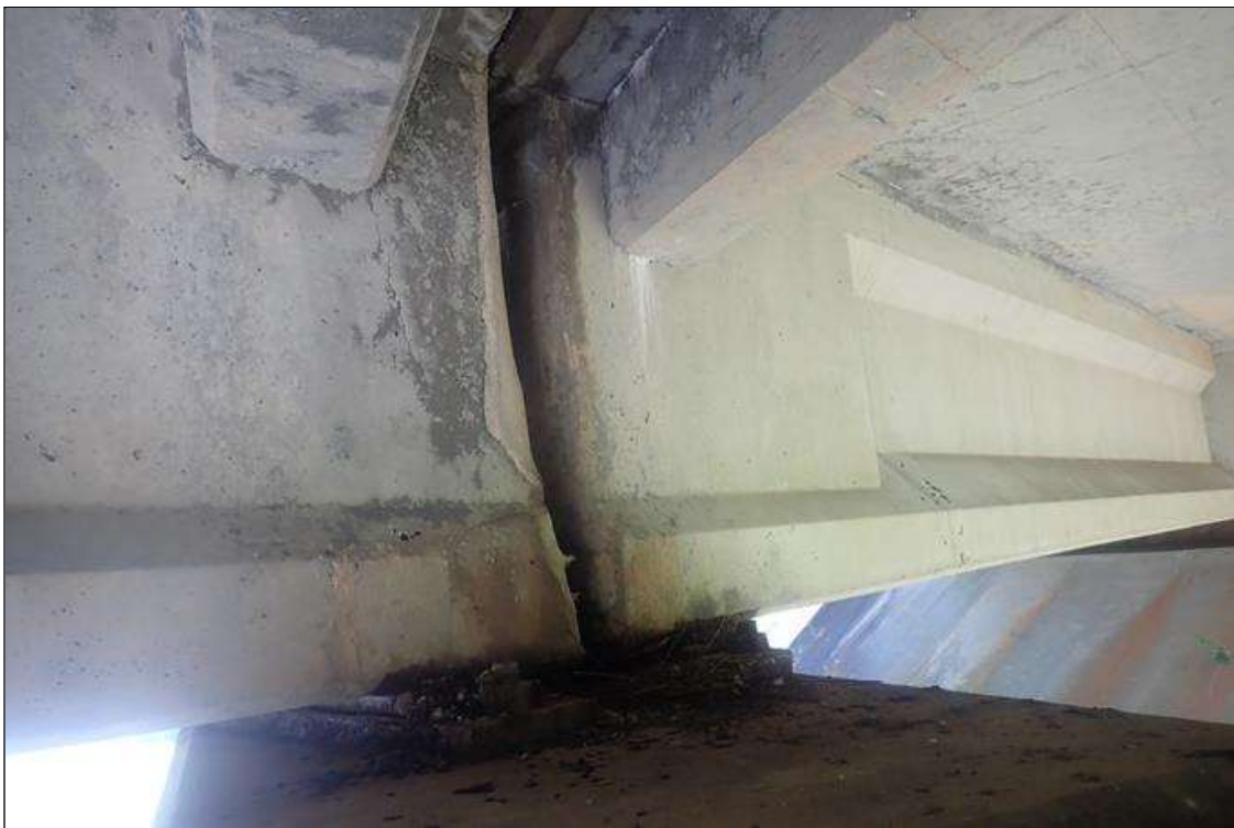
beams over bent
