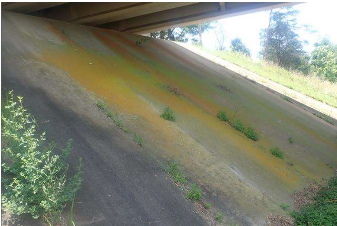
end bent 1 slope protection
