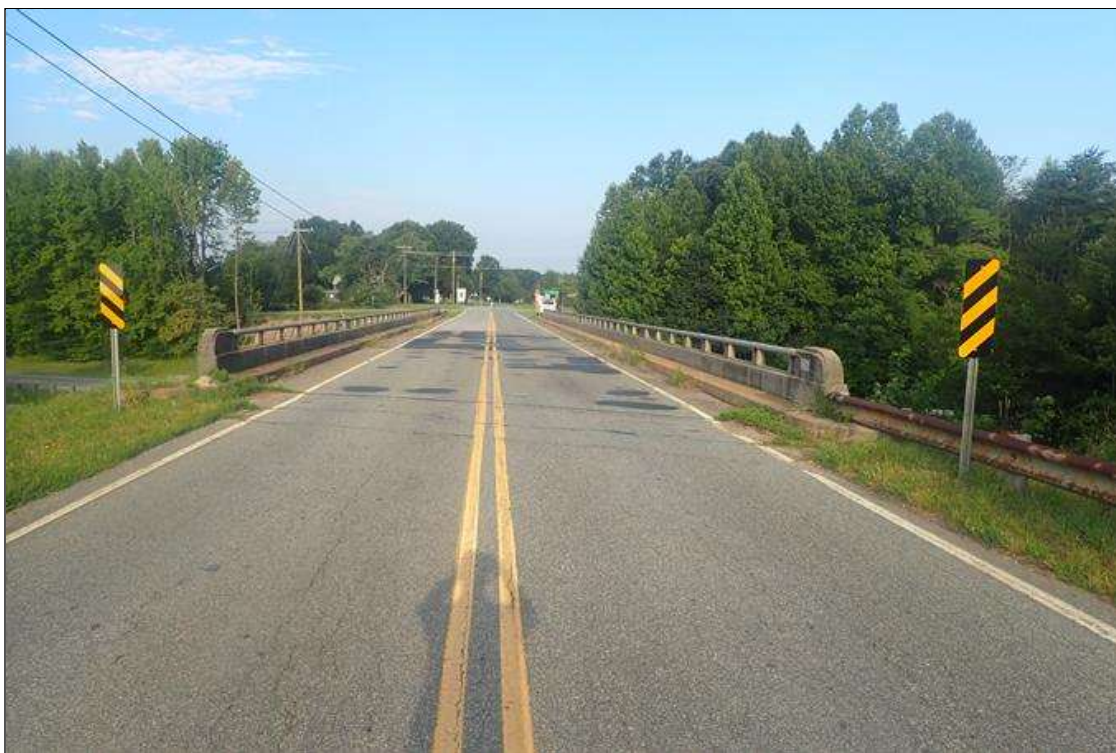
south approach looking north
