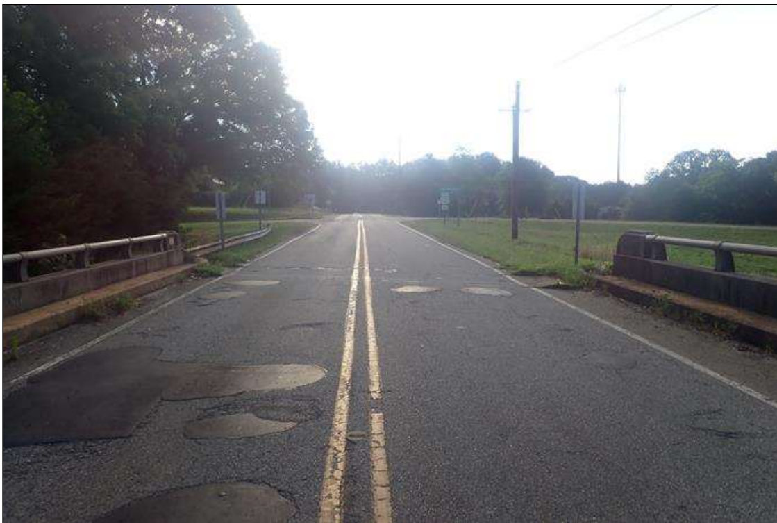
south approach looking south
