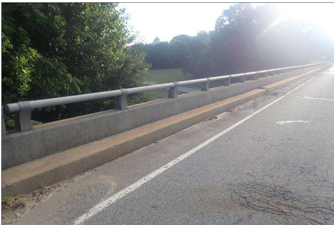
right bridge rail
