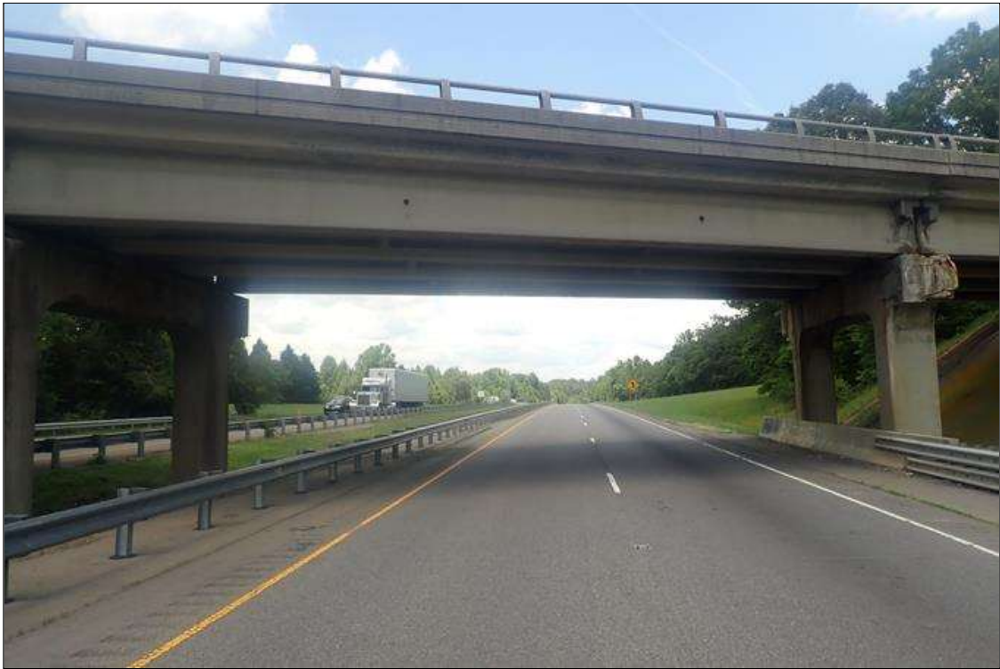
roadway under span 2, looking east (US-220 northbound)
