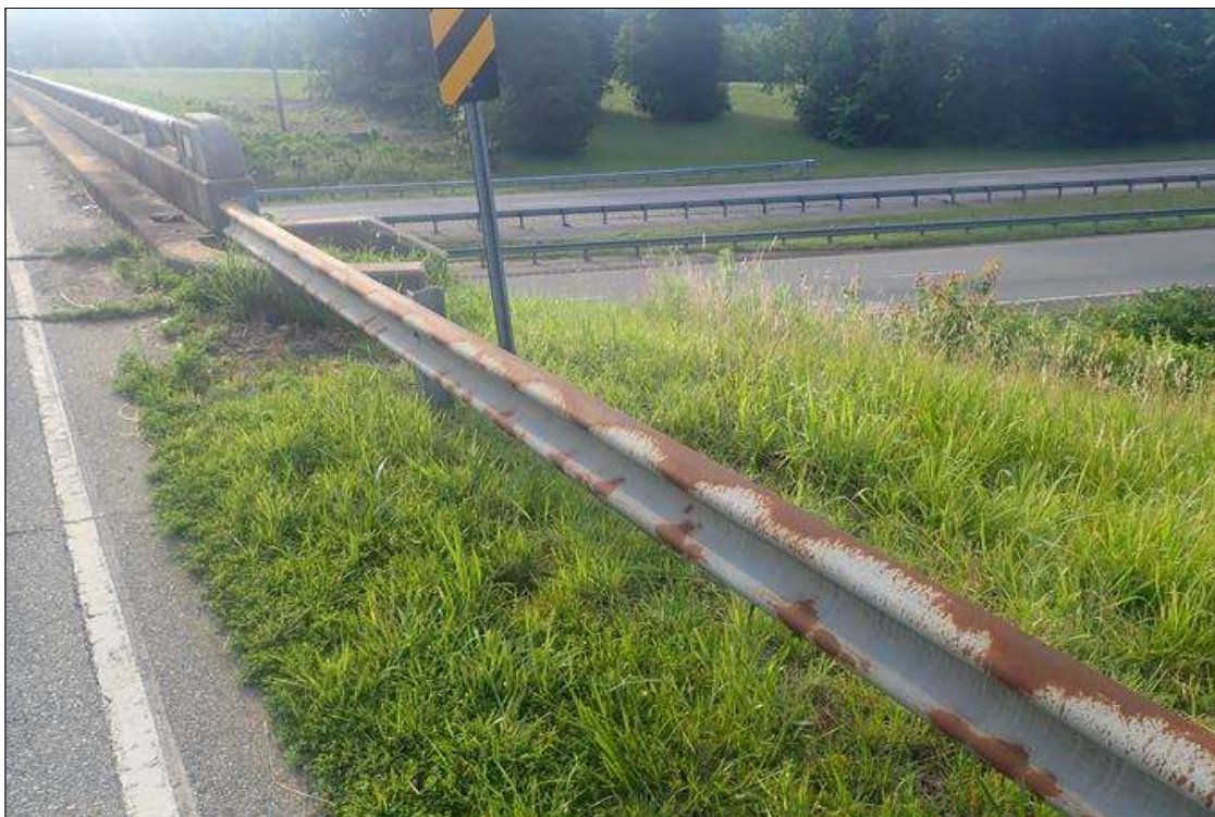
northwest guardrail, no transition
