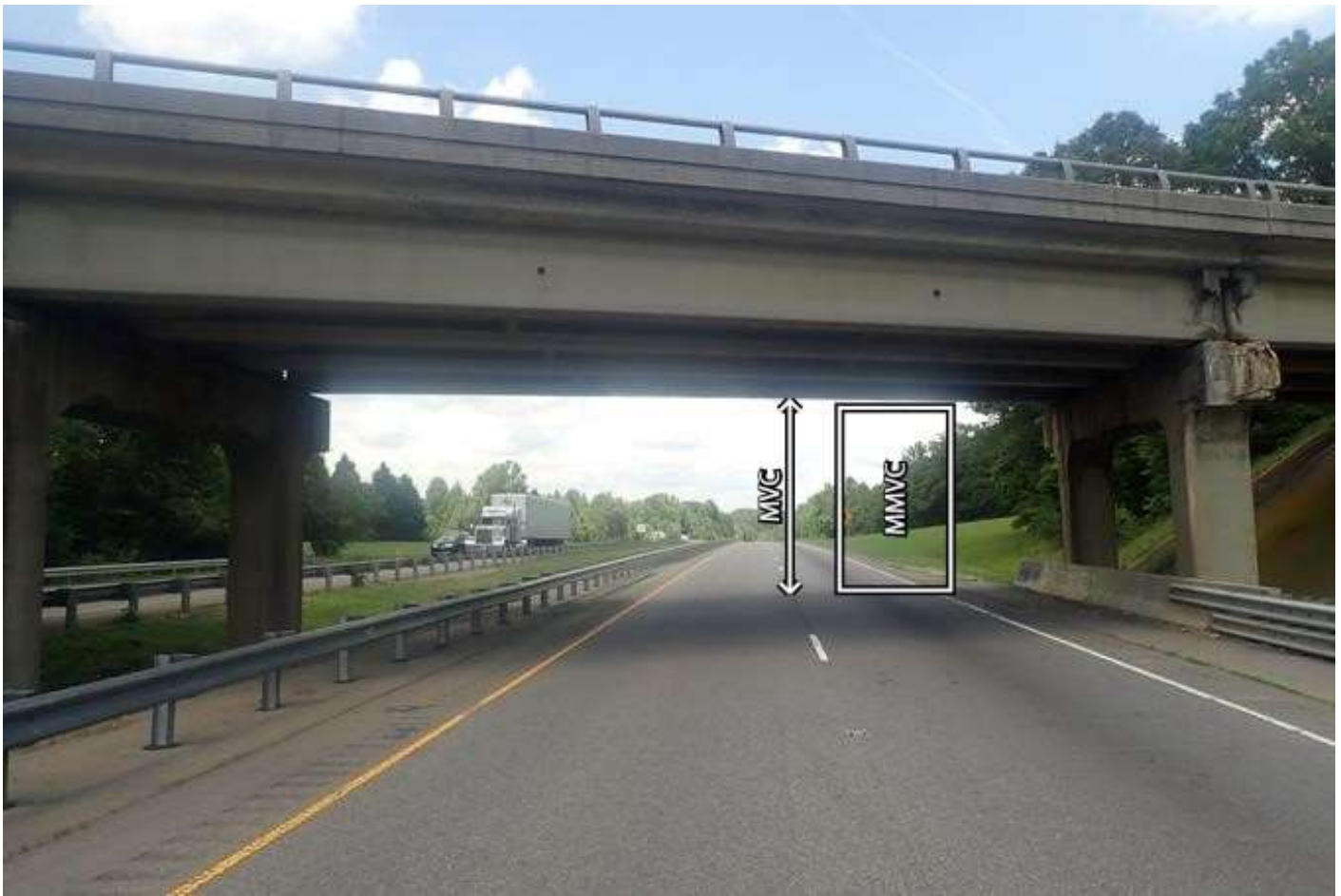
roadway under span 2, looking east (US-220 northbound)
