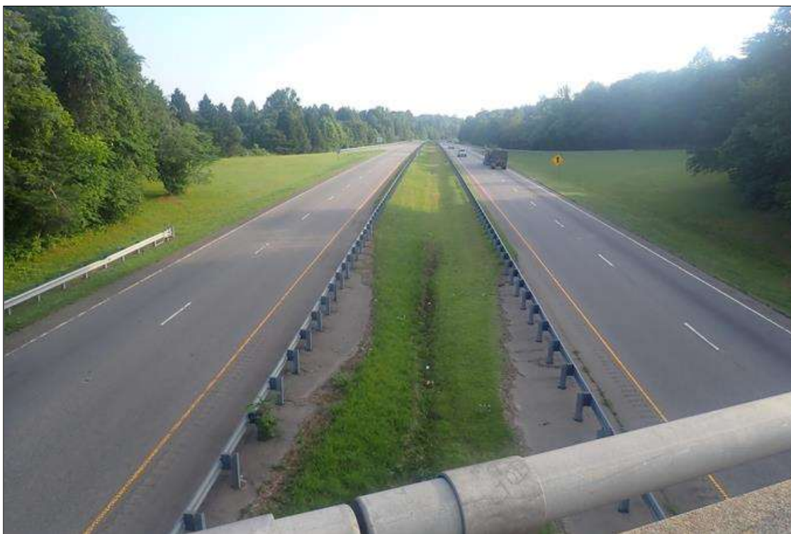
roadway looking east
