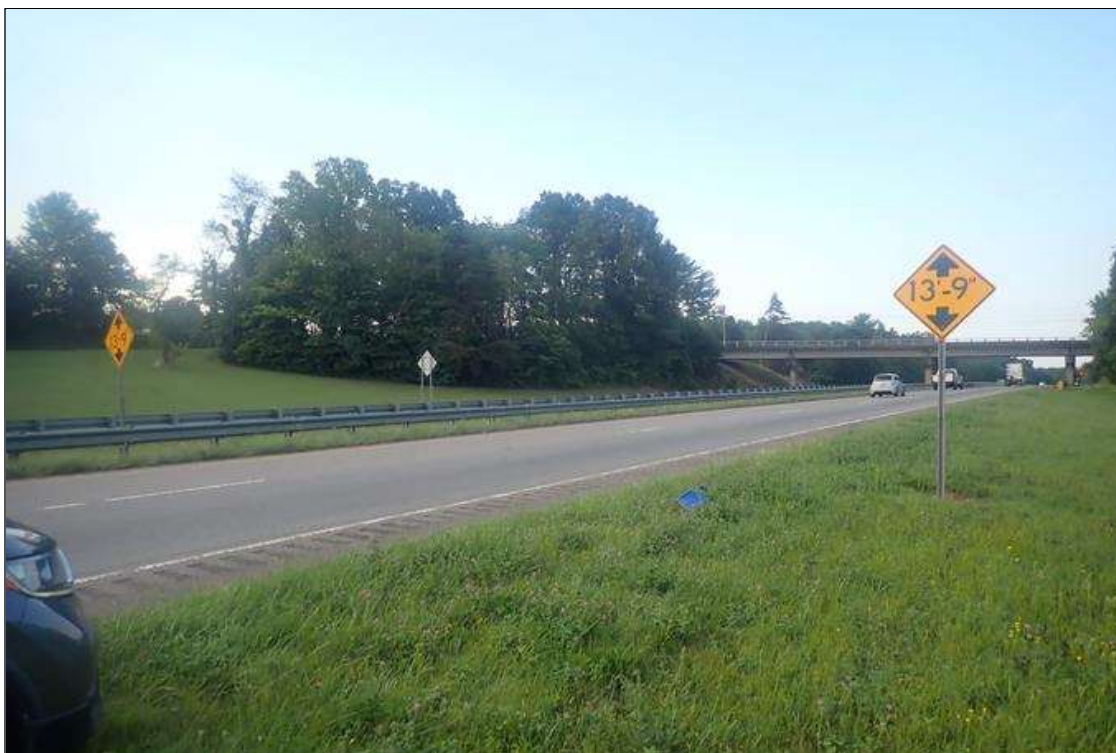
(2) vertical clearance signs, US220 southbound, 370 feet from bridge
