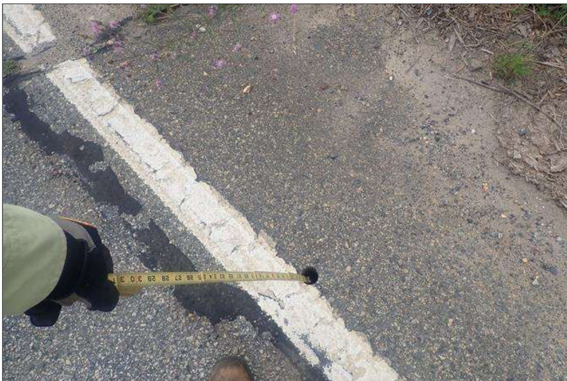
Span 3 Deck: left shoulder, near bent 2, core hole (1.5 inch diameter)
