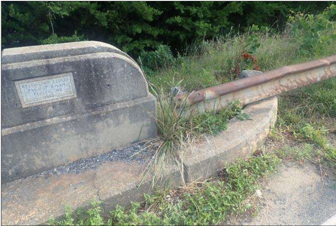
southeast guardrail at bridge
