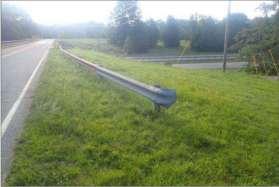
northwest guardrail and termination
