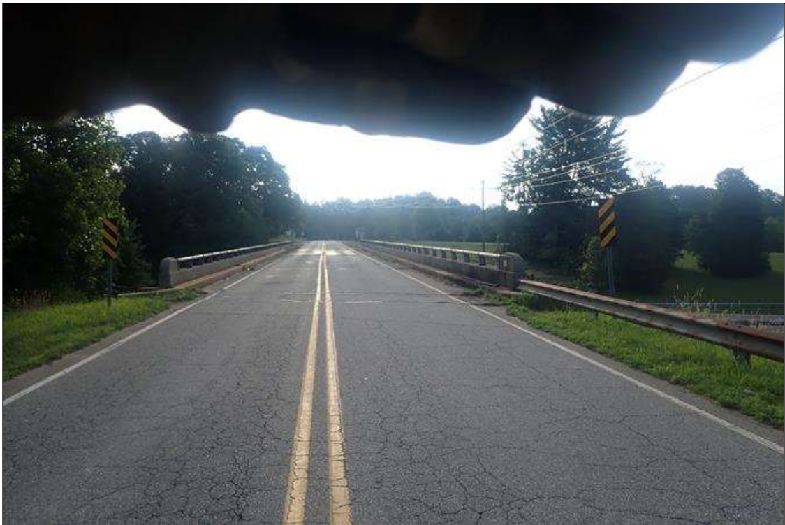
north approach looking south
