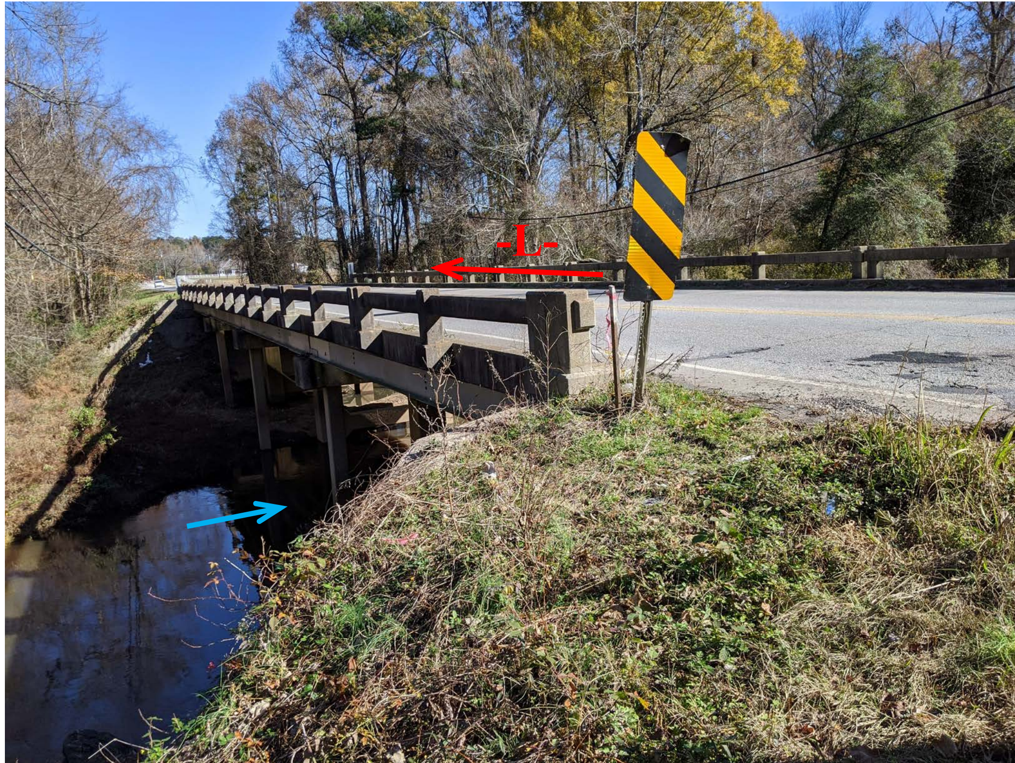
Looking Northeast towards End Bent 2
