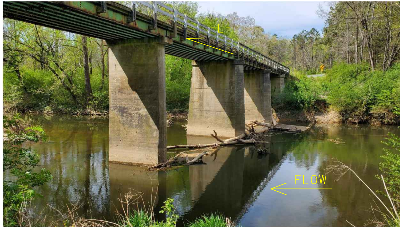
Photo #1: North side of existing bridge looking south/southwest (downstation)
