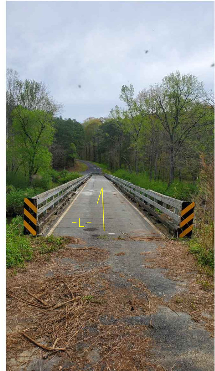
Photo #3: End Bent 1 looking north/northeast (upstation)
