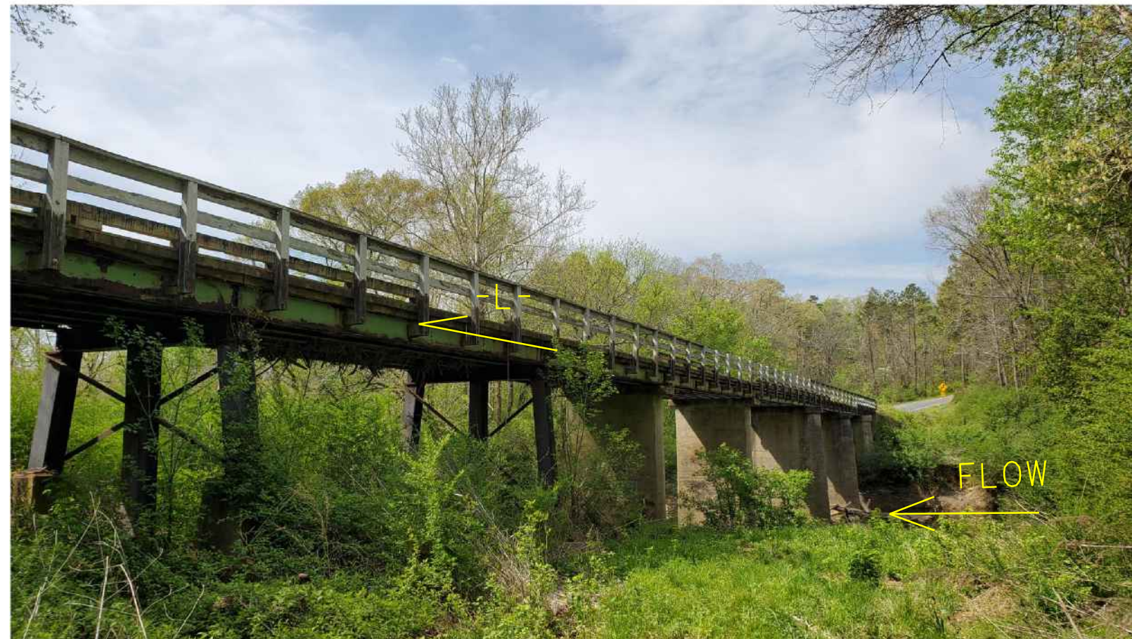
Photo #2: North side of existing bridge looking south/southwest (downstation)
