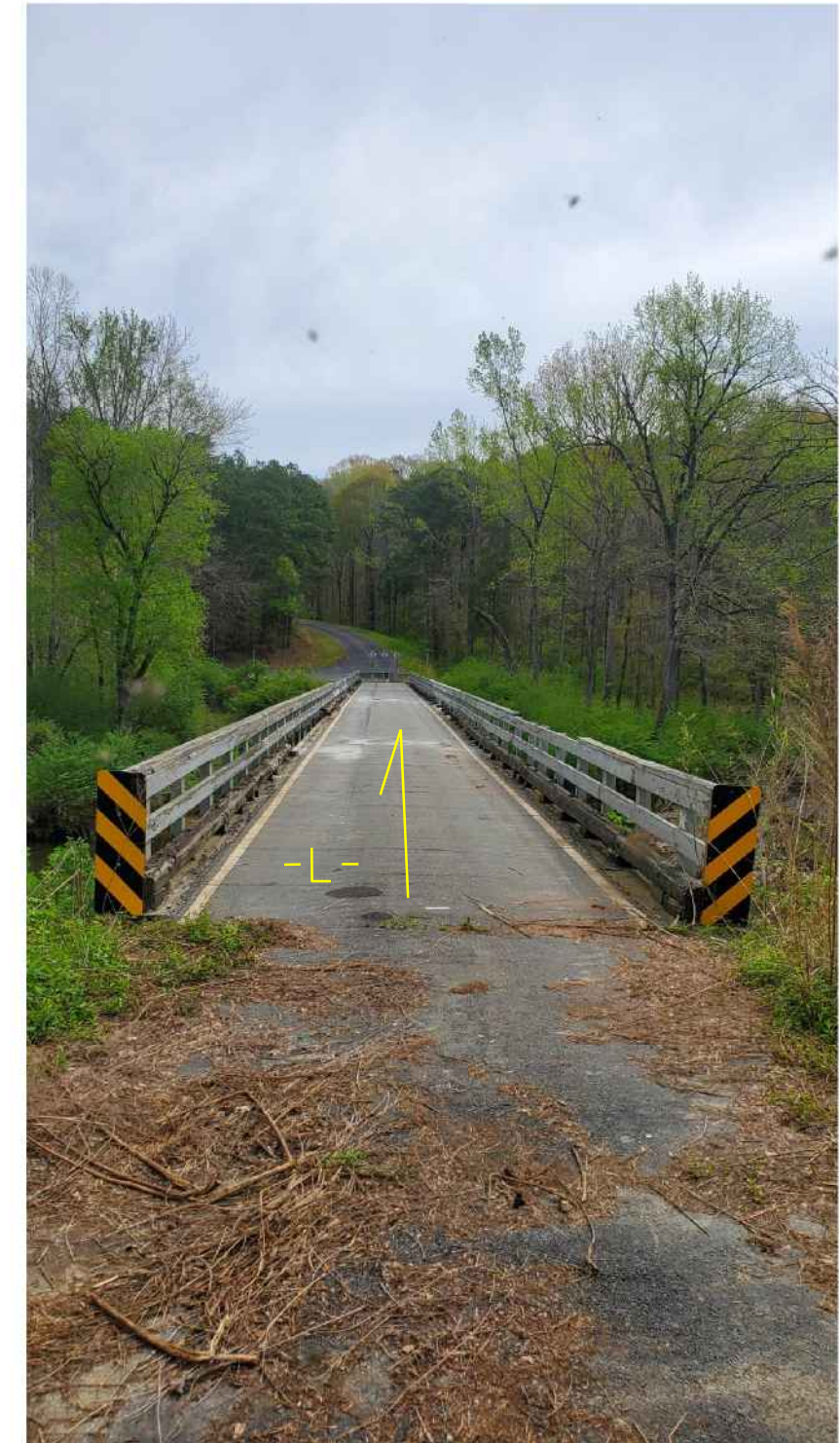
Photo #3: End Bent 1 looking north/northeast (upstation)
