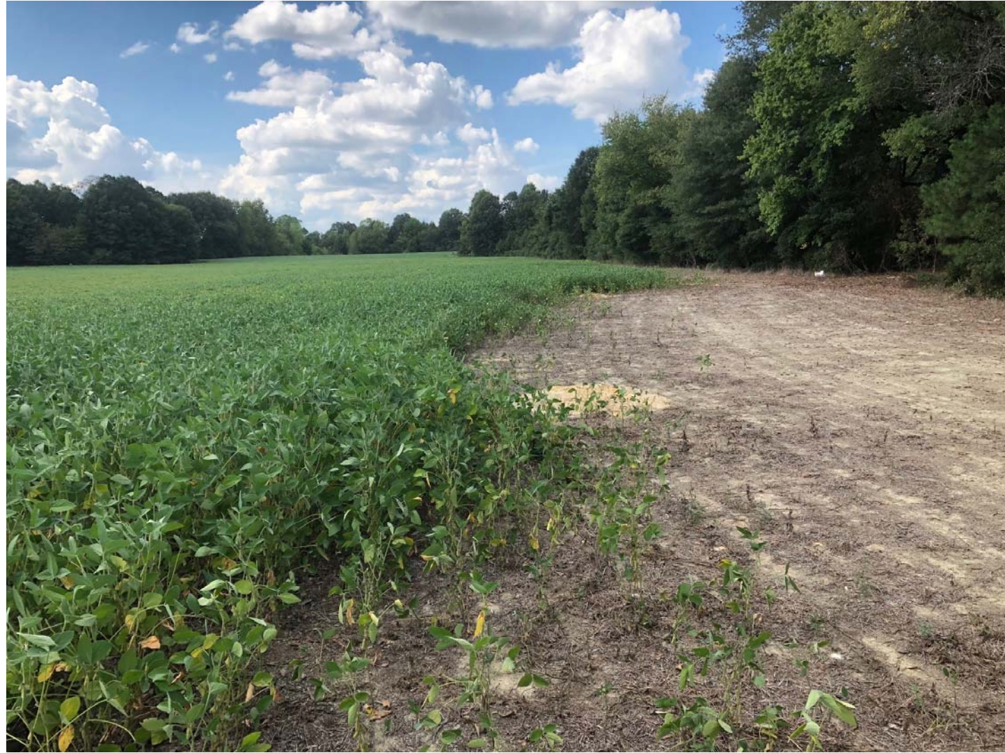
END BENT 1, LOOKING FROM RT TO LT.
