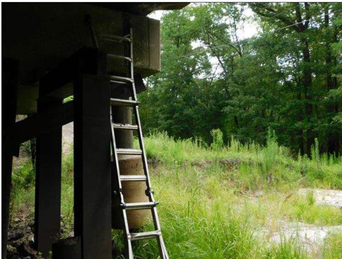
LADDER USED FOR INSPECTION
