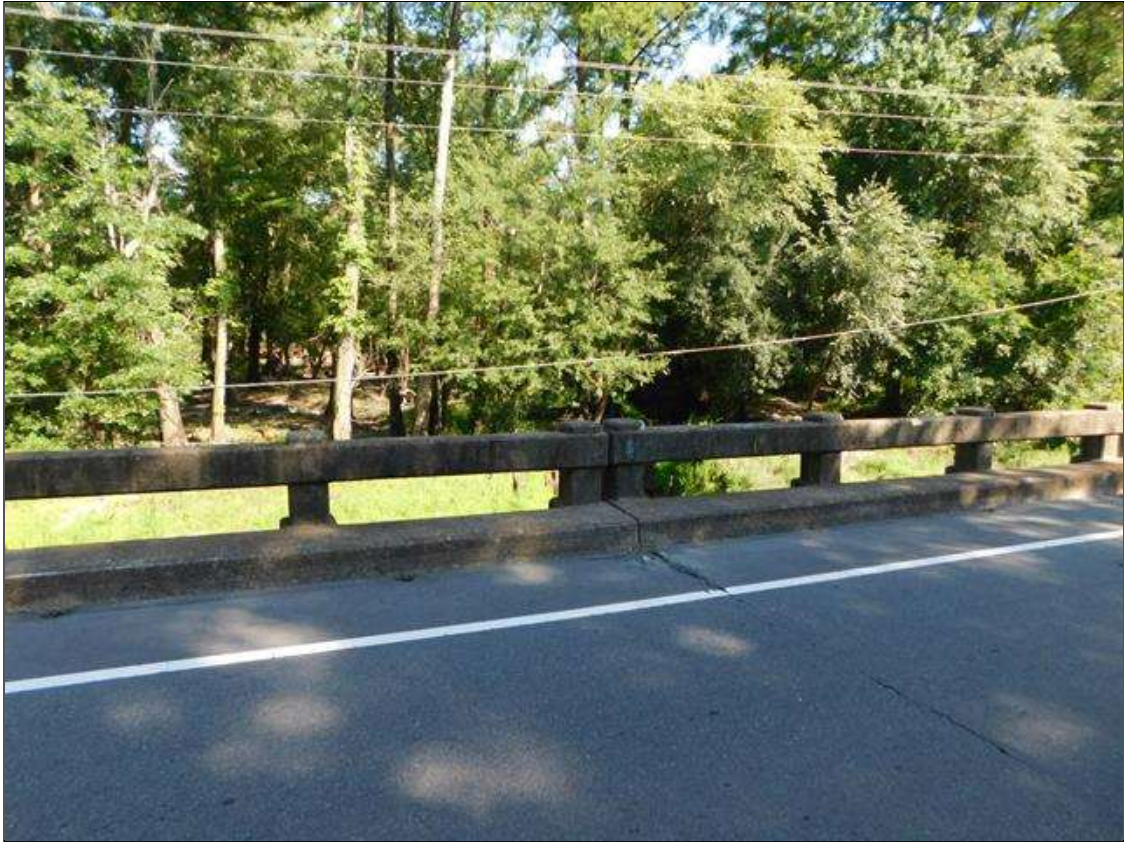
FROM BRIDGE LOOKING EAST DOWNSTREAM
