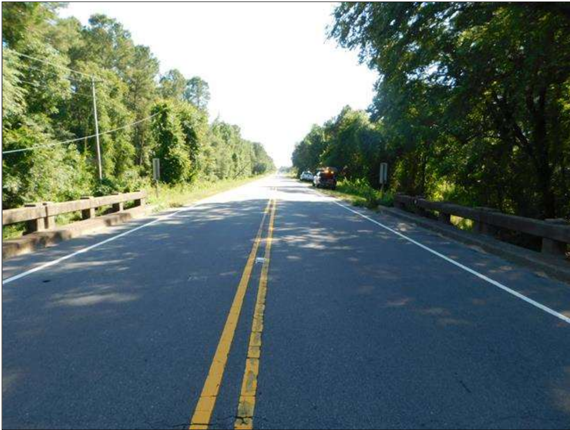
FROM BRIDGE LOOKING SOUTH
