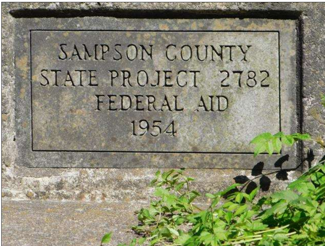
BRIDGE ID PLATE
