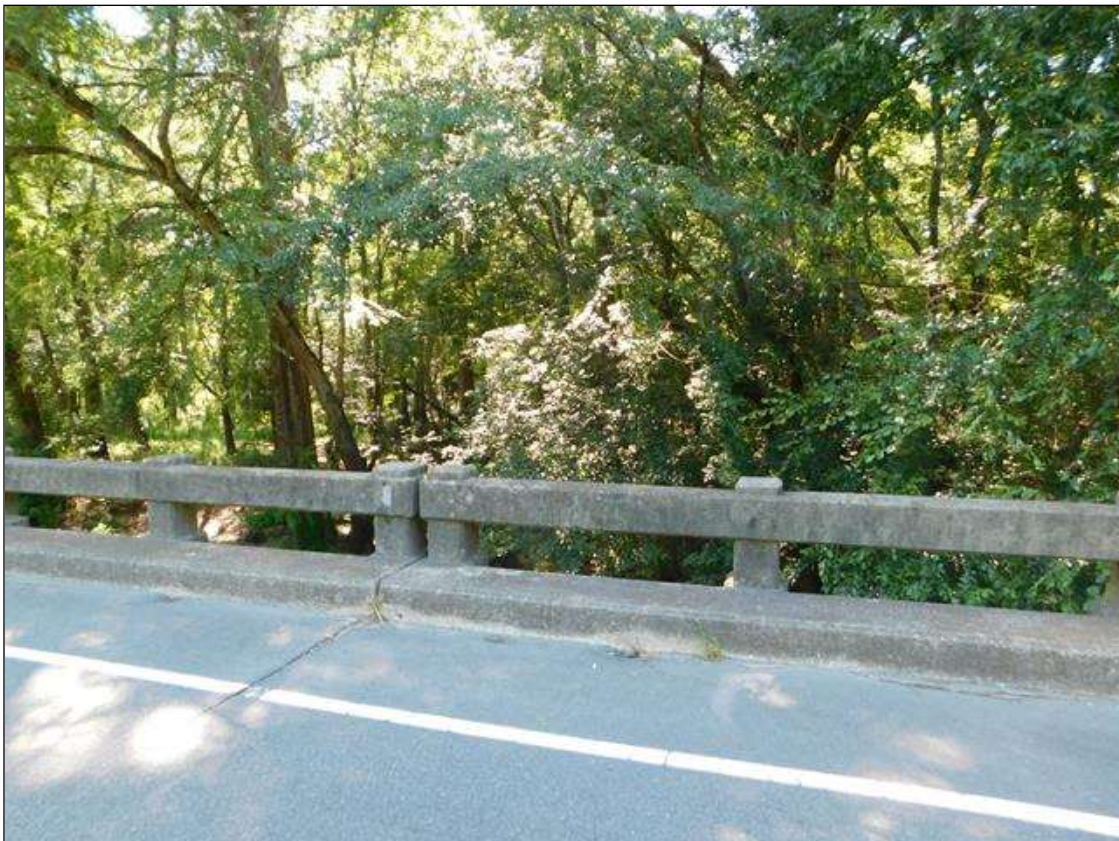
FROM BRIDGE LOOKING WEST UPSTREAM
