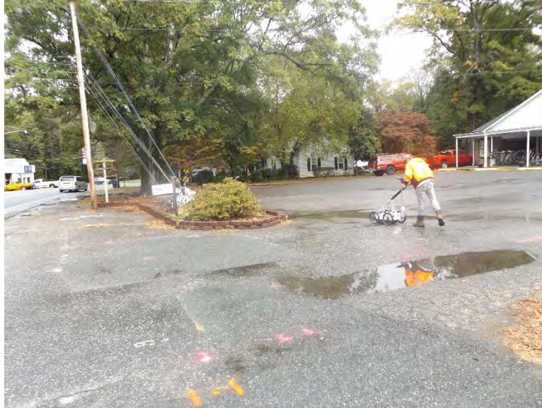
Photograph 2. Paved and landscaped investigation area.
