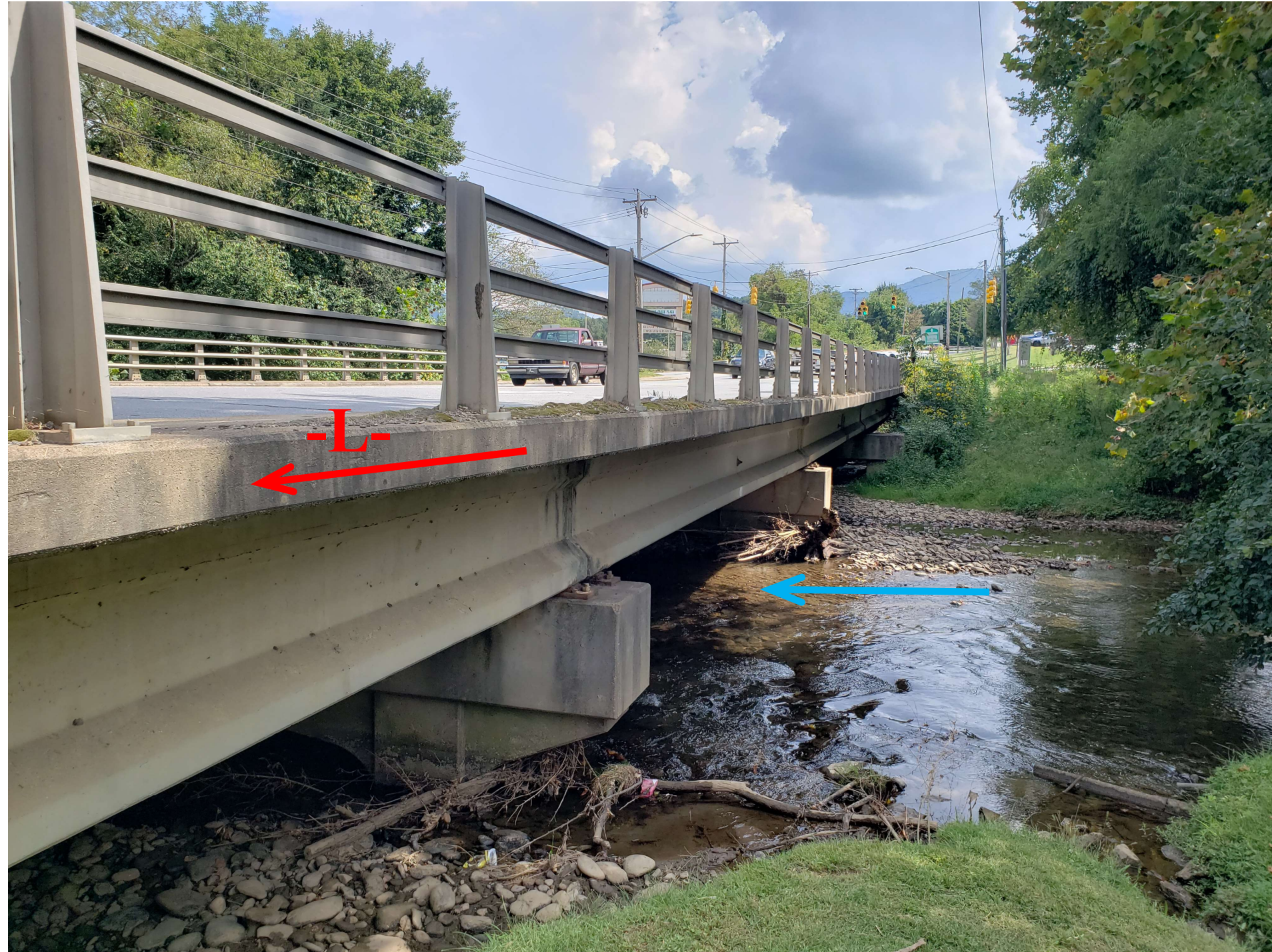
Bridge No. 186 on -L- (US 276) over Richland Creek
