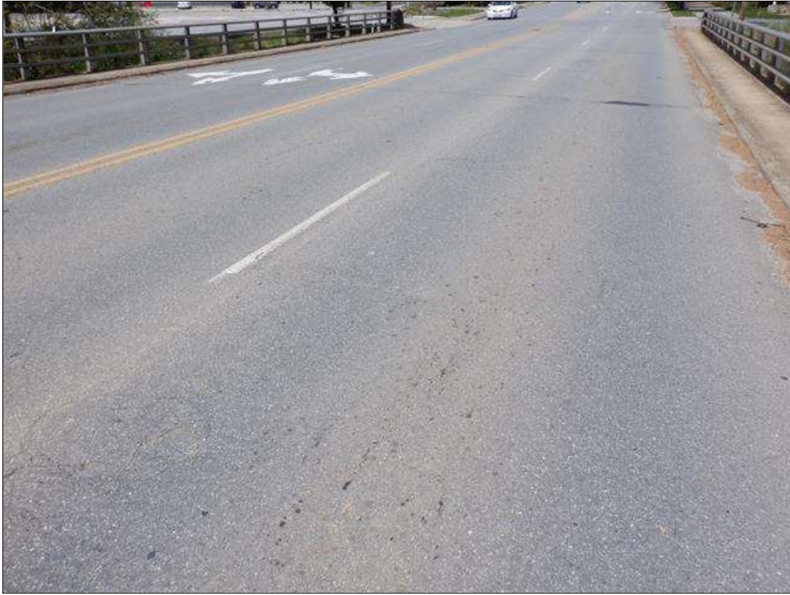
SPAN 2 ASPHALT WEARING SURFACE LOOKING NORTH
