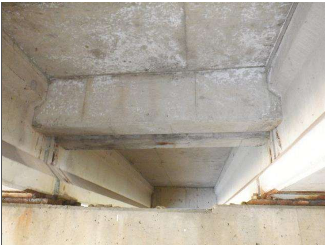
BENT 2 BAY 6 DIAPHRAGM LOOKING SOUTH (OTHERS SIMILAR)
