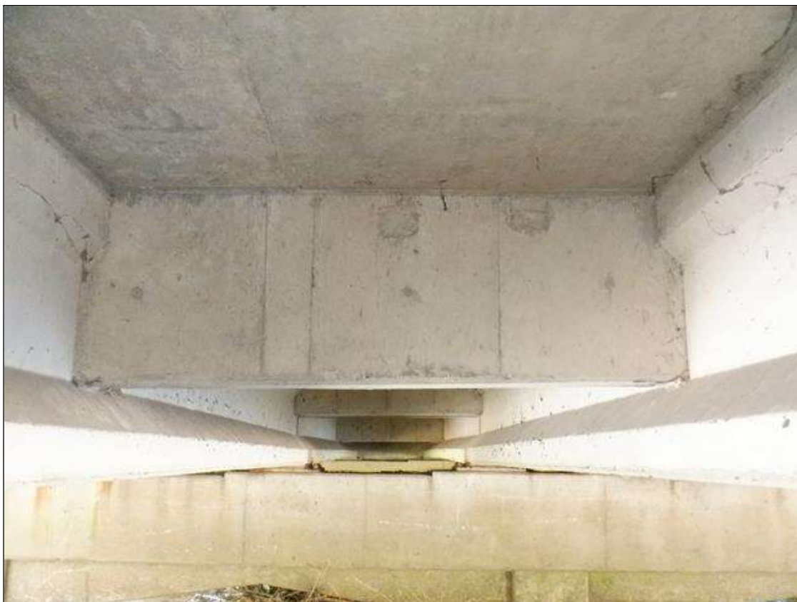
SPAN 3 BAY 3 INTERMEDIATE DIAPHRAGM LOOKING NORTH (OTHERS SIMILAR)
