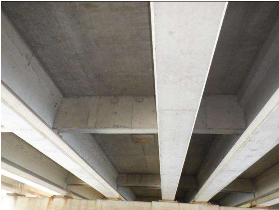
SPAN 3 SUPERSTRUCTURE UNDERSIDE LOOKING NORTH
