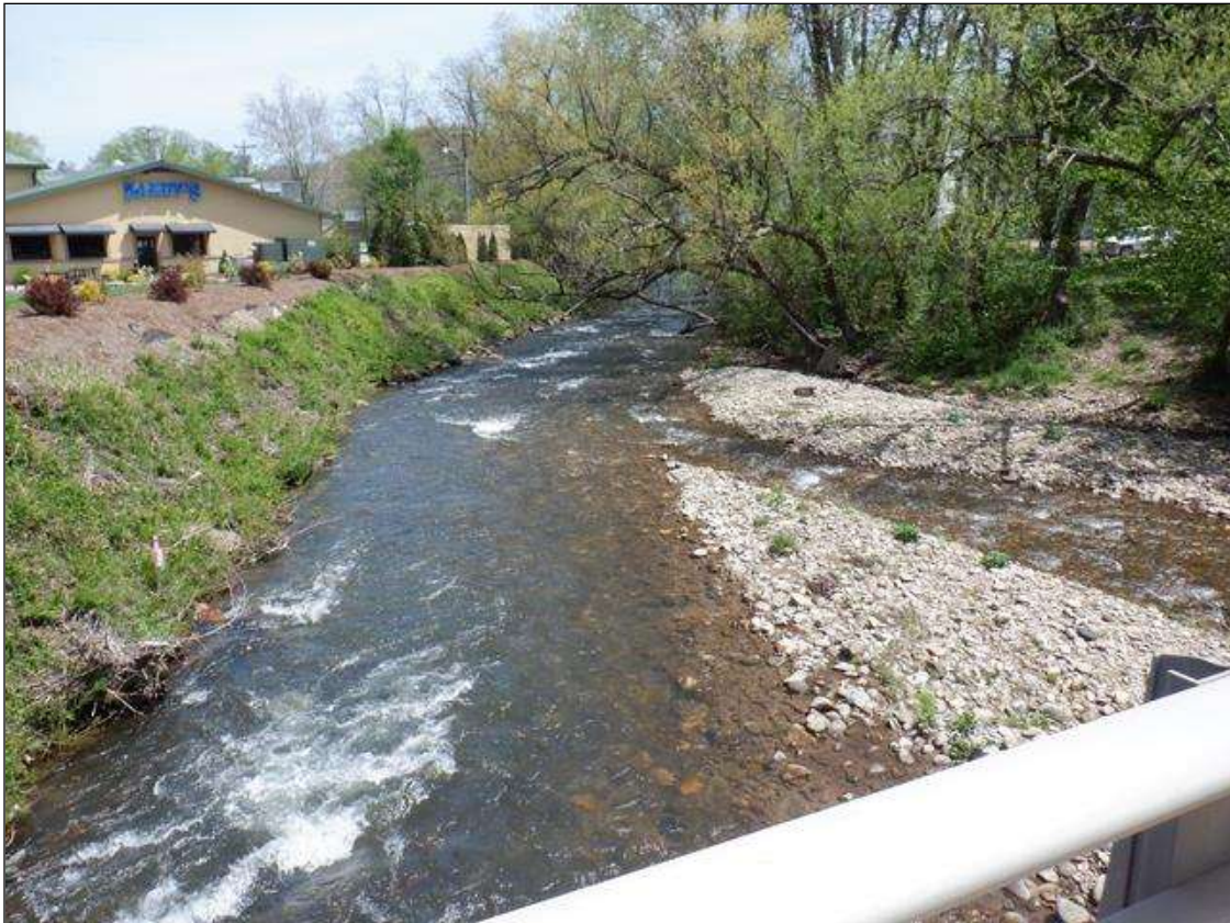
DOWNSTREAM VIEW FROM BRIDGE LOOKING EAST
