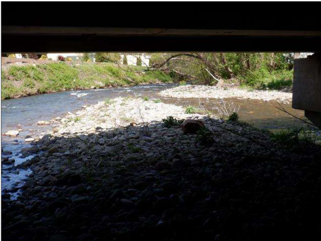
SPAN 3 DOWNSTREAM VIEW LOOKING EAST
