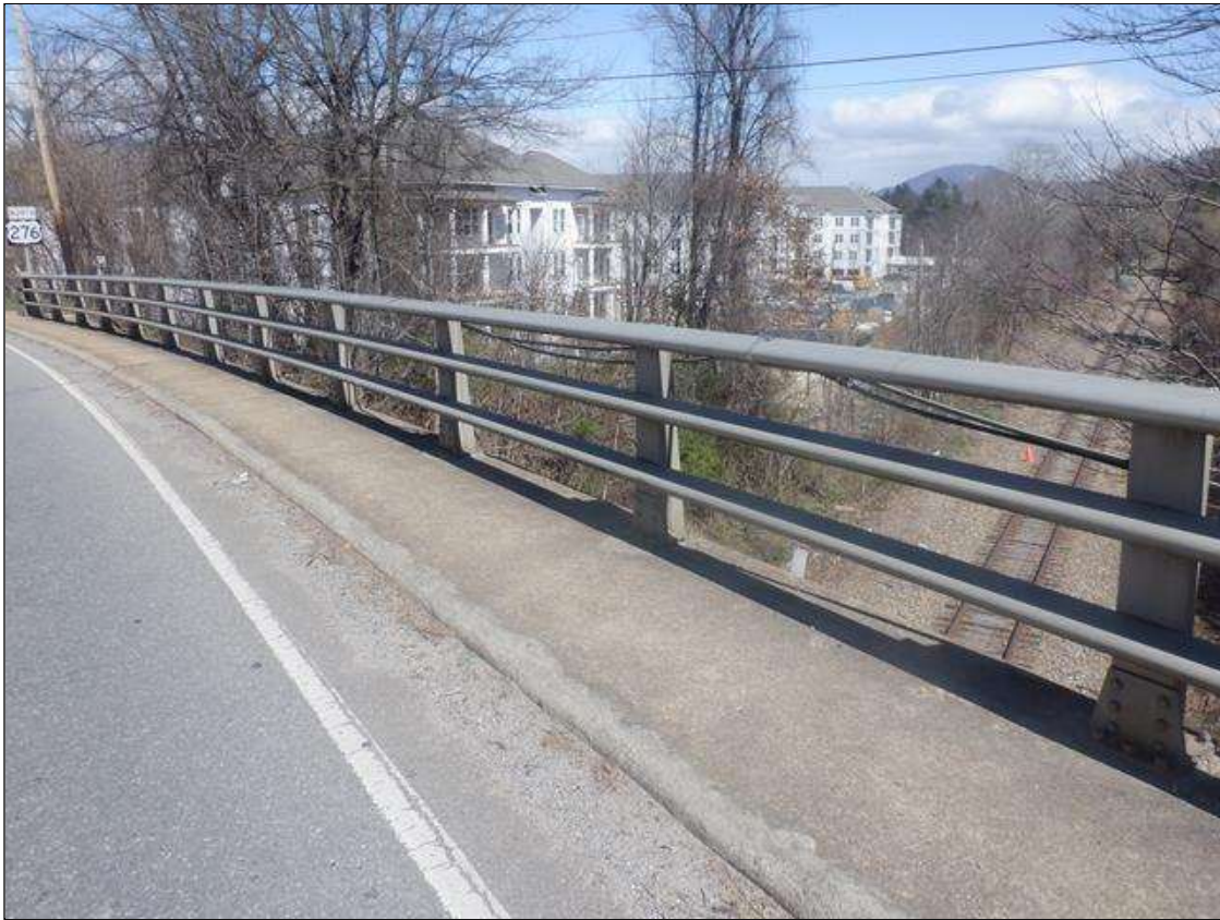
RIGHT BRIDGE RAIL (LEFT BRIDGE RAIL SIMILAR)
