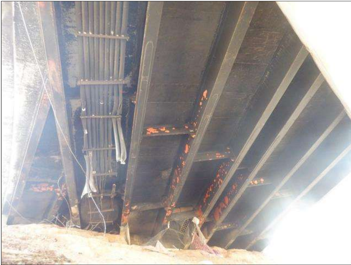
TYPICAL SUPERSTRUCTURE FRAMING AND UNDERSIDE OFF DECK (SPAN 1)
