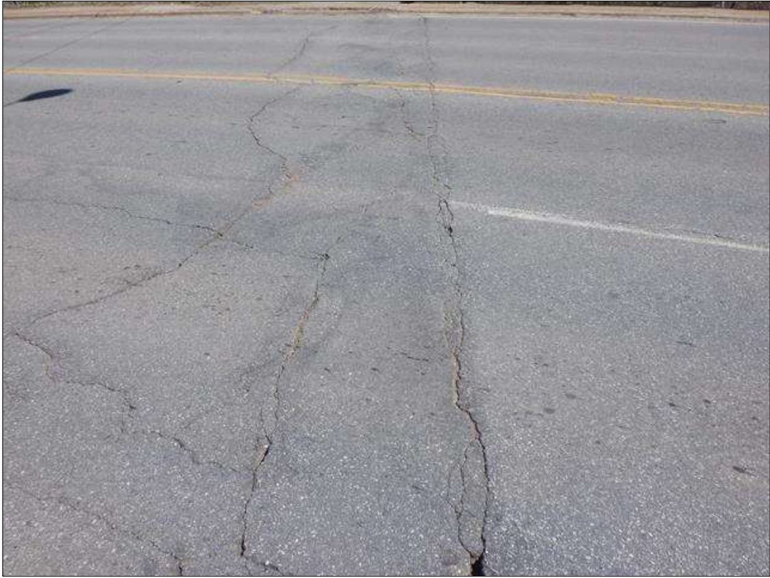
ASPHALT OVER END BENT 2 (ASPHALT OVER END BENT 1 SIMILAR)
