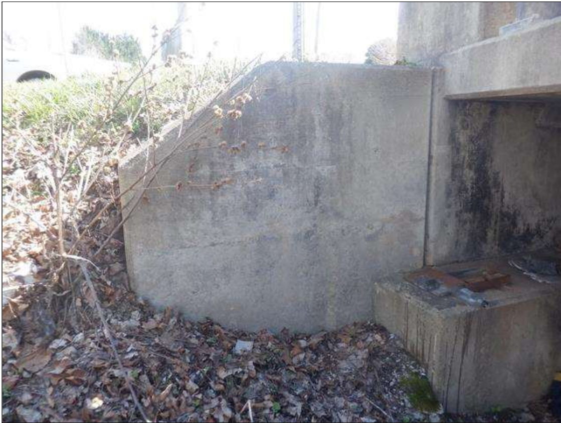
TYPICAL WINGWALL (SOUTHEAST IN VIEW)
