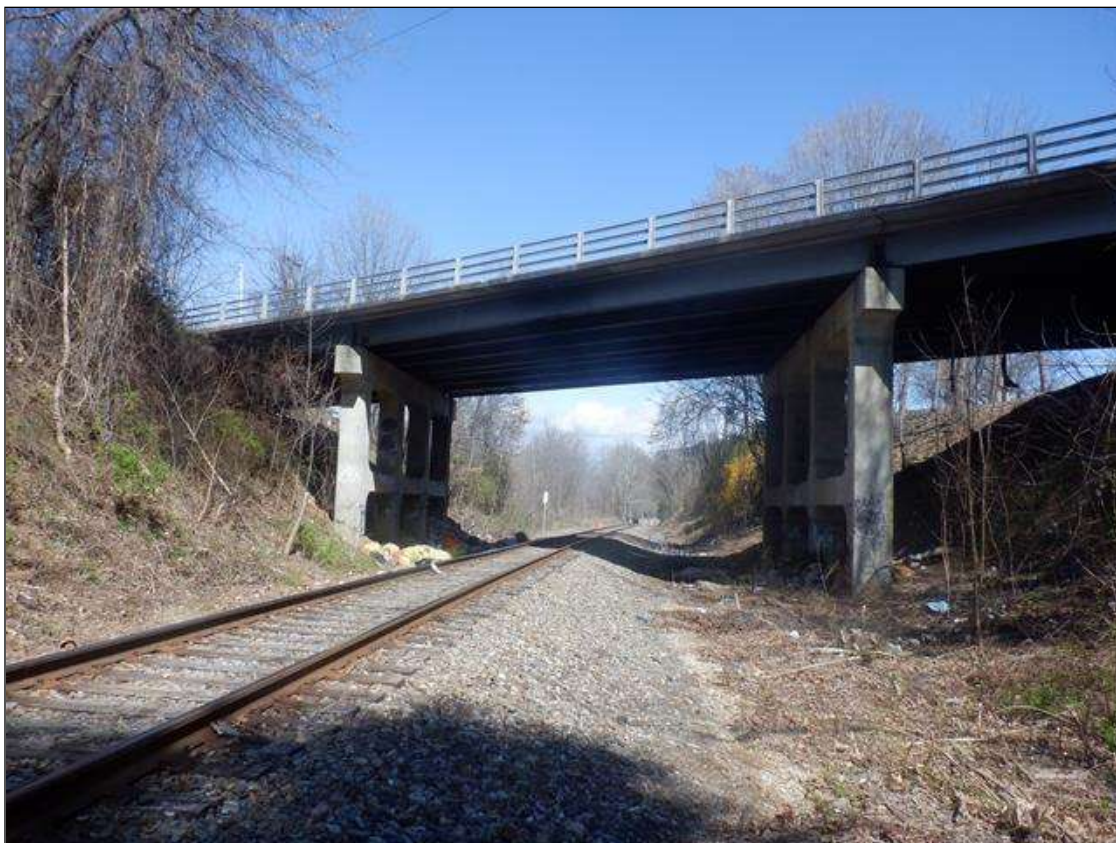
SPAN 2 VERTICAL CLEARANCE LOOKING EAST
