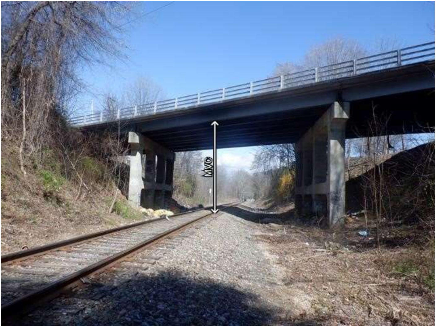
SPAN 2 VERTICAL CLEARANCE LOOKING EAST
