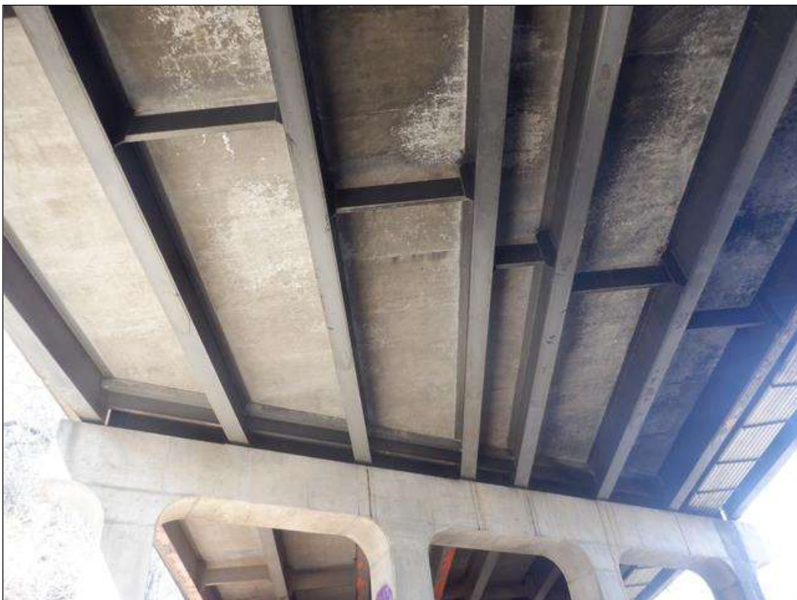
TYPICAL SUPERSTRUCTURE FRAMING AND UNDERSIDE OF DECK (SPAN 2)
