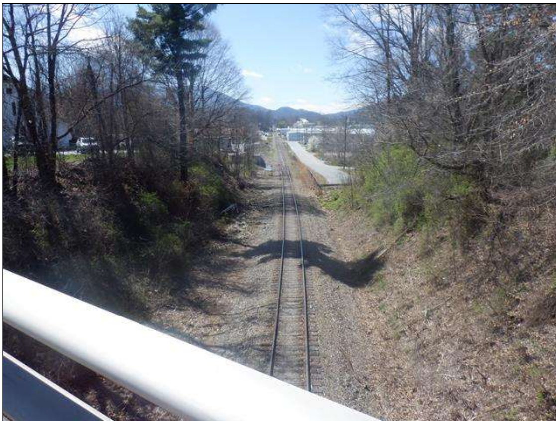
LOOKING WEST FROM BRIDGE
