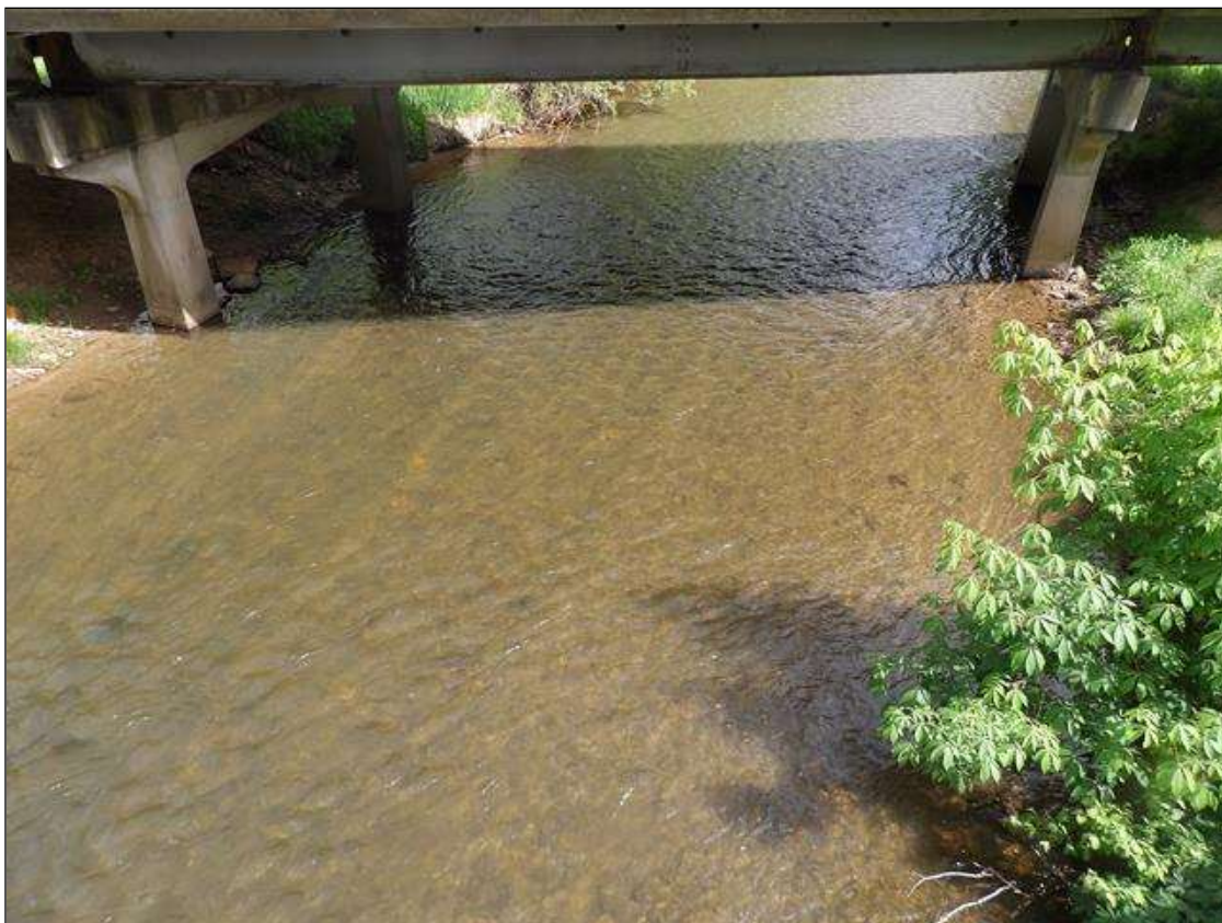
LOOKING EAST UPSTREAM
