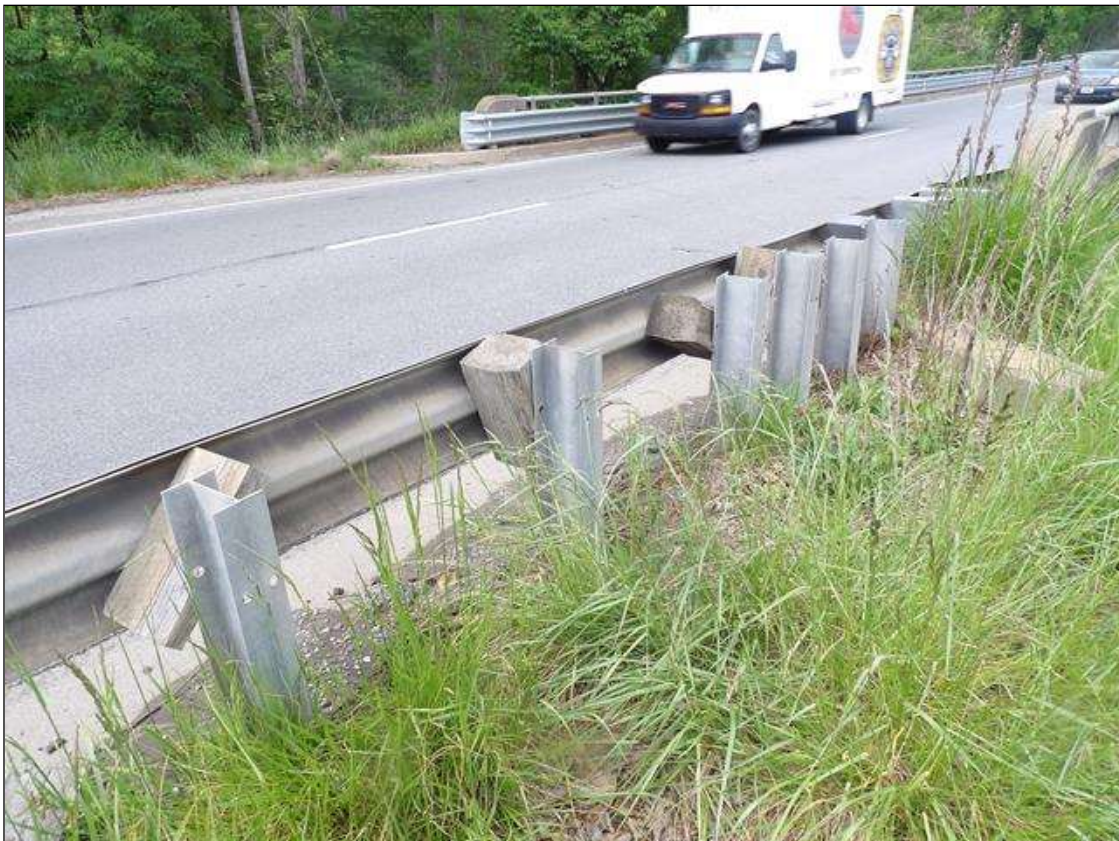
GUARDRAIL POST SPACING AT BRIDGE SOUTHEAST SHOWN NORTHWEST AND NORTHEAST SIMILAR
