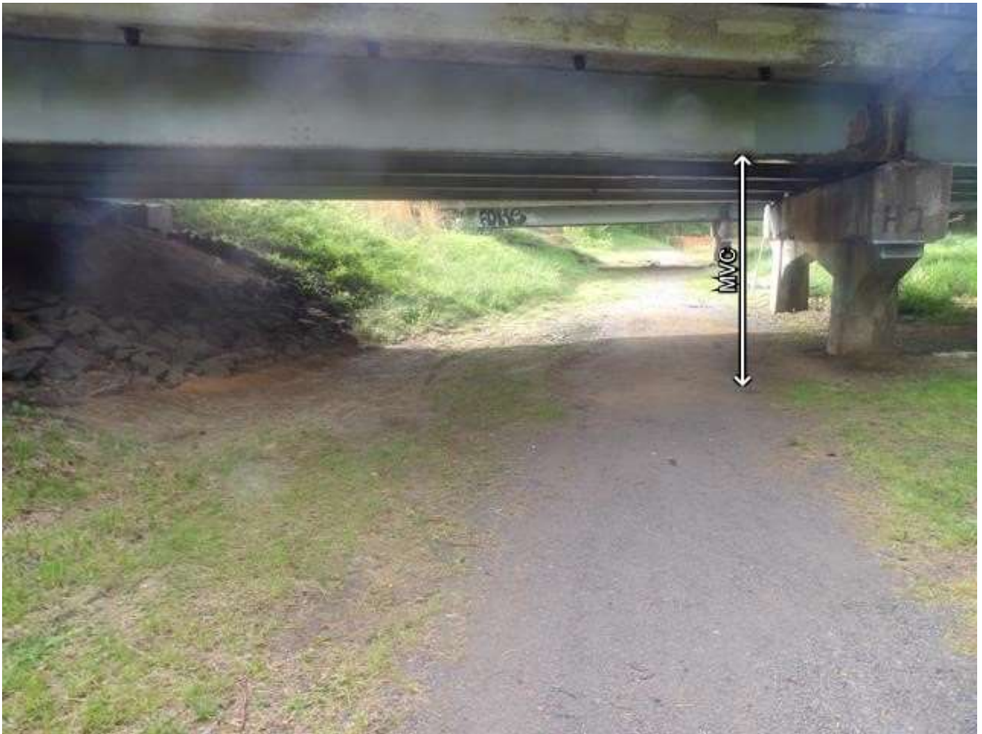
LOOKING EAST THROUGH SPAN 4
