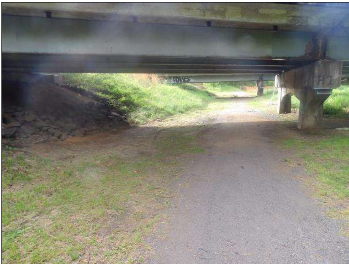
LOOKING EAST THROUGH SPAN 4
