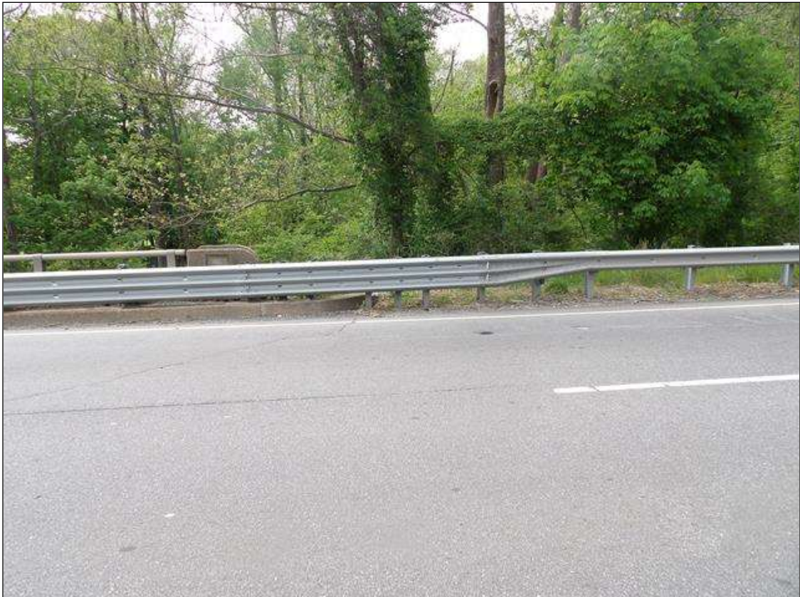
GUARDRAIL TRANSITION TO BRIDGE NORTHWEST CORNER
