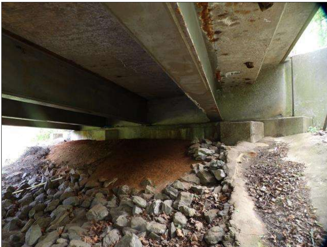
ABUTMENT 1, ABUTMENT 2 SIMILAR
