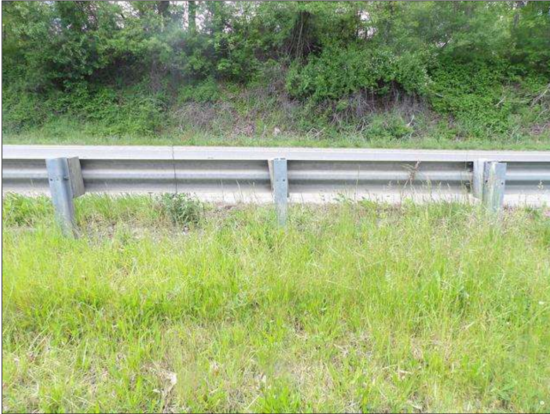
GUARDRAIL POST SPACING MIDWAY SOUTHEAST SHOWN NORTHWEST AND NORTHEAST SIMILAR
