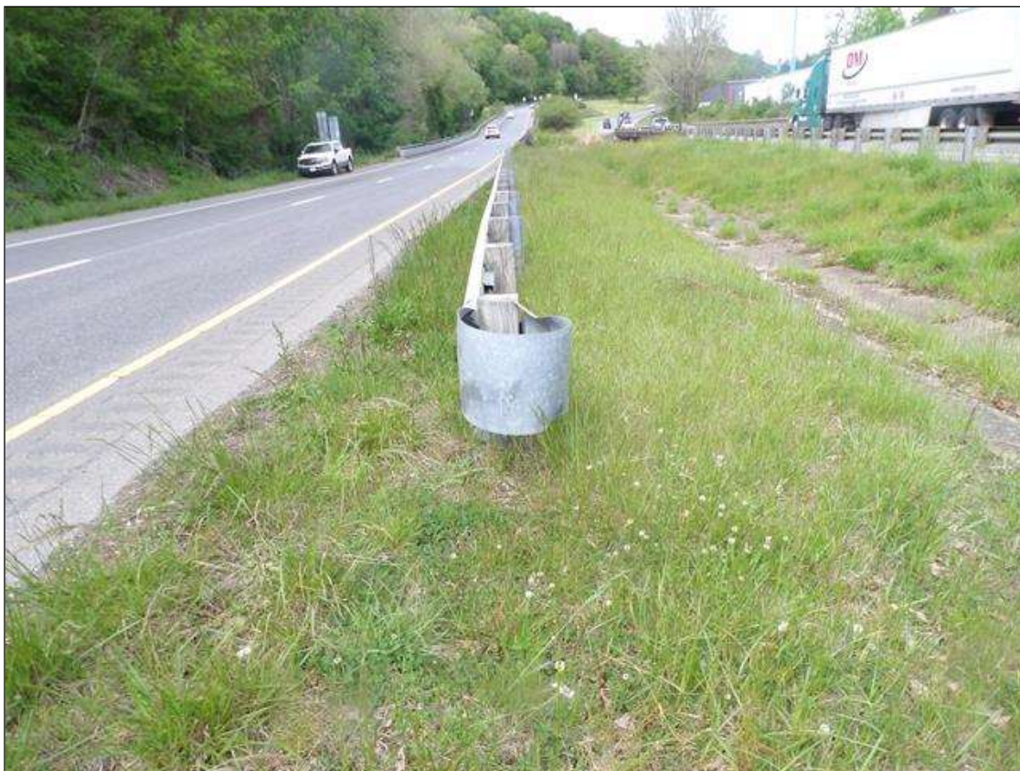
GUARDRAIL TERMINAL END SOUTHEAST CORNER
