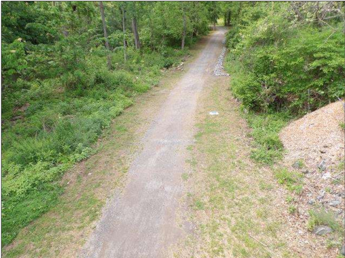
LOOKING WEST SPAN 4
