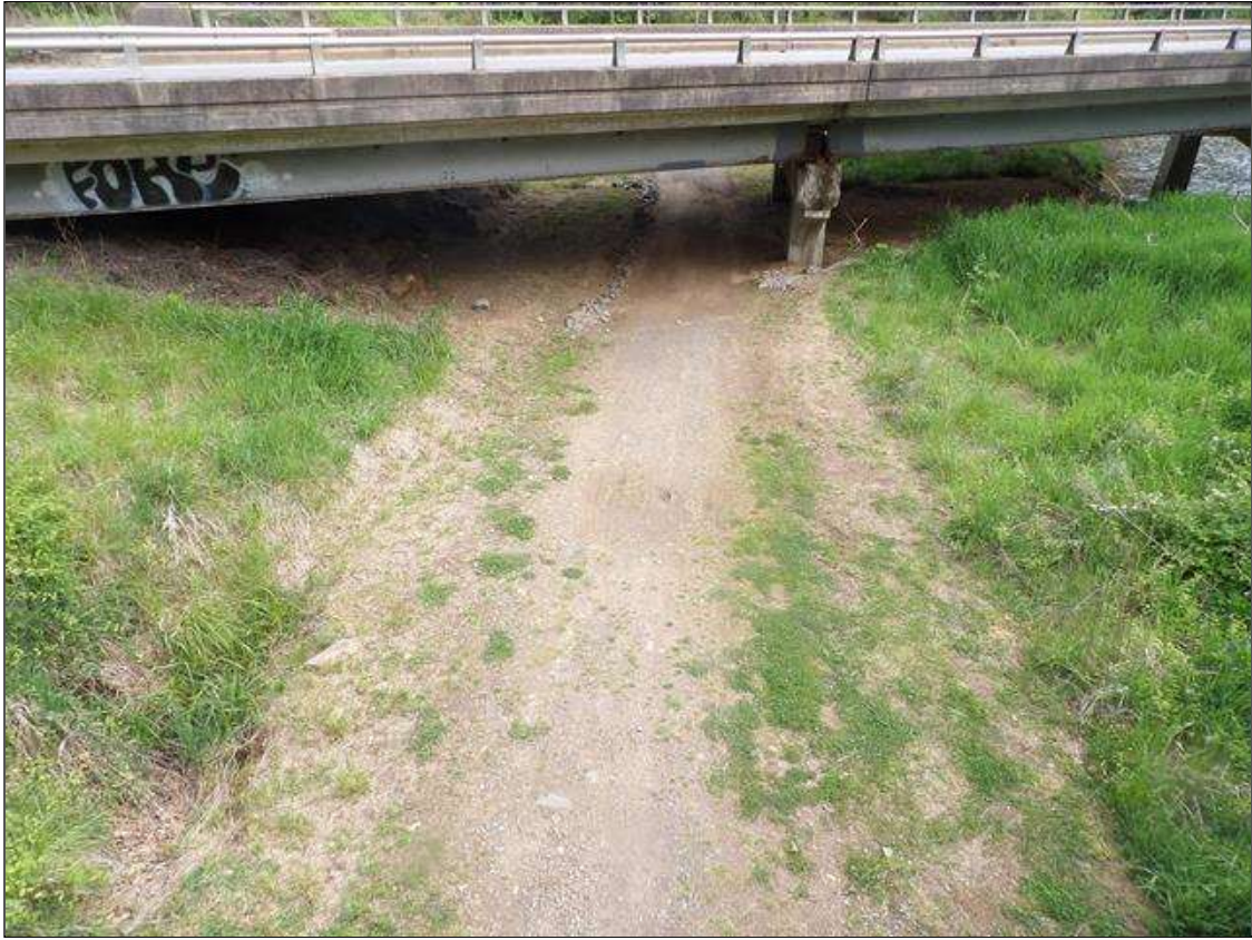
LOOKING EAST SPAN 4
