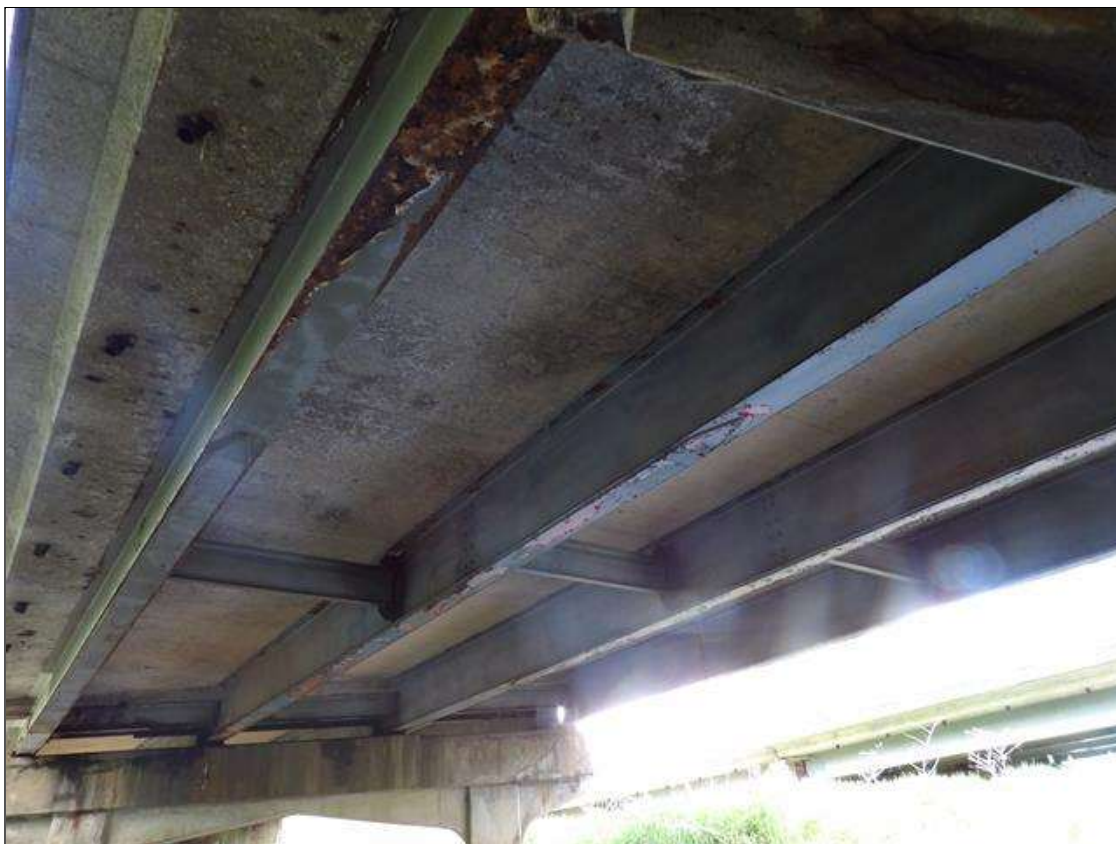
SUPERSTRUCTURE UNDERSIDE SPAN 2, ALL OTHERS SIMILAR
