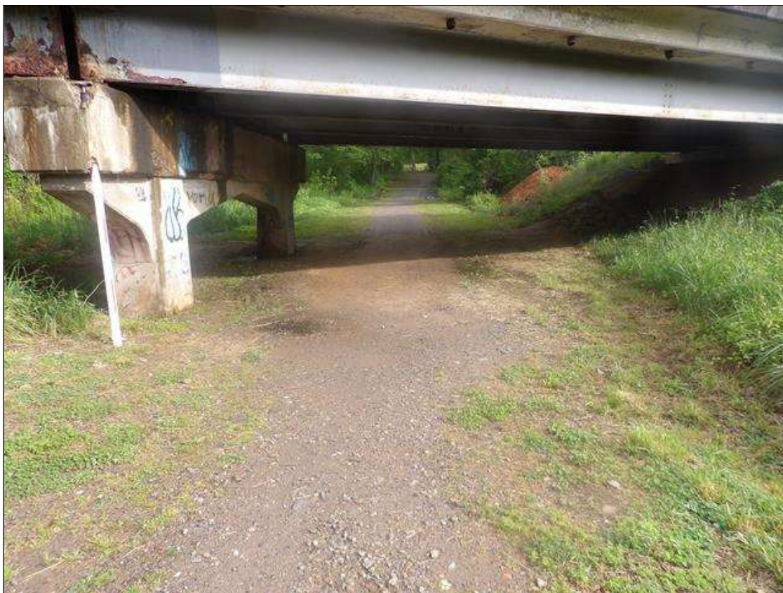
LOOKING WEST THROUGH SPAN 4
