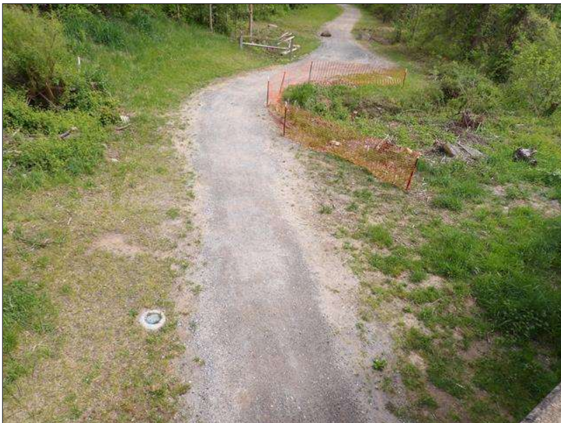
LOOKING EAST FROM SPAN 4
