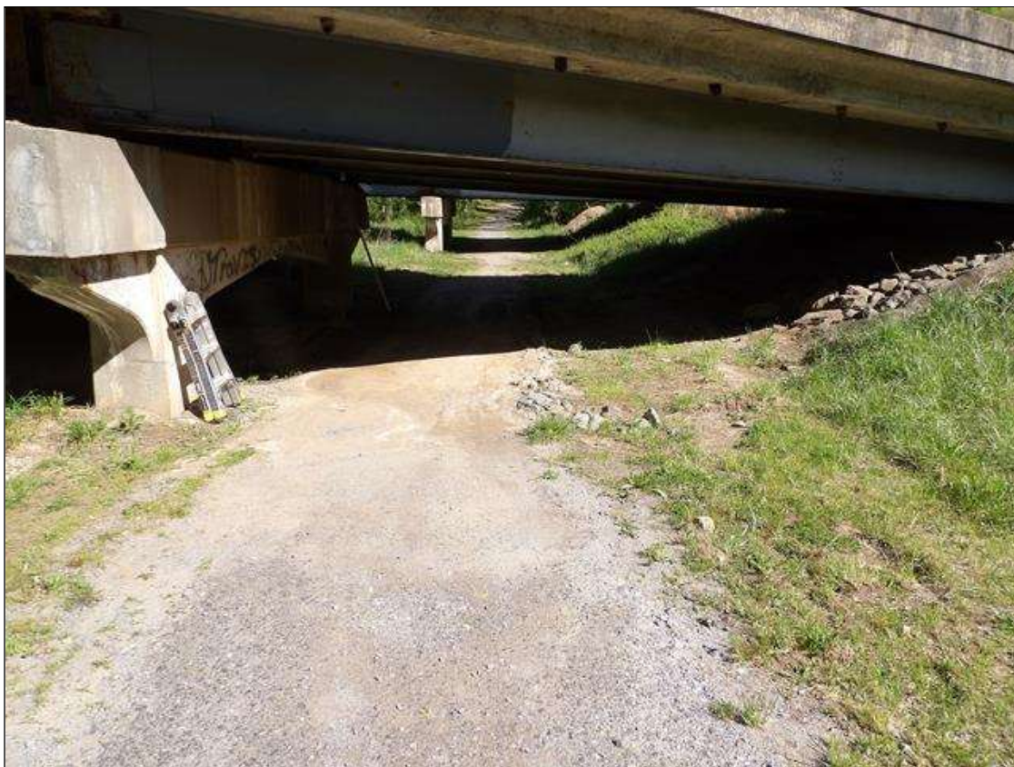
LOOKING WEST THROUGH SPAN 4
