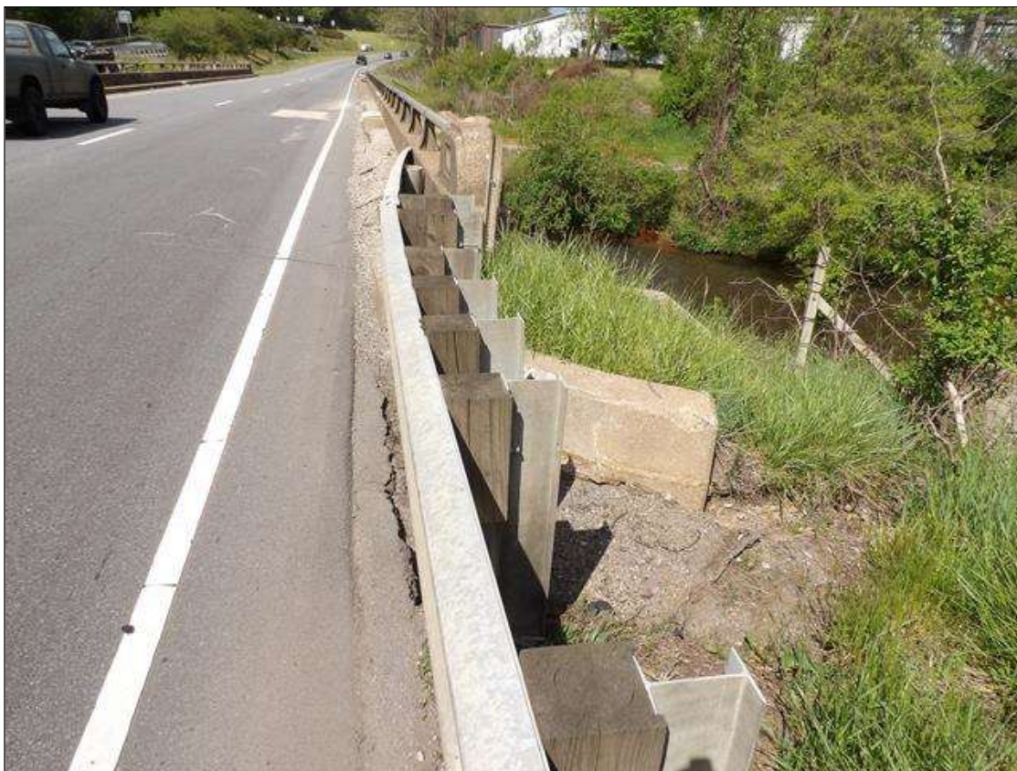
GUARDRAIL POST SPACING AT BRIDGE SOUTHEAST SHOWN SOUTHWEST AND NORTHEAST SIMILAR
