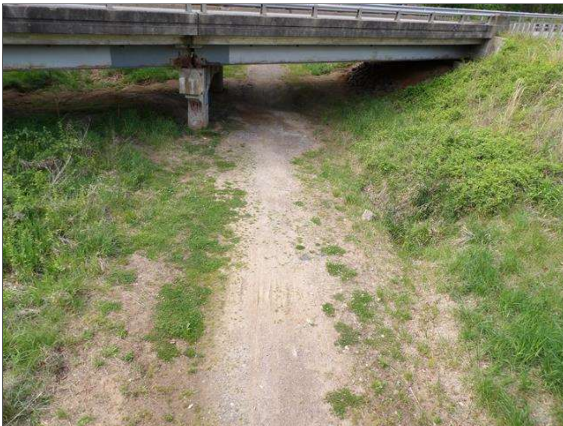
LOOKING WEST FROM SPAN 4
