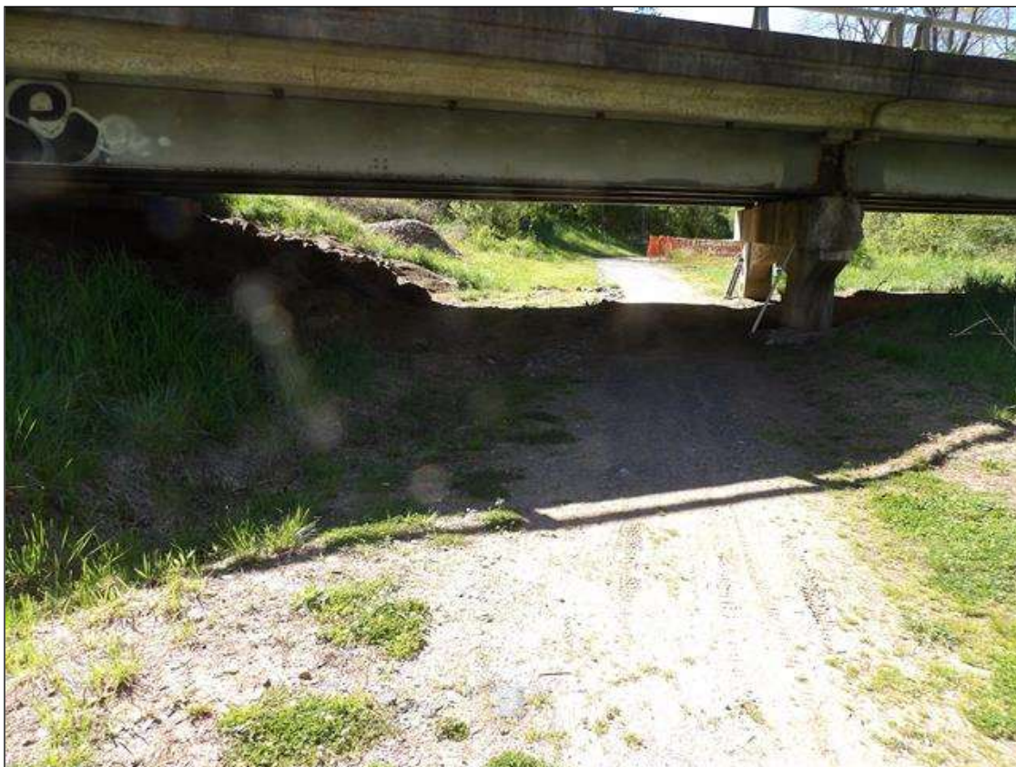
LOOKING EAST THROUGH SPAN 4
