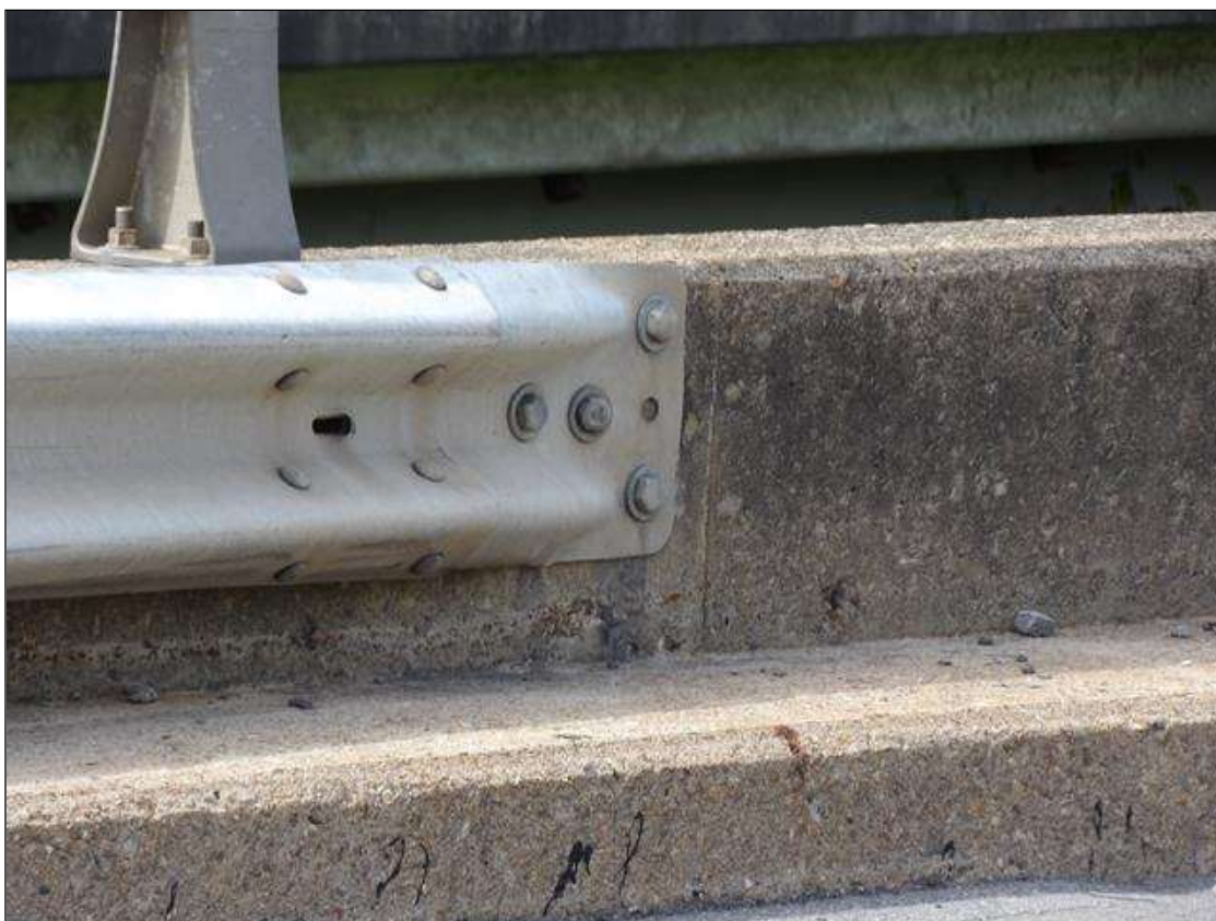
GUARDRAIL ATTACHMENT TO BRIDGE SOUTHWEST SHOWN SOUTHEAST AND NORTHEAST SIMILAR
