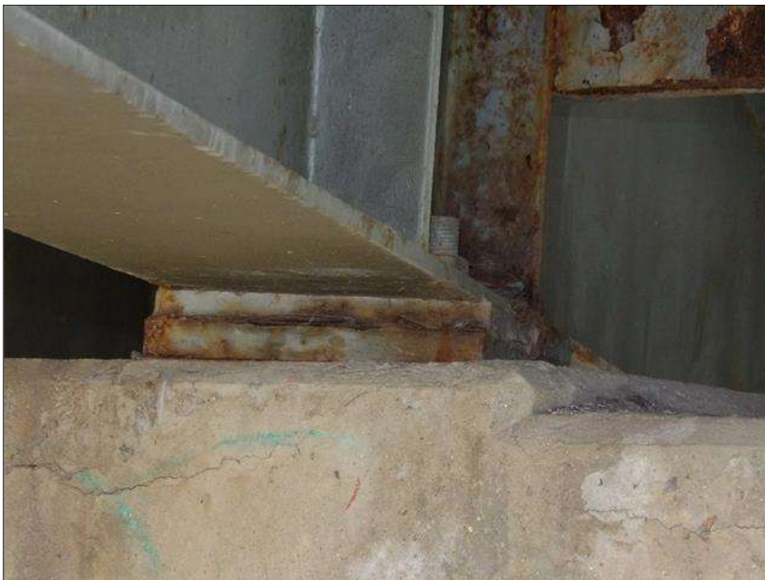
TYPICAL BEARING BEAM 3 AT PIER 3 SPAN 3 SHOWN
