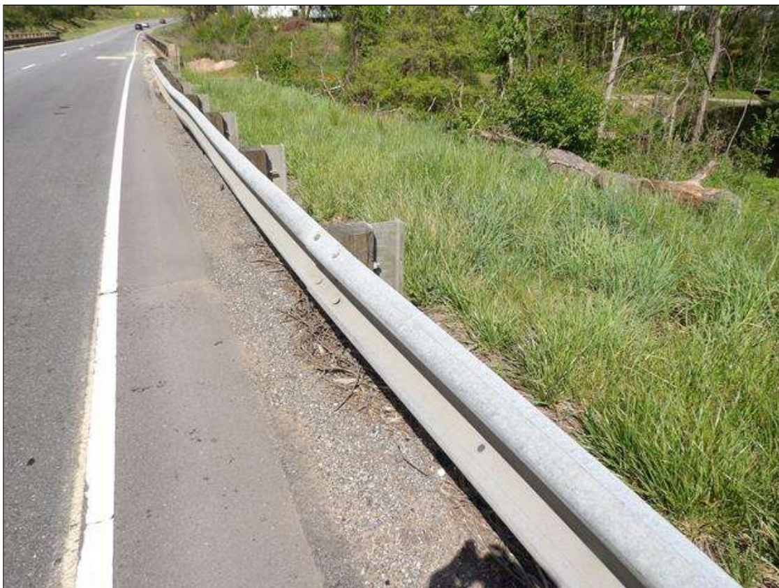
GUARDRAIL POST SPACING MIDWAY SOUTHEAST SOUTHWEST AND NORTHEAST SIMILAR
