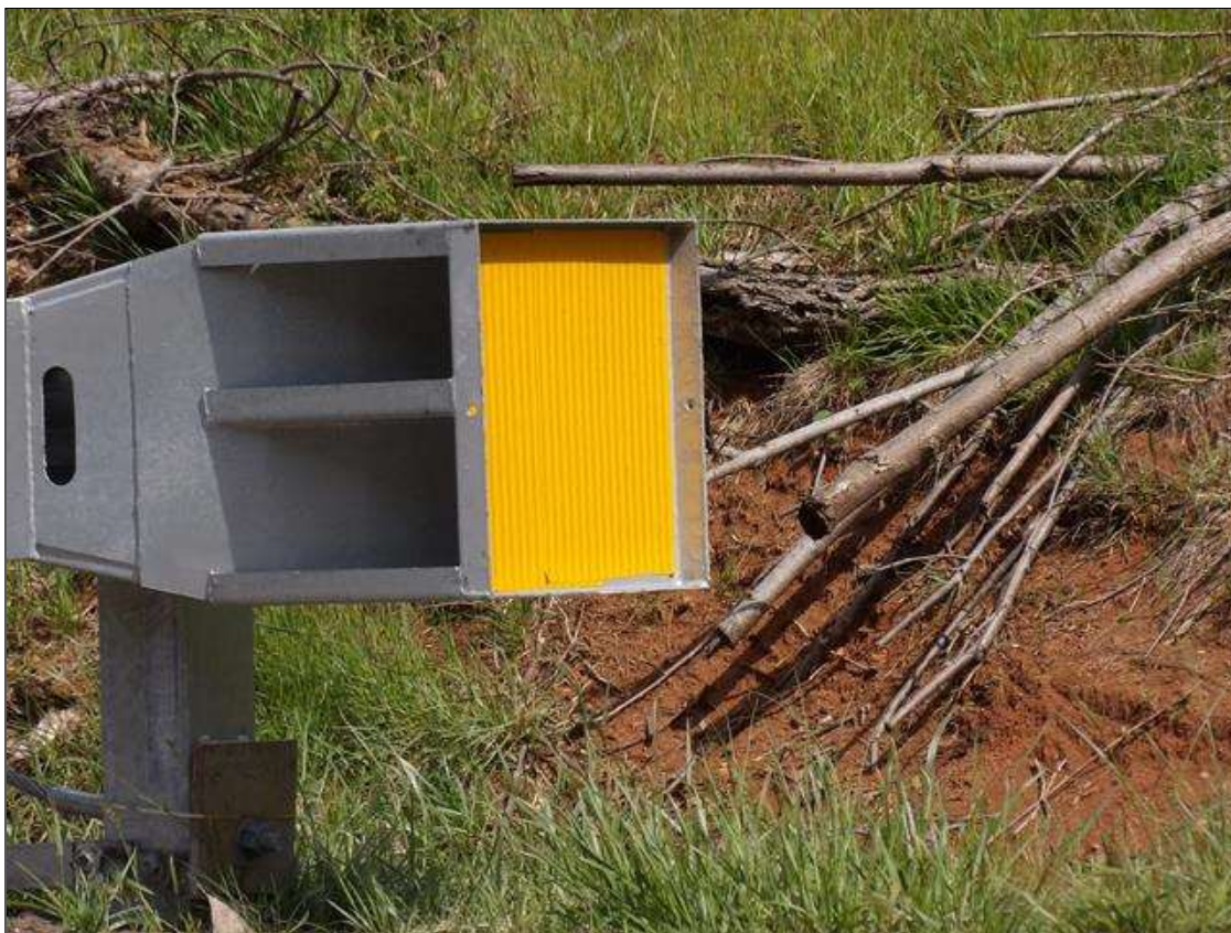
GUARDRAIL TERMINAL END SOUTHEAST CORNER
