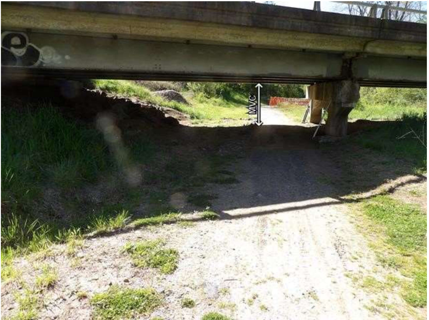
LOOKING EAST THROUGH SPAN 4
