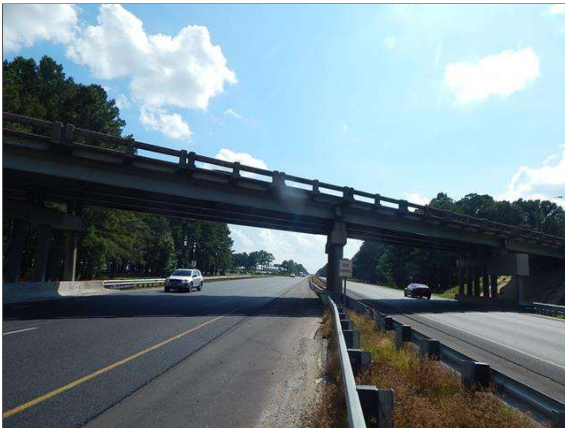
North profile, looking South
