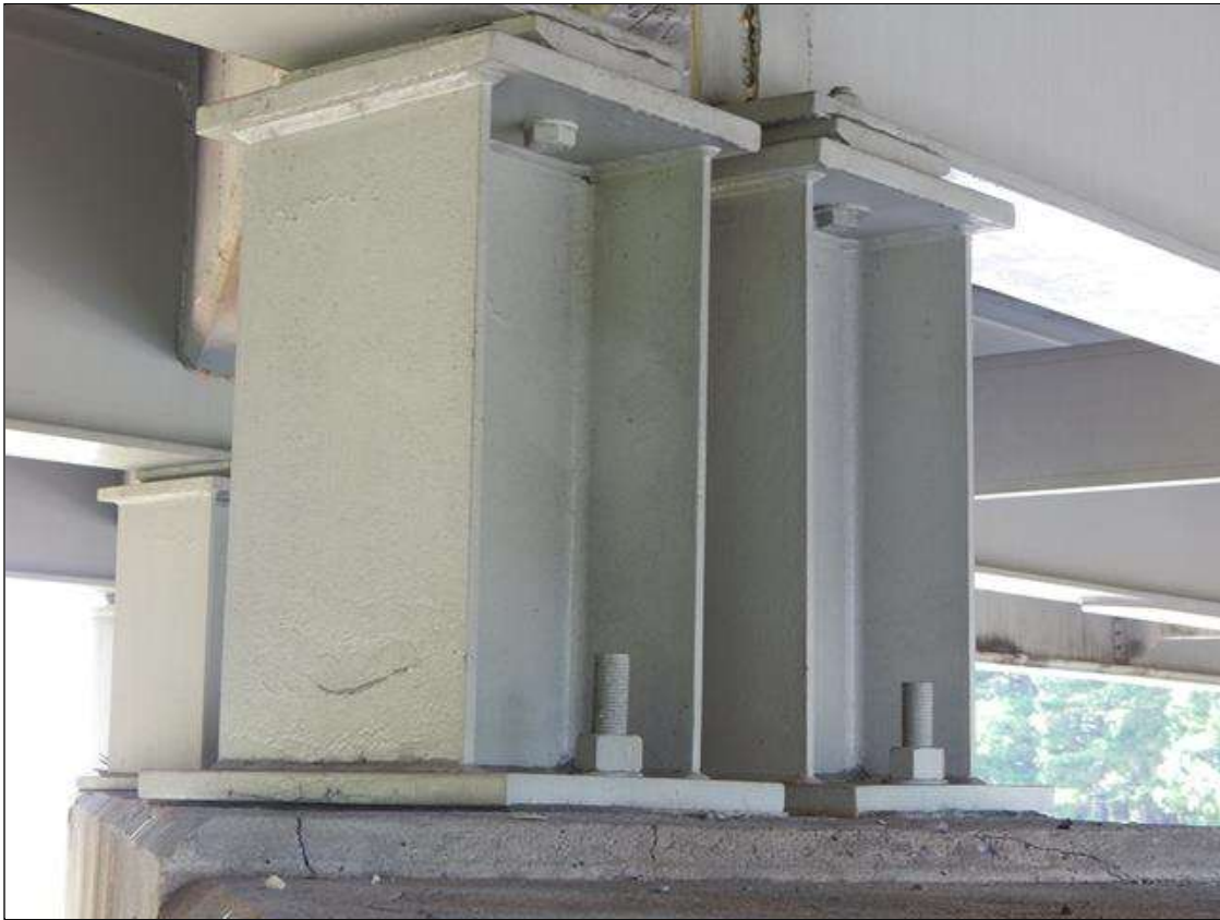
Bent bearing (Beam 2, Bent 3 shown)
