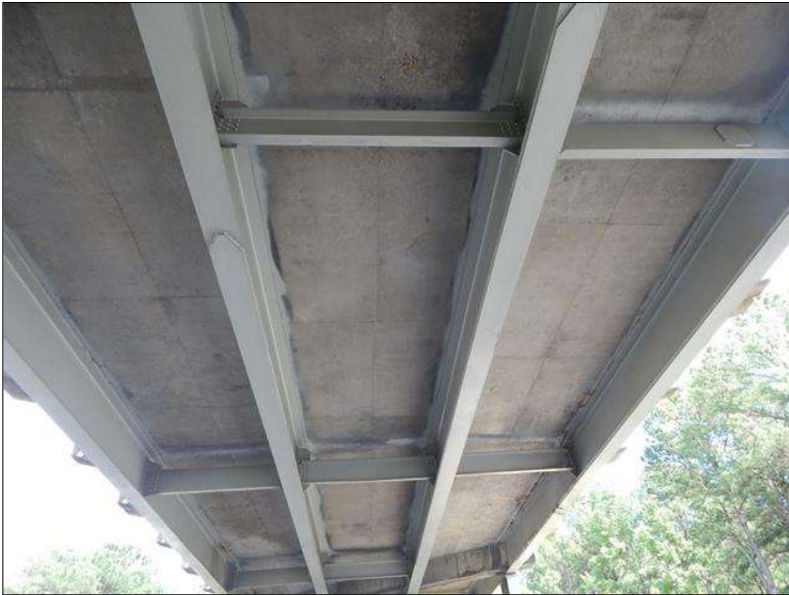
Underside of superstructure (Span 3 shown)
