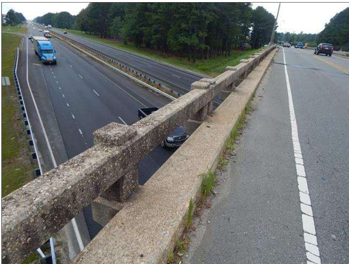
South bridge rail (North bridge rail similar)
