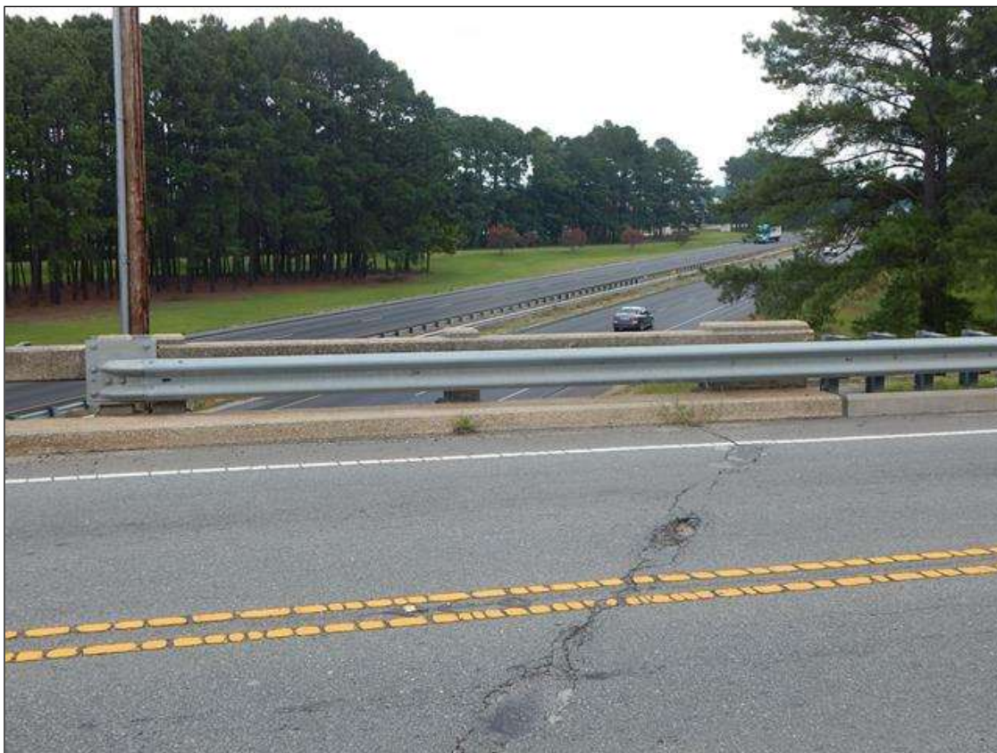
Northeast guardrail attachment (All others similar)
