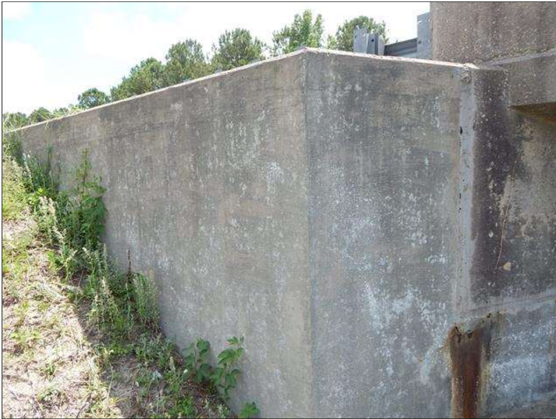
Northeast wingwall (All others similar)
