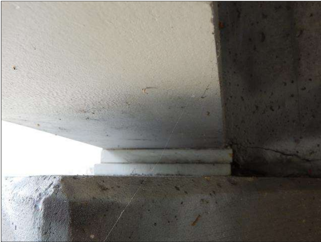
End Bent bearing (Beam 4, End Bent 1 shown)
