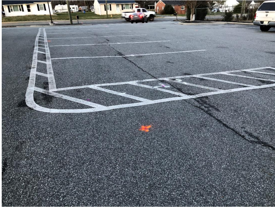
Photo 11: Looking north across parking lot towards Old Hollow Rd. showing unknown utilities and a proposed boring location.
