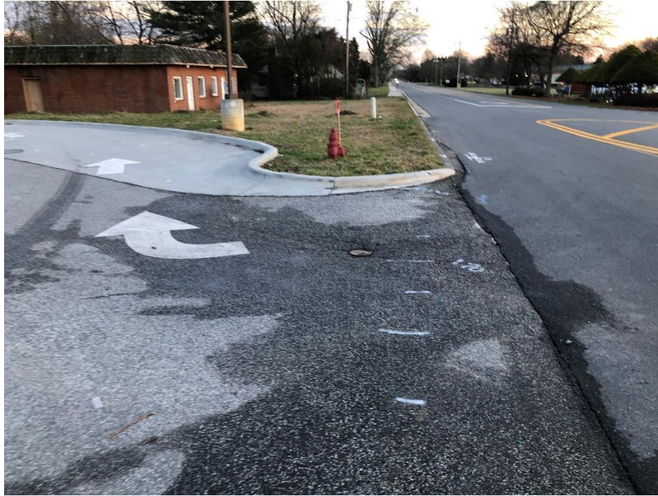
Photo 5: Looking southeast along Darrow Rd. showing utility features.
