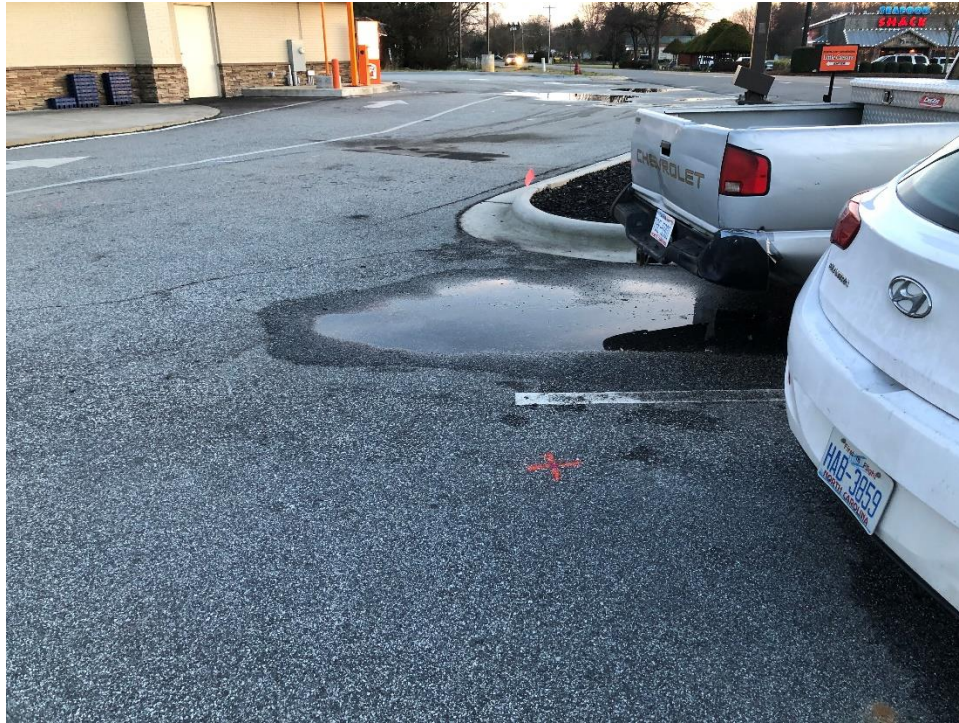
Photo 3: Looking southeast from west parking spaces.
