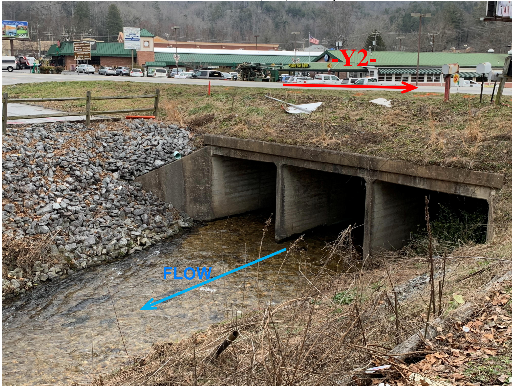
Culvert No. 0099 on -Y2- (US 64) over Turkey Creek
