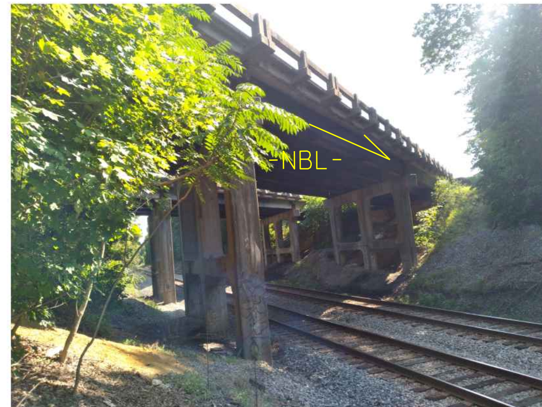
PHOTO #4: END BENT 1 OF EXISTING BRIDGE 164 LOOKING EAST (UPSTATION)
