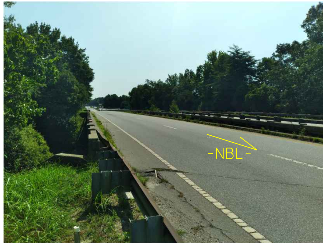
PHOTO #1: END BENT 2 OF EXISTING BRIDGE 164 LOOKING WEST (DOWNSTATION)
