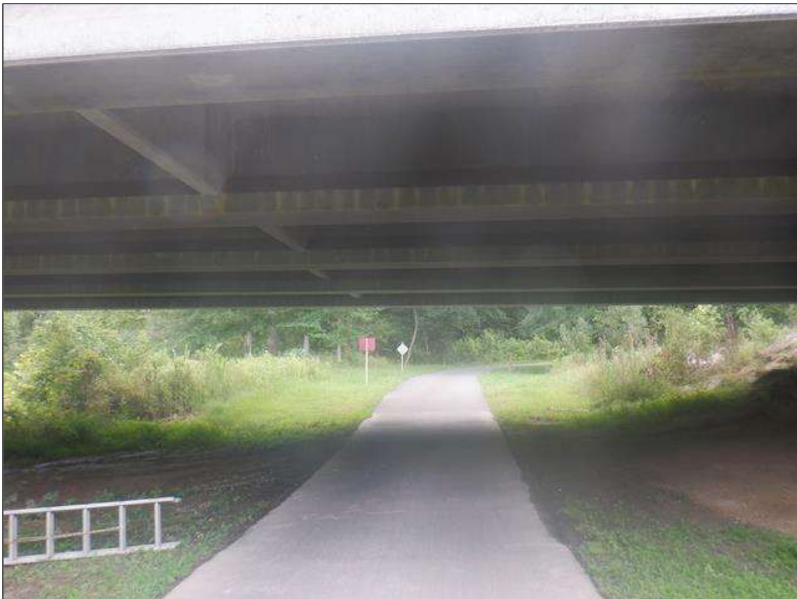
WEST UNDERCLEARANCE PROFILE LOOKING EAST IN SPAN 1
