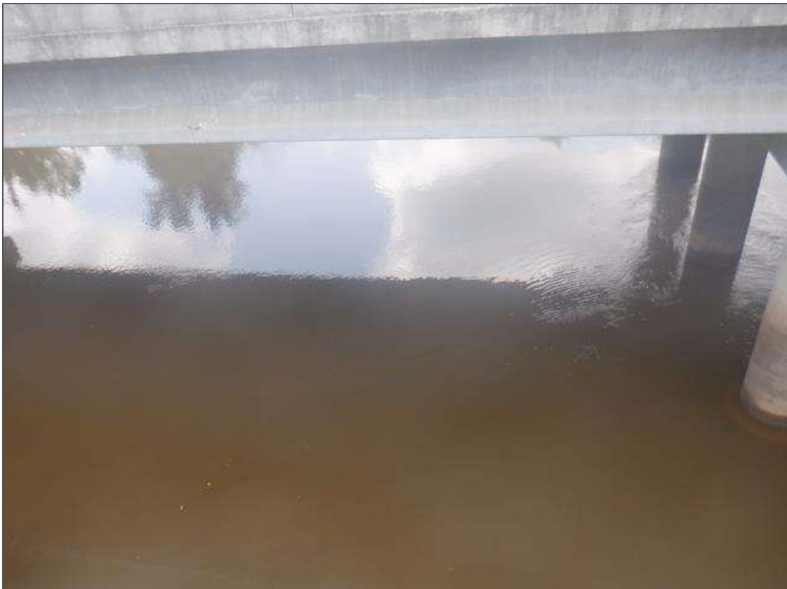
LOOKING WEST/UPSTREAM FROM TOP OF BRIDGE. NOTE SOUTH BOUND LANE BRIDGE.
