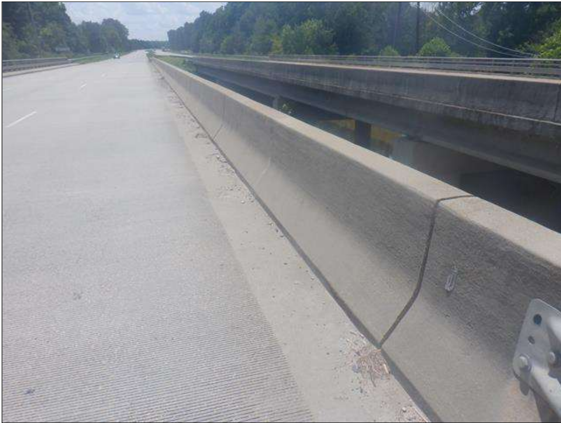
WEST BRIDGE RAIL
