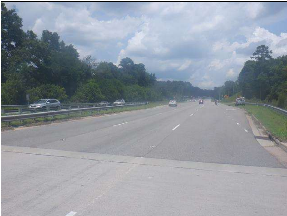
APPROACH 2 LOOKING NORTH
