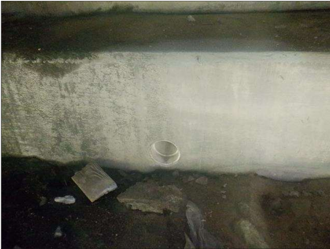
TYPICAL DRAINAGE PIPES IN FRONT FACE OF CAP
