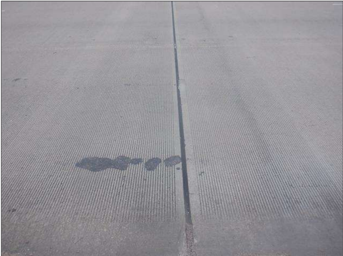
EXPANSION JOINT OVER BENT 2
