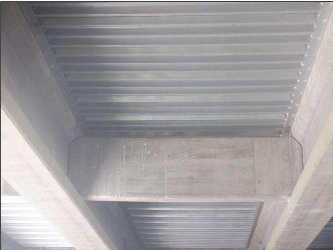
INTERMEDIATE DIAPHRAGM IN SPAN 4, BAY 2. SIMILAR IN SPAN 3.
