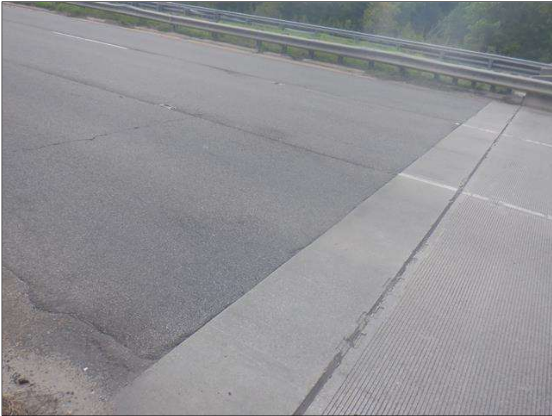
APPROACH SLAB AT END BENT 1
