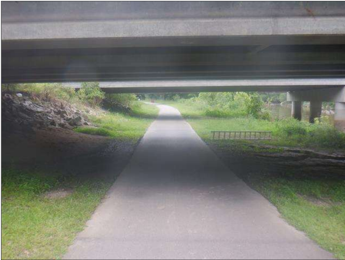
EAST UNDERCLEARANCE PROFILE LOOKING WEST IN SPAN 1
