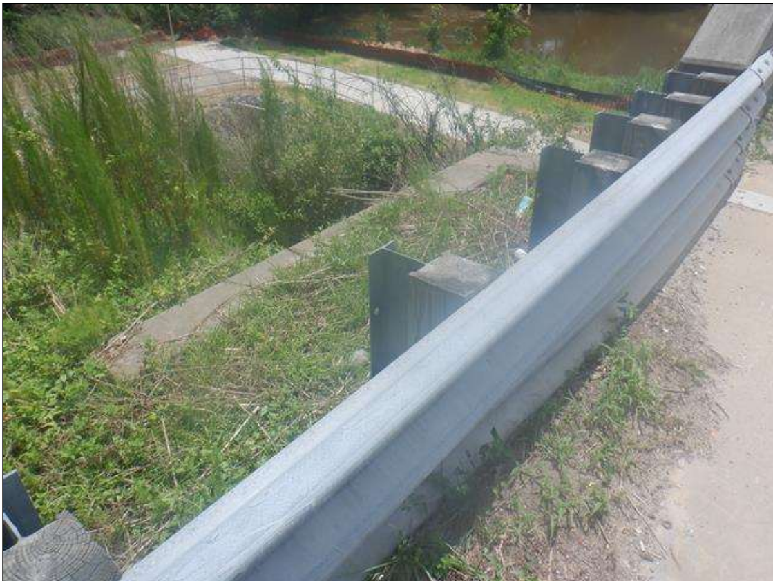
TYPICAL POST SPACING AT BRIDGE AT NORTHEAST CORNER.
