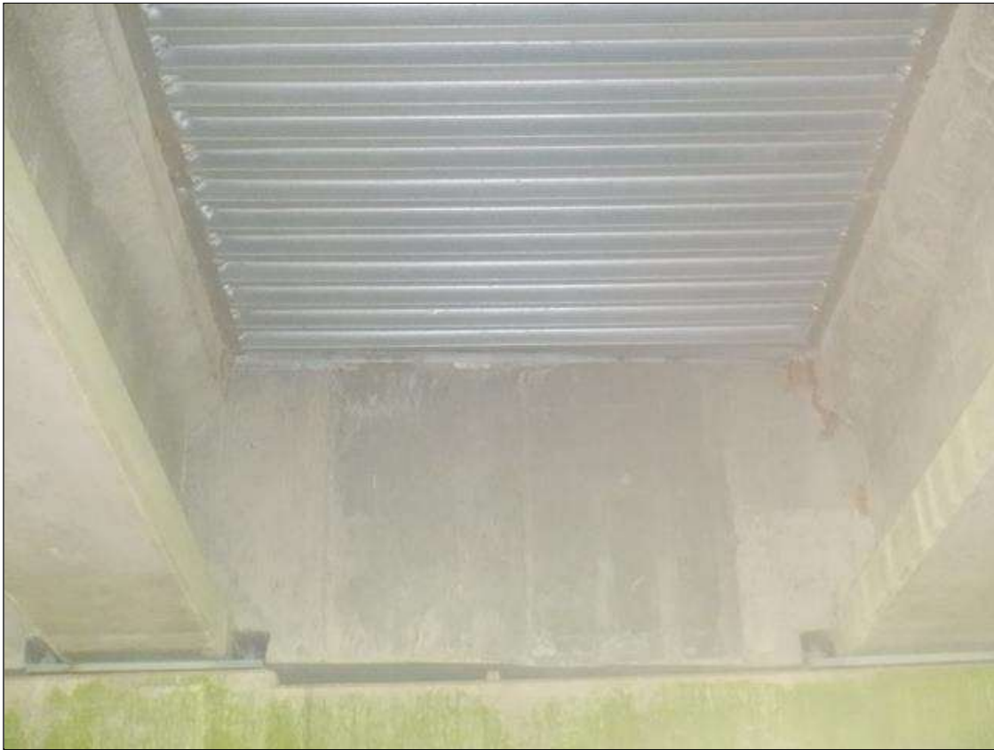
TYPICAL BENT DIAPHRAGM AT BENT 1, BAY 3
