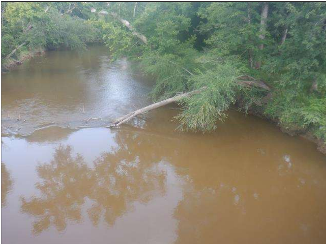
DRIFT UP TO 60 FT LONG X 10 FT HIGH X 6 FT WIDE AT THE DOWNSTREAM END OF BRIDGE, STARTING APPROX. 50 FT FROM THE BRIDGE
