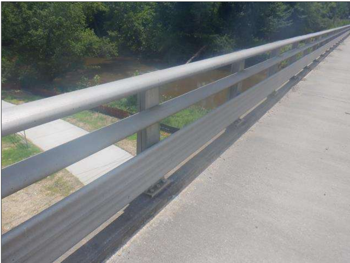
EAST BRIDGE RAIL AND SIDEWALK
