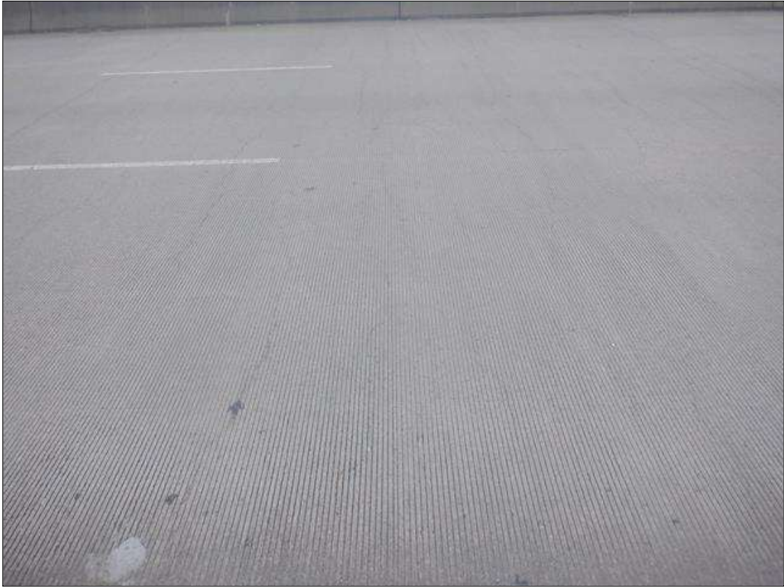
DECK OVER BENT 1
