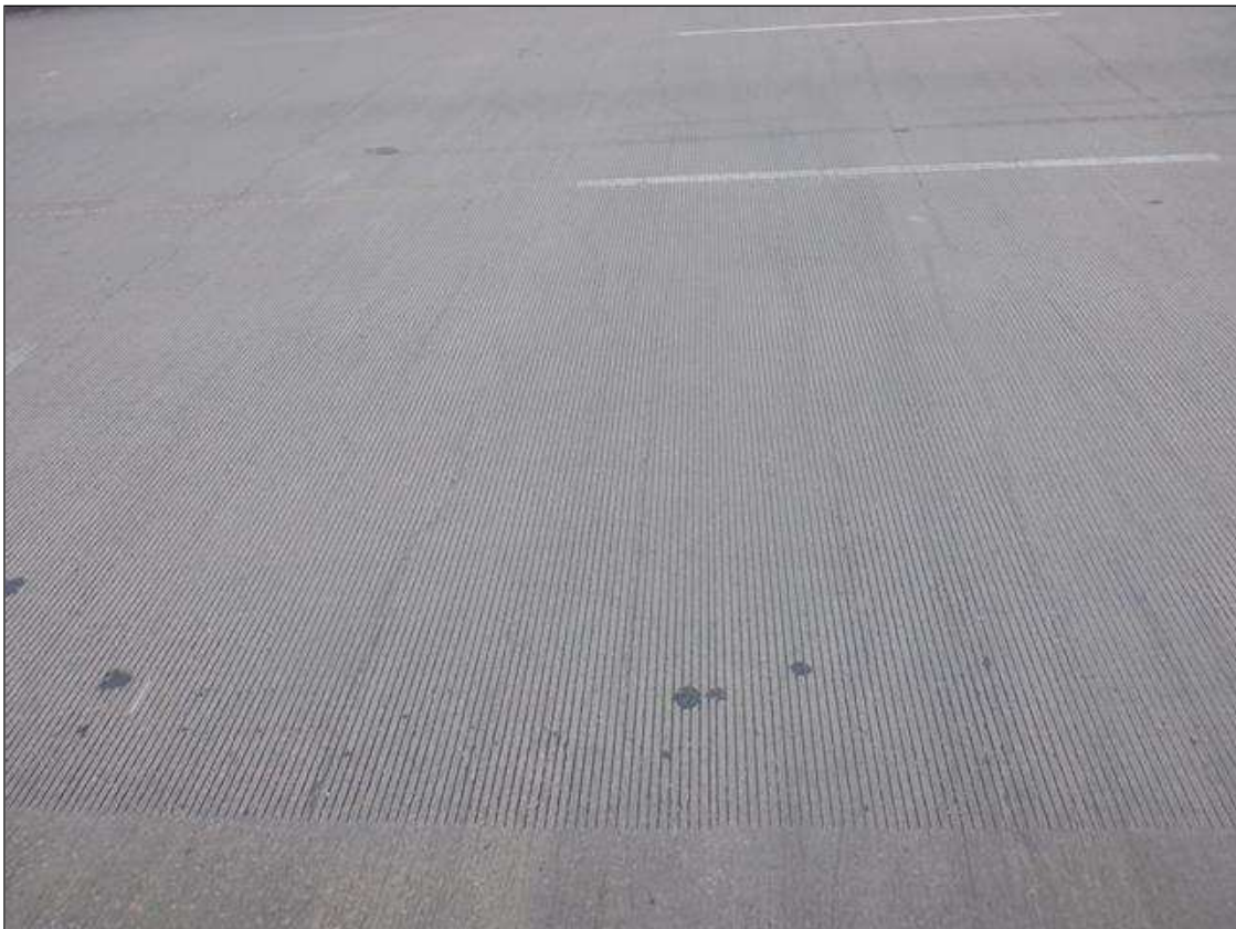
TOP OF DECK OVER BENT 3
