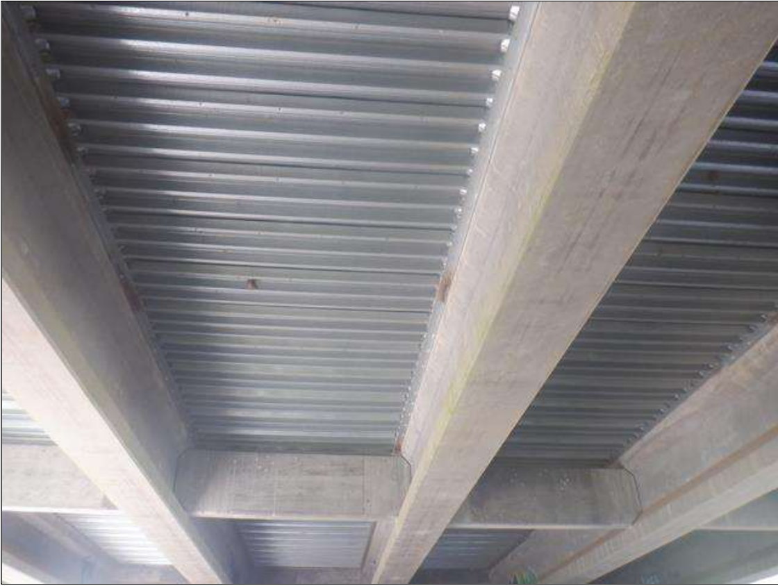
SUPERSTRUCTURE UNDERSIDE IN SPAN 4. SIMILAR IN SPAN 3
