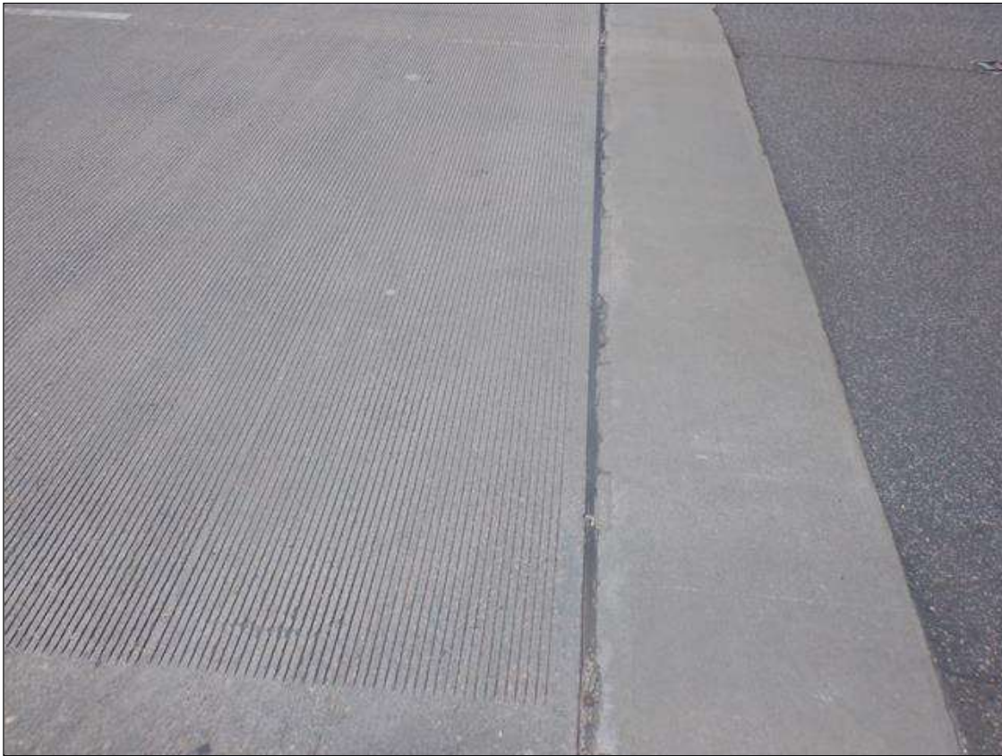
EXPANSION JOINT AT END BENT 2
