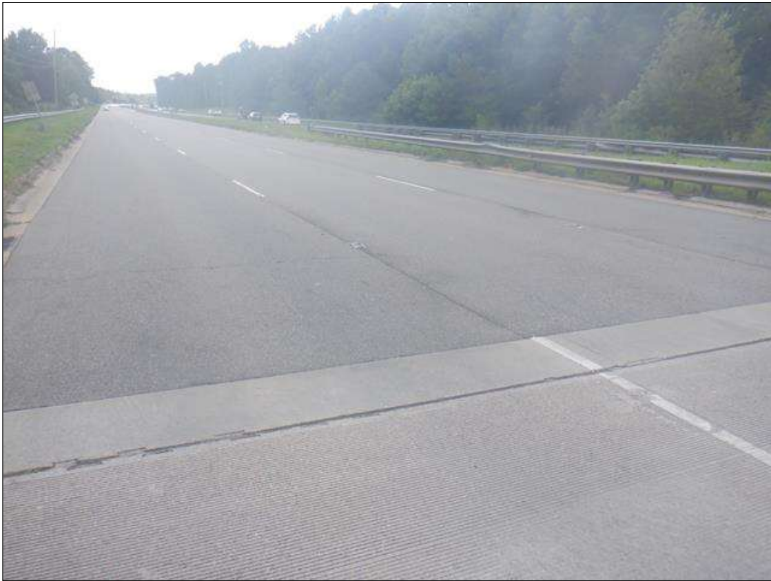
APPROACH 1 LOOKING SOUTH
