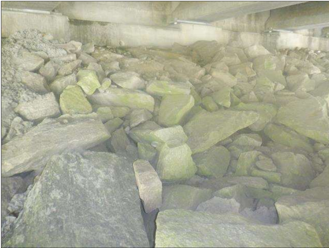
SLOPE PROTECTION AT END BENT 1
