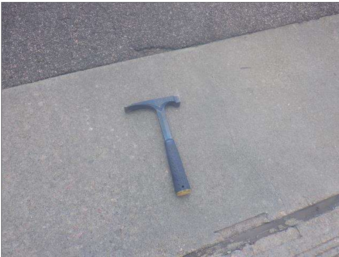
Approach 1 : 16 SQUARE FEET UP TO 1/32" LONGITUDINAL CRACKS, AT RANDOM THROUGHOUT ALL TRAVEL LANES.
