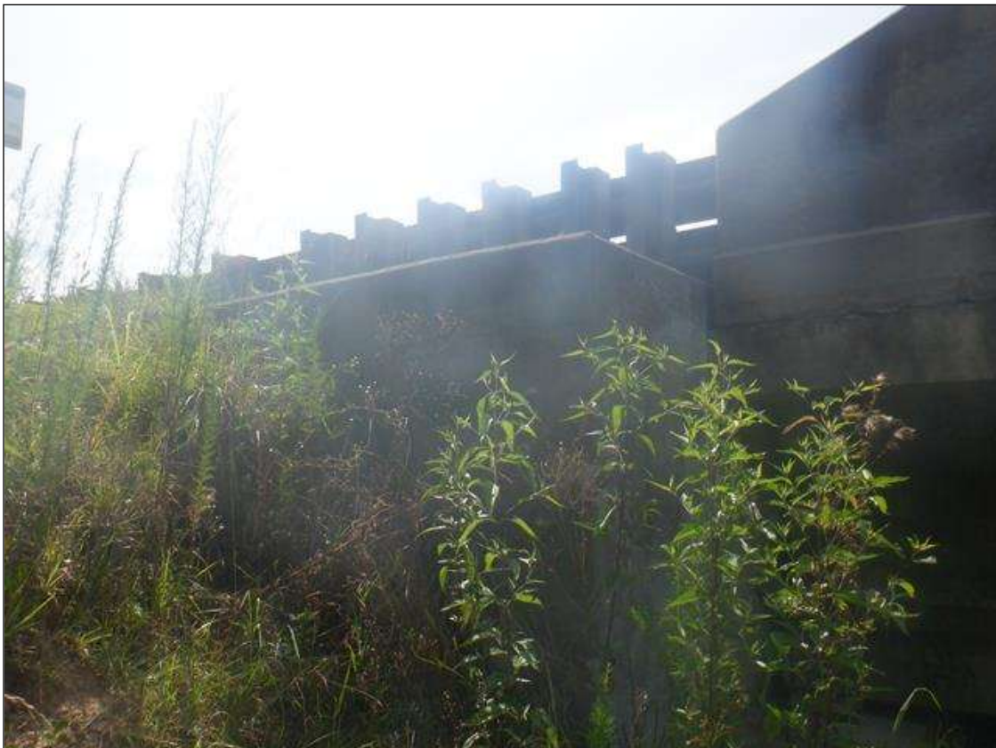
TYPICAL ABUTMENT EXTENSION WALL AT SOUTHWEST CORNER
