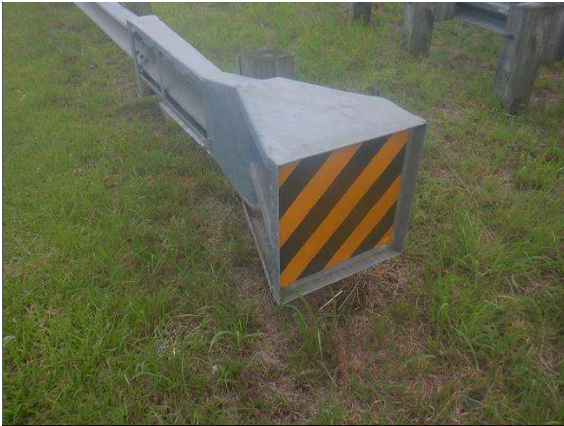
NORTHWEST GUARDRAIL END TERMINAL
