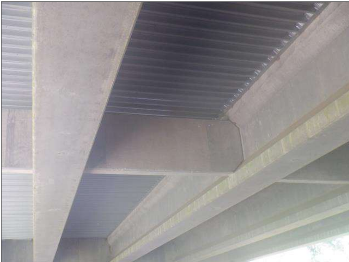
SUPERSTRUCTURE UNDERSIDE IN SPAN 1
