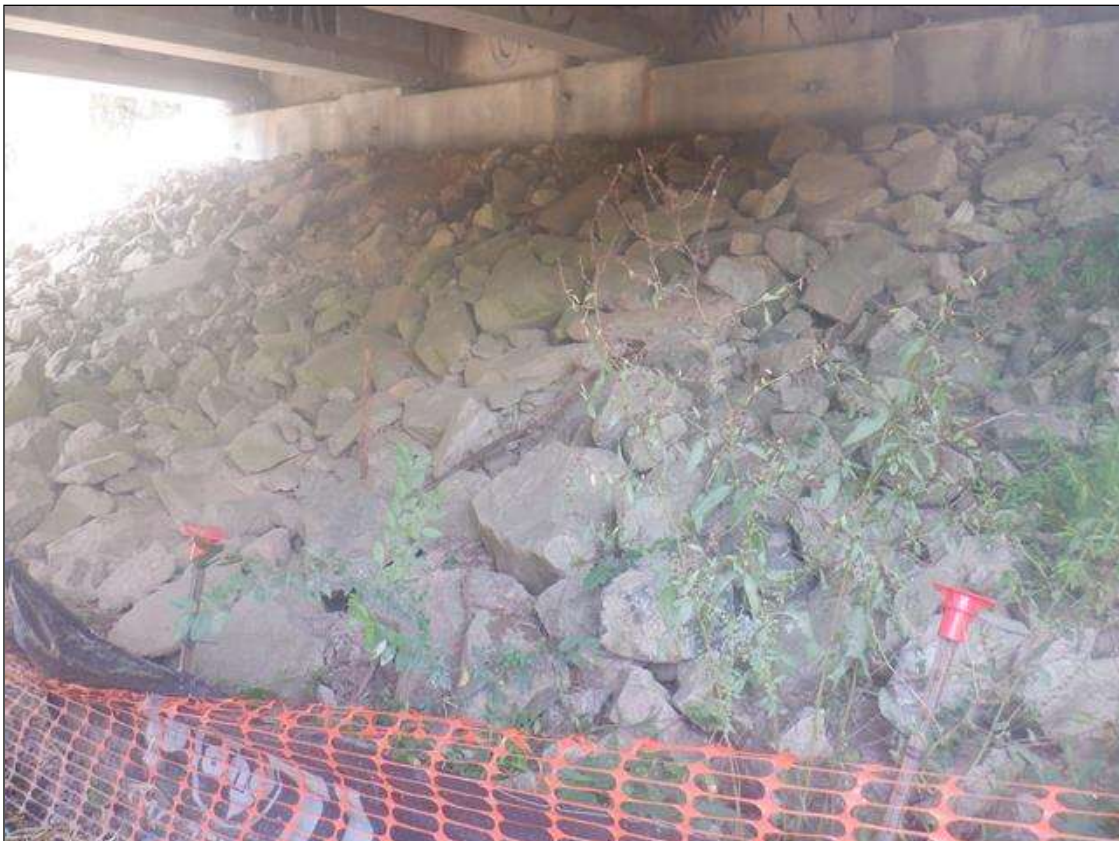
SLOPE PROTECTION AT END BENT 2
