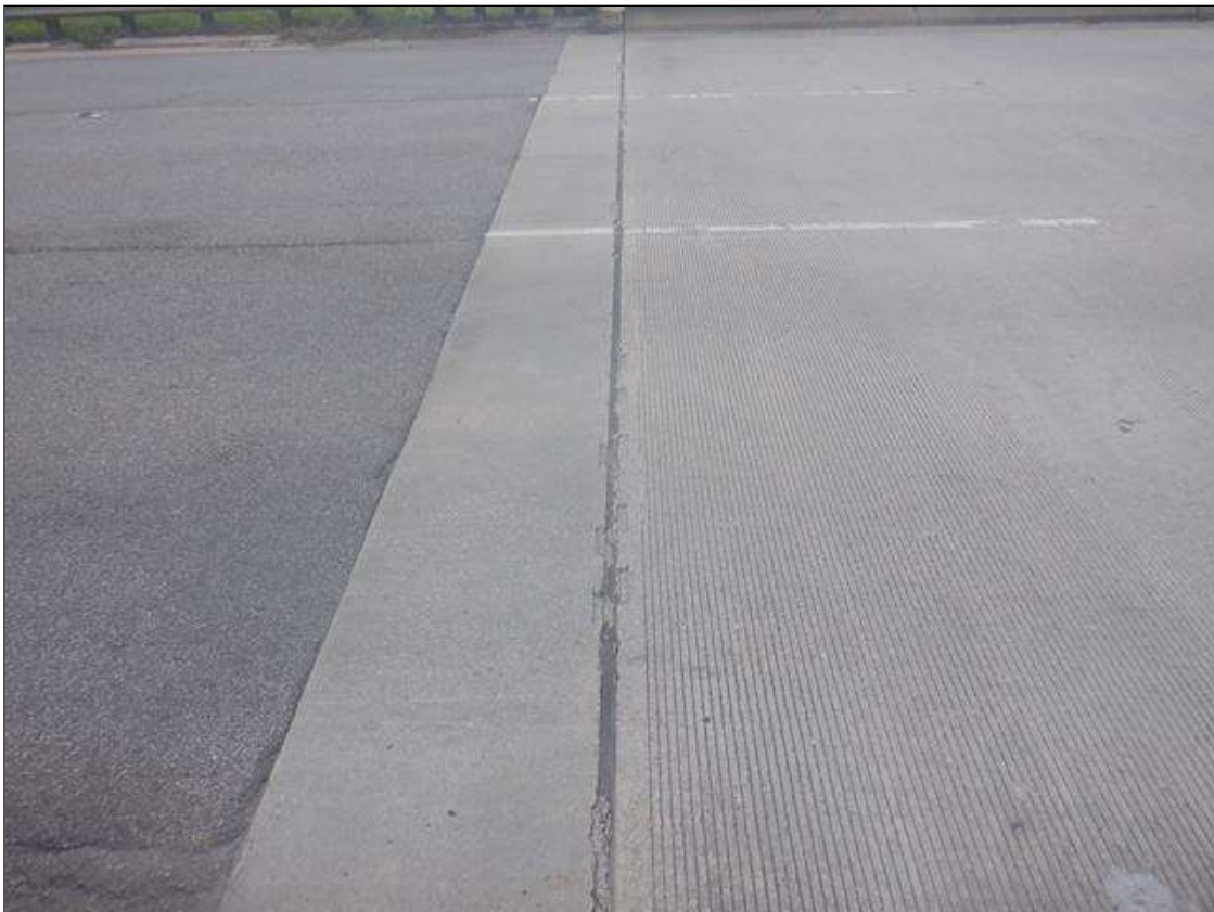
EXPANSION JOINT AT END BENT 1
