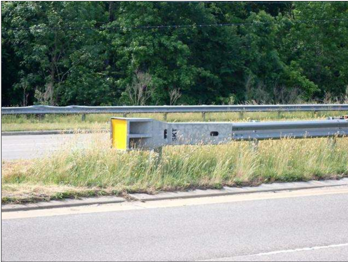
NORTHEAST GUARDRAIL TERMINATION
