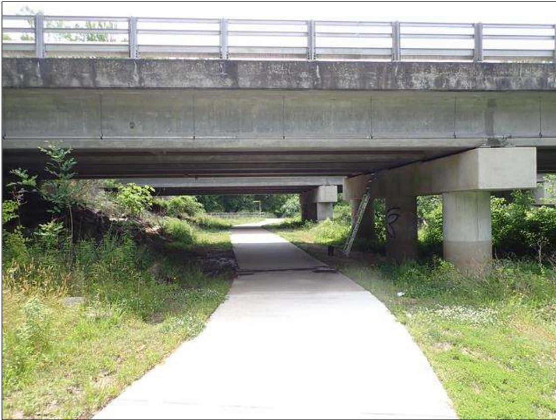
SPAN 4 UNDERCLEARANCE LOOKING EAST (GREENWAY)
