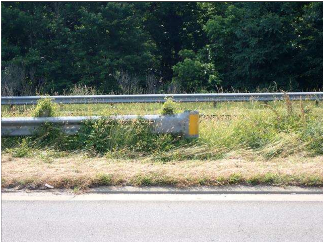
SOUTHEAST GUARDRAIL TERMINATION
