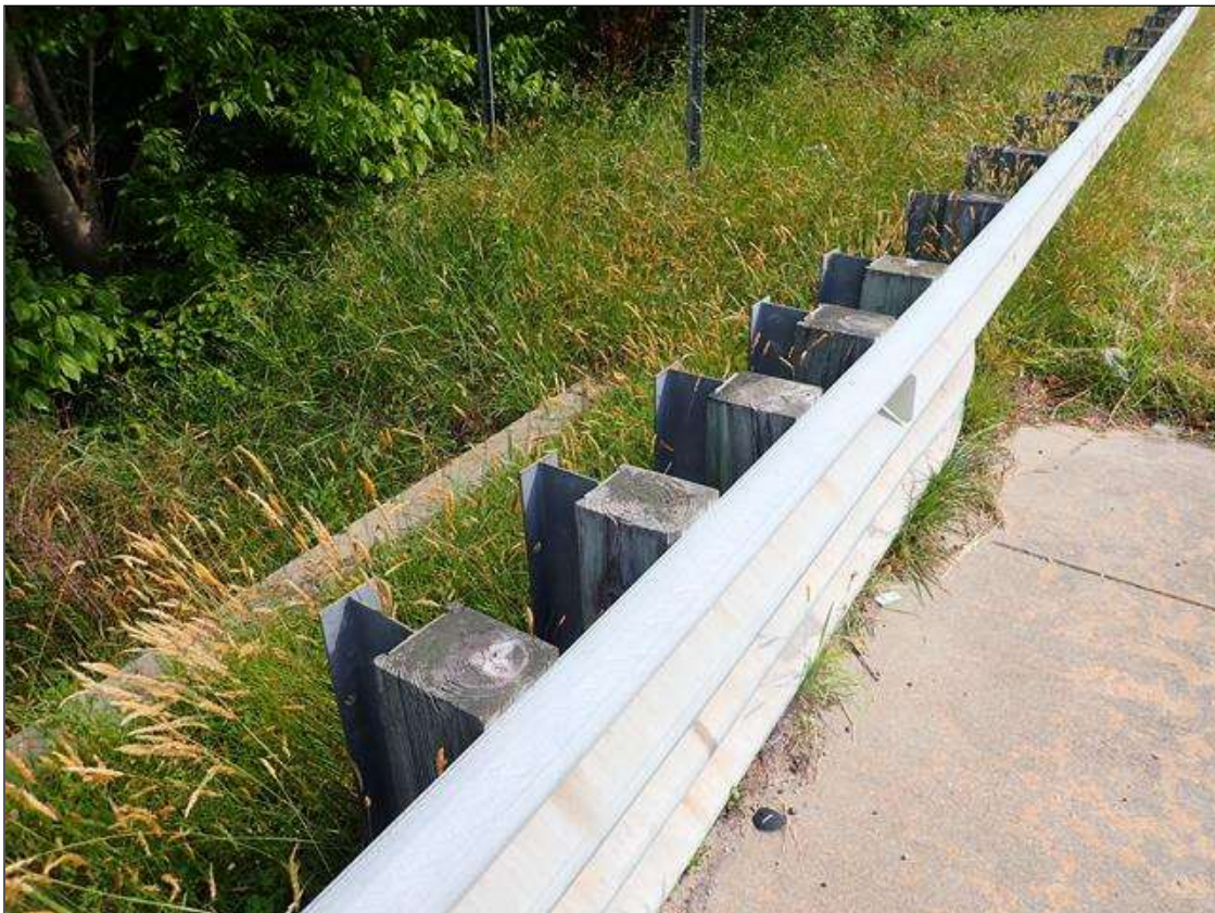
NORTHWEST GUARDRAIL TRANSITION, NORTHEAST SIMILAR
