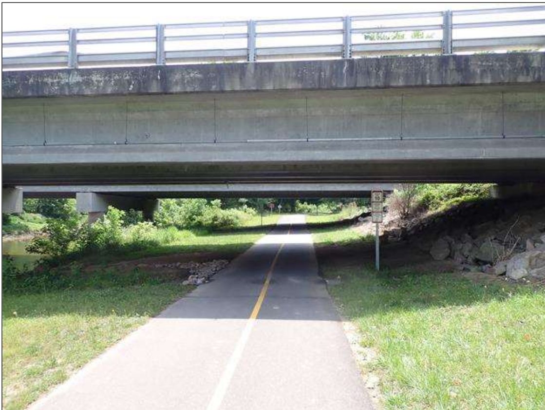
SPAN 1 UNDERCLEARANCE LOOKING EAST (GREENWAY)
