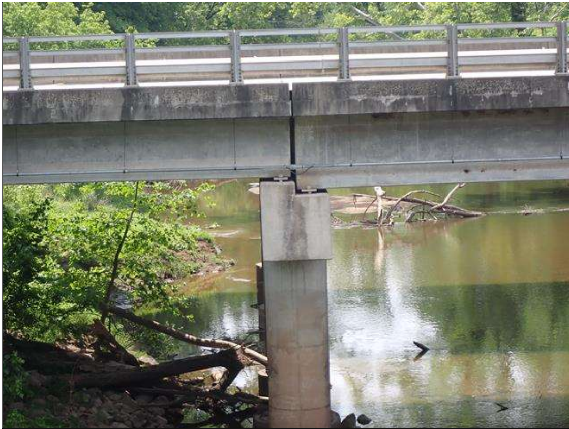
END OF BENT 2 CAP
