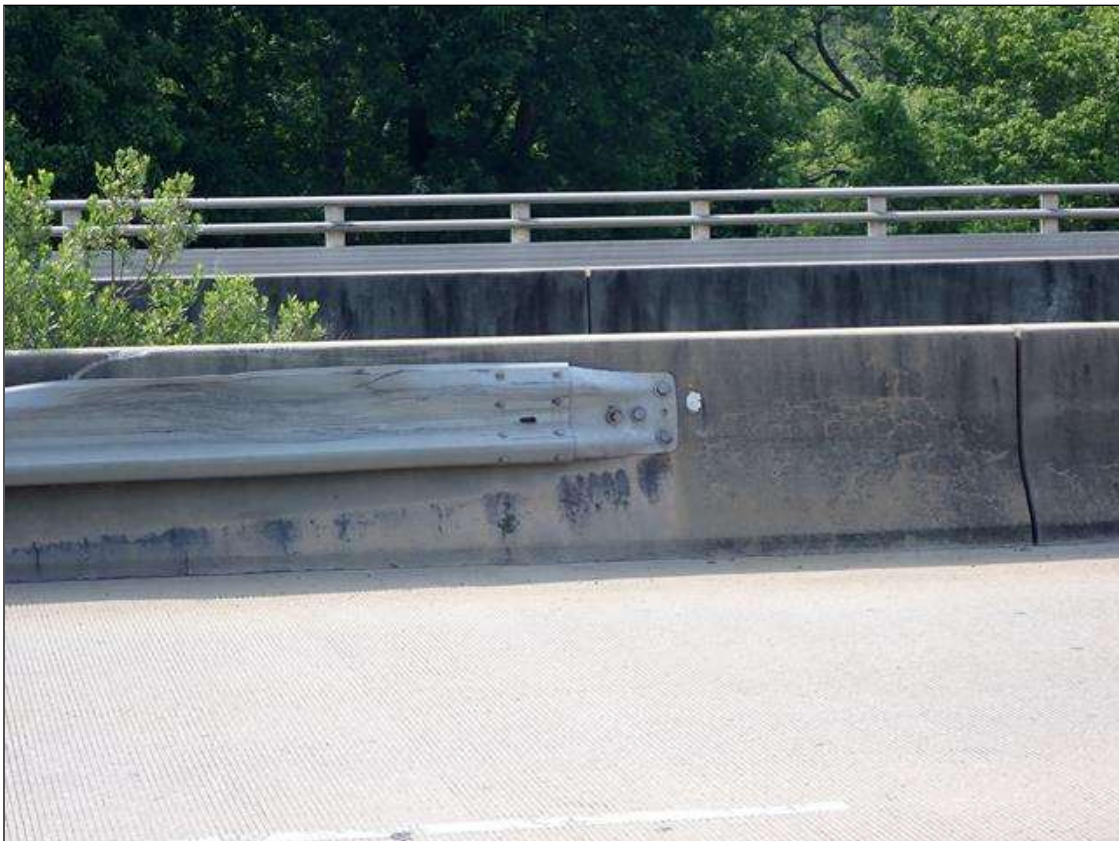
NORTHEAST GUARDRAIL ATTACHMENT
