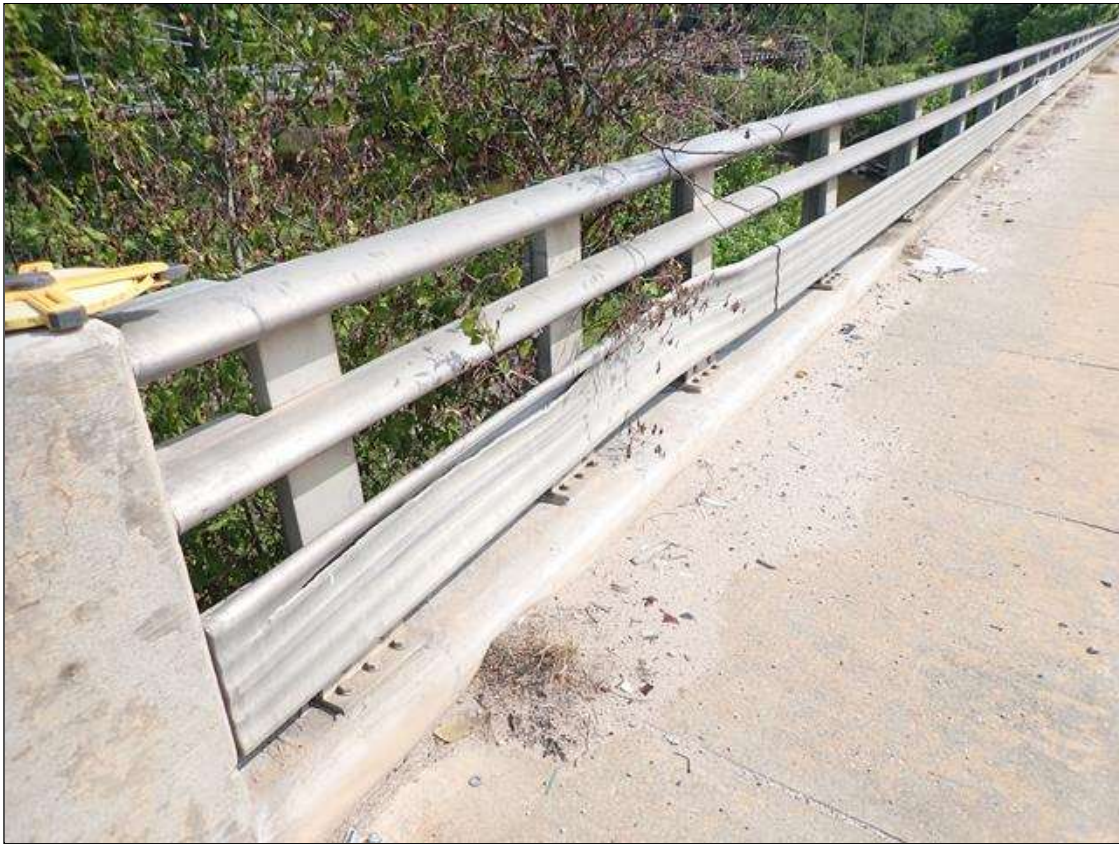
LEFT BARRIER RAIL
