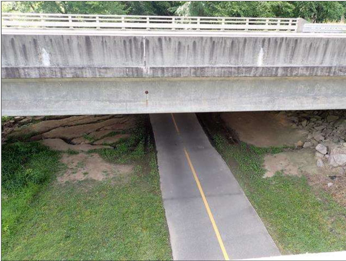
LOOKING EAST OVER SPAN 1 GREENWAY
