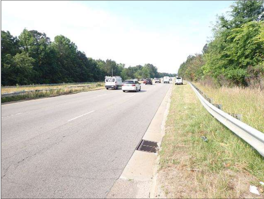
SOUTH APPROACH LOOKING SOUTH
