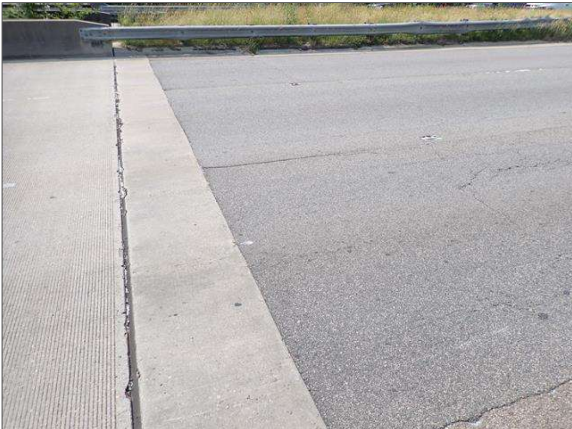
SOUTH APPROACH SLAB, NORTH SIMILAR
