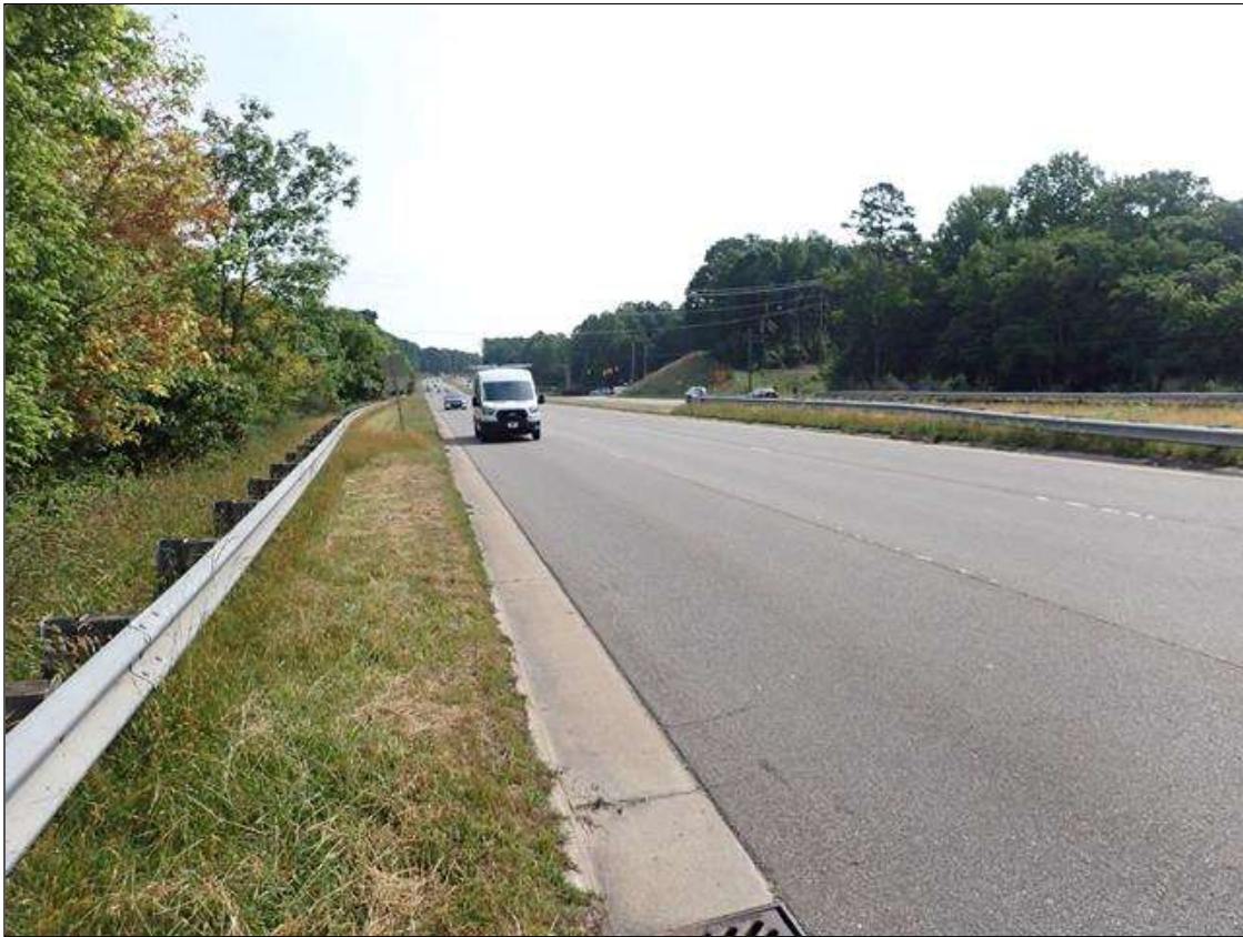
NORTH APPROACH LOOKING NORTH
