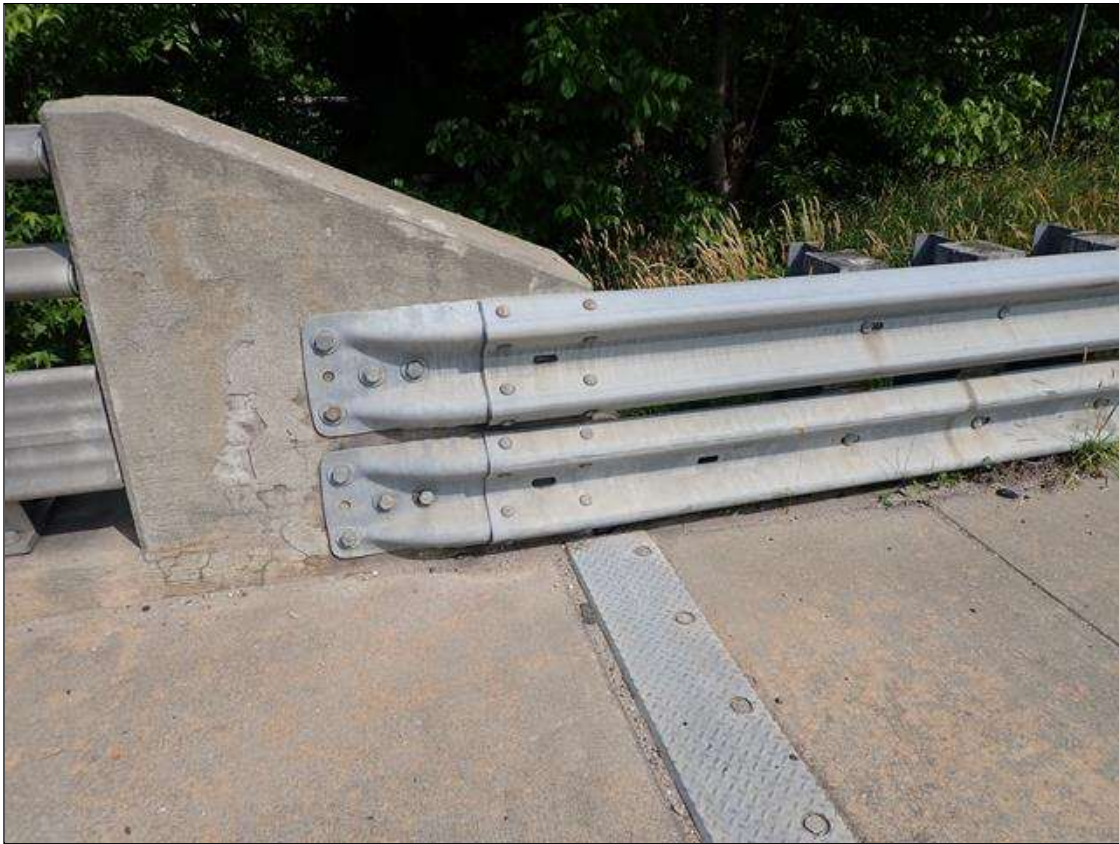
NORTHWEST GUARDRAIL ATTACHMENT
