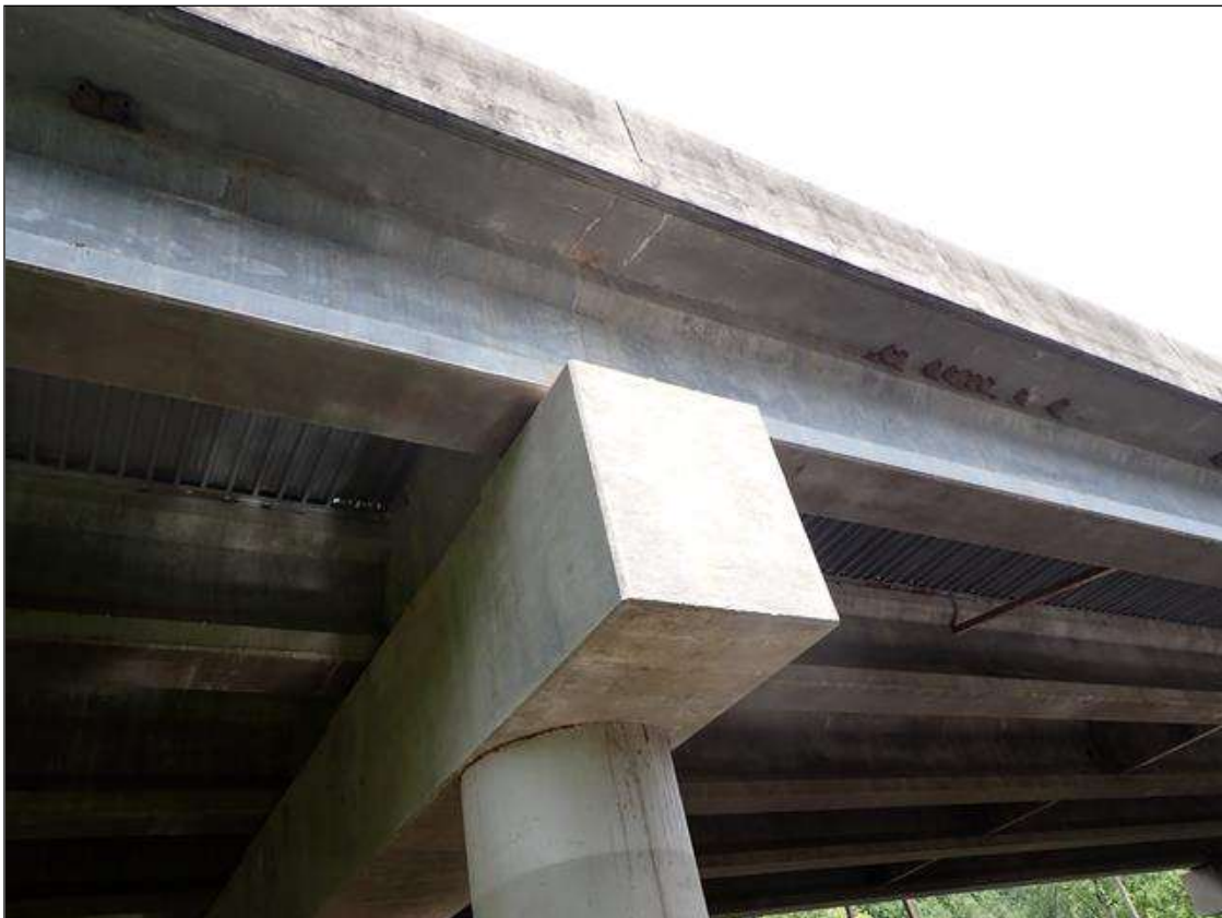
END OF BENT 1 CAP
