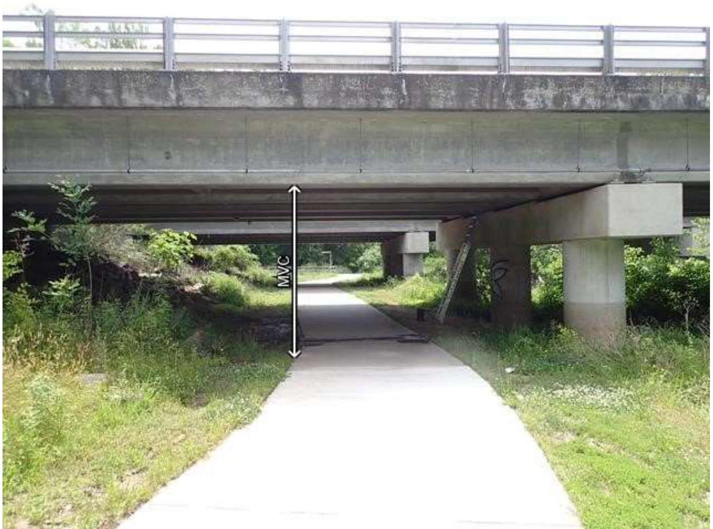
SPAN 4 UNDERCLEARANCE LOOKING EAST (GREENWAY)
