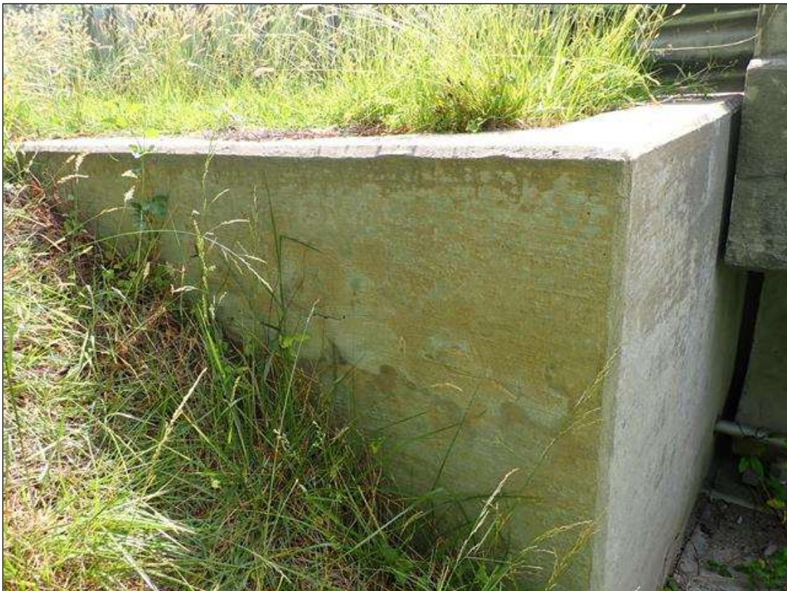
NORTHWEST WINGWALL, TYPICAL
