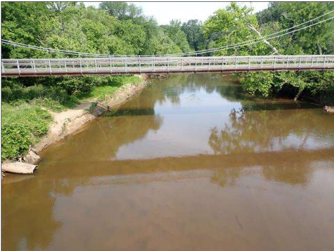
LOOKING UPSTREAM (WEST) OVER WATERWAY FROM SPAN 2
