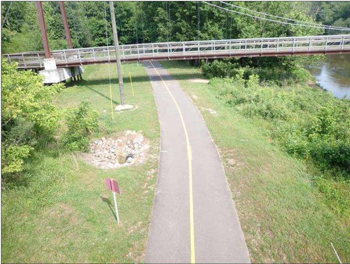
LOOKING WEST OVER SPAN 1 GREENWAY
