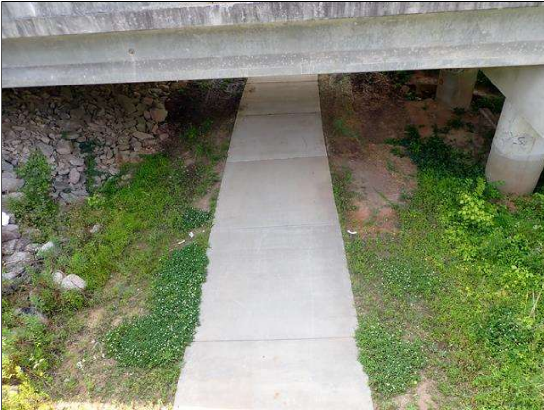
LOOKING EAST OVER SPAN 4 GREENWAY
