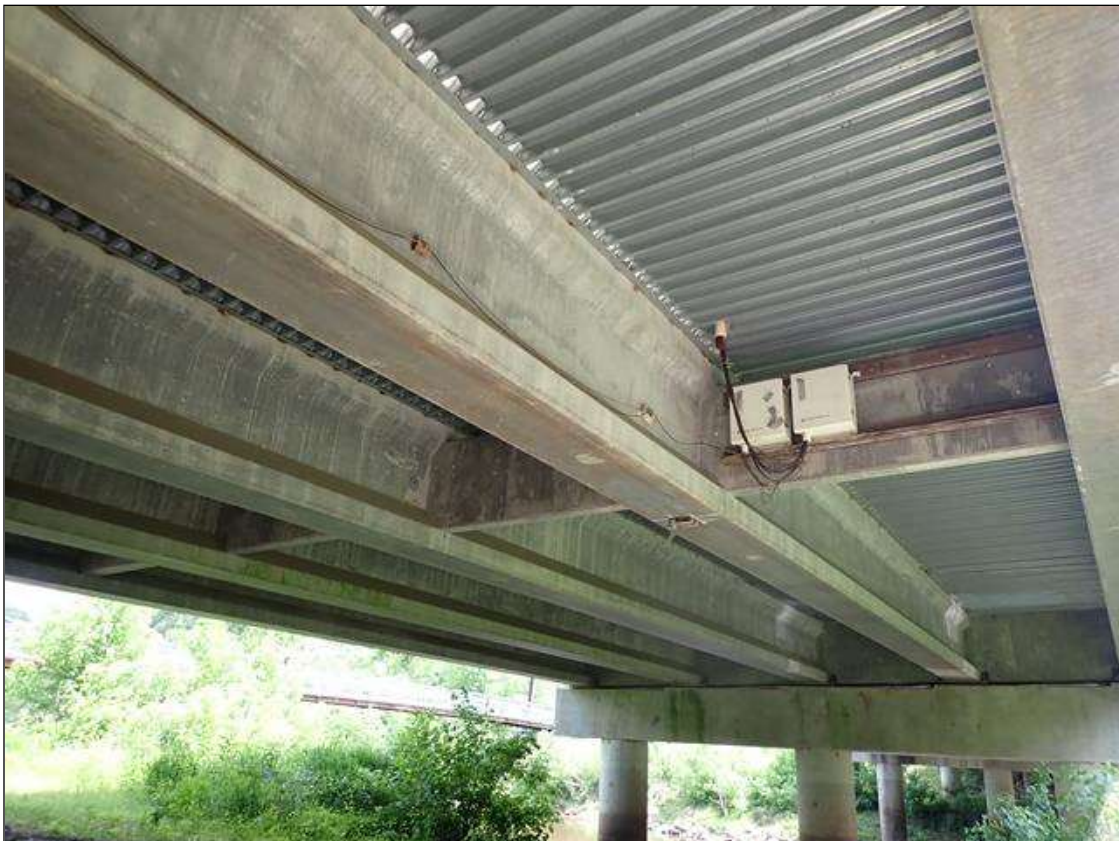
SUPERSTRUCTURE UNDERSIDE, TYPICAL
