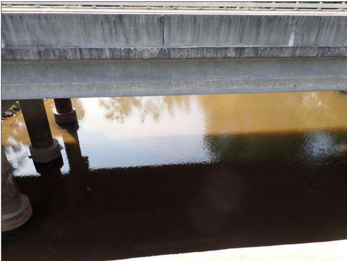
LOOKING DOWNSTREAM (EAST) OVER WATERWAY FROM SPAN 2
