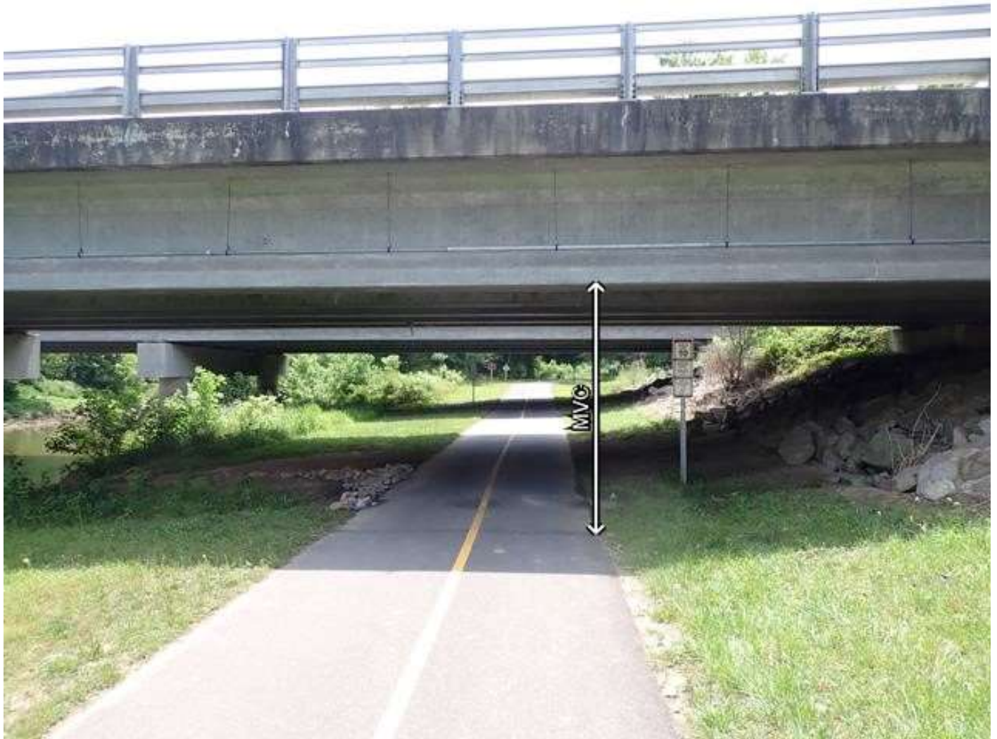
SPAN 1 UNDERCLEARANCE LOOKING EAST (GREENWAY)
