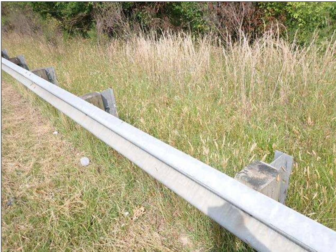
GUARDRAIL POST SPACING, TYPICAL
