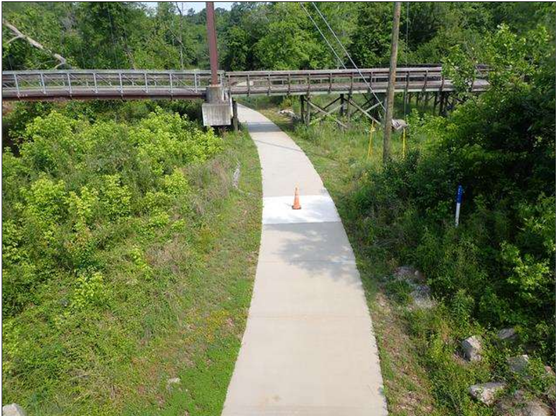
LOOKING WEST OVER SPAN 4 GREENWAY
