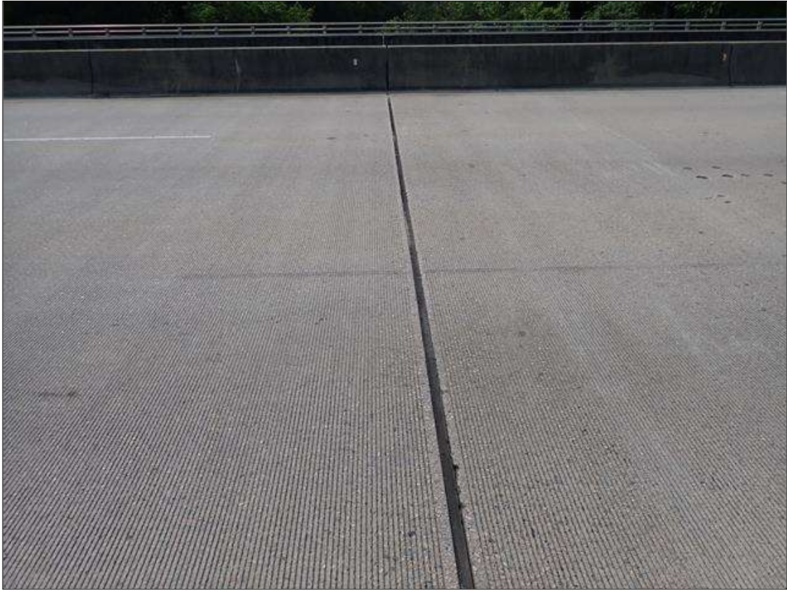
JOINT AT BENT 3
