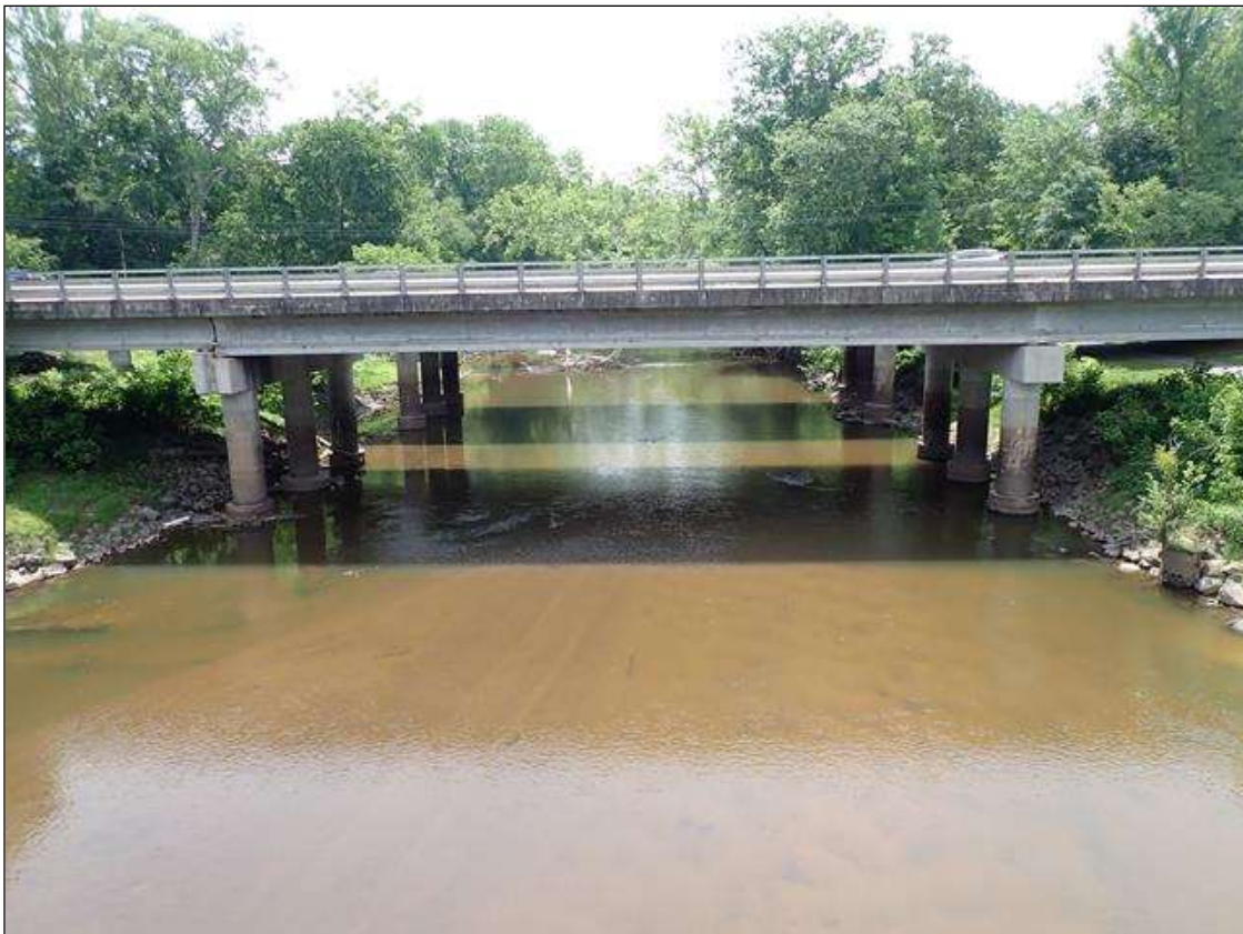
UPSTREAM WATERWAY OPENING LOOKING DOWNSTREAM
