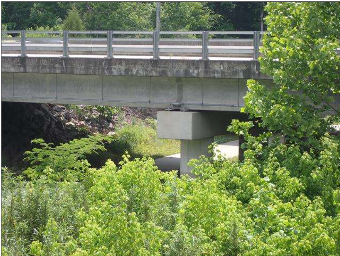
END OF BENT 3 CAP
