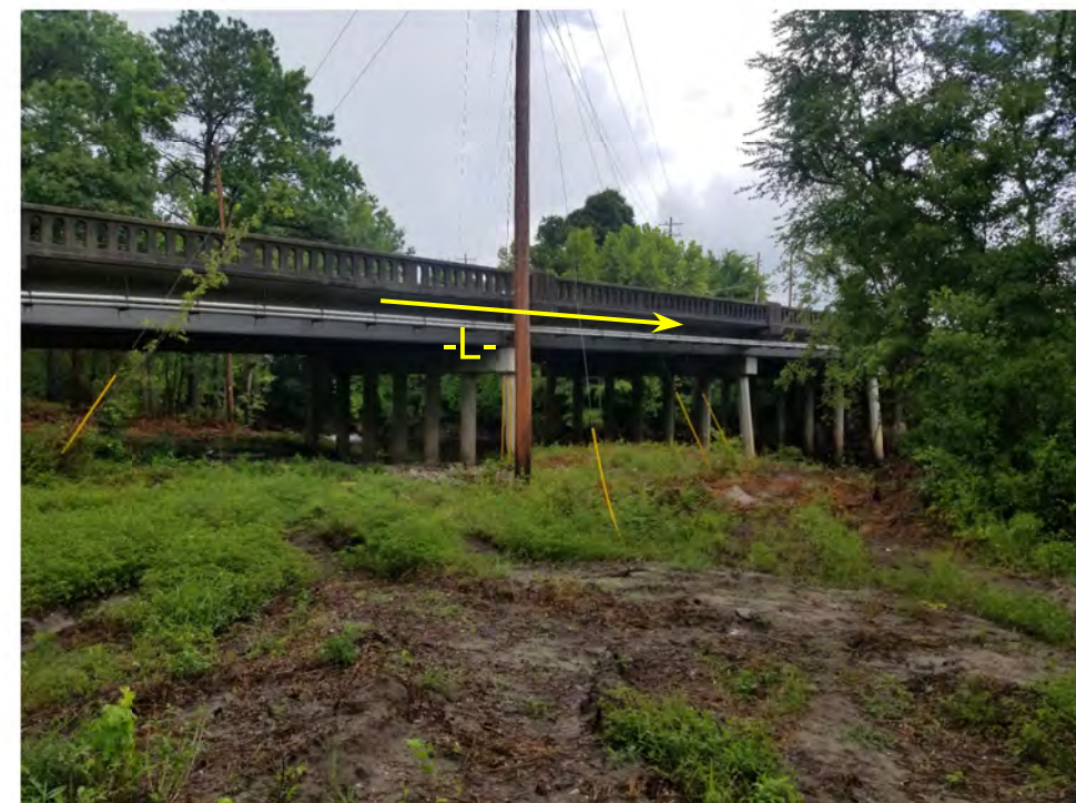
DOWNSTREAM (RIGHT) OF -L- FACING NORTH
