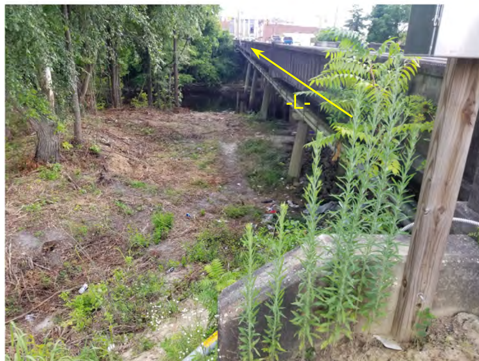
NEAR END BENT 1 LEFT OF -L- FACING EAST TO END BENT 2
