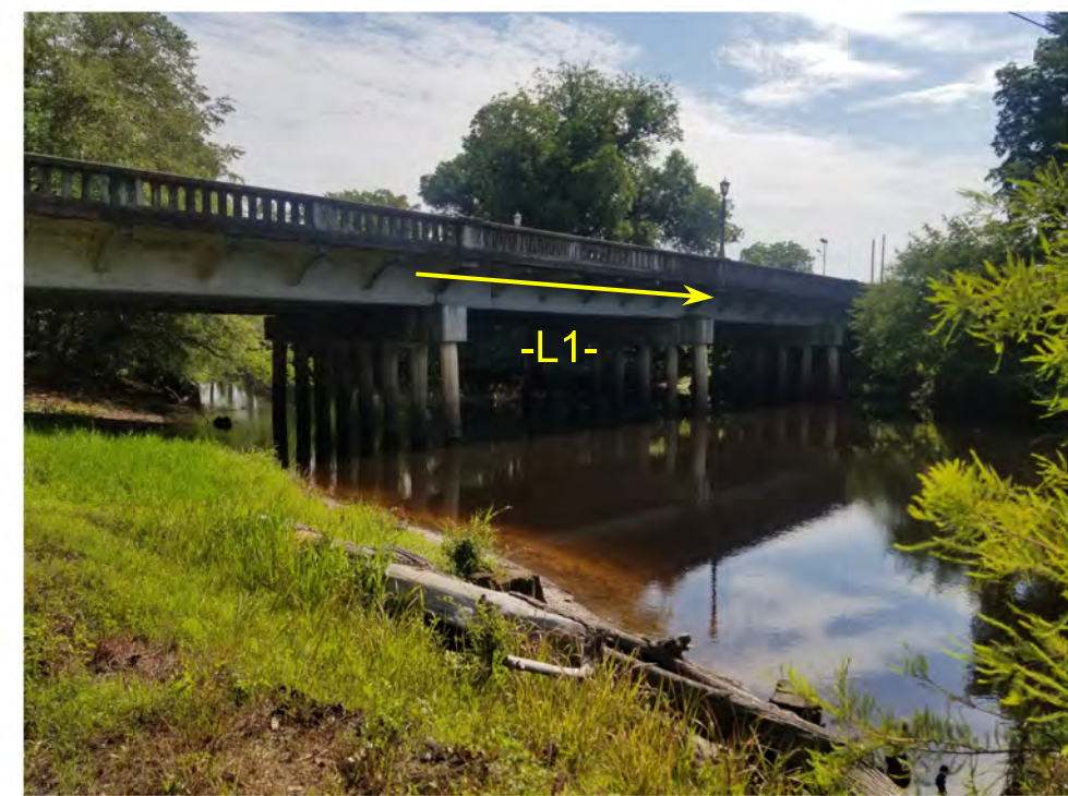
DOWNSTREAM (RIGHT) OF -L1- FACING NORTH
