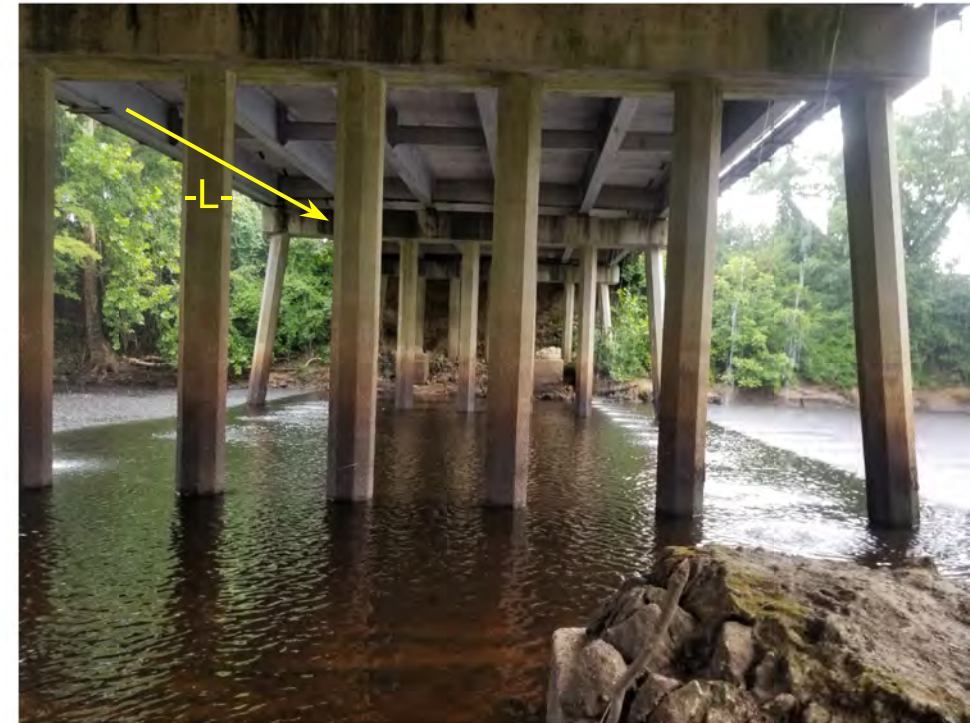
NEAR BENT 1 FACING EAST TO END BENT 2
