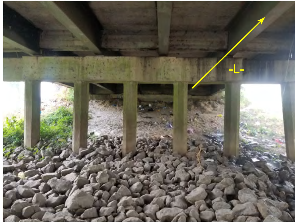
NEAR BENT 1 FACING WEST TO END BENT 1
