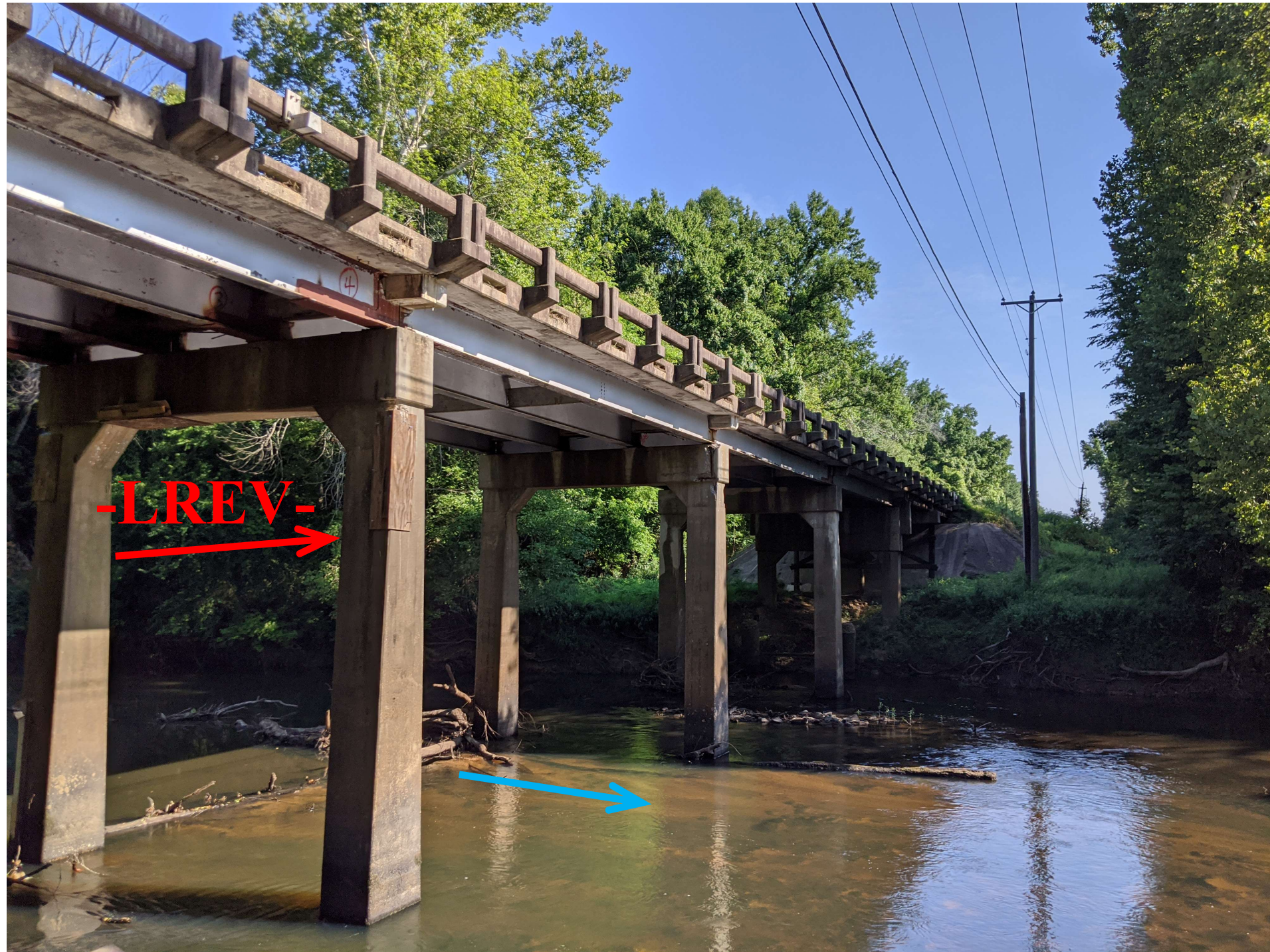
Looking Northwest towards End Bent 2
