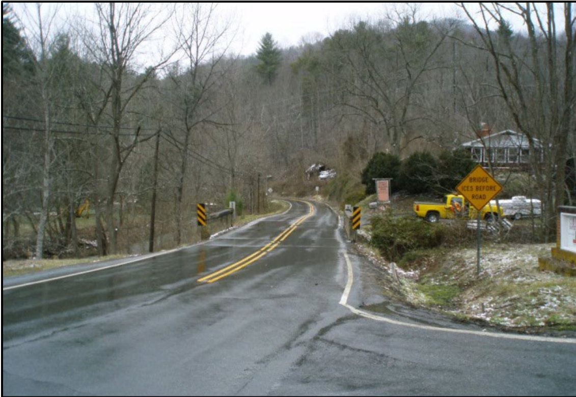
Figure 6: West view of Bridge 19.
