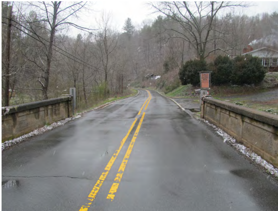
Bridge No. 19 West Approach
