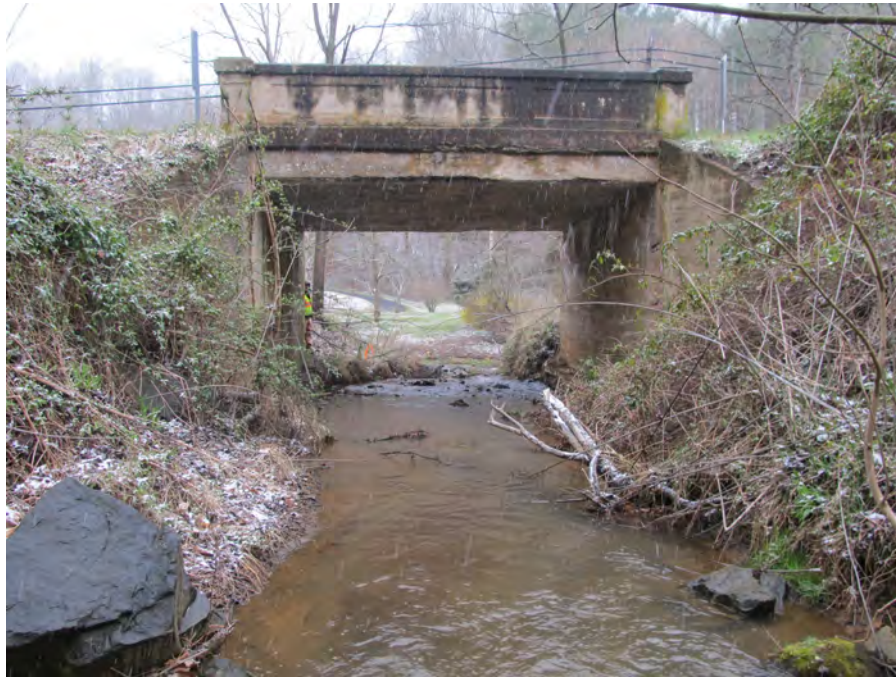
Bridge No. 19 Upstream Bridge Face
