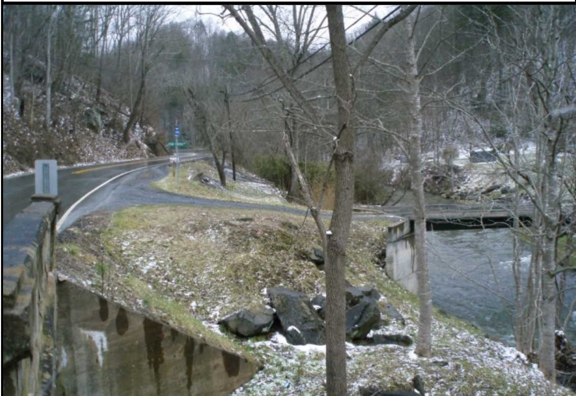
Figure 4: Southeast view of the southeast quadrant.
