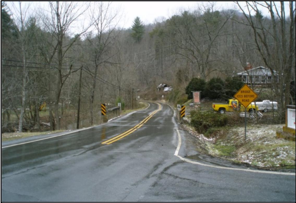
Figure 1: West view of Bridge 19.
