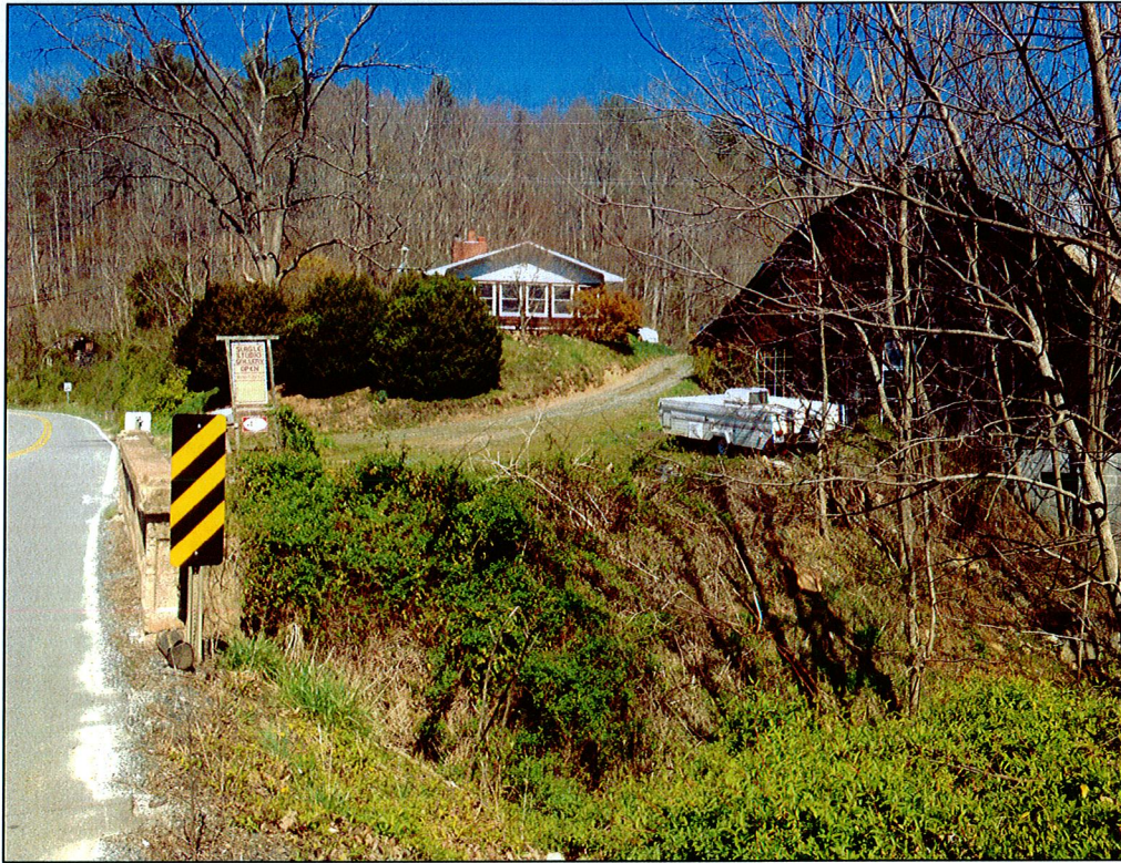
House and barn directly northwest of bridge. Not eligible for NR listing.
