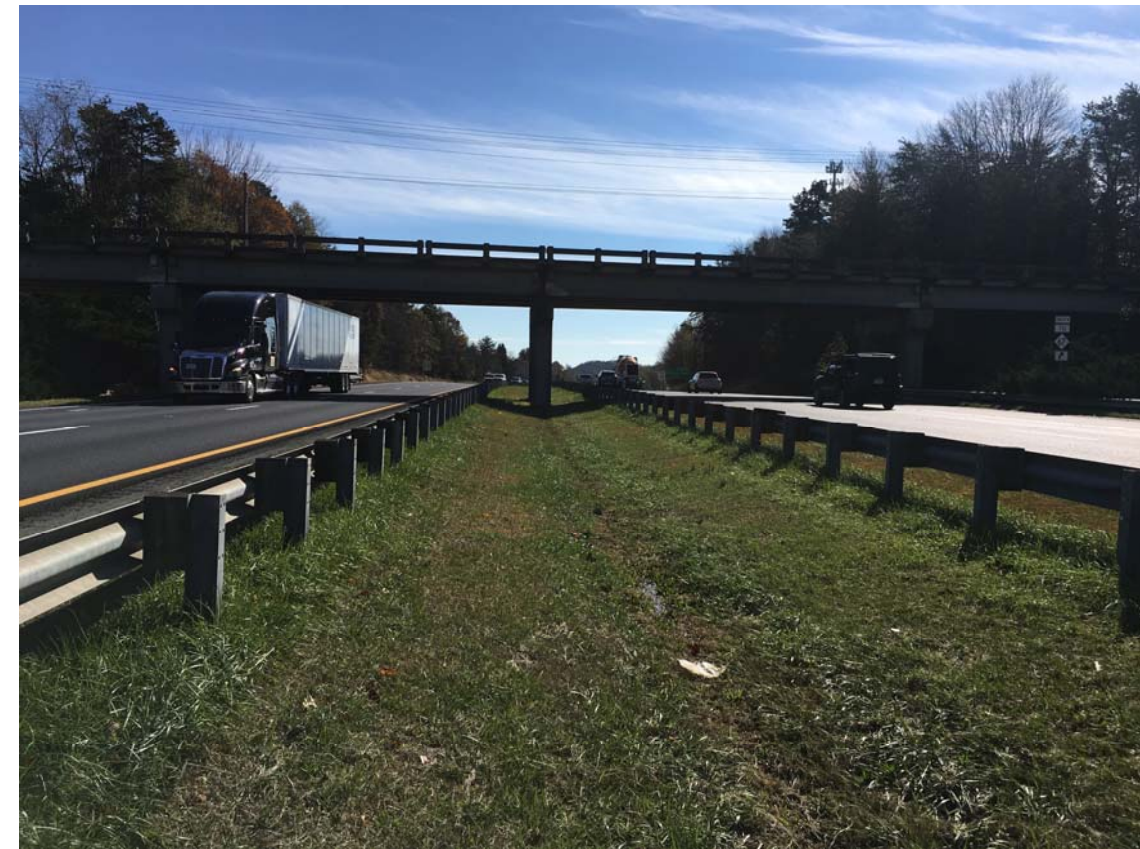
BENT 1, LOOKING FROM RT TO LT.
