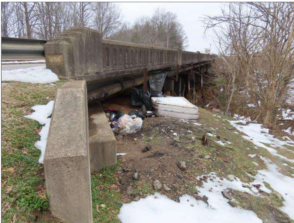
SOUTH ELEVATION, LOOKING AHEAD
