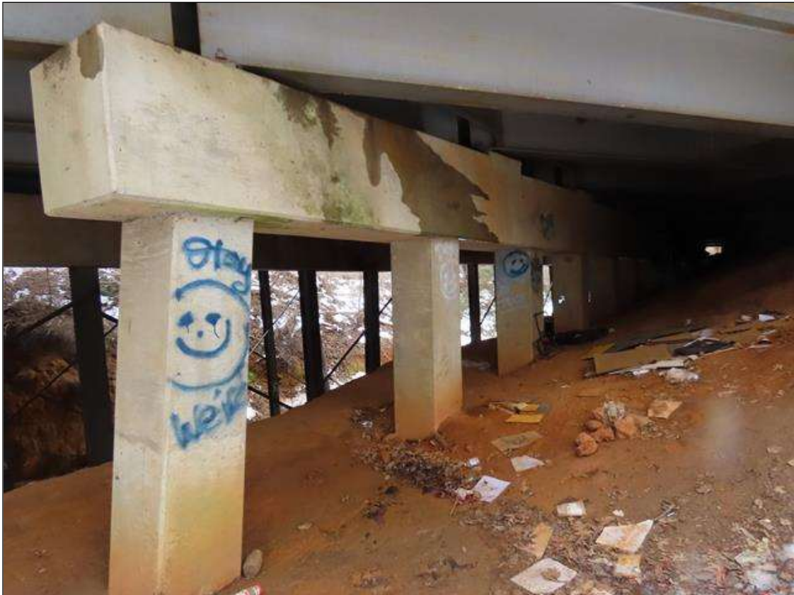
BENT 1, NEAR SIDE
