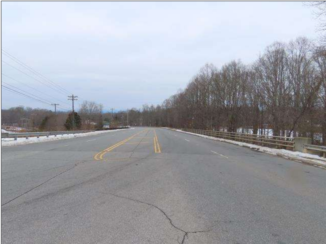
LOOKING STATIONS BACK, WEST
