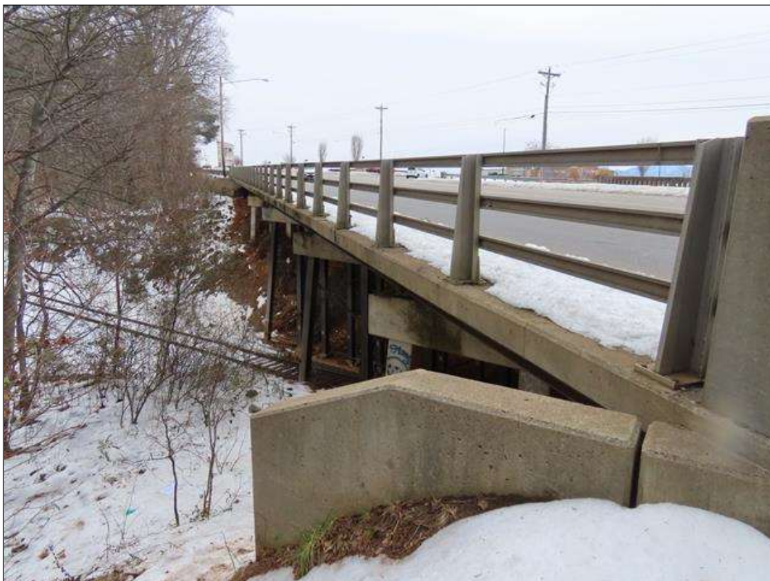
NORTH ELEVATION, LOOKING AHEAD
