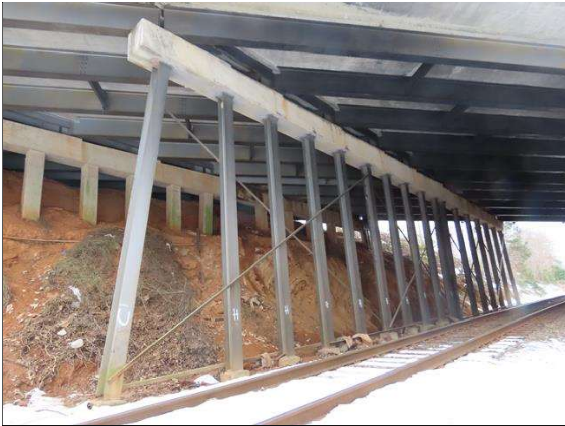
BENT 3, NEAR SIDE
