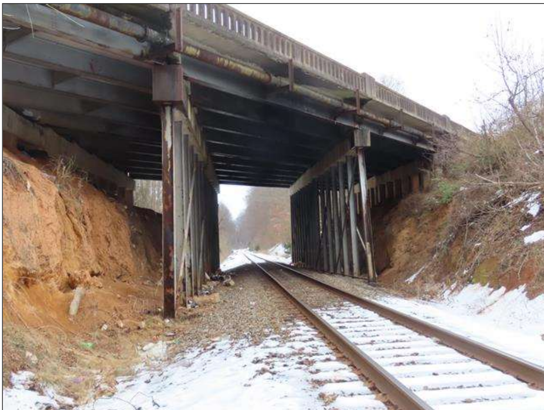
SPAN 3 VERTICAL CLEARANCE, LOOKING NORTH
