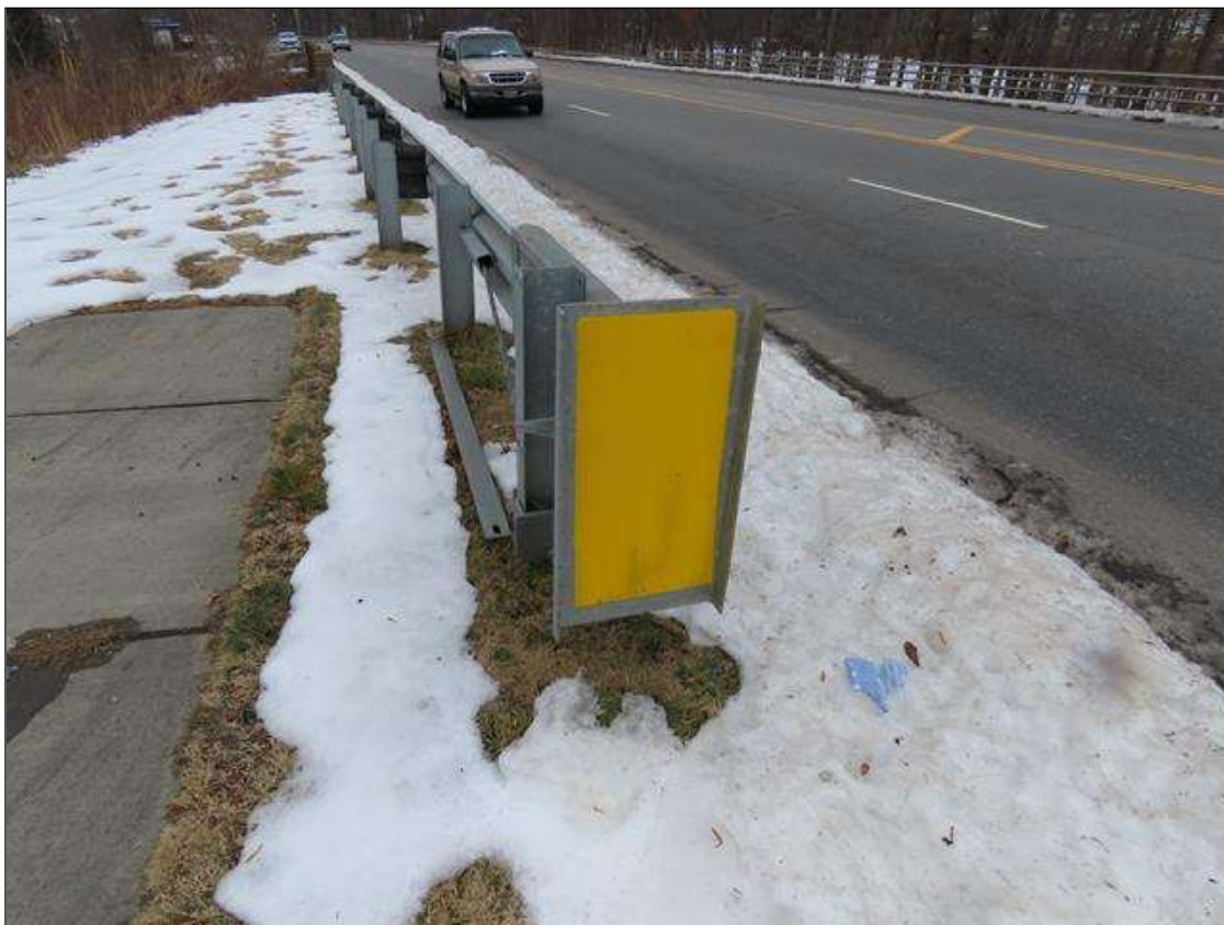
GUARDRAIL END TREATMENT AT FAR RIGHT
