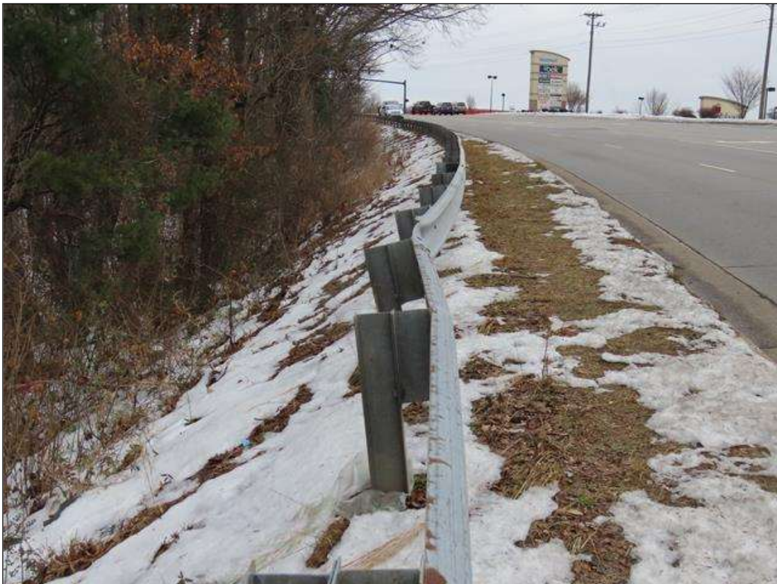
FAR LEFT GUARDRAIL - MODERATE IMPACT DAMAGE (20FT L. X 1FT DISTORTION) STARTING 60FT FROM BRIDGE
