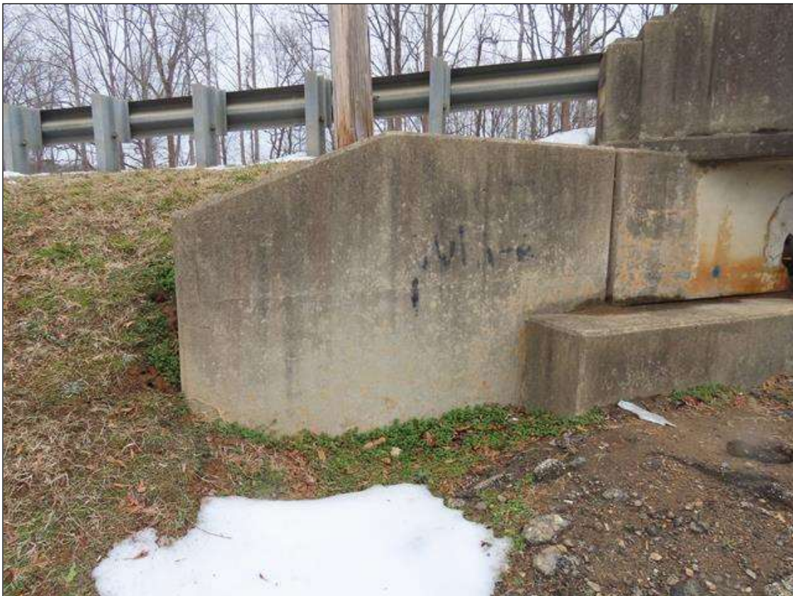
TYP. WINGWALL, NEAR RIGHT
