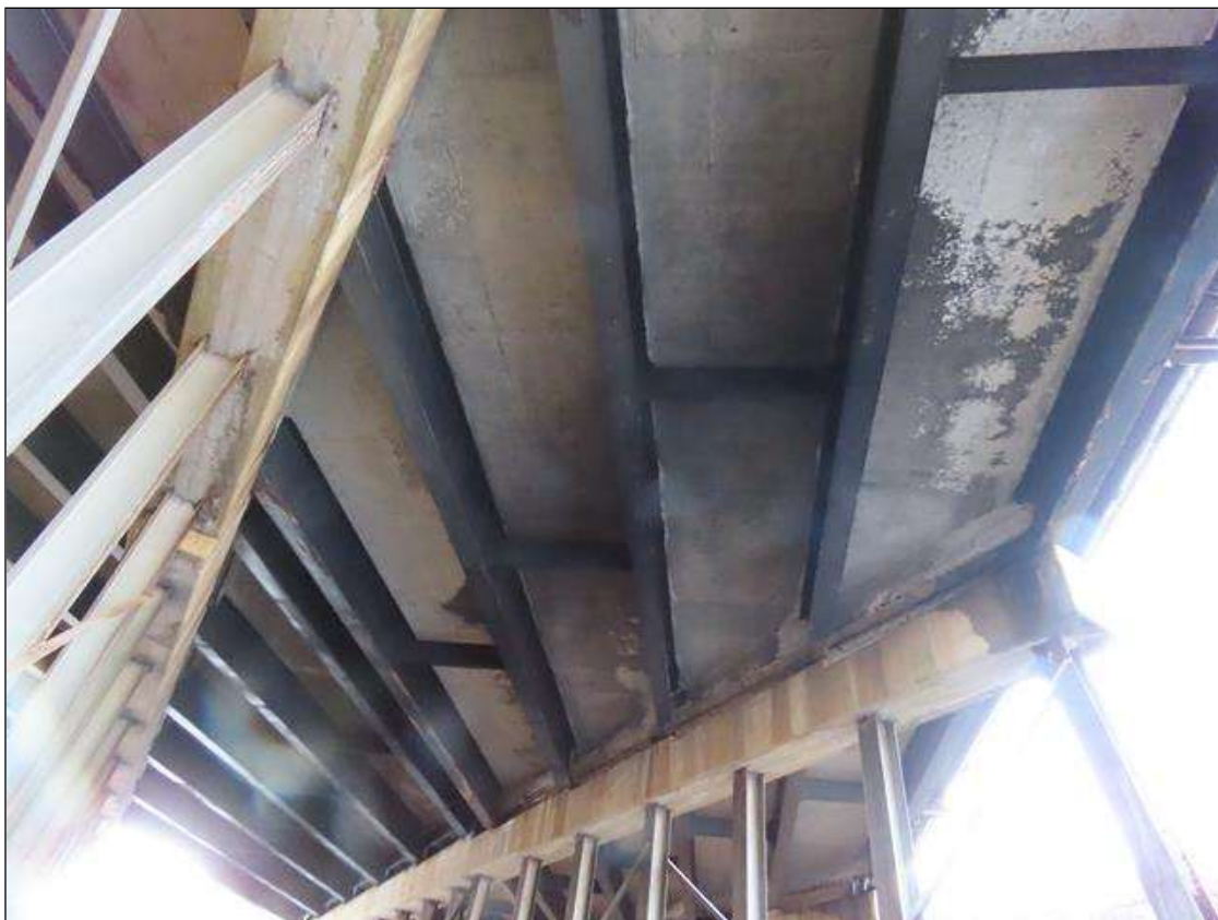
TYP. SUPERSTRUCTURE, SPAN 3 LOOKING AHEAD
