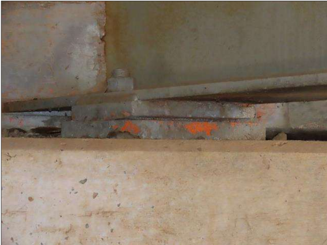
TYP. BEARING AT END BENT 1, BEAM 1 (BEAM 2-6 SIMILAR)
