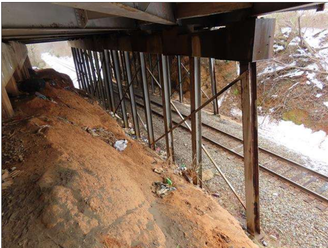
BENT 2, NEAR SIDE
