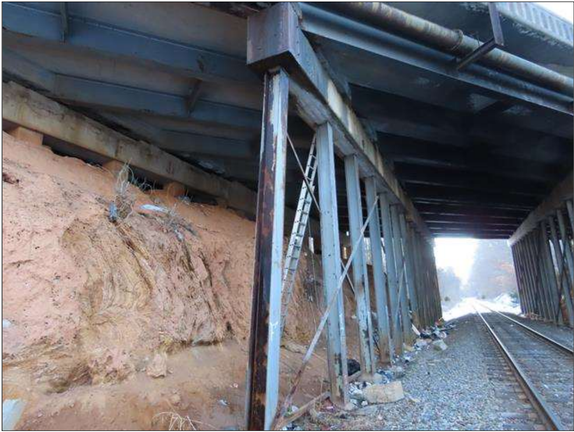
BENT 2, FAR SIDE
