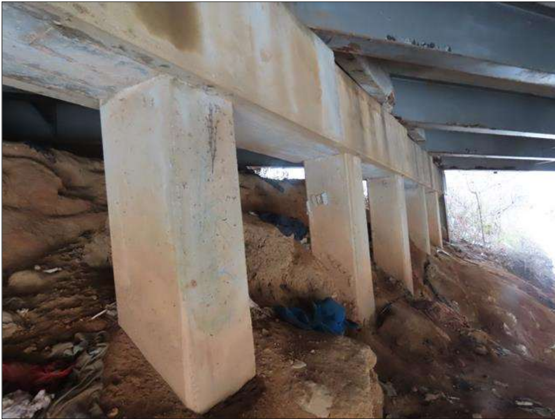
BENT 4 CAP, RIGHT SIDE
