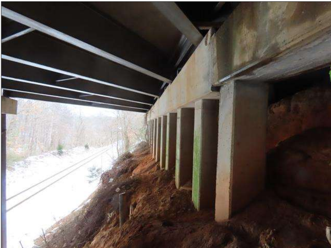
BENT 4 CAP, LEFT SIDE
