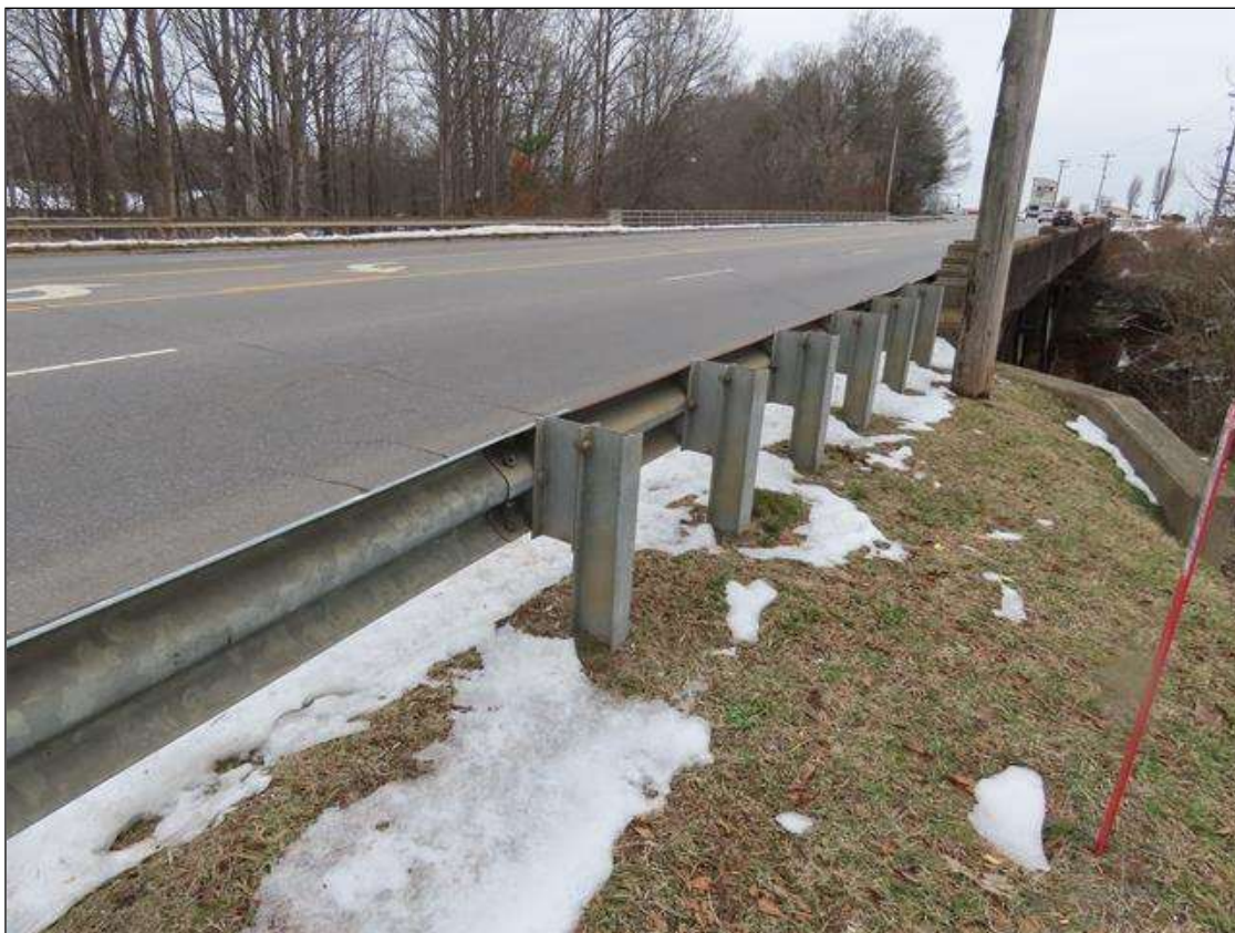
GUARDRAIL POST SPACING / TRANSITION AT NEAR RIGHT
