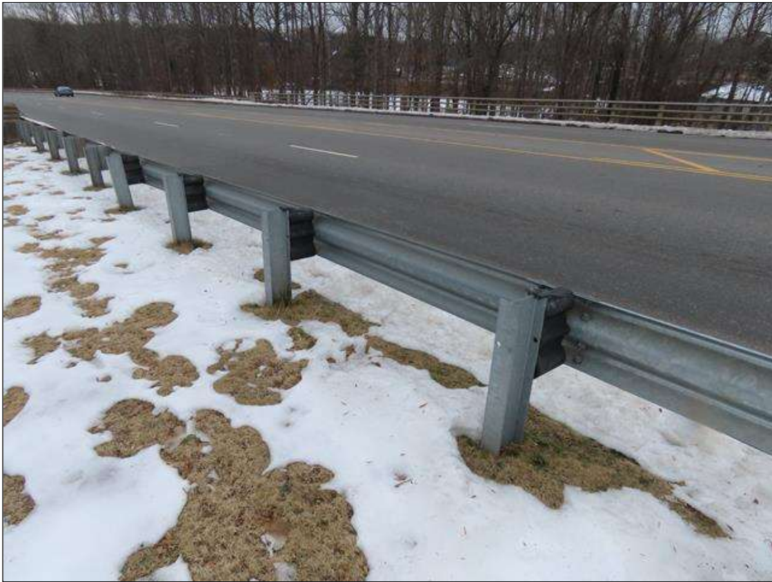
TYP. GUARDRAIL POST SPACING, FAR RIGHT
