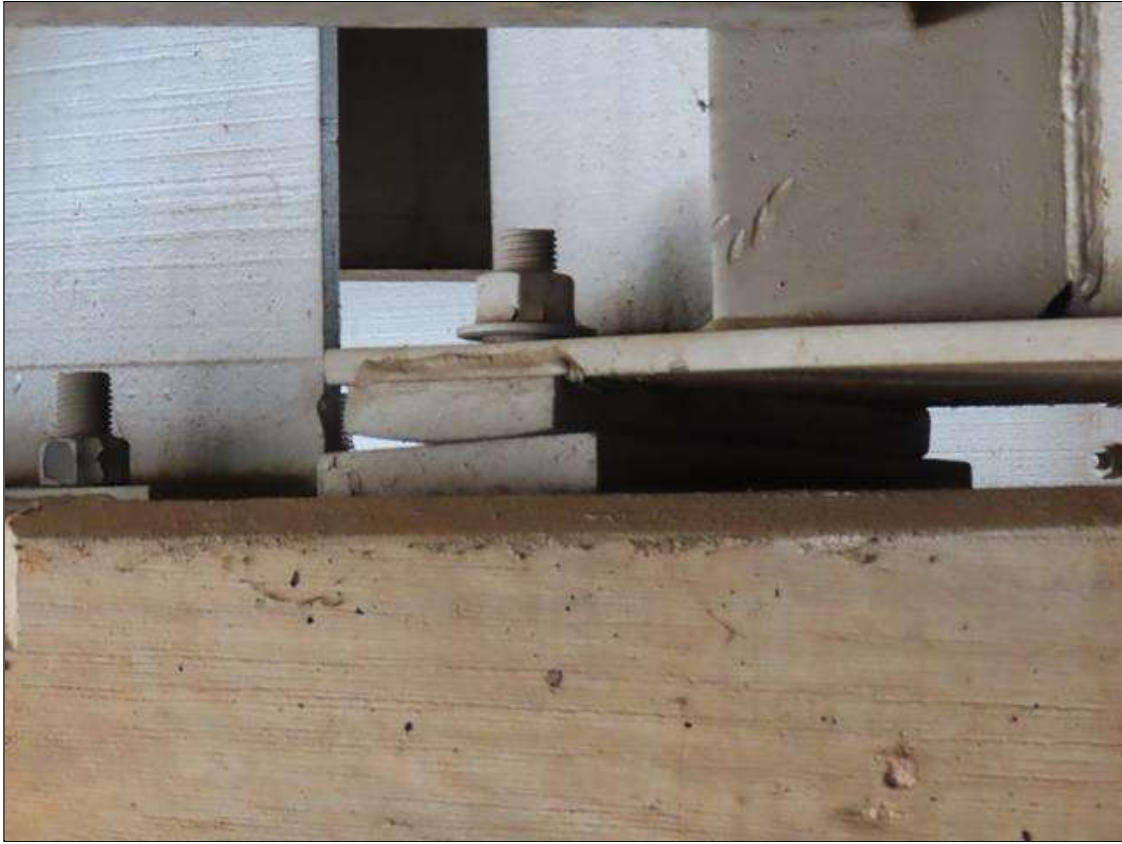
TYP. BEARING AT BENT 1, BEAM 2 (BEAM 1-6 SIMILAR)
