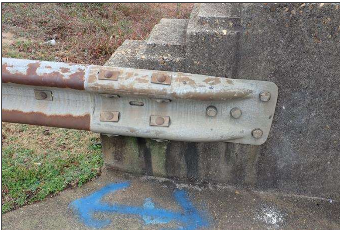
southeast guardrail attachment
