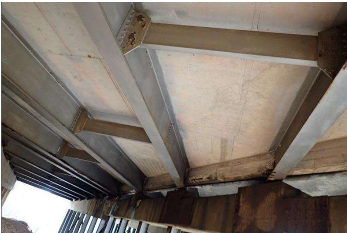
superstructure underside, span 2
