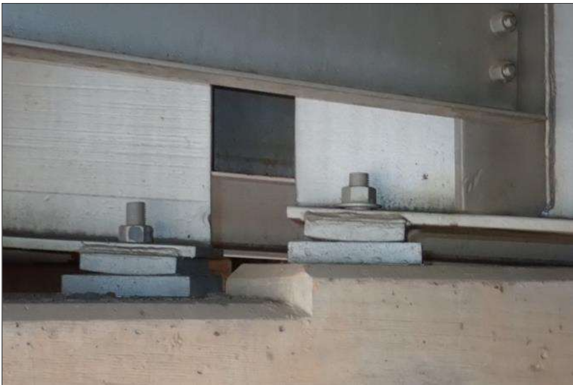
interior bearing assembly, bent 1, beams 1-7
