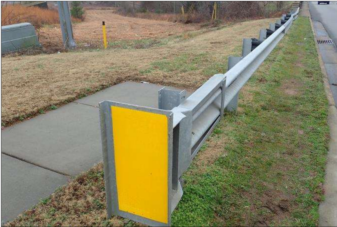
southeast guardrail and termination
