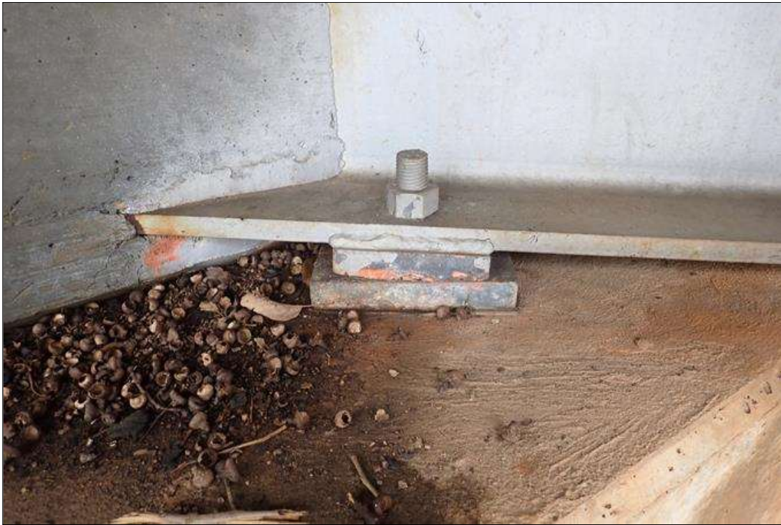
end bearing assembly, end bent 2
