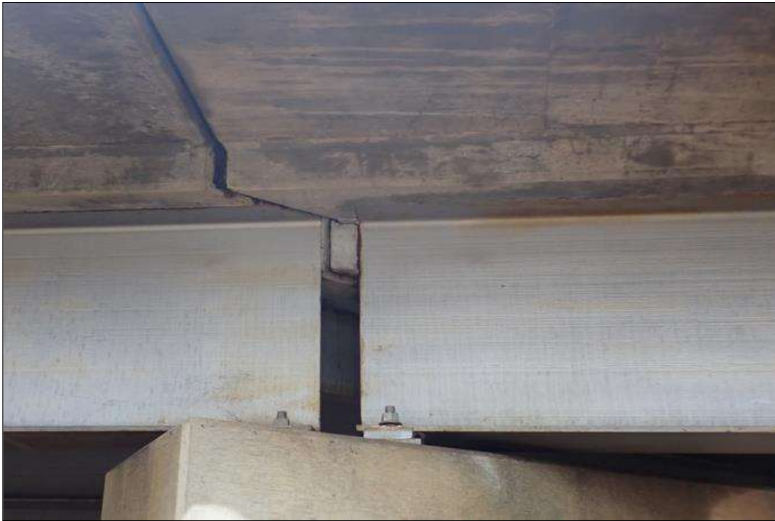
beams over bent 1, beams 1-7
