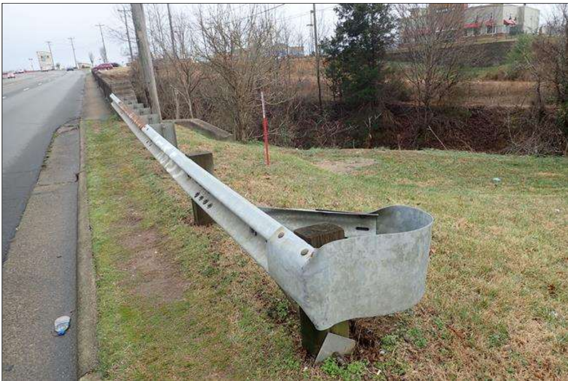
southwest guardrail and termination
