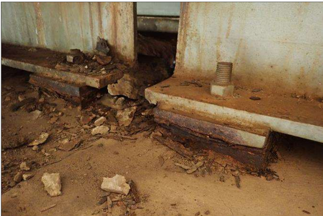
interior bearing assembly, bent 1, beams 8-11
