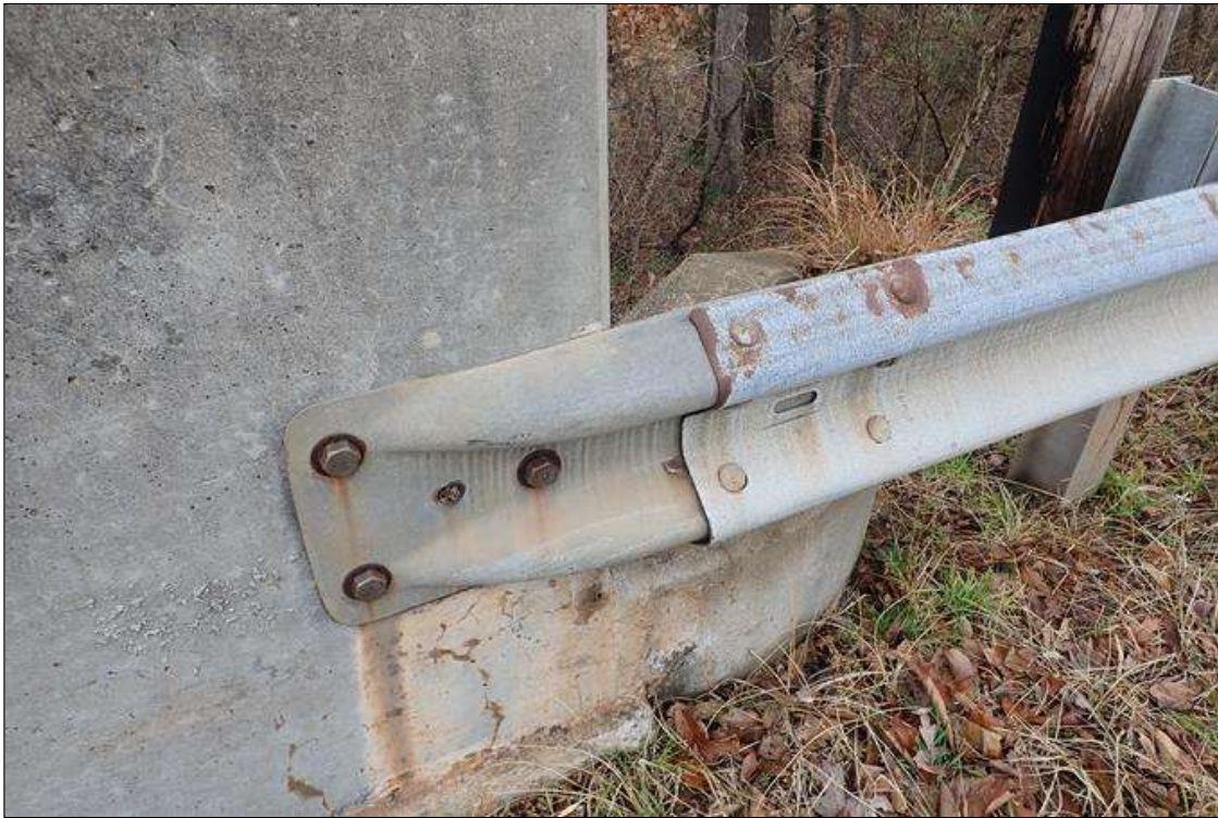
northeast guardrail attachment
