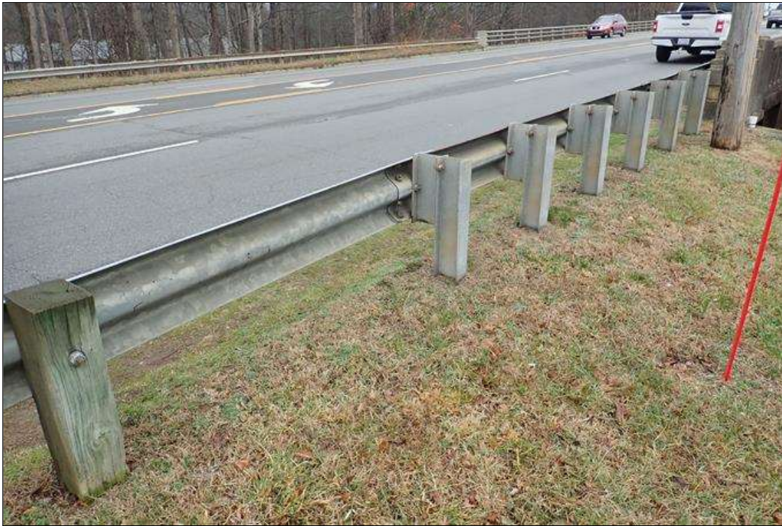
southwest guardrail transition
