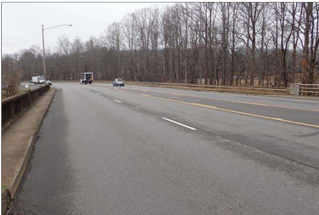
west approach looking west
