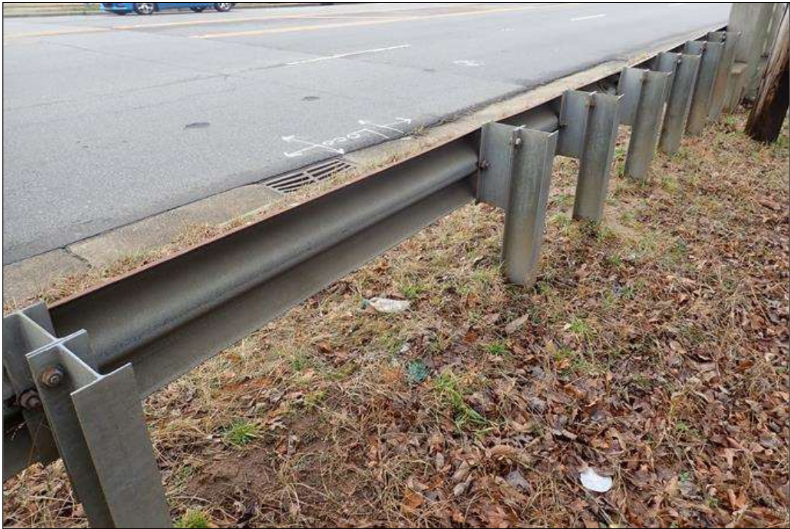
northeast guardrail transition
