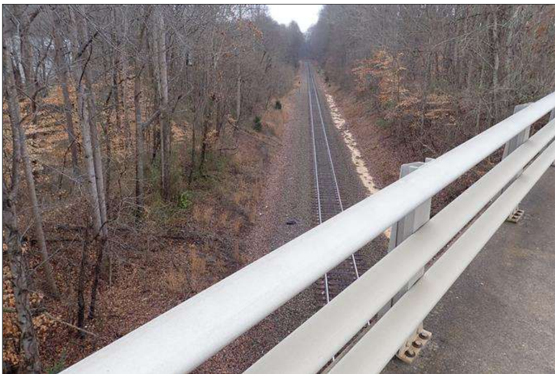
tracks looking north, span 3
