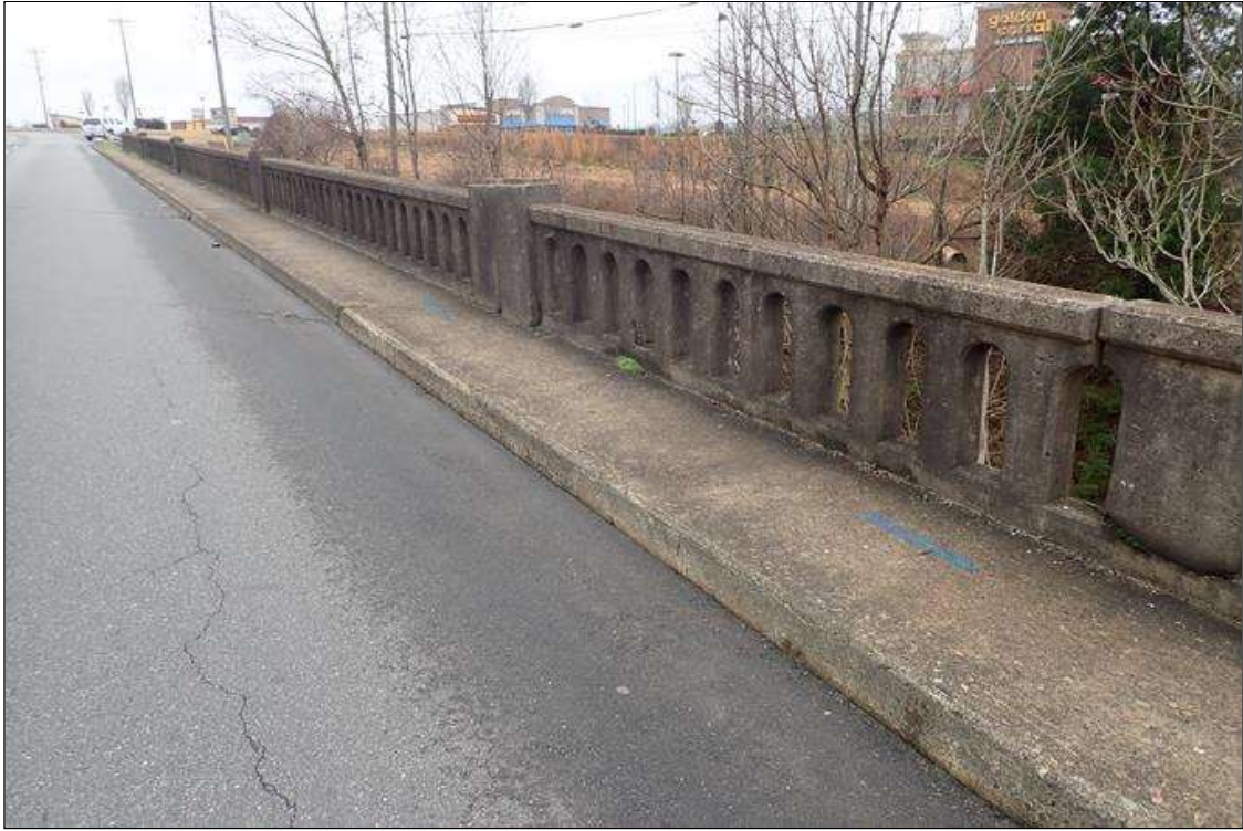
right bridge rail
