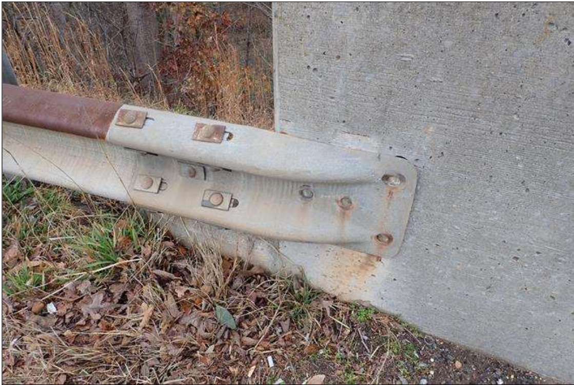
northwest guardrail attachment
