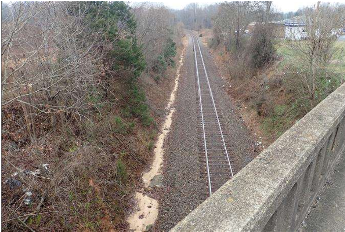
tracks looking south, span 3
