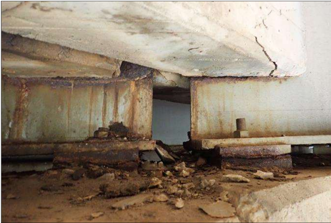
beams over bent 1, beams 8-11
