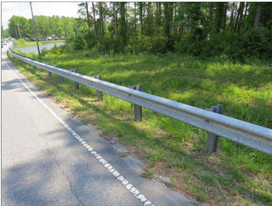
TYPICAL GUARDRAIL POST SPACING, FAR LEFT
