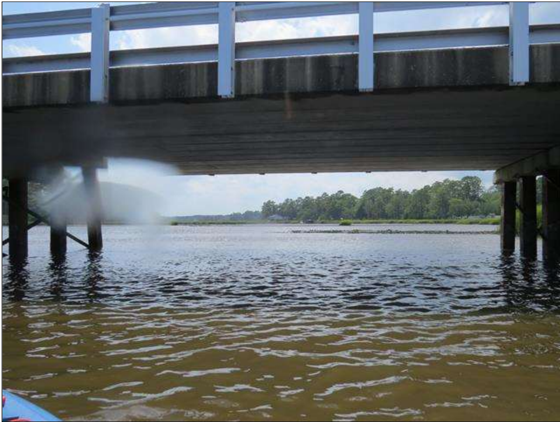
LOOKING DOWNSTREAM THROUGH SPAN 3
