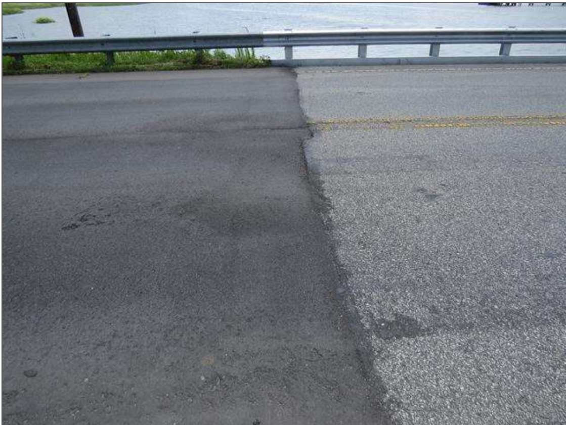
JOINT 1 OVER END BENT 1, LOOKING LEFT
