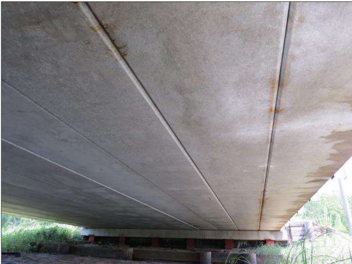
TYPICAL SUPERSTRUCTURE, SPAN 1
