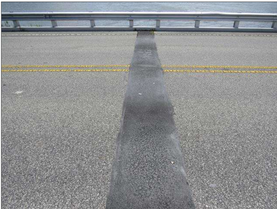
TYPICAL ASPHALT PLUG JOINT, JOINT 1 AT BENT 1
