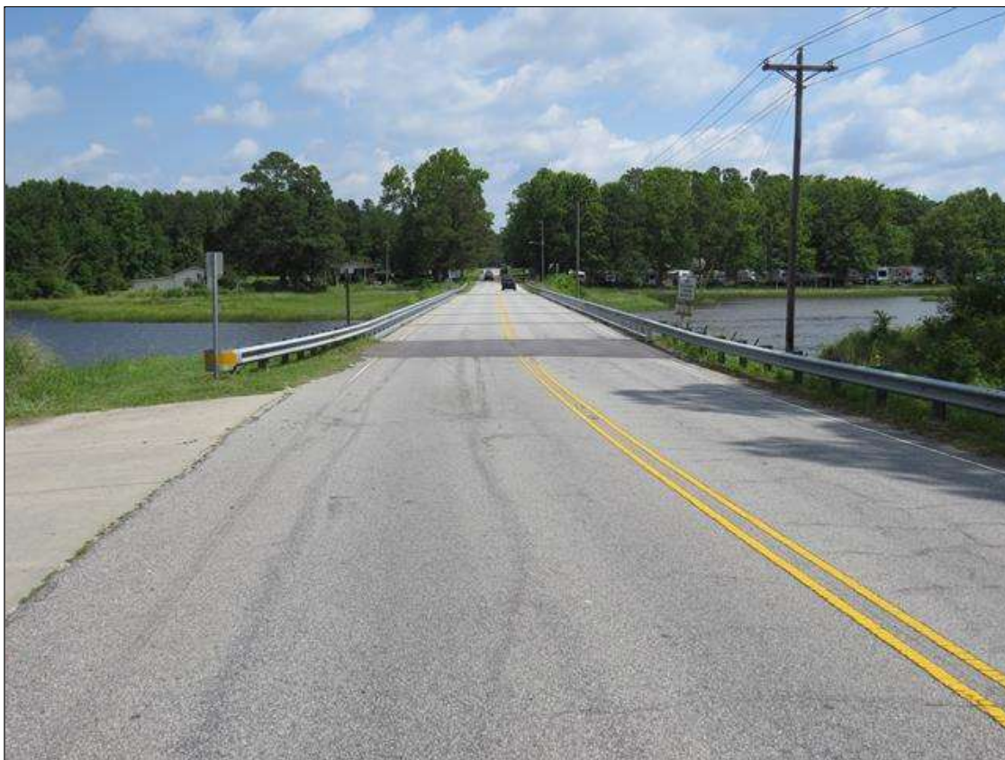
LOOKING STATIONS BACK - WEST
