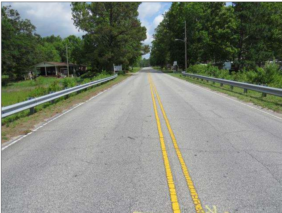
LOOKING BACK FROM BRIDGE
