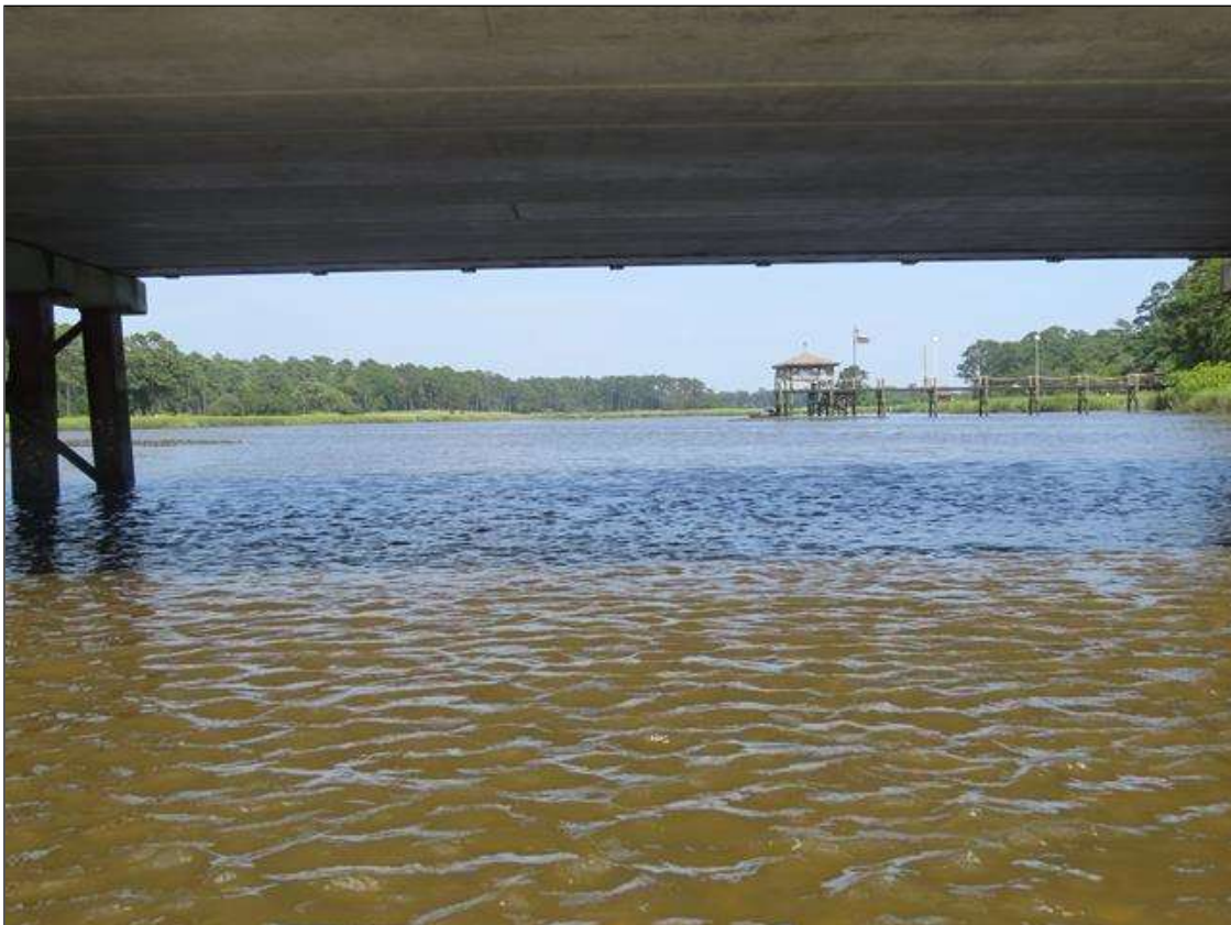
LOOKING DOWNSTREAM THROUGH SPAN 4
