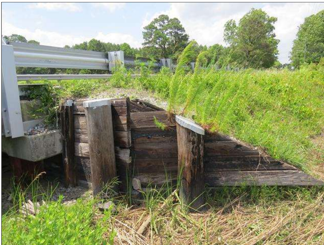
NEAR LEFT WING WALL
