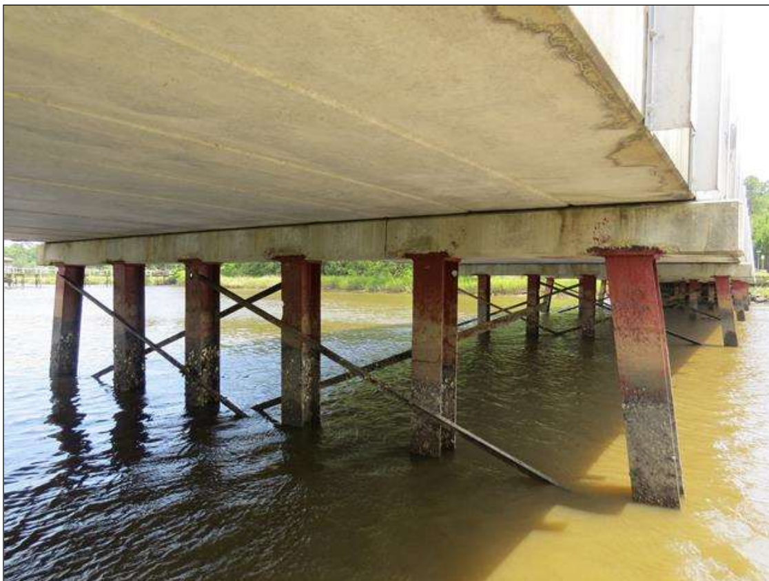
BENT 2 - NEAR FACE
