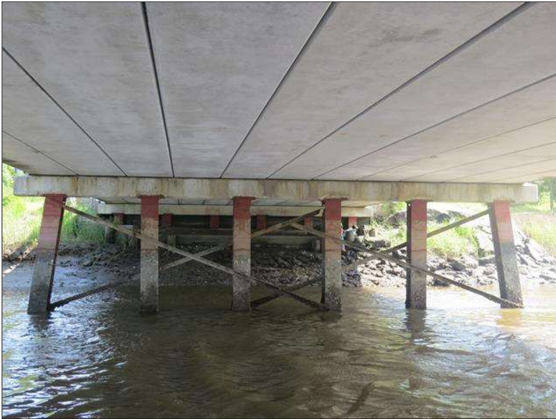
BENT 6, NEAR FACE
