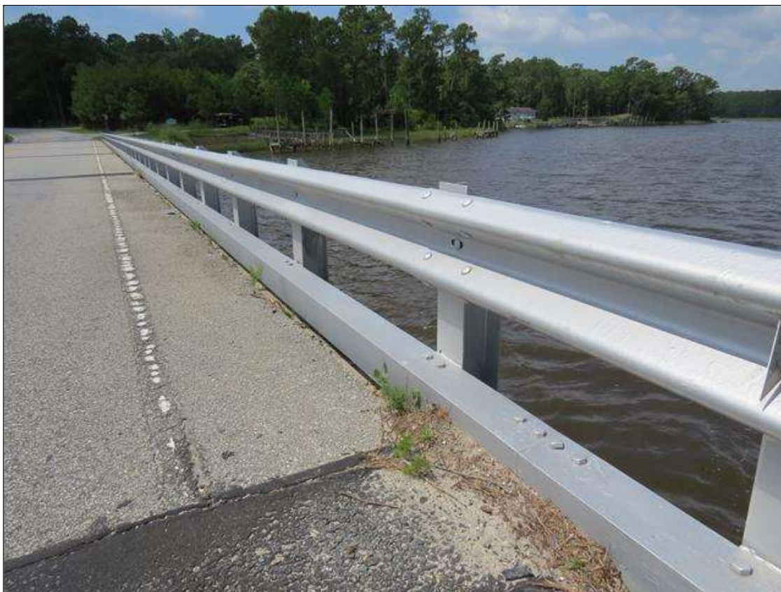
TYPICAL GUARDRAIL, LOOKING AHEAD AT BENT 2
