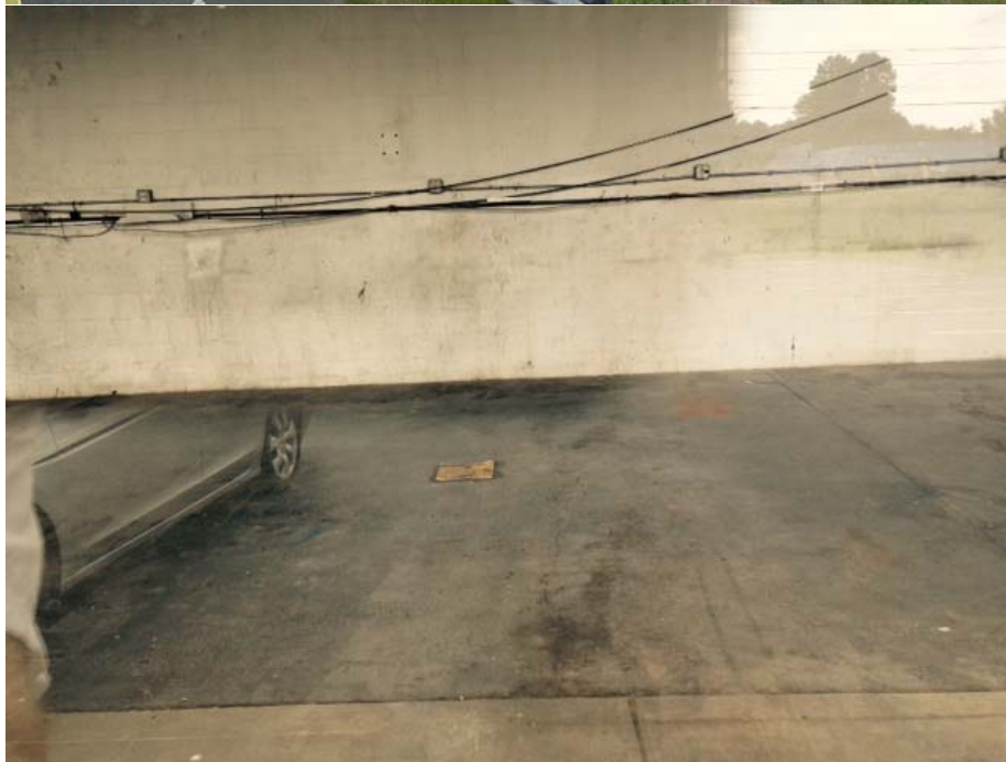
View north-northeastward (Google Streetview c. 2015)
