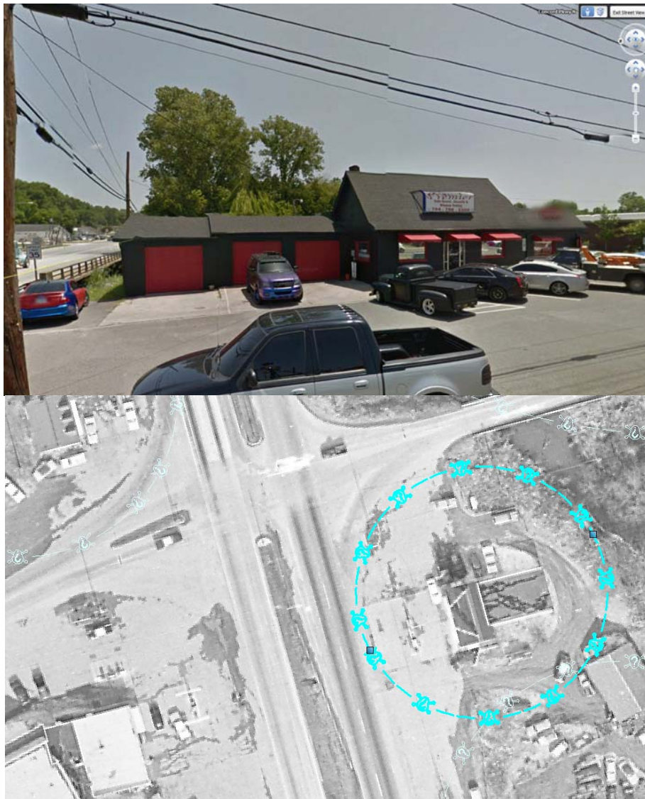
First Image Streetview c. 2015 view eastward Image c. 2015; Second image NCDOT Historical Aerial 2/1/1961 Mission 129, exposure 13 (top of page is northward)
