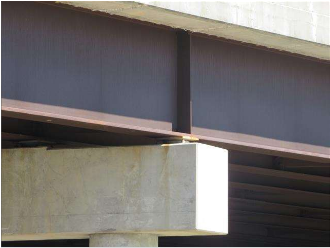
BEAM OVER CAP AT BENT 1
