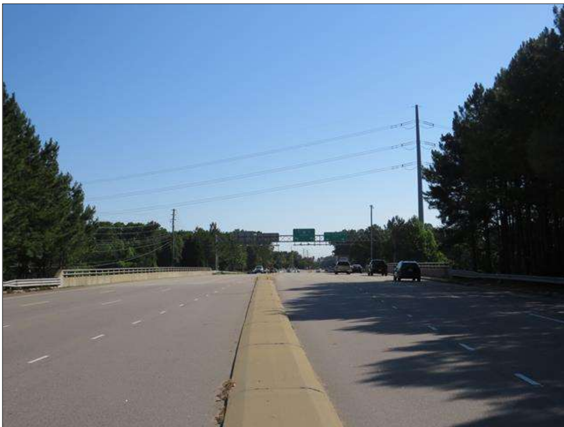
SOUTH APPROACH LOOKING NORTH
