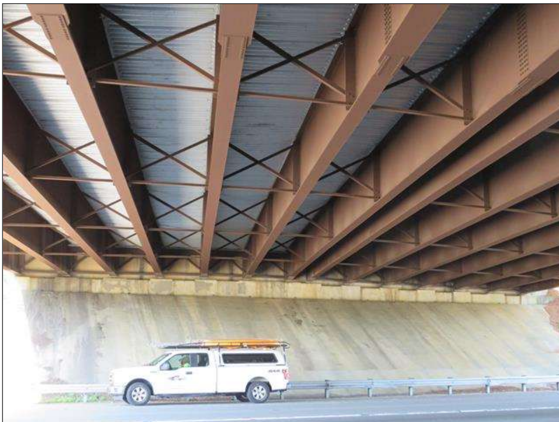
END BENT 1 LOOKING SOUTH
