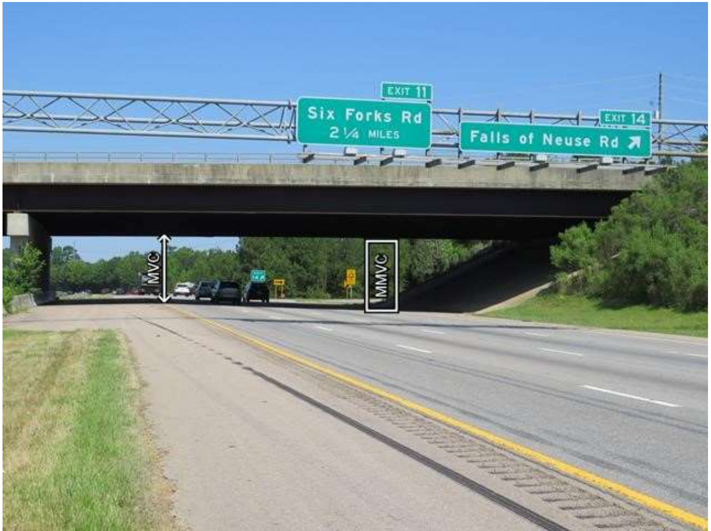
SPAN 2 OPENING LOOKING WEST
