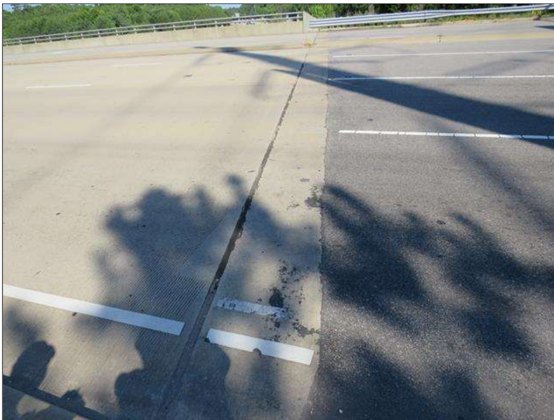
END BENT 2 JOINT
