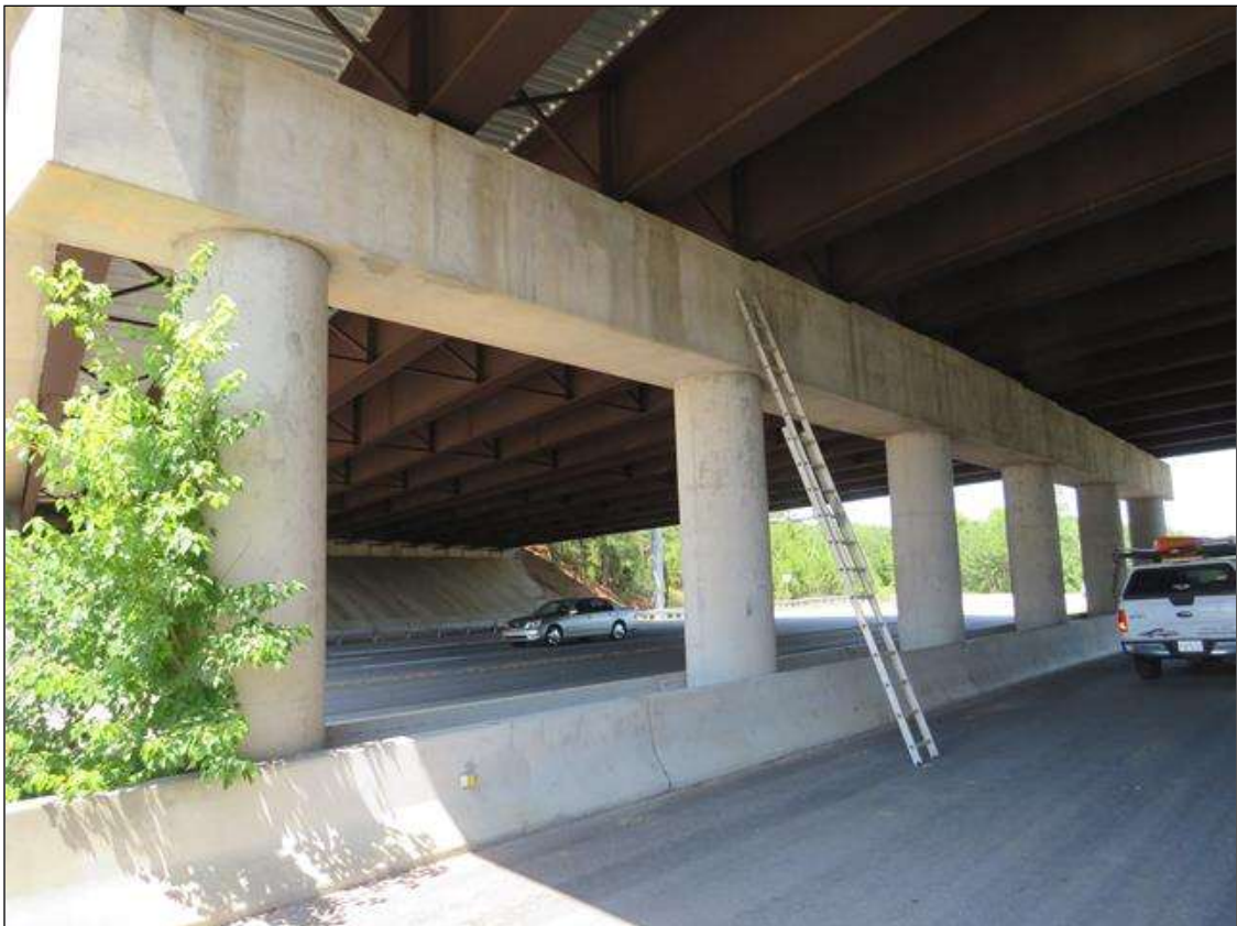
BENT 1 LOOKING SOUTH
