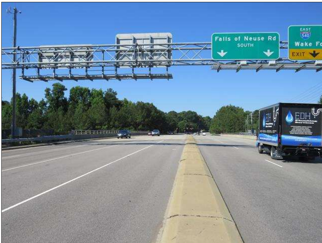
NORTH APPROACH LOOKING SOUTH
