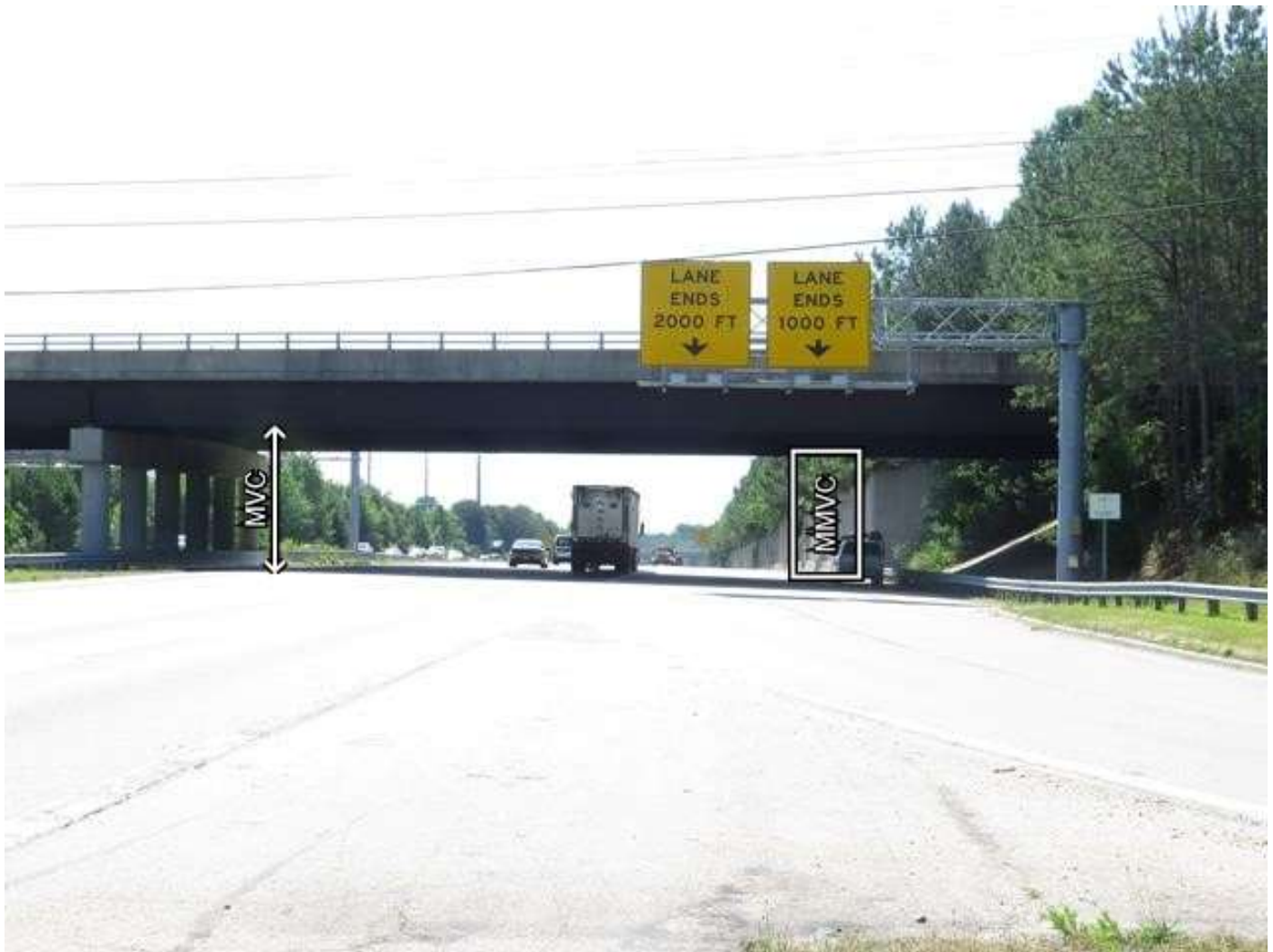
SPAN 1 OPENING LOOKING EAST
