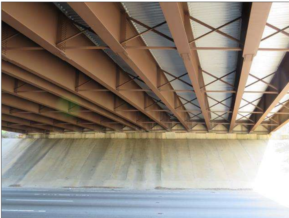
END BENT 2 LOOKING NORTH
