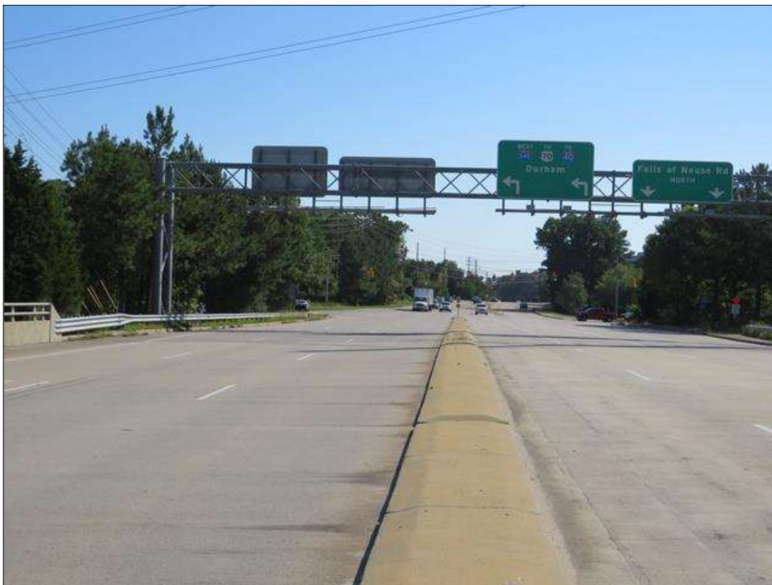
NORTH APPRAOCH LOOKING NORTH
