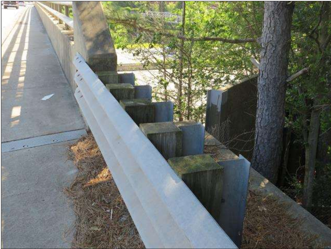
GUARDRAIL POST SPACING 1.55' AT BRIDGE
