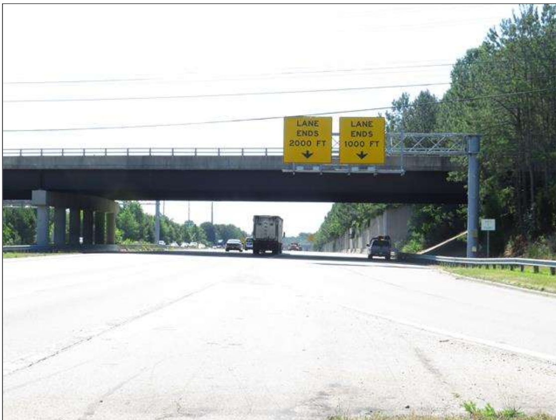
SPAN 1 OPENING LOOKING EAST
