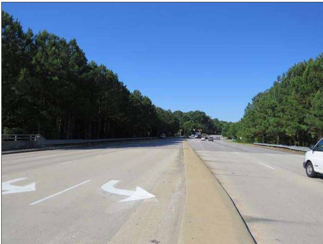
SOUTH APPROACH LOOKING SOUTH
