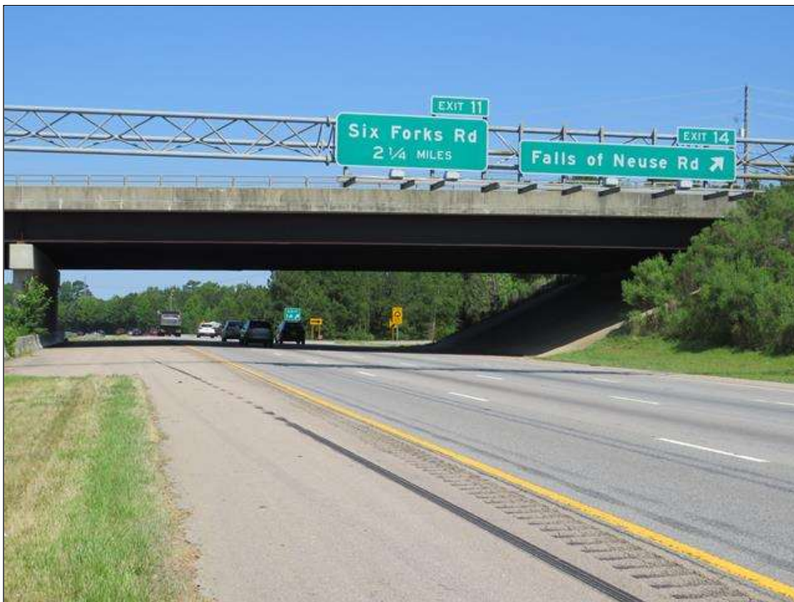
SPAN 2 OPENING LOOKING WEST
