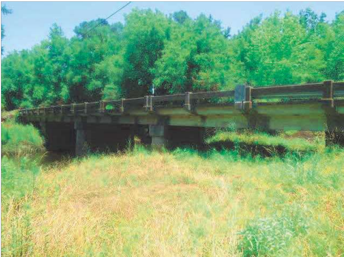
DOWNSTREAM PROFILE, LOOKING SOUTHEAST
