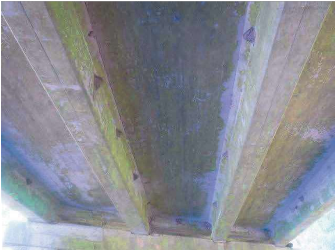
SPAN 2 UNDERDECK, OTHERS SIMILAR
