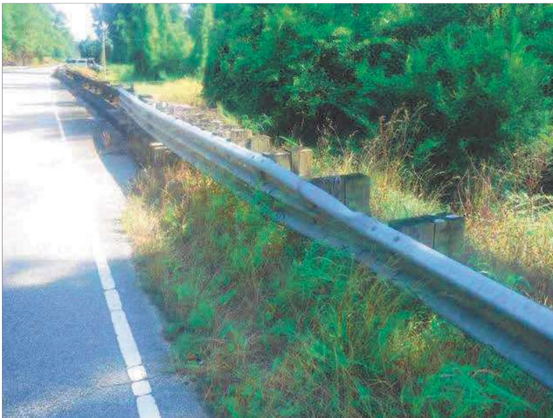
NORTHEAST APPROACH GUARDRAIL POST SPACING AT BRIDGE, OTHERS SIMILAR
