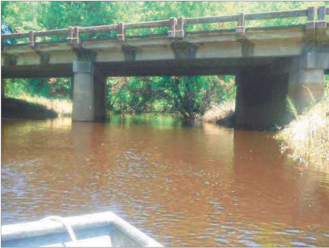
SPAN 2 DOWNSTREAM PROFILE, LOOKING SOUTH
