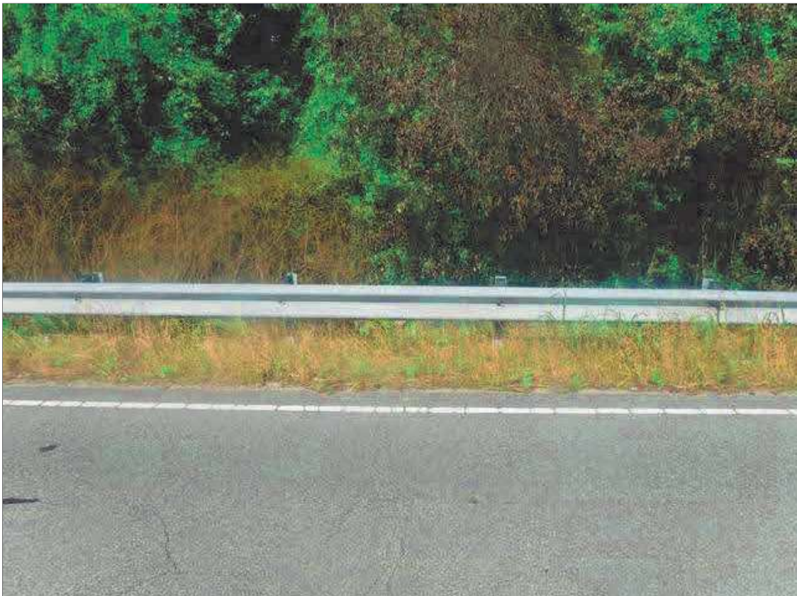
SOUTHEAST APPROACH GUARDRAIL POST SPACING AT MID LENGTH, OTHERS SIMILAR
