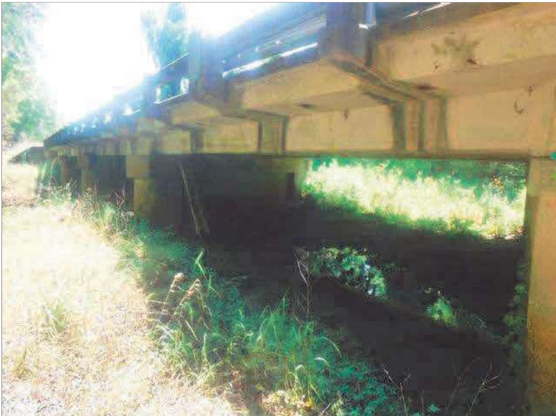
UPSTREAM PROFILE, LOOKING NORTHWEST
