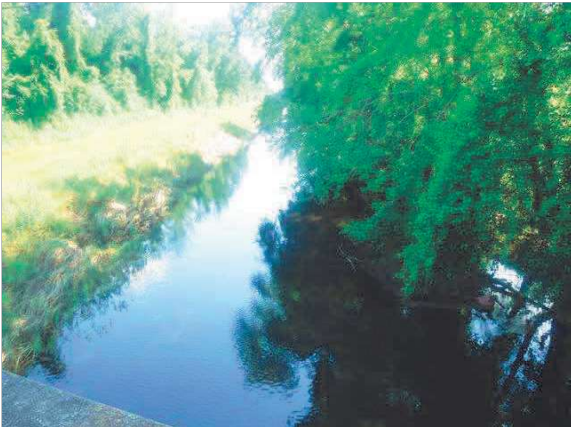
LOOKING DOWNSTREAM, NORTH
