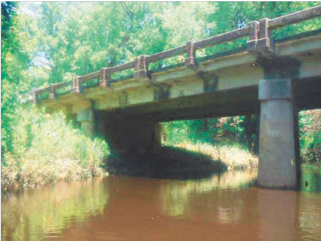
SPAN 3 DOWNSTREAM PROFILE, LOOKING SOUTHEAST
