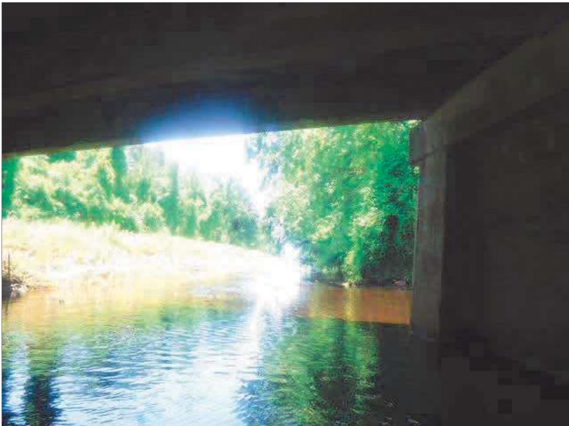
LOOKING DOWNSTREAM, NORTHWEST
