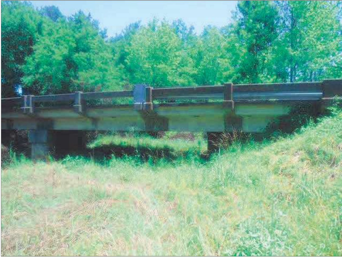
SPAN 1 DOWNSTREAM PROFILE, LOOKING SOUTH
