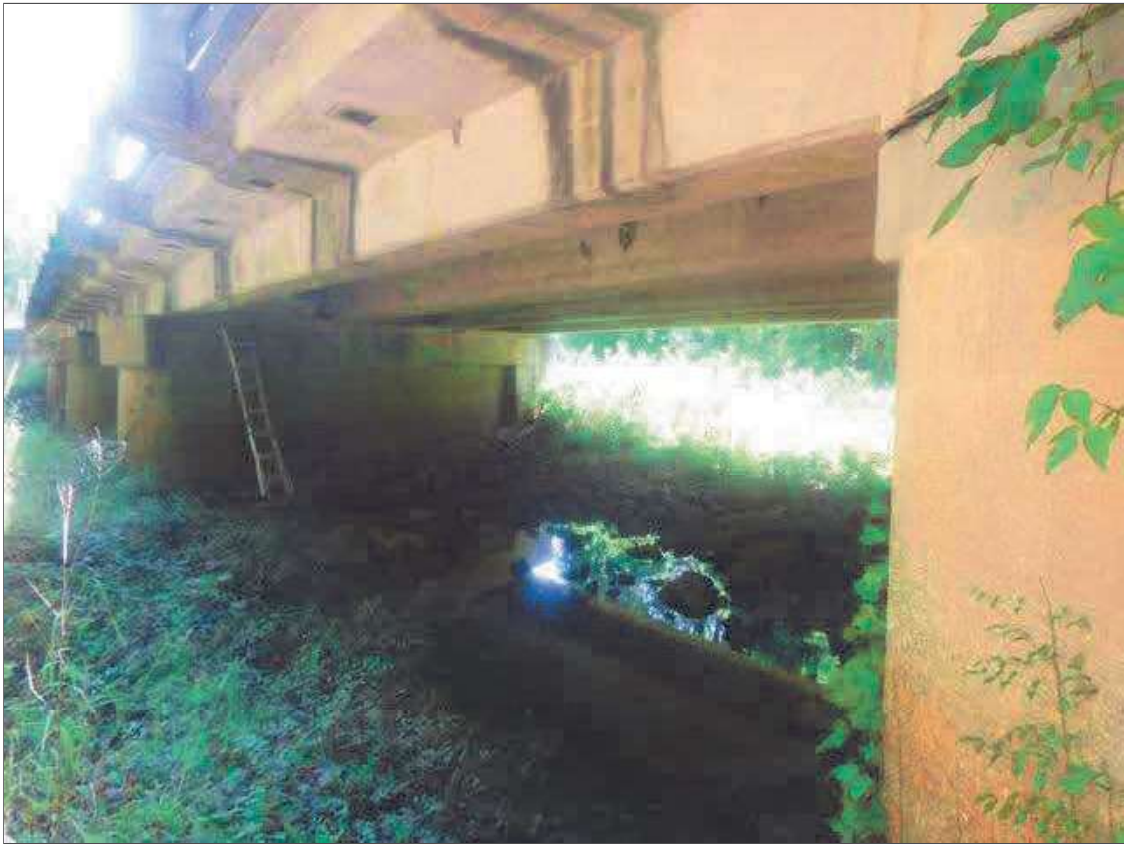
SPAN 4 UPSTREAM PROFILE, LOOKING NORTHWEST
