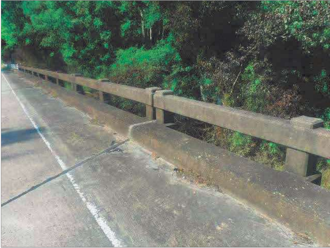
RIGHT RAIL, LEFT RAIL SIMILAR
