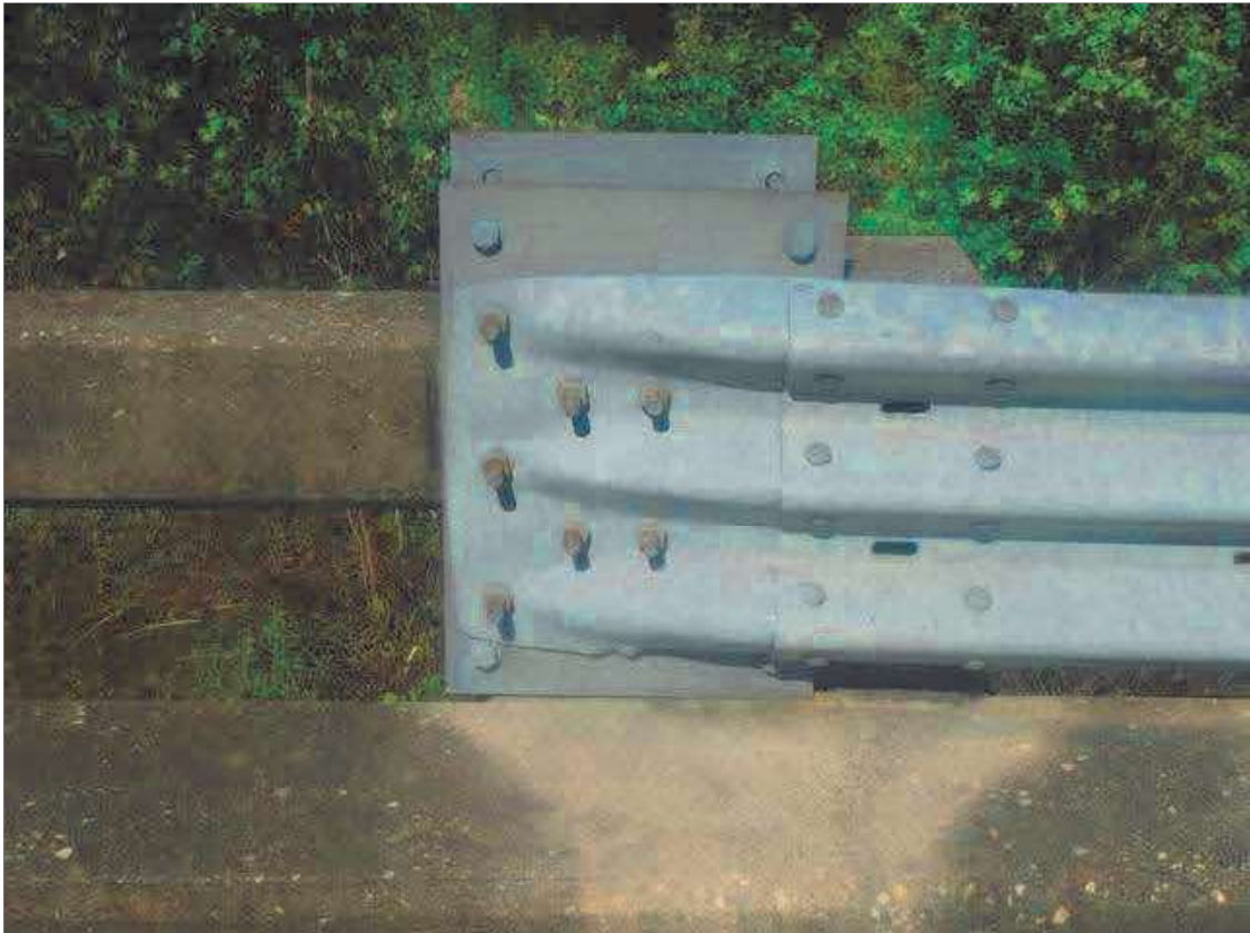
GUARDRAIL TO BRIDGE RAIL CONNECTION AT SOUTHWEST CORNER, OTHERS SIMILAR
