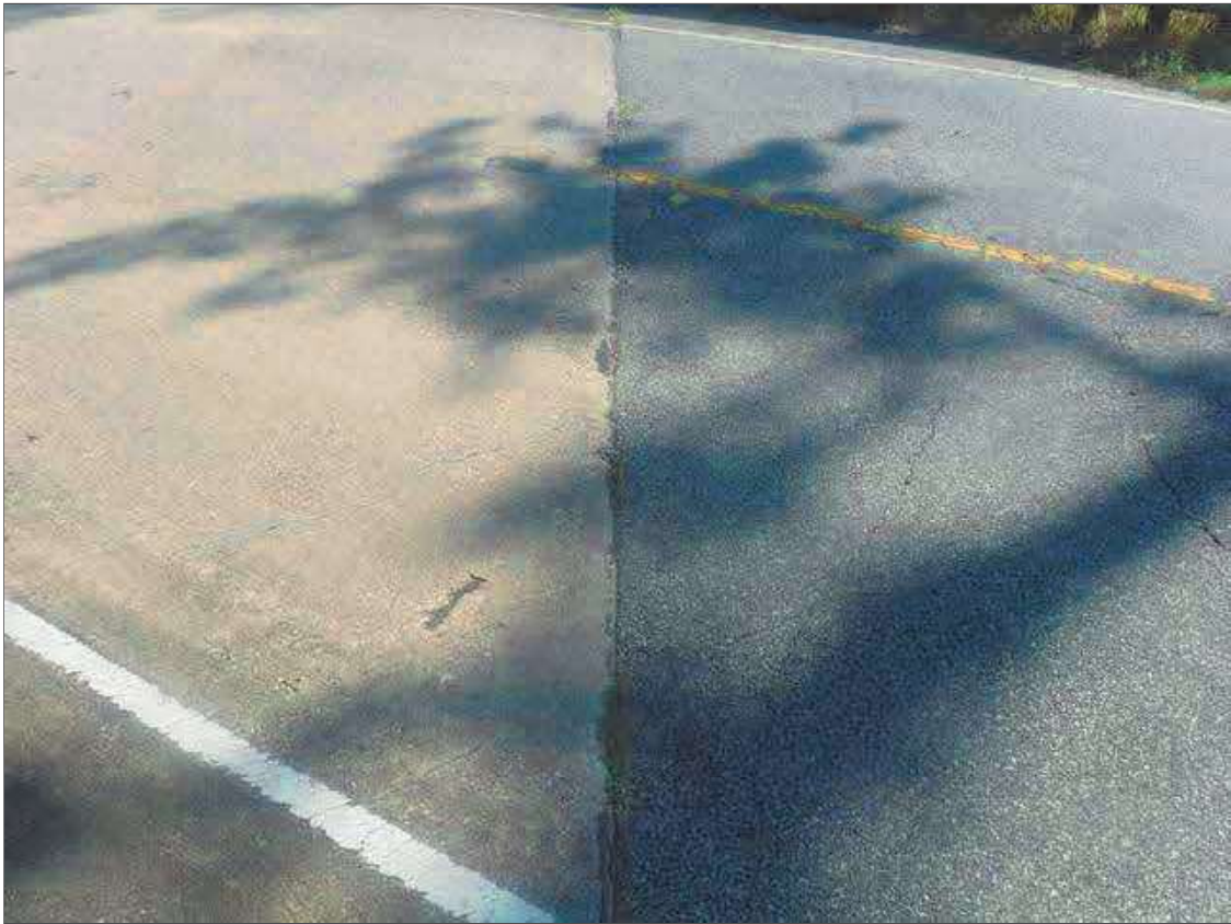
TRANSITION ALONG ABUTMENT 2 FILL FACE, TRANSITION ALONG ABUTMENT 1 FILL FACE SIMILAR
